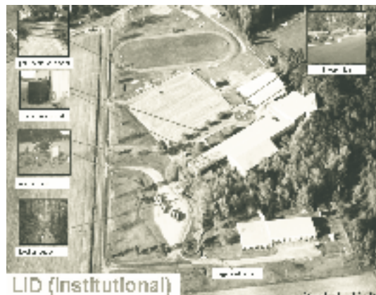
LID: Institutional Retrofit in Williamston, NC
