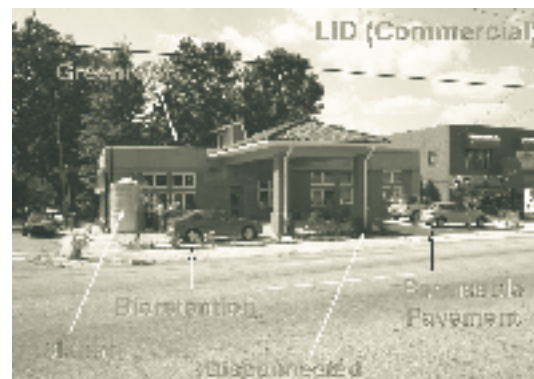
LID: Commercial Project in Raleigh, NC
