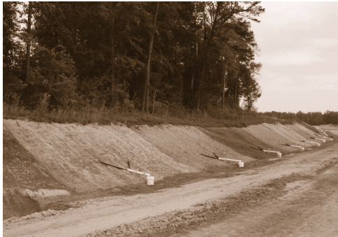
Figure 1. Plots at Site 2 showing runoff collection system.
