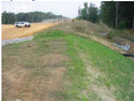
Fig. 5. Road section showing bank created by fill.
