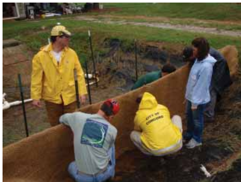
Figure 1. Installation of coir baffles into a sediment basin.
