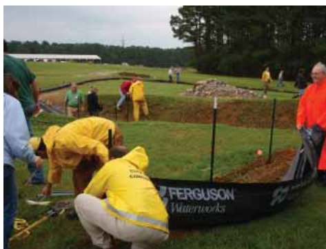
Figure 2. Installation of Silt Fence
