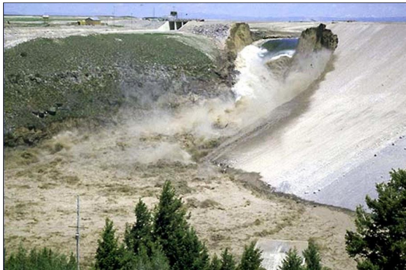
Failure of Teton Dam (Idaho) from seepage (1976)
