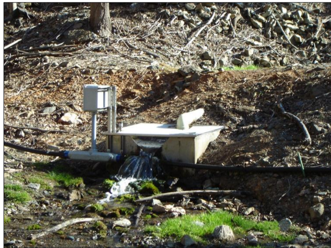
Seepage weir and collection box
