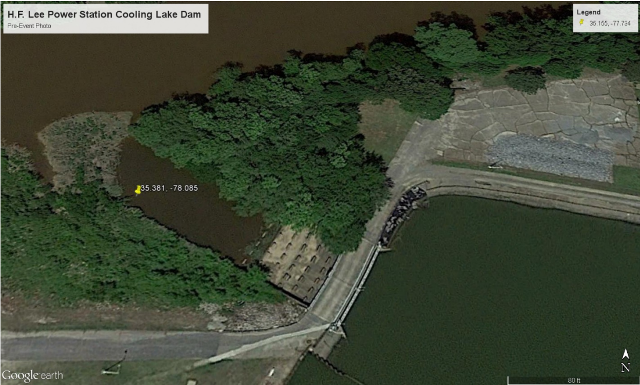
Figure A19.1: H.F. Lee Power Station Cooling Lake Dam pre-event photo; Credit: Google Maps
