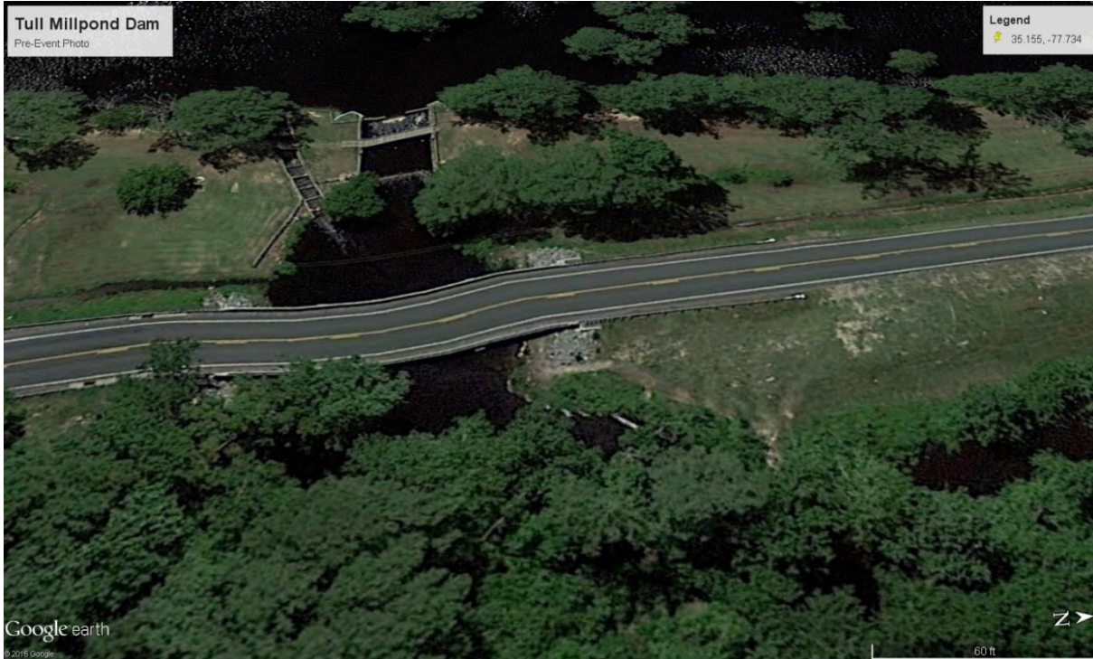
Figure A15.1: Tull Millpond Dam pre-event photo; Credit: Google Earth
