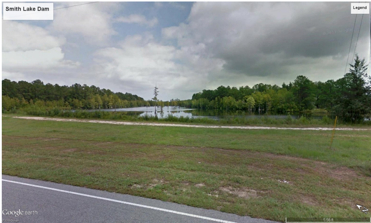
Figure A3.1: Smith Lake Dam pre-event image; Credit: 2016 Google Earth Streetview
