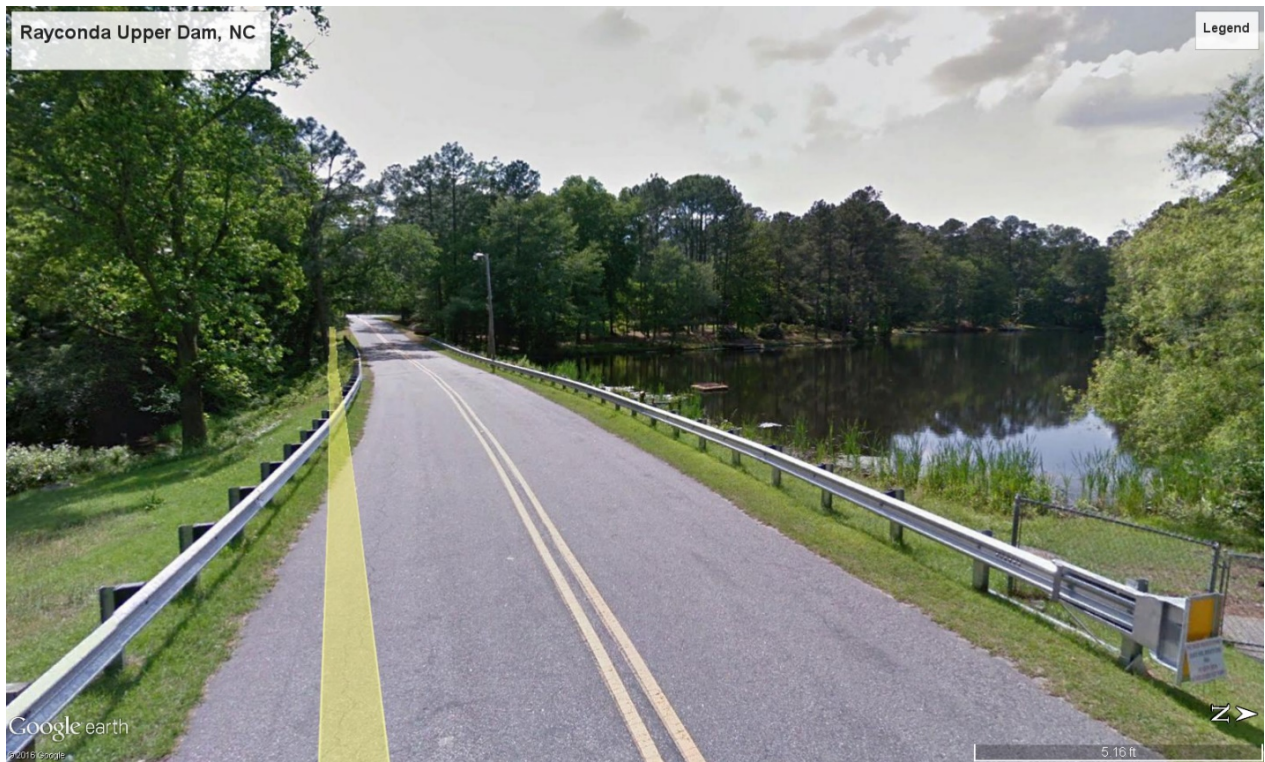
Figure A10.1: Rayconda Upper Dam pre-event photo; Credit: Google Maps Streetview
