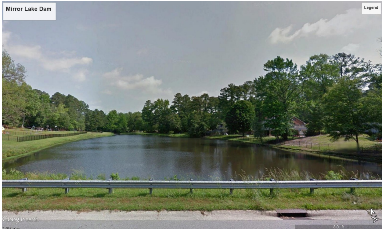
Figure A7.1: Mirror Lakes Dam pre-event image; Credit: 2016 Google Earth Streetview
