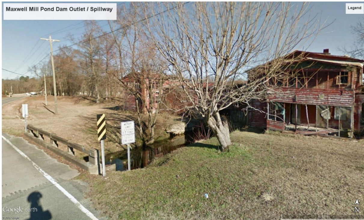
Figure A12.2: Maxwell Mill Pond Dam South spillway and Maxwell Mill Road pre-event photo; Credit: Google Maps Streetview
