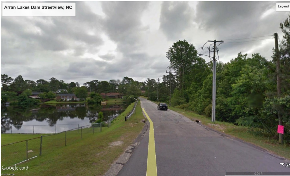
Figure A4.1: Arran Lakes Dam pre-event image; Credit: 2016 Google Earth Streetview
