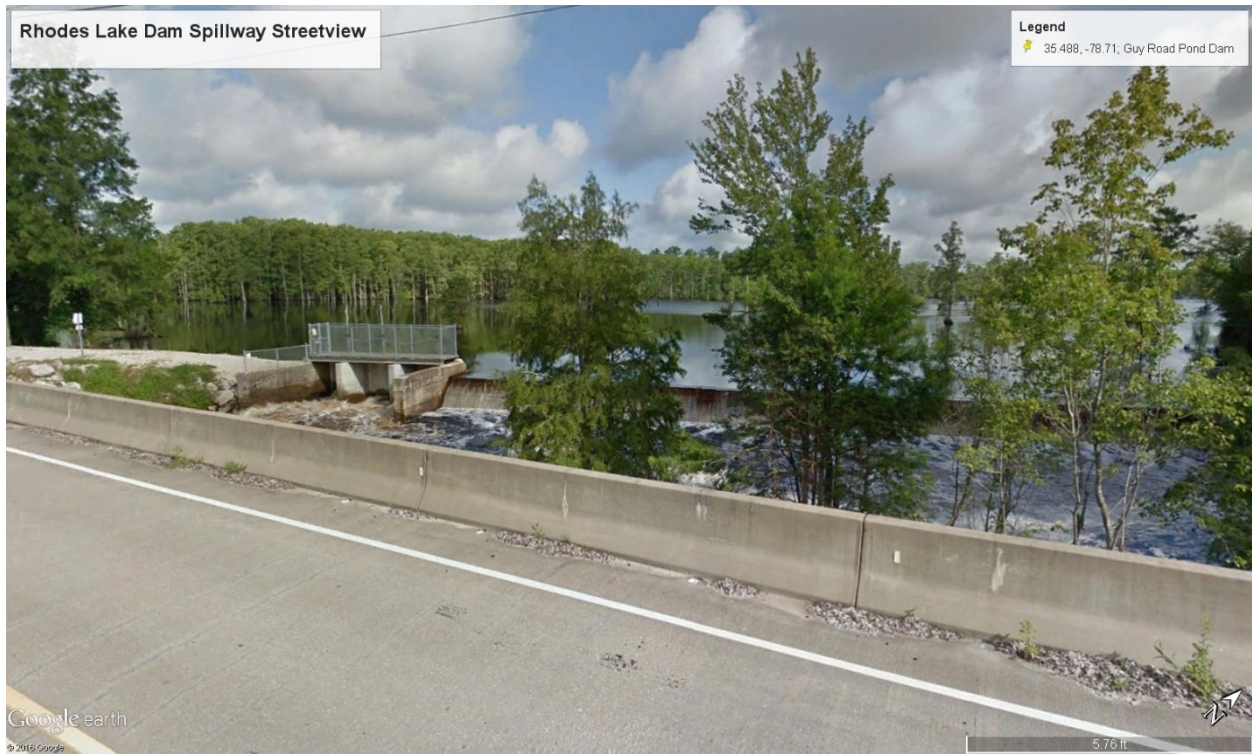
Figure A5.1: Rhodes Lake Dam Spillway pre-event photo; Credit: 2016 Google Earth Streetview
