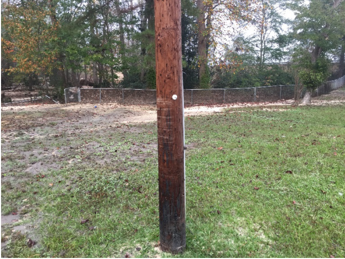
Photo of HWM3 at Fair mudline on power pole 479128301 in back yard of house at 1603 Greenock Ave., Fayetteville, NC. Marked with nail/hwm disc. Cumberland County, NC, 10/21/2016. Photograph by Chris Brown, USGS GA.
