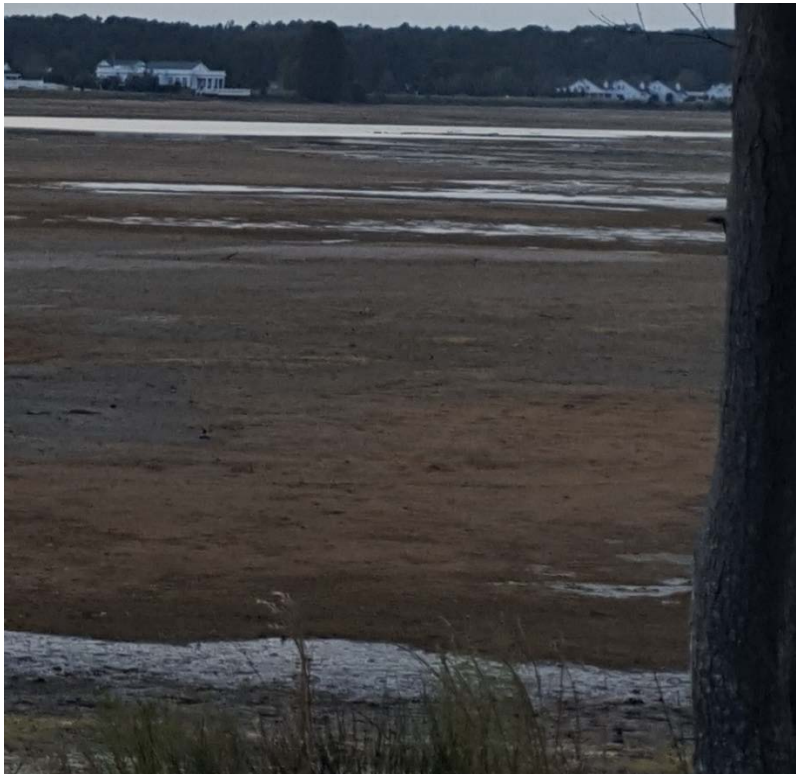
Figure 8.7 Woodlake Dam drained reservoir October 27, 2016; Credit: NC DEMLR
