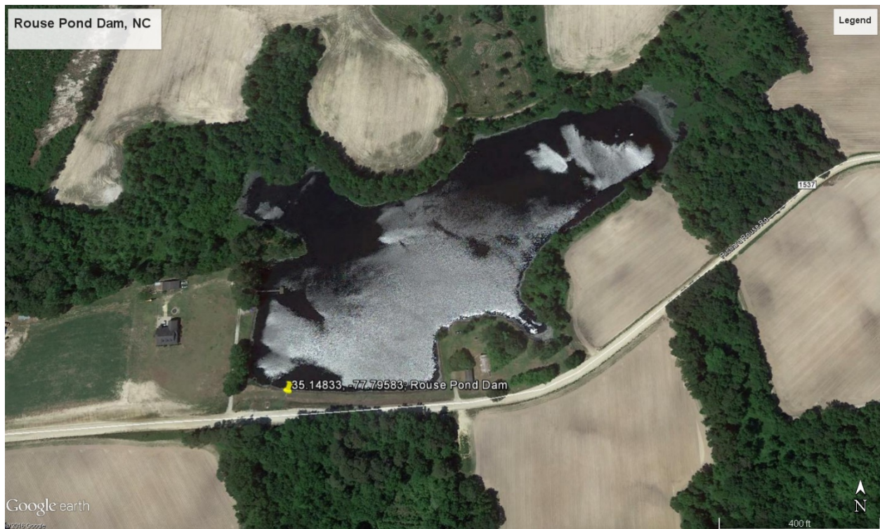
Figure 11.2: Rouse Pond Dam Overview Credit: Map data: 2016 Google; Google Earth
