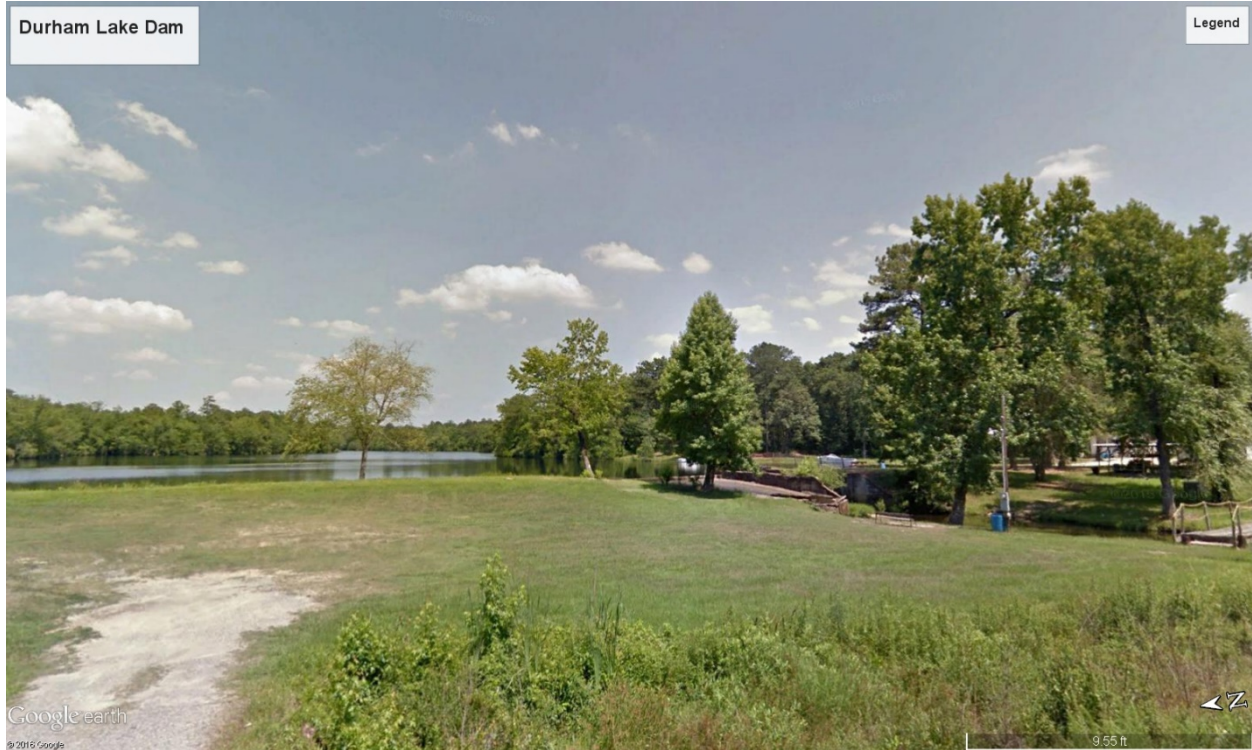
Figure A18.1: Durham Lake Dam pre-event image; Credit: 2016 Google Earth Streetview
