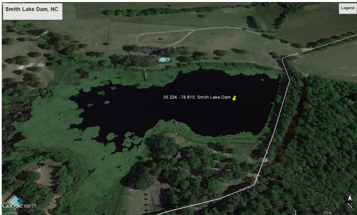
Figure A6.2: Smith Lake Dam Site Overview Credit: Map data: 2016 Google Earth
