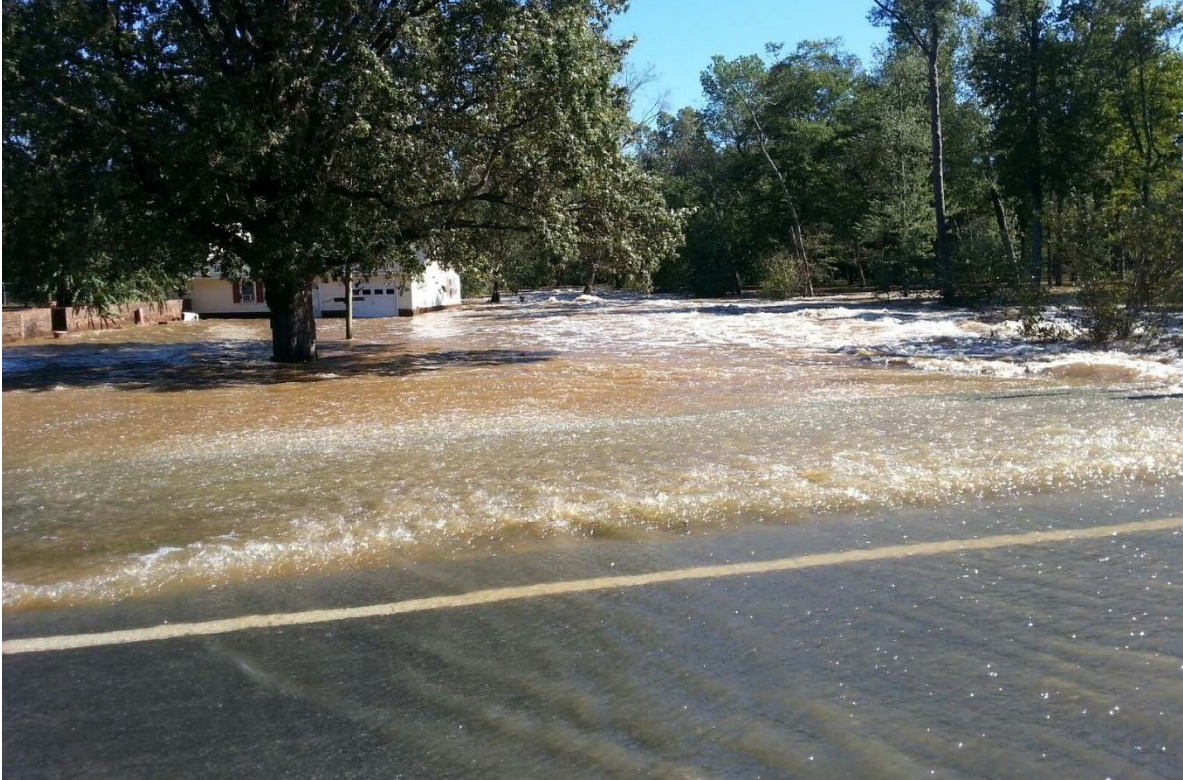
Figure 8.12 Consequences of Flooding and Lake Wilson Dam overtopping Credit: NC DEMLR
