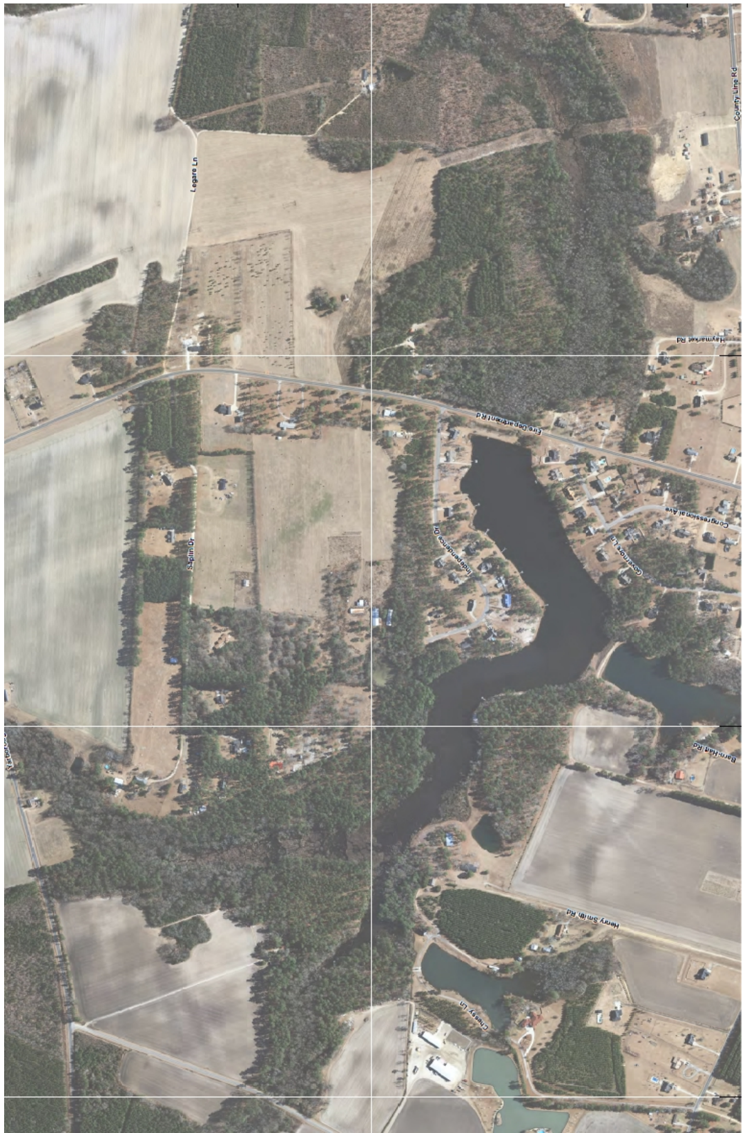
Figure A8.2: Mount Vernon Estates Dam in blue circle; FIRM cropped; FIRM details in spreadsheet above
