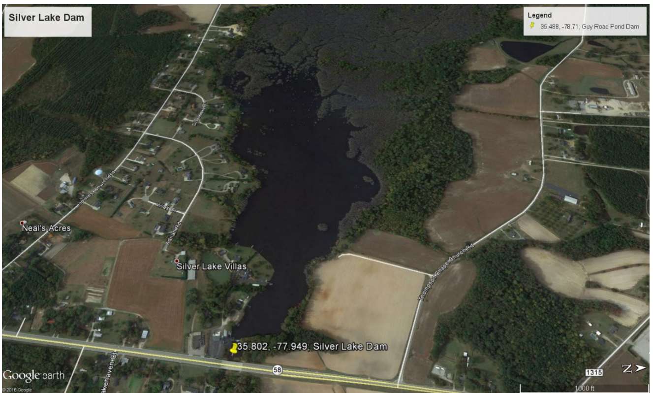
Figure A20.3: Silver Lake Dam Site Area Map Credit: Map data: 2016 Google; Google Earth
