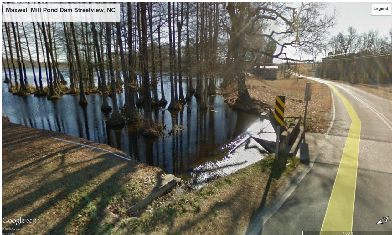
Figure A12.1: Maxwell Mill Pond Dam north spillway and Maxwell Road pre-event photo; Credit: Google Maps Streetview
