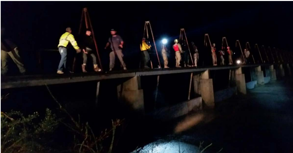
Figure 8.3 National Guard and others placing sandbags at Woodlake Dam Credit: NC DEMLR
