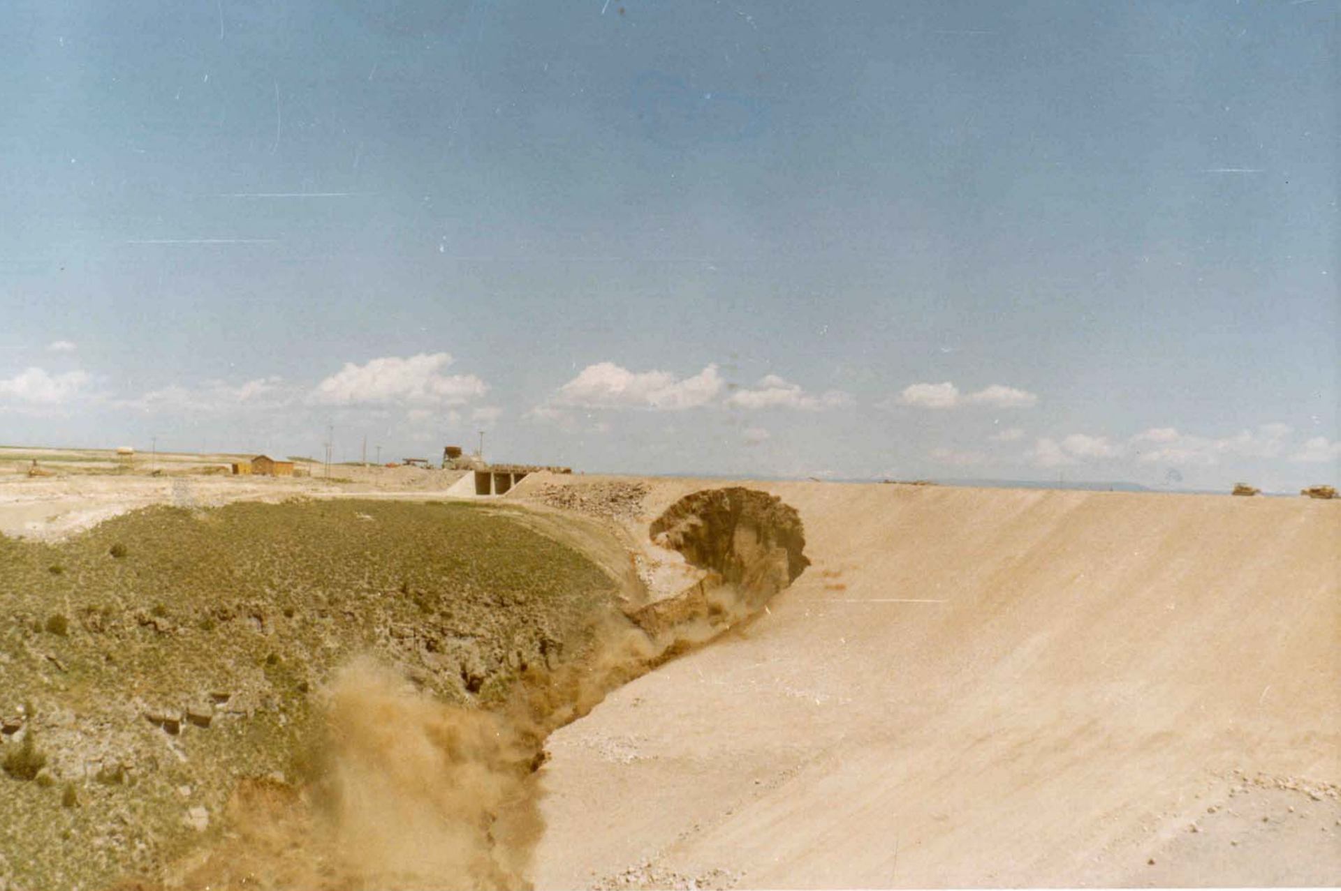
Large Masses of Dam Caving into Erosion Hole about 11:50 am.
