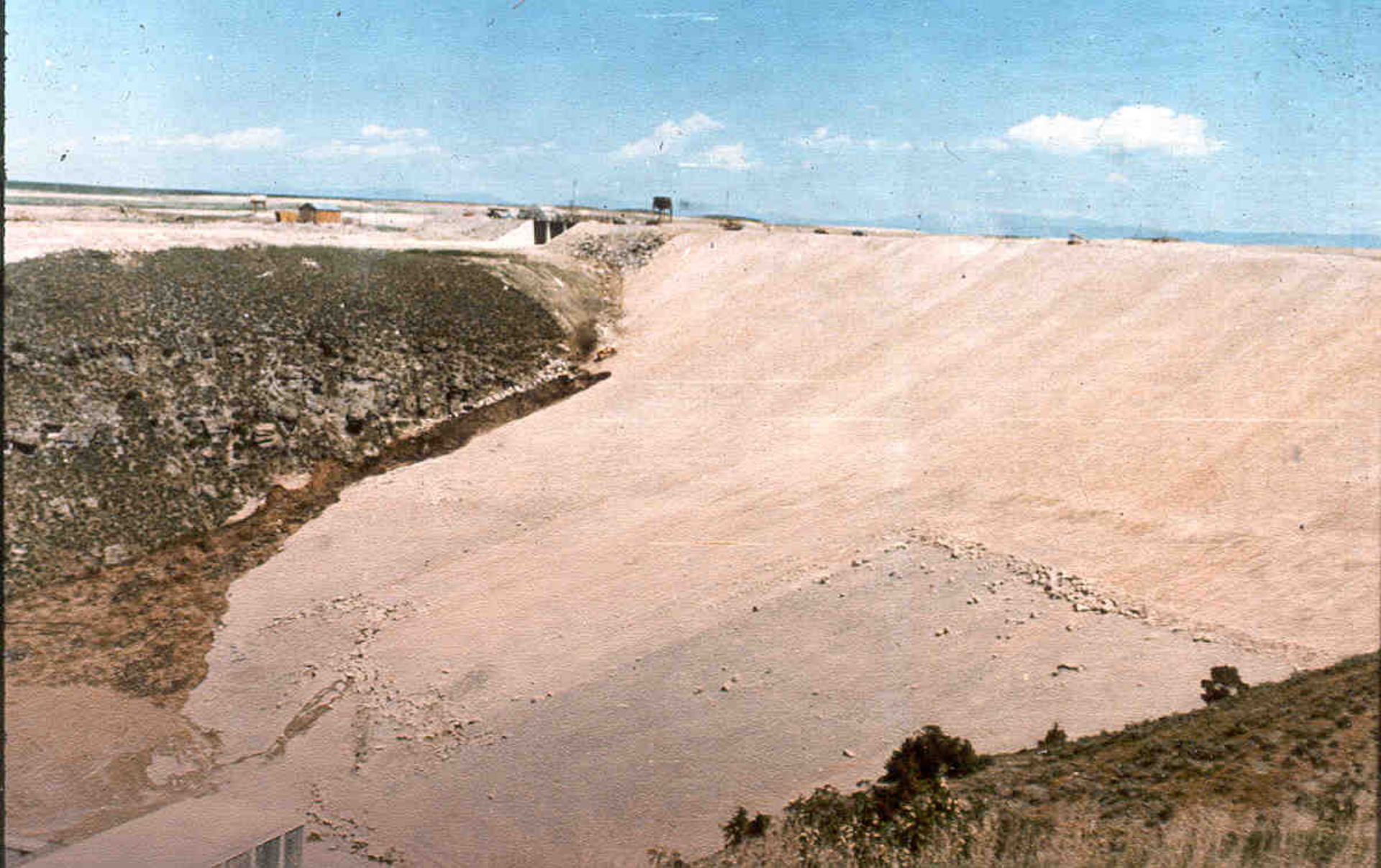
Flow Increasing, Dozers Sent to Fill Hole at Elevation 5200 about 10:45 am
