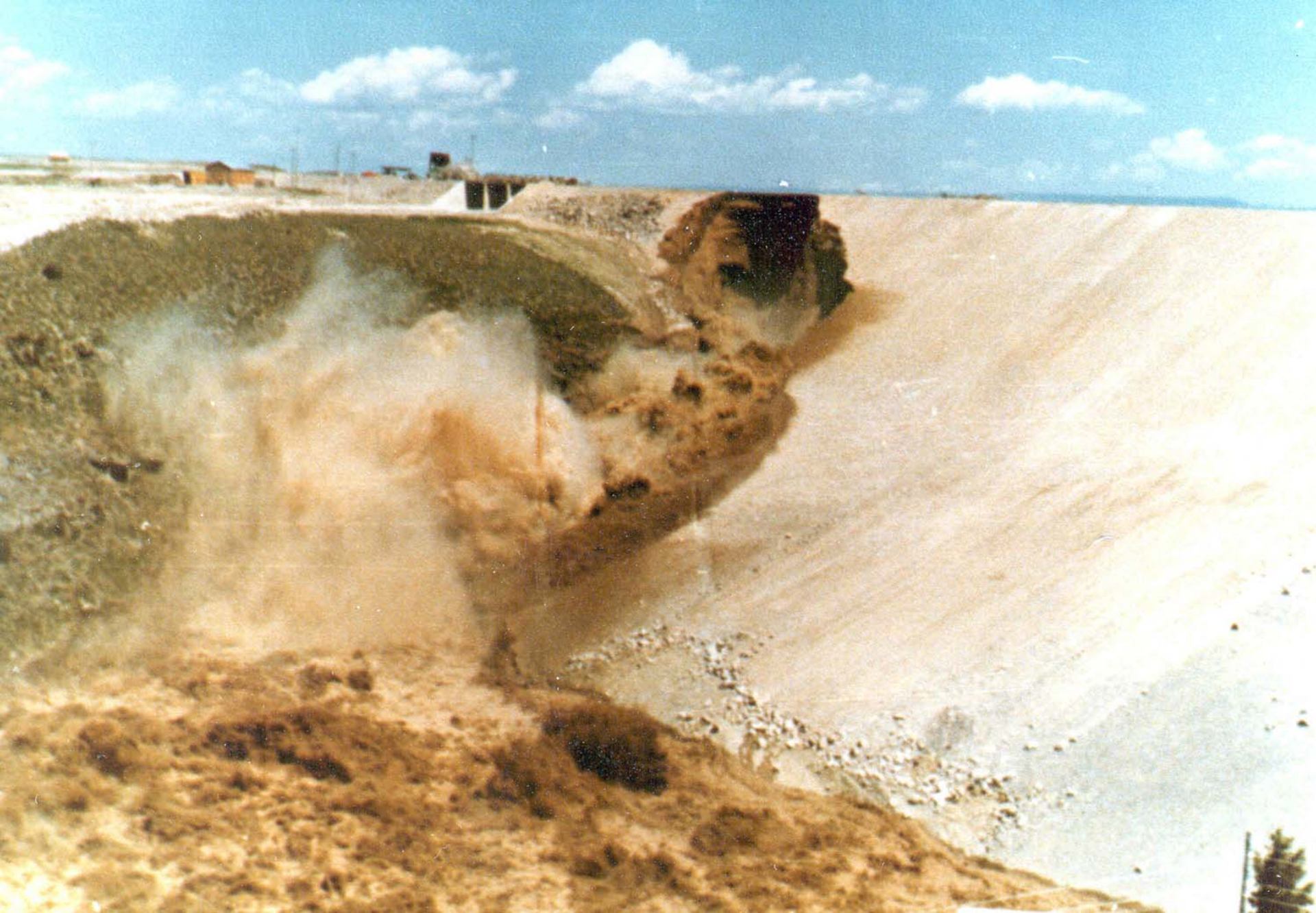
Dam Crest Breaching at 11:55 am, June 5, 1976
