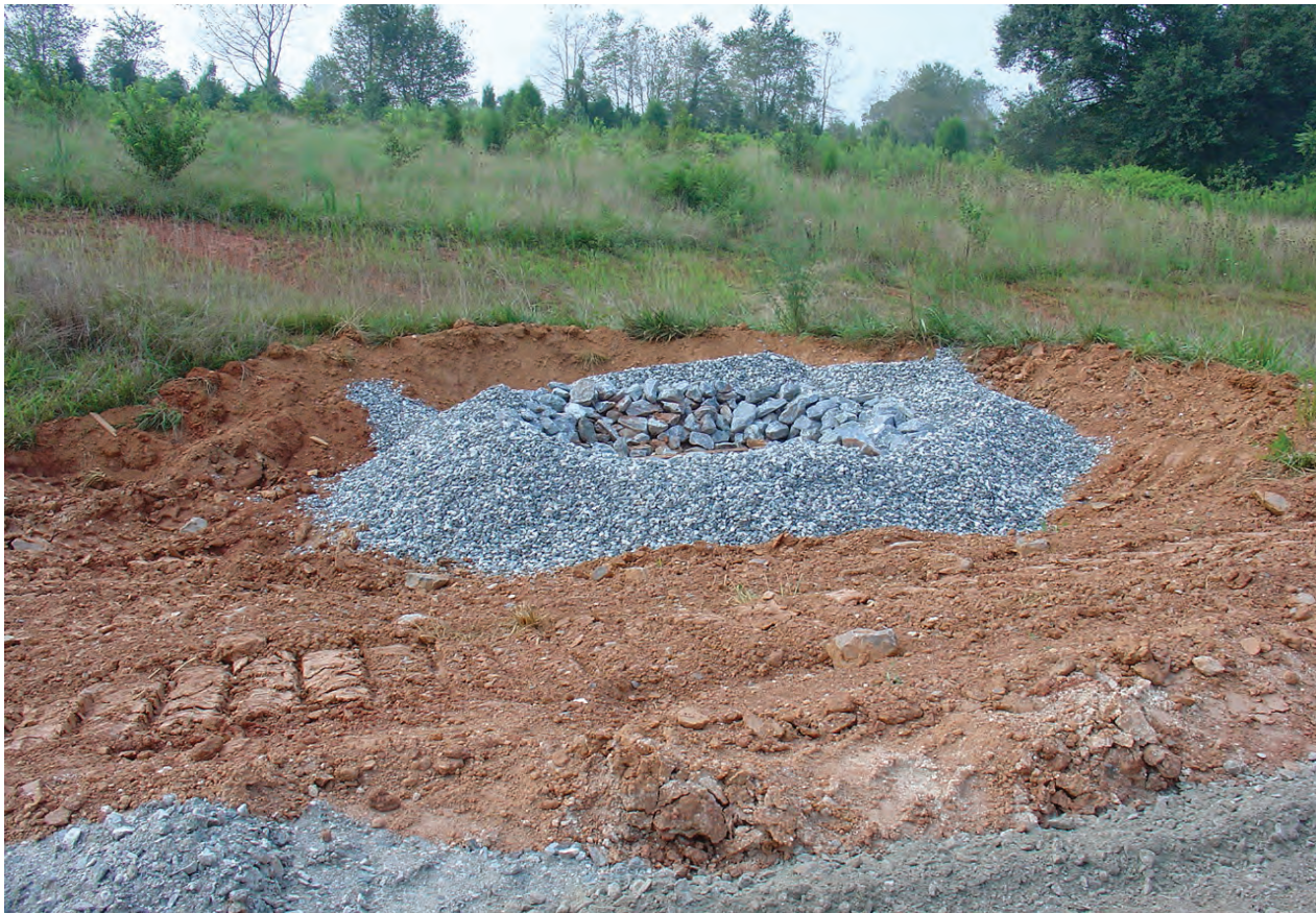
Rock Doughnut Inlet Protection uses larger riprap for the structure base and smaller washed stone to keep smaller particles of sediment from entering the storm drain inlet.
