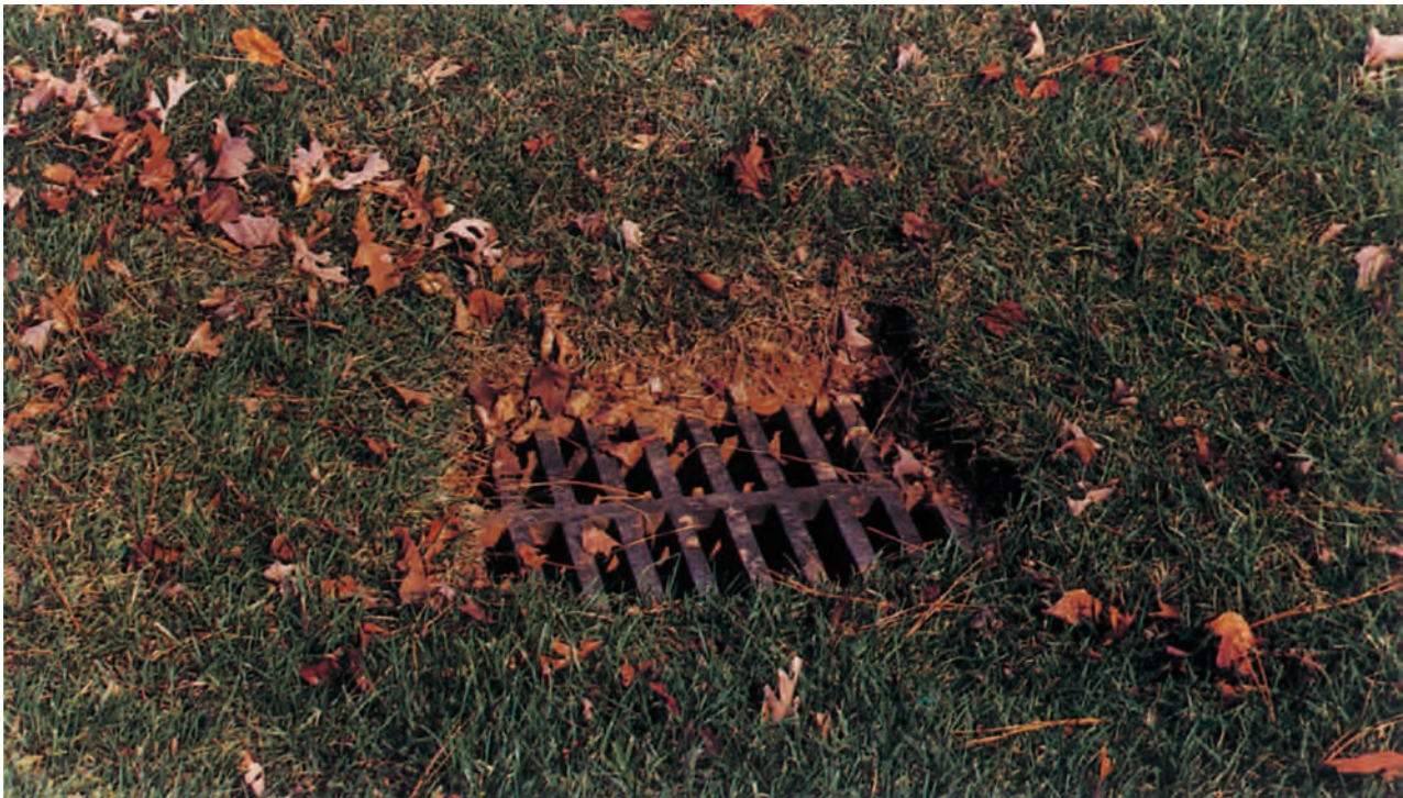
Sod drop inlet provides permanent protection for a storm drain after the drainage area is stabilized.
