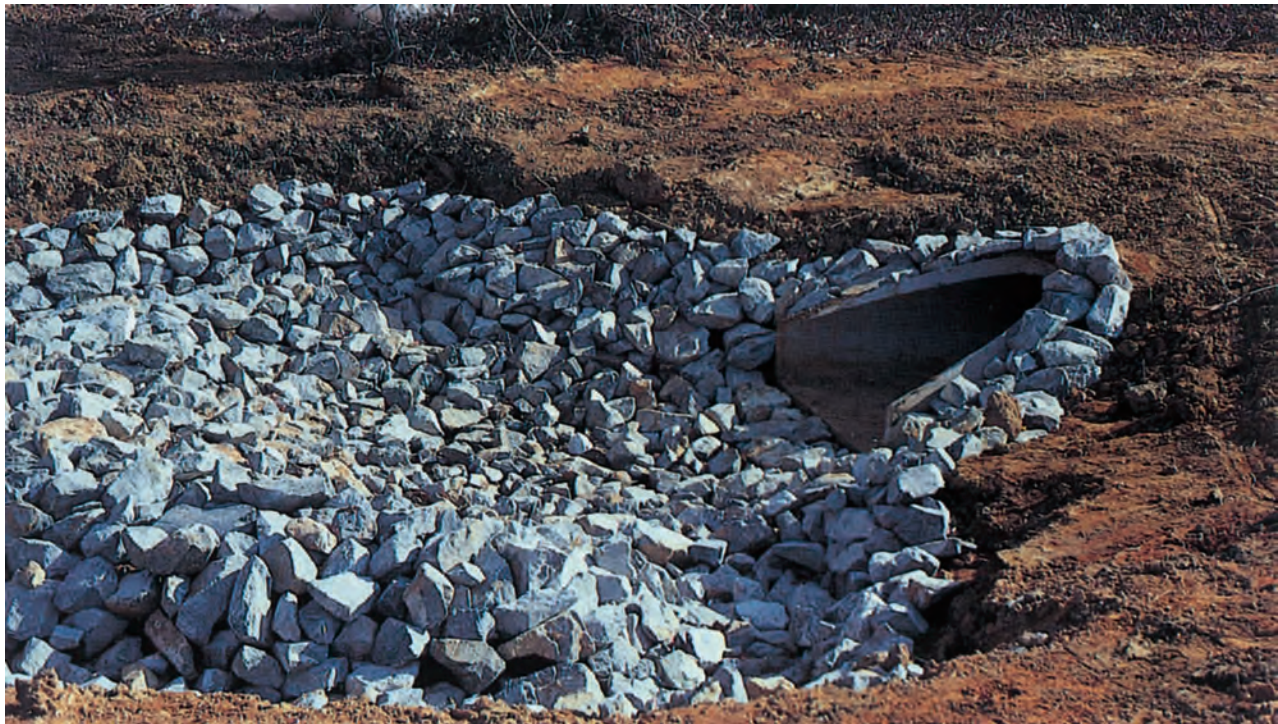
Outlet stabilization with riprap prevents erosion from high-velocity, concentrated flow.
