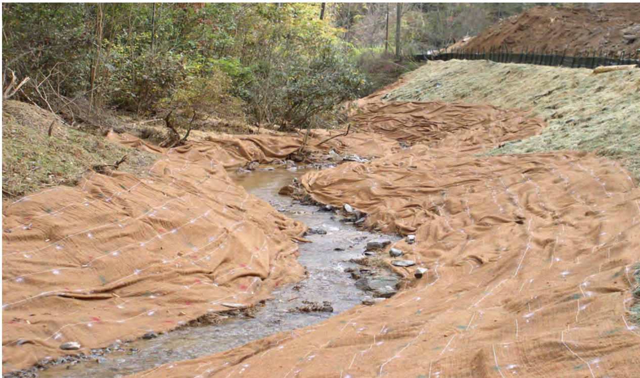
Vegetative Streambank Stabilization protect streambanks from erosion
