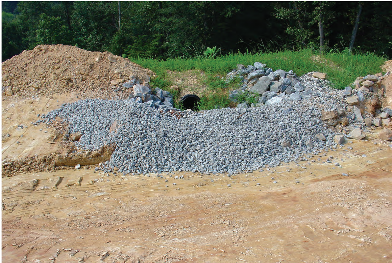
Rock Pipe Inlet Protection uses a small rock dam-type barrier to divert sediment laden water away from the pipe.
