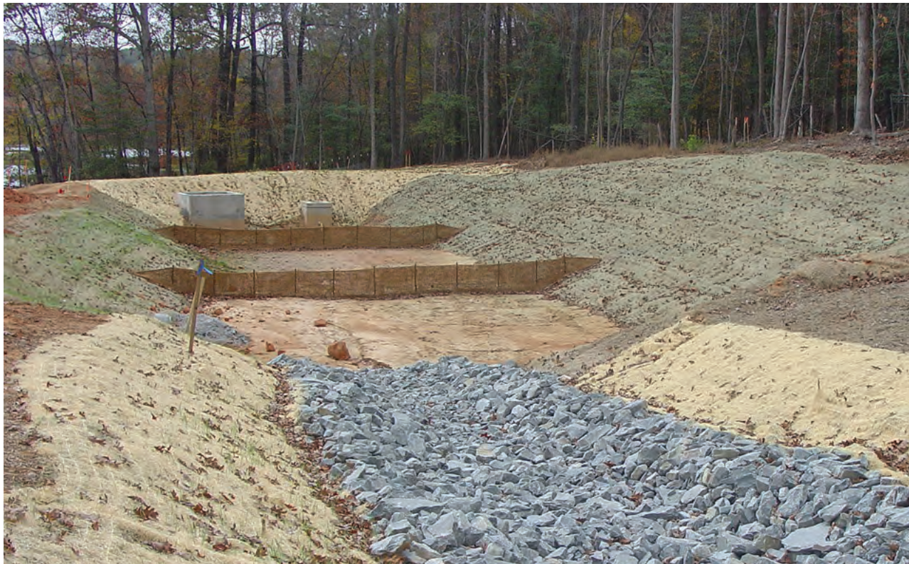
Sediment basins are strategically located to trap sediment near the outlet of a work site.
