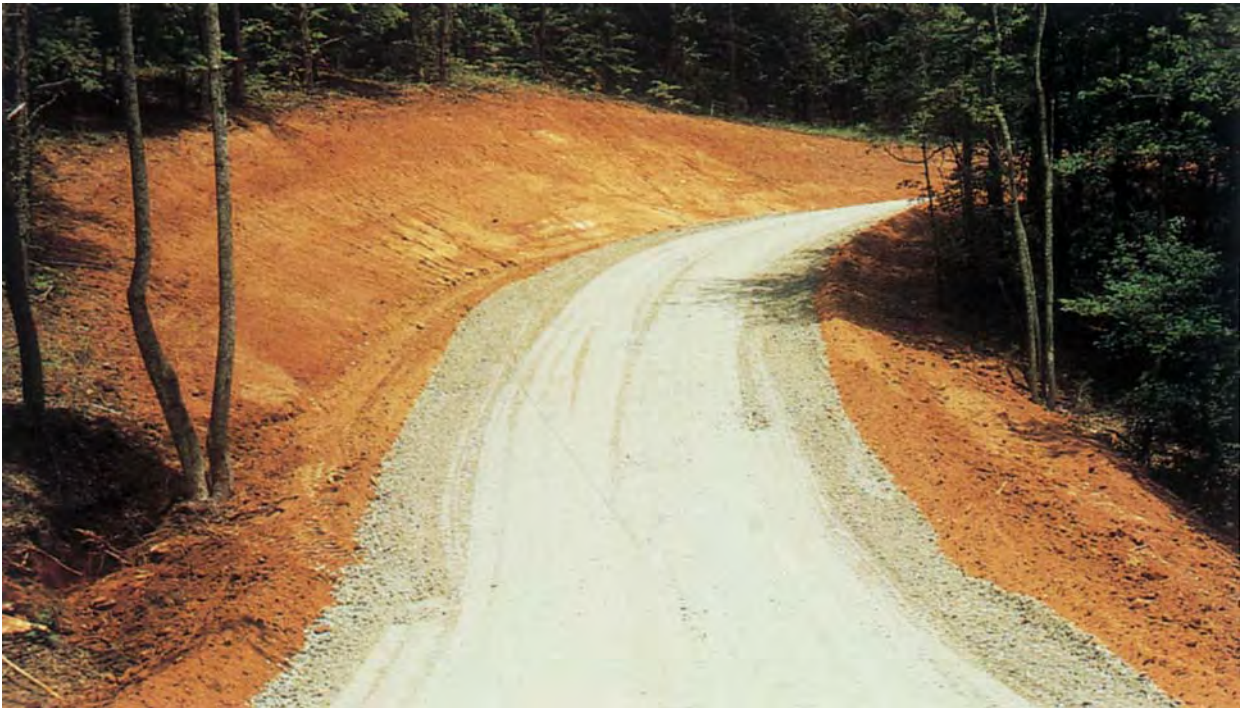
Construction road stabilization improves work efficiency and prevents erosion.
