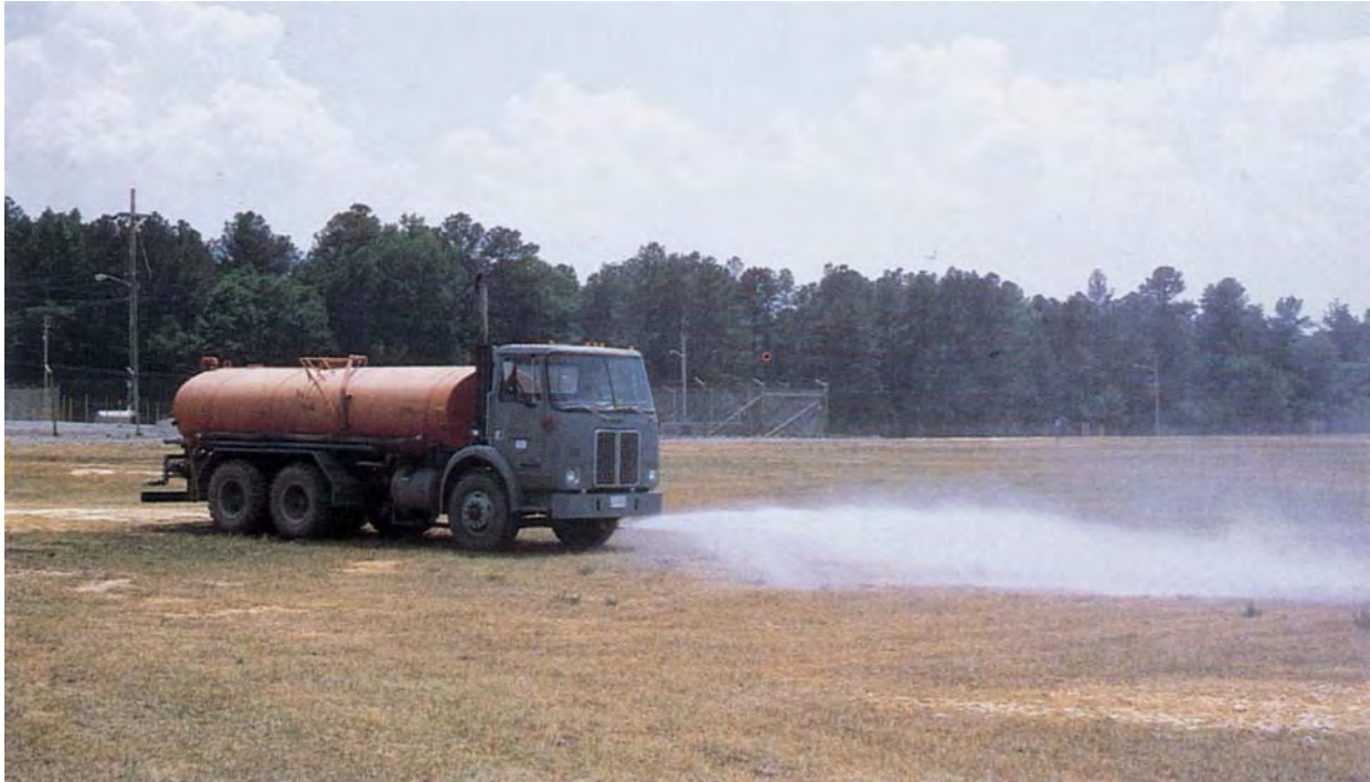
Dust control by watering provides immediate protection, but water must be applied periodically throughout dry periods (source: SCS).
