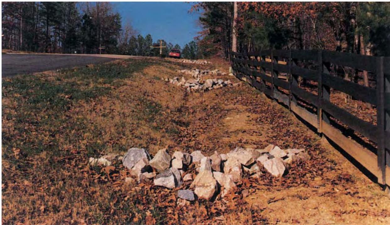
Check dams slow velocity of flow in temporary, low-flow channels.
