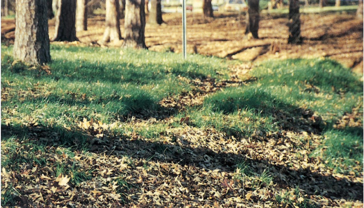
Level spreader releases flow from a diversion onto a uniform stable area.
