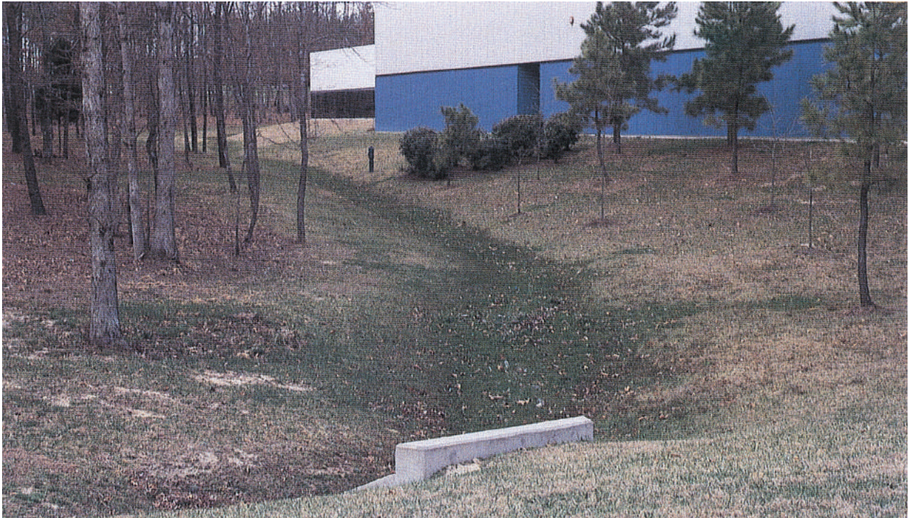
Grass-lined channels are preferred where flow velocities are within permissible limits.
