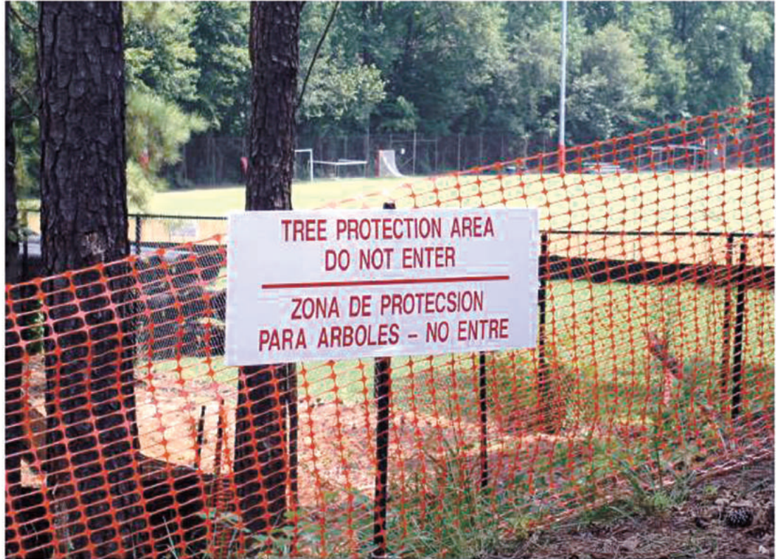
Figure 6.05a Tree protection zone. A protected zone preserves roots and soil and keeps branches clear of contact with construction equipment and materials.
