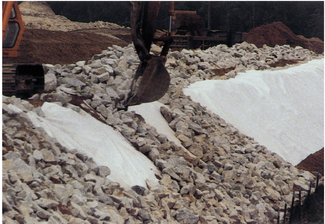
Riprap can be used to line slopes or channels to prevent erosion.
