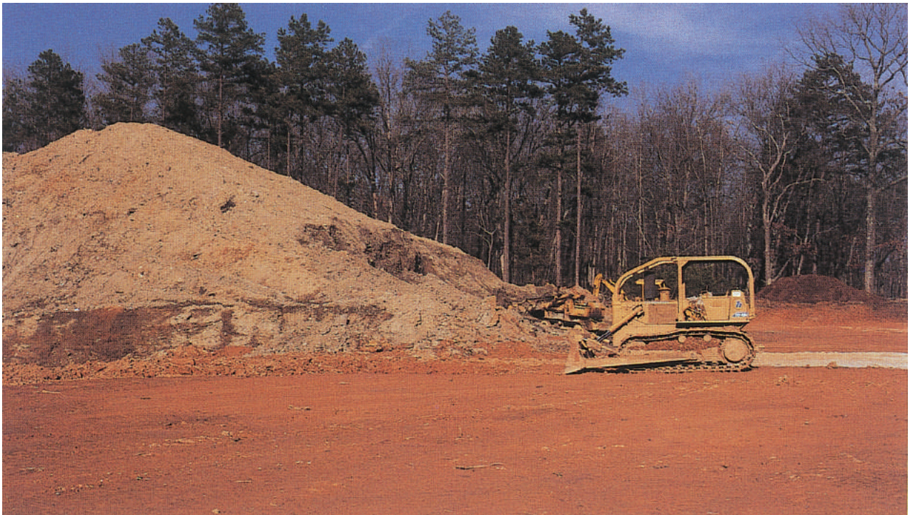
Topsoil is stockpiled for final site preparation and stabilization.
