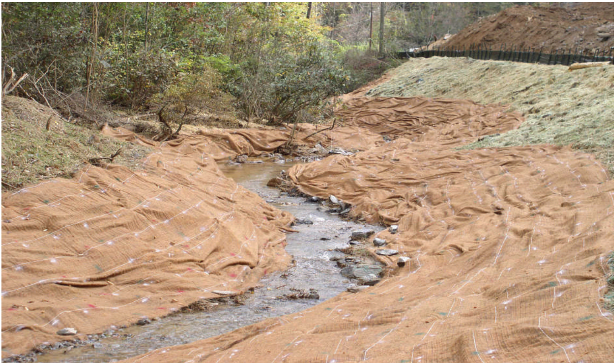
Vegetative Streambank Stabilization protect streambanks from erosion
