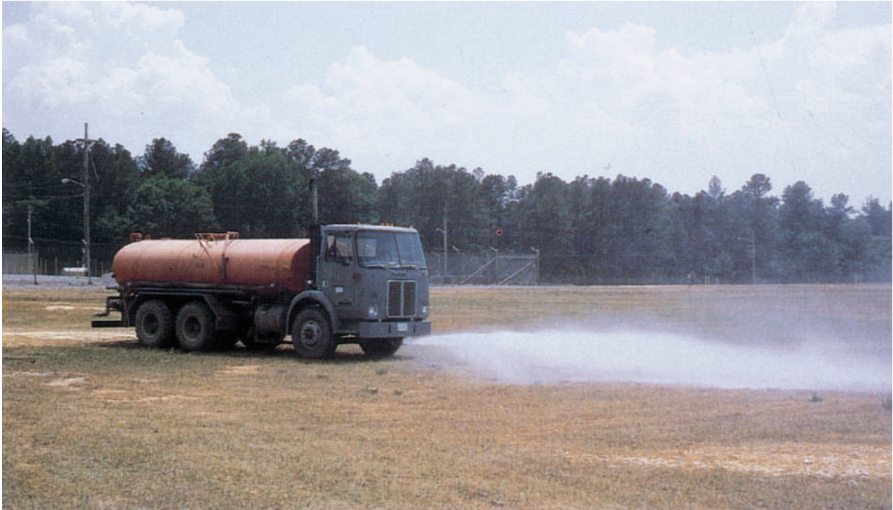
Dust control by watering provides immediate protection, but water must be applied periodically throughout dry periods (source: SCS).
