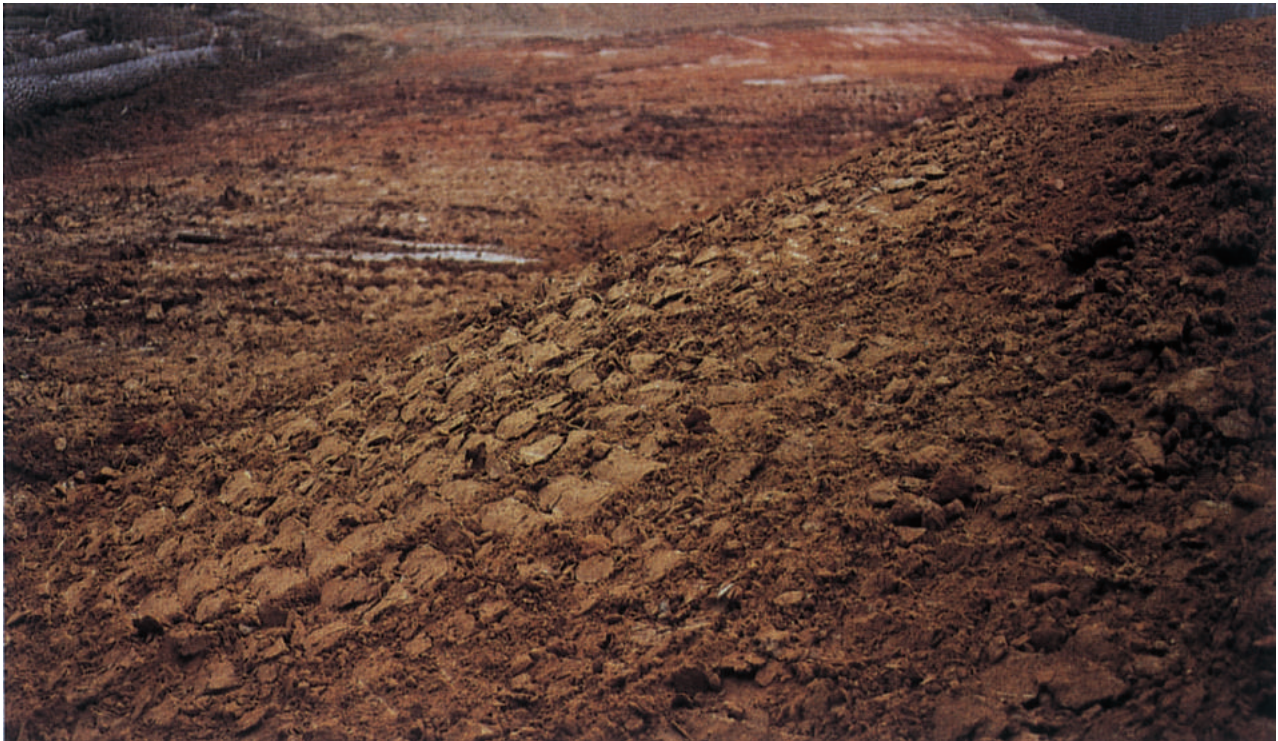
Surface roughening is the first step in vegetative stabilization.
