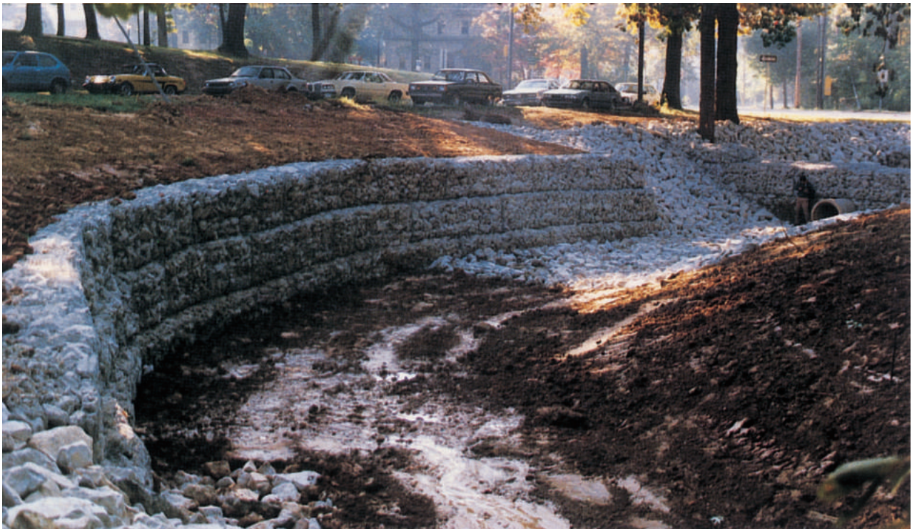
Structural streambank stabilization such as gabions and riprap is necessary where stream velocities are high and side slopes are steep.
