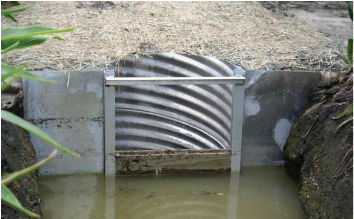
Figure 6.61c Flashboard Riser installation example. Photo credit: NC State University
