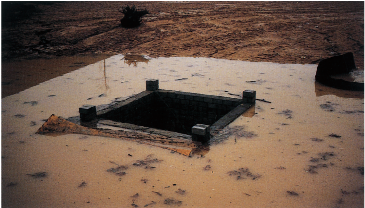
Temporary excavated drop inlet protection creates an effective settling pool to remove sediment at a stormwater inlet.
