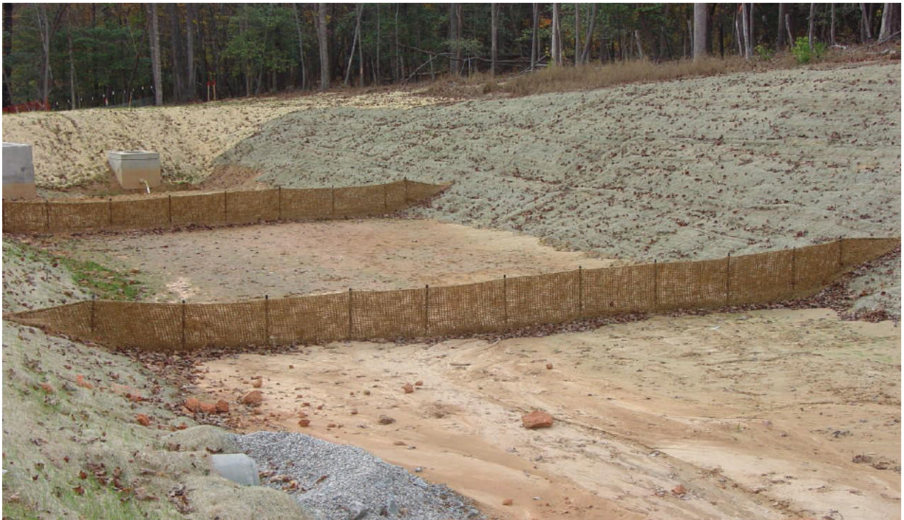
Baffles reduces the velocity and turbulence of water flowing through a measure and assists in the settling of sediment before the water exits the site.
