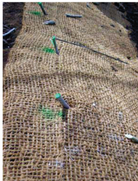
Figure 6.72d Live cuttings installed in fabric
