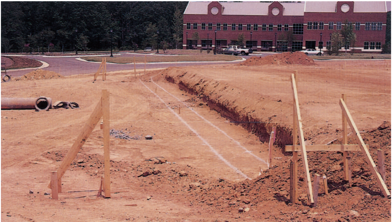
Land grading shapes the surface to a specific line and grade.
