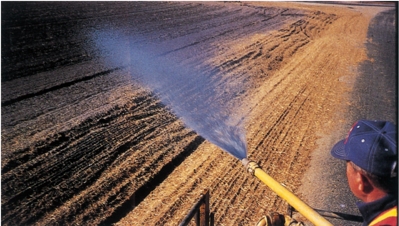
Mulch must be held in place—especially on slopes (source: NC DOT).
