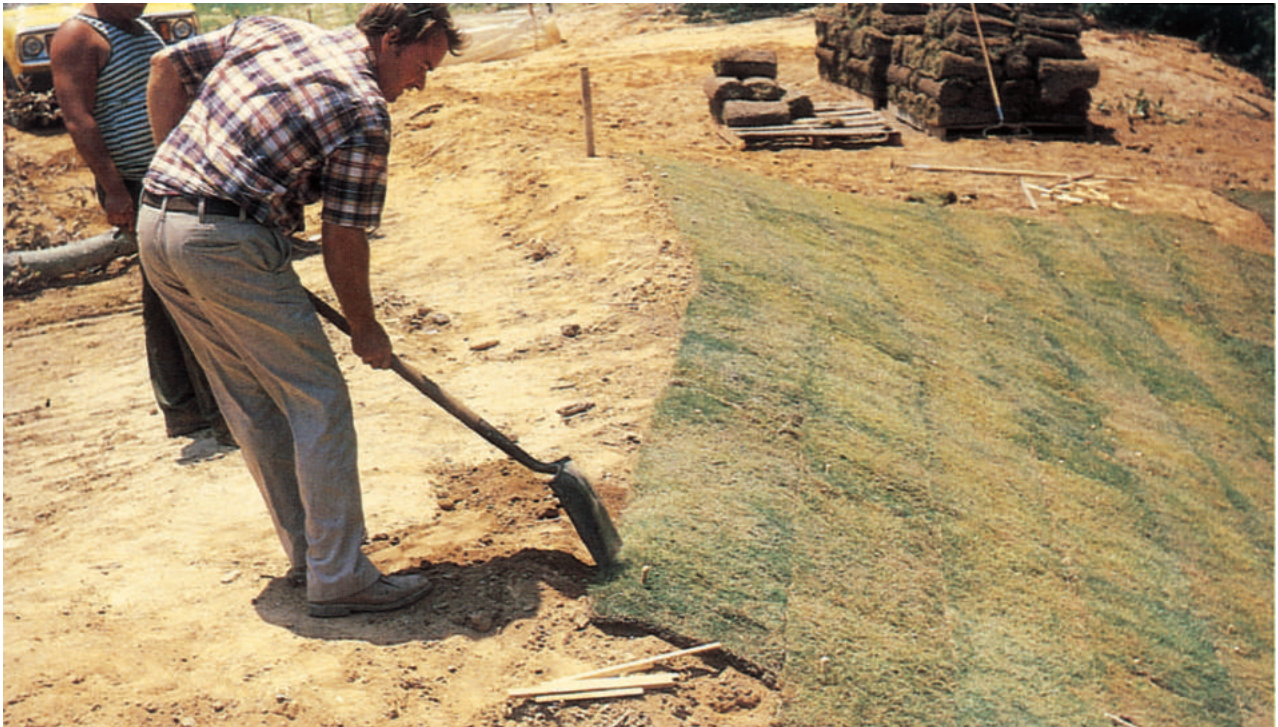
Sodding is an effective way to immediately stabilize a critical area (Source: NC DOT).
