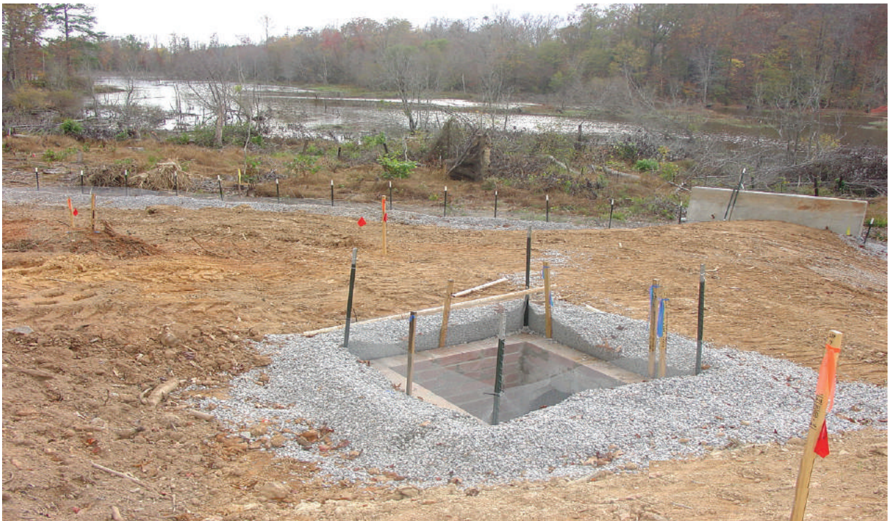
Hardware cloth and gravel inlet protection keeps sediment and debris from construction out of this drop inlet.
