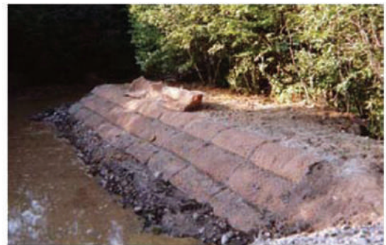
Figure 6.73e Vegetated gabions under construction
