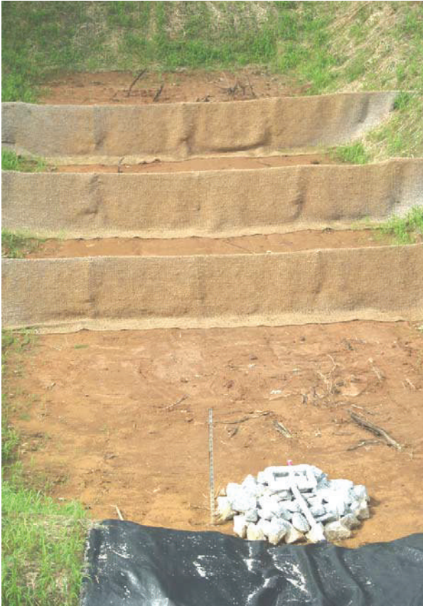
Figure 6.65c Example of porous baffles made of 700 g/m 2 coir erosion blanket as viewed from the outlet.
