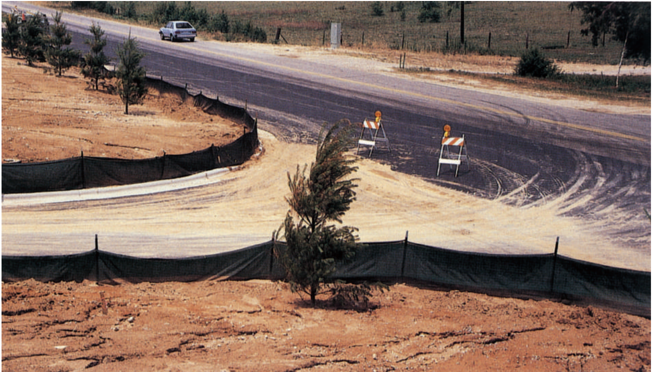
Sediment fences help prevent off-site sedimentation when properly located, installed, and maintained.
