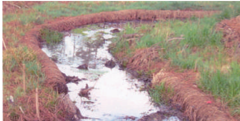
Figure 6.72b Coir log installation, NC Ecosystem Enhancement Program
