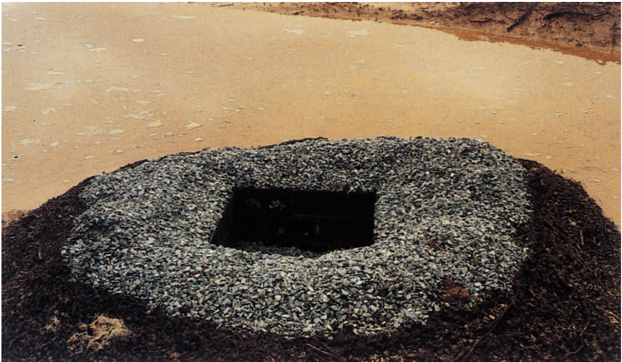
Block and gravel inlet protection prevents sediment from entering this storm drain during construction.
