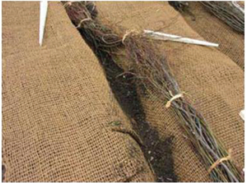
Figure 6.72c Combining fascines and fabric
