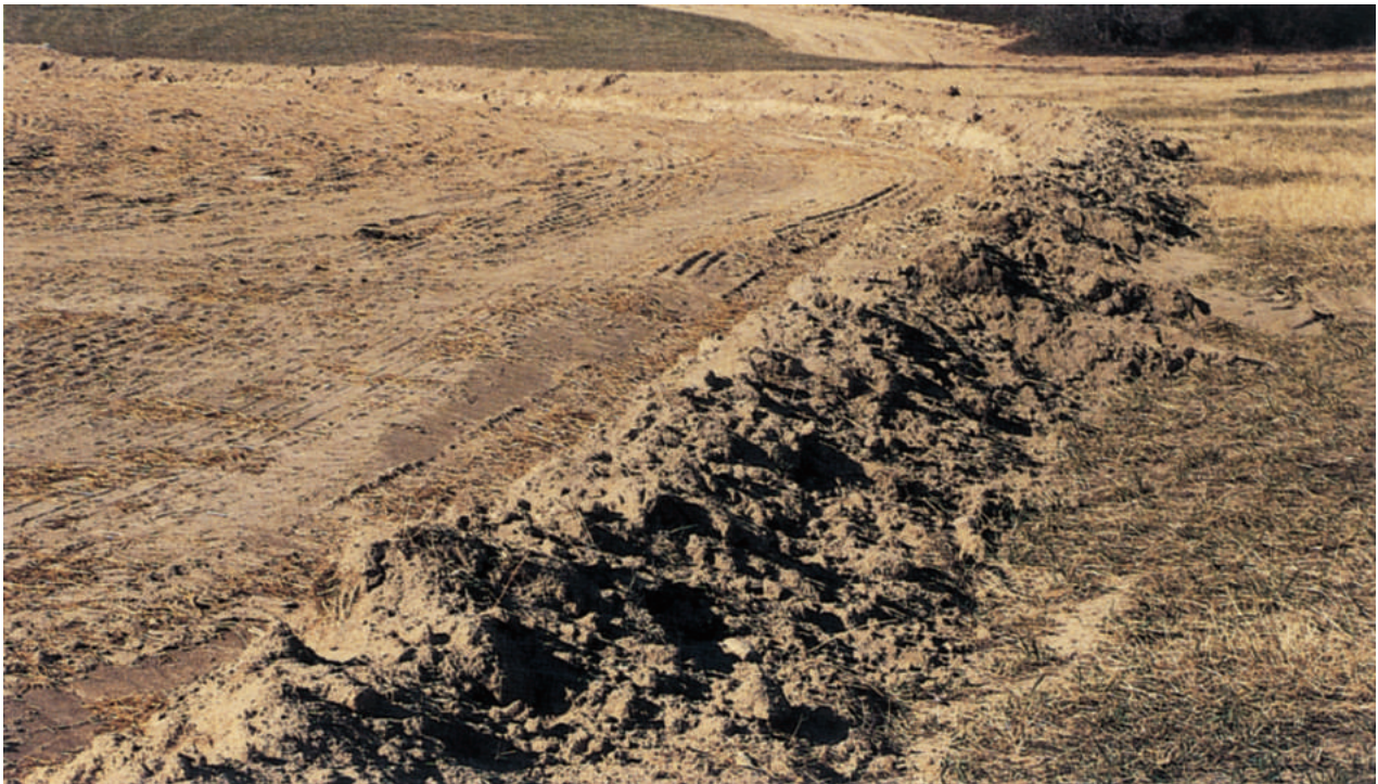
Temporary diversion across a slope helps prevent sheet and rill erosion.
