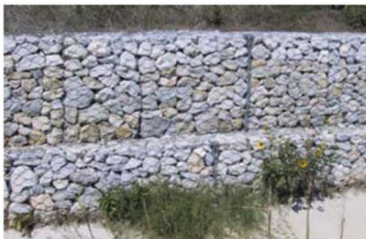
Figure 6.73d Gabions showing a neat, compact, placement of stone with a uniform appearance
