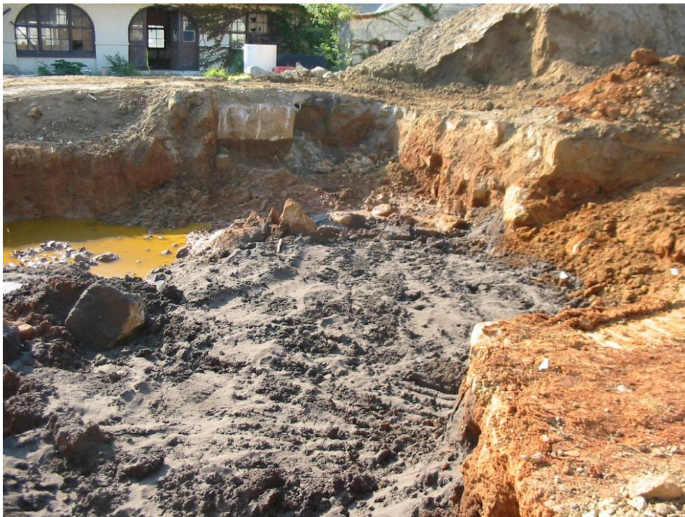
Figure 5. DARAMEND application as excavation backfill.
