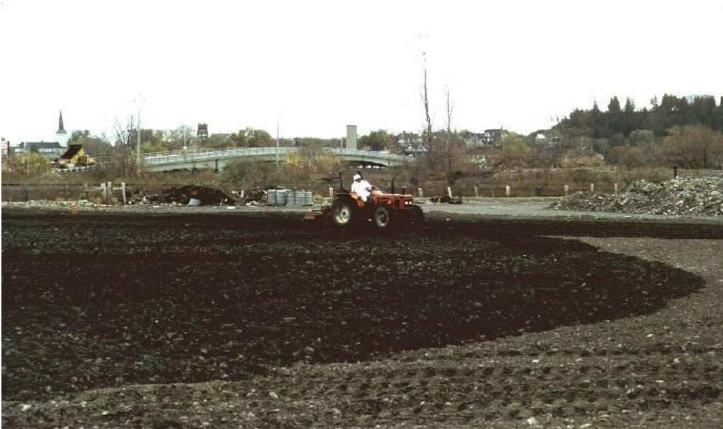
Figure 3. DARAMEND® in situ treatment (upper 60 cm of soil using conventional agricultural machinery with specialized tiller).
