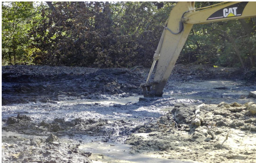
Figure 6. DARAMEND direct soil mixing.
