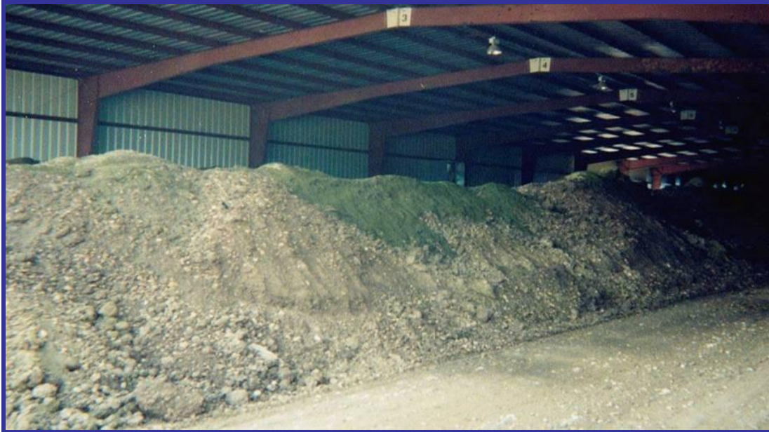
Figure 2. DARAMEND Engineered BioPile Treatment (Joliet Arsenal – Illinois).
