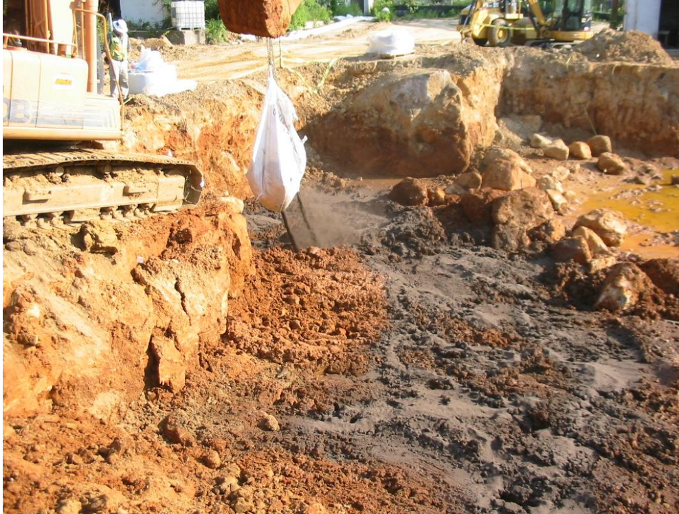
Figure 4. DARAMEND application as excavation backfill.
