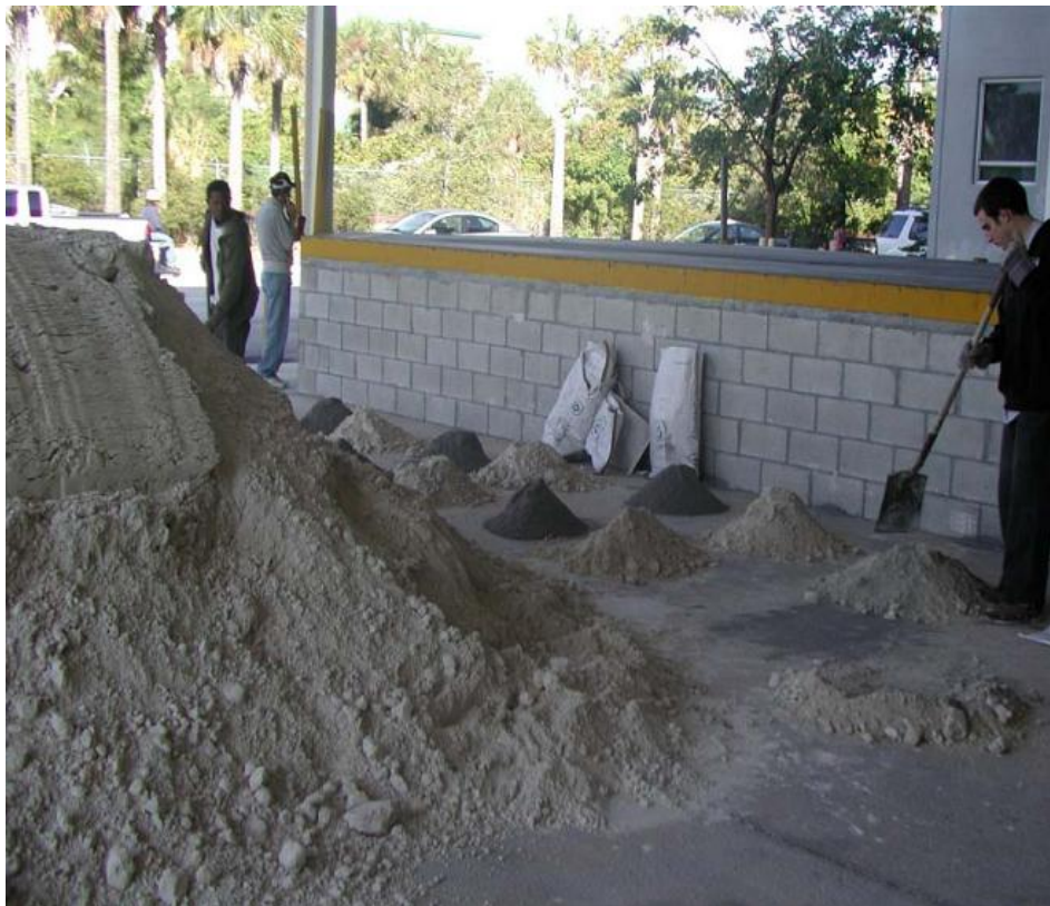
Figure 11. Application of ISCR Reagent to Backfill material.
