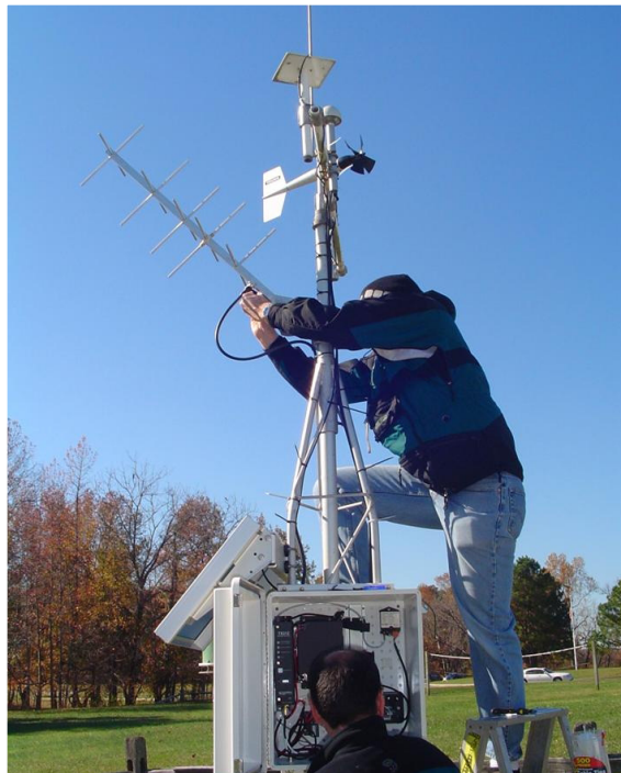
Installing a weather station (photo credit: Chesapeake Bay VA NERR)
