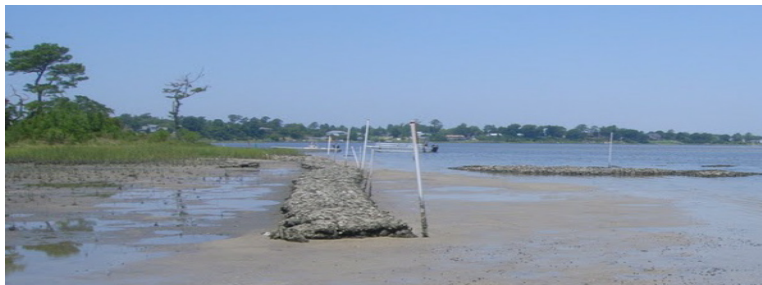
Marsh sill with offshore oyster reefs
