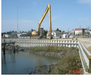
Bulkhead under construction
