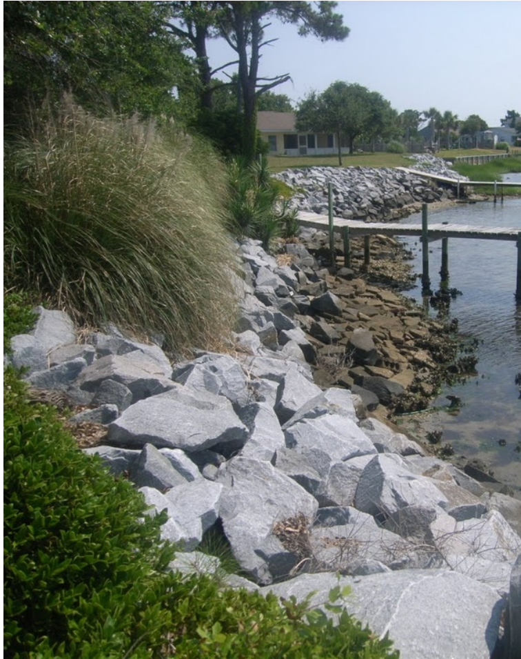
Riprap revetment with grasses and lawn
