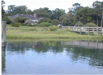
Bulkhead with planted marsh, Beaufort, NC
