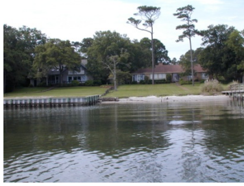
Neighboring properties with different erosion protection approaches
