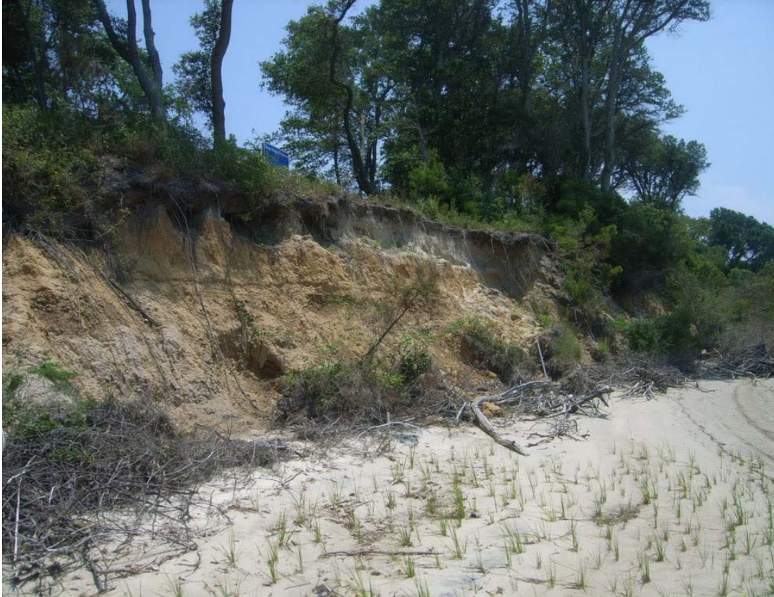
Figure 3: Eroding high bank bluff with marsh plantings in front at Jones Island, Onslow County.
