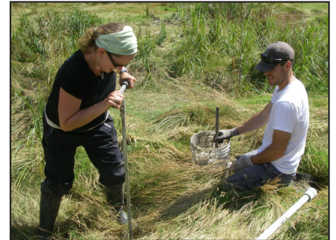
Deep groundwater well installation.
