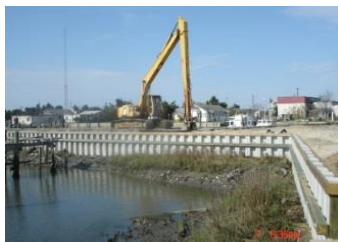
Bulkhead under construction, Radio Island, N.C.
