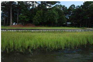
Vinyl bulkhead with waterward marsh, N.C.
