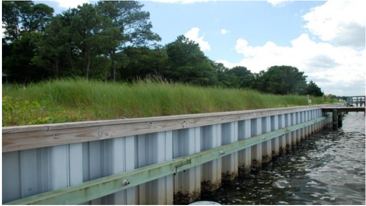
Bulkhead constructed using vinyl, Pivers Island, N.C.
