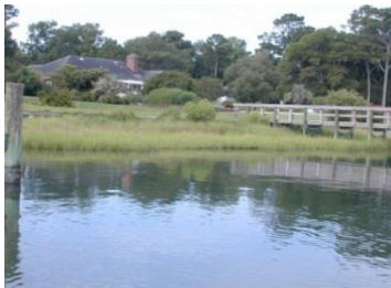
Bulkhead with marsh, Beaufort, N.C.
