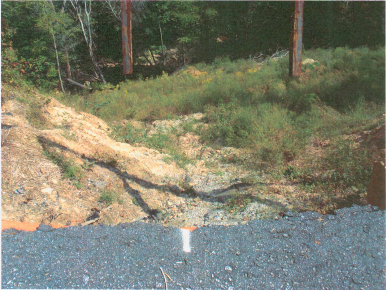
Slide path into Tuckseigee River
