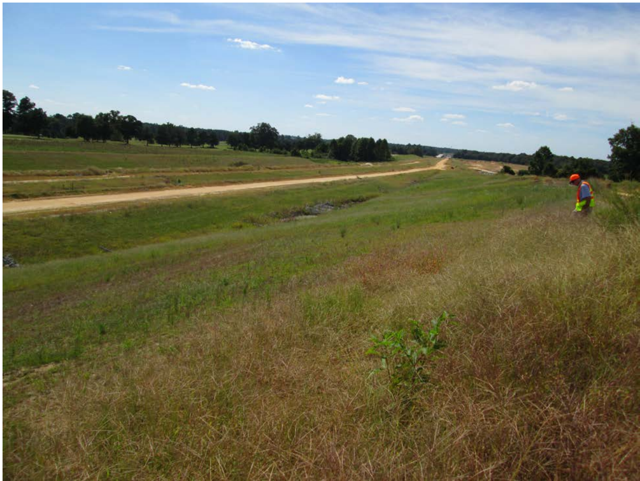
Excellent Temporary and Permanent, US 70
