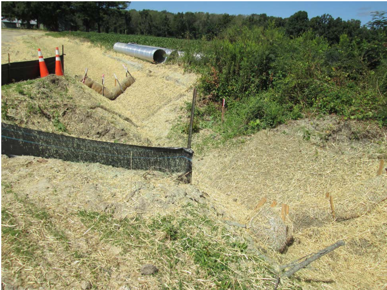
Wattles and Mulched Ditching, Mills Field Road
