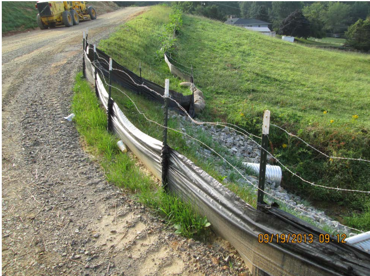
Shady Brook Road, SR 1870—Combination silt fence/horse fence along widened road.
