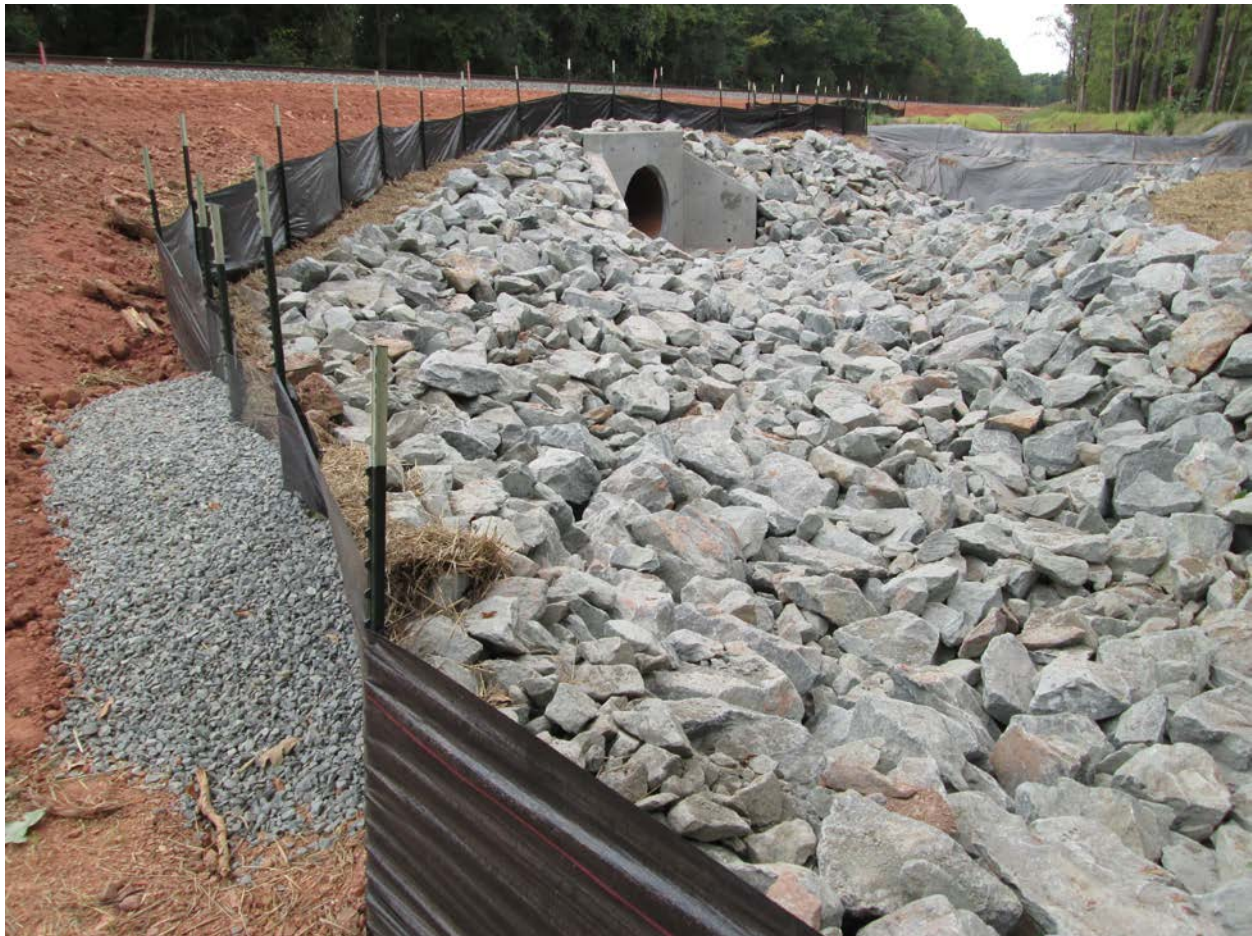
Stabilized culvert outlet underneath the track, Hopson Road
