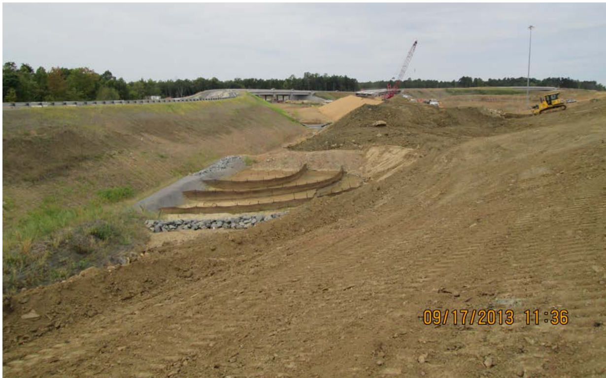
I-485 and I-85 Interchange—Actively graded fill slope and large sediment trap.
