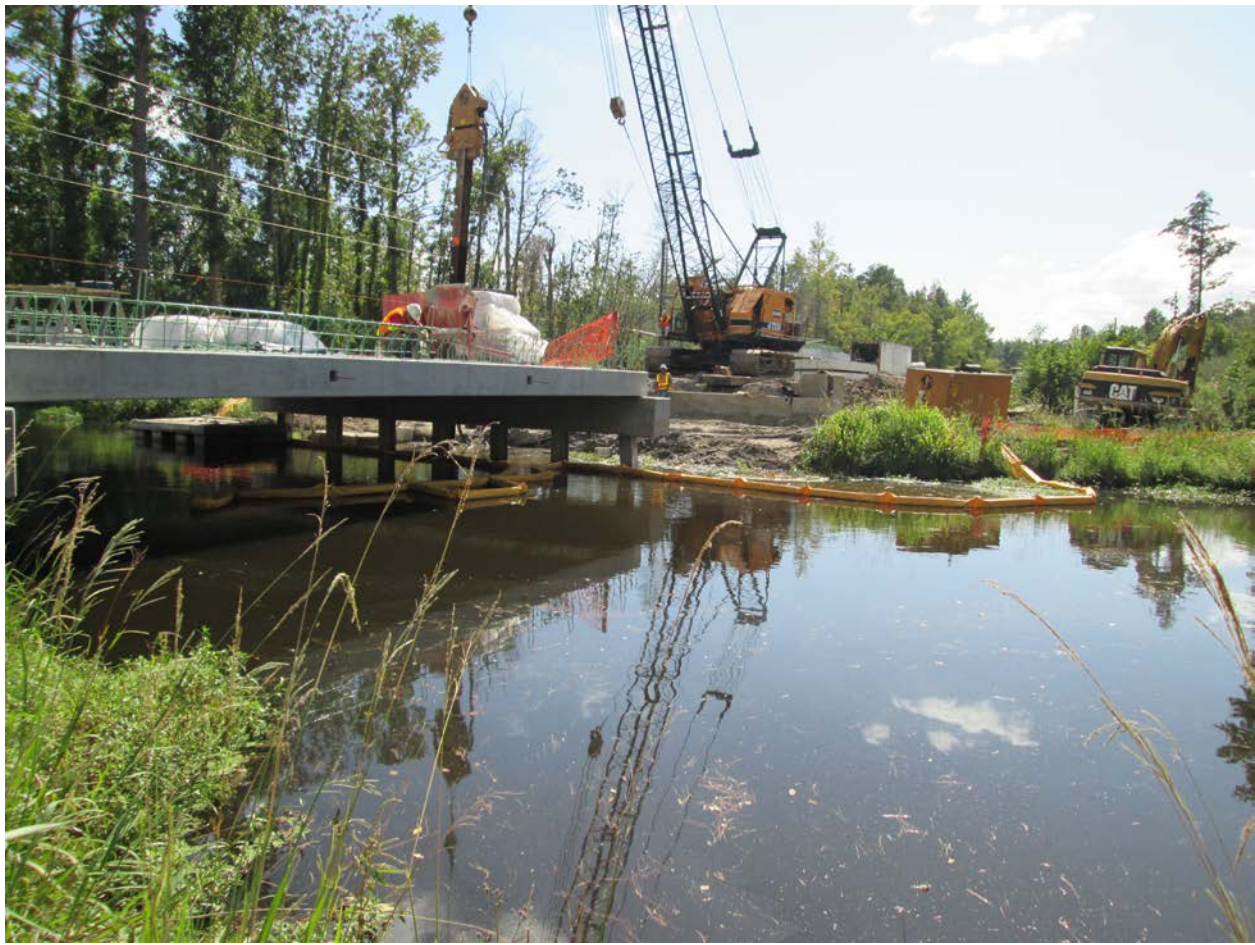
Turbidity Curtain, Broad Creek, US 264
