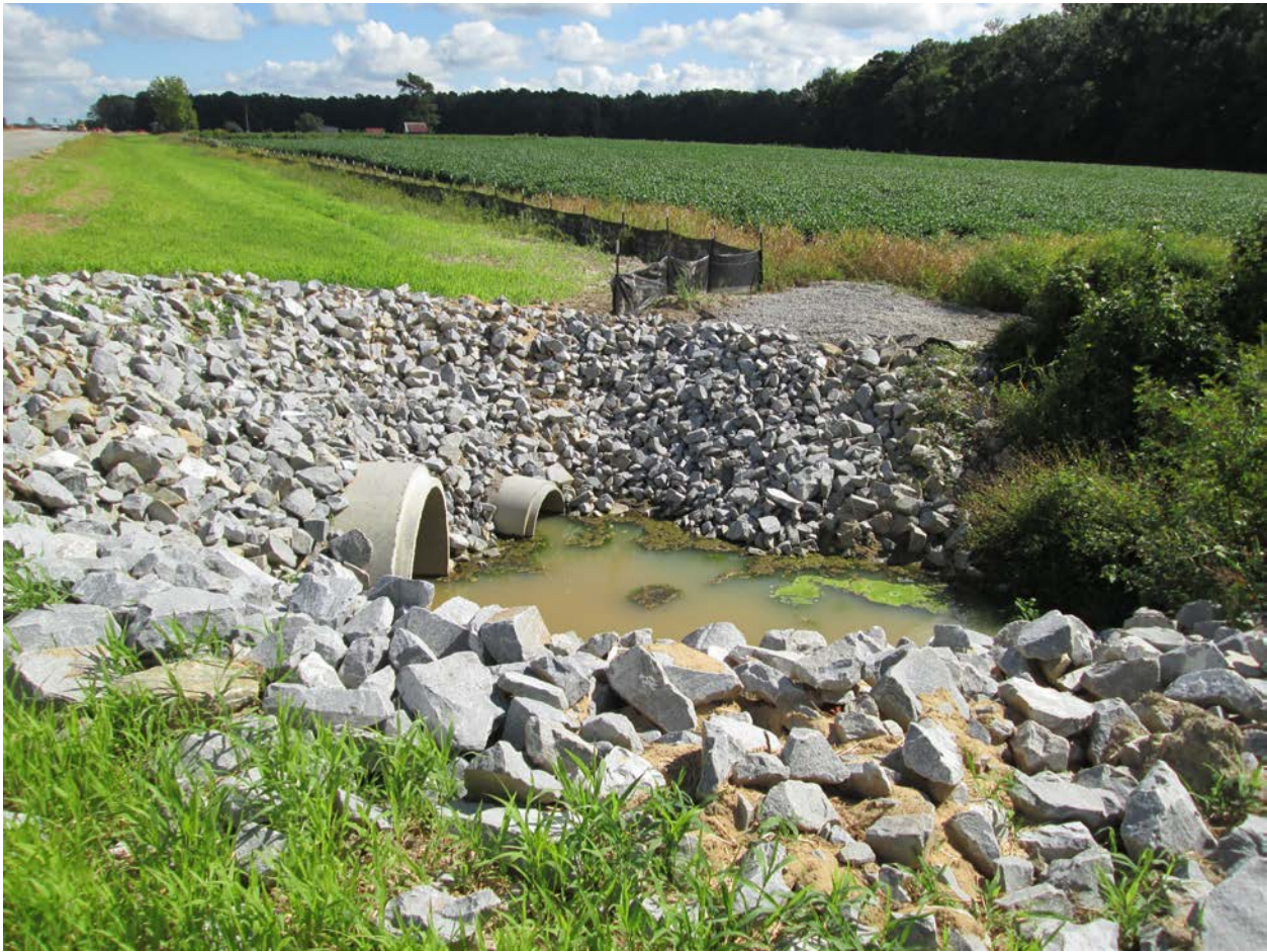
Equalizer outlet and stabilized easement US 158, Tarheel
