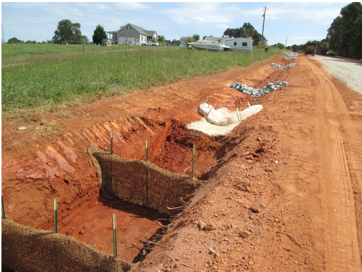
Ditching along Lindo Johnson Road, Chatham County
