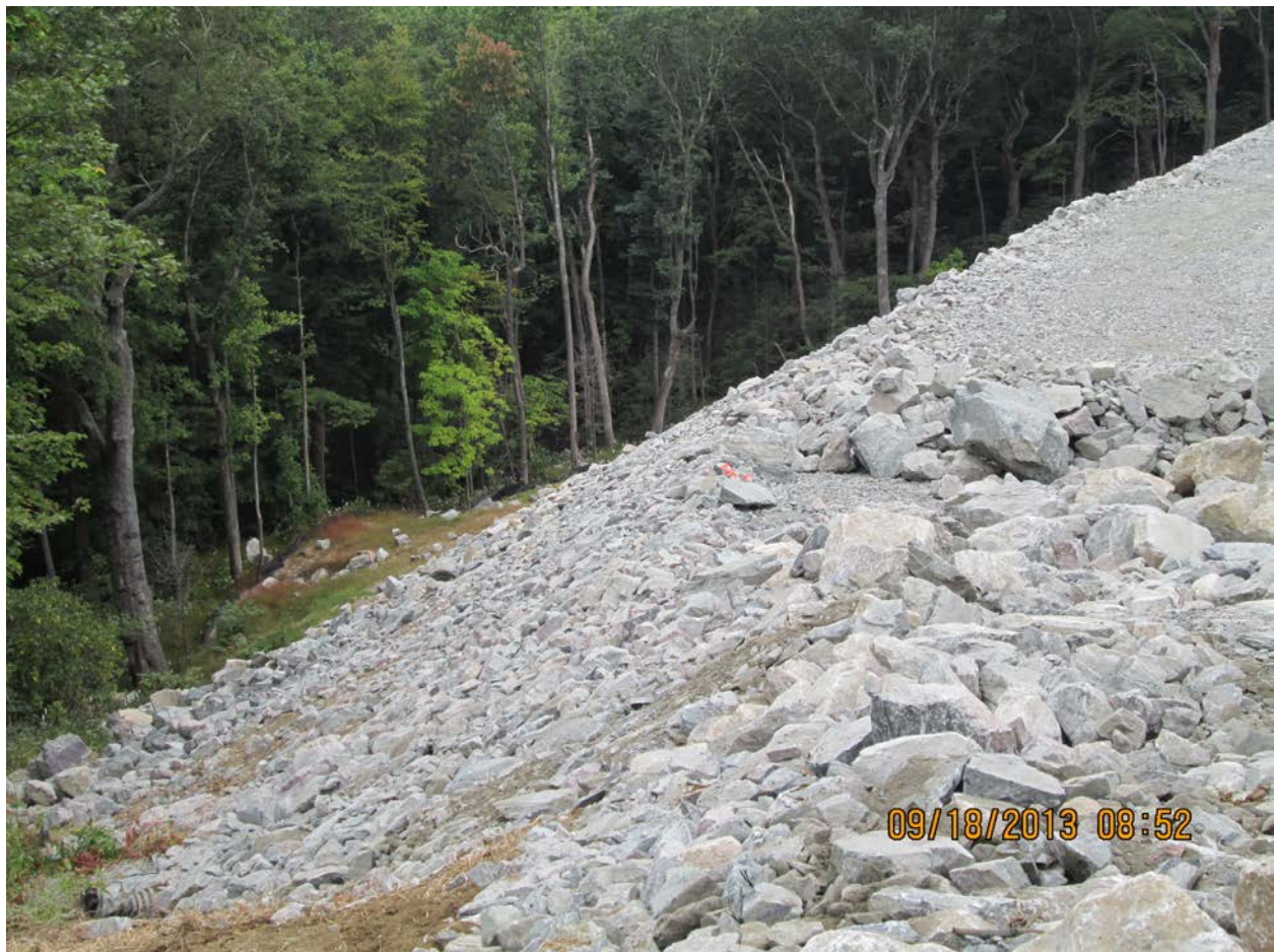
US 321—Fill slope built with rock.
