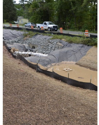
Design: Geotextile is sometimes used to prevent erosion in transitional phases of construction.
