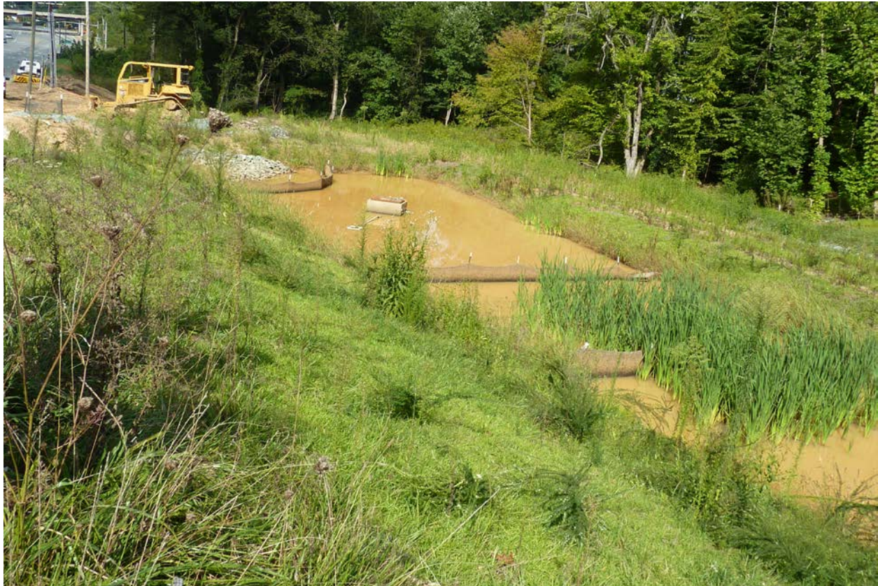
Large skimmer basin, Smith Level Road Widening
