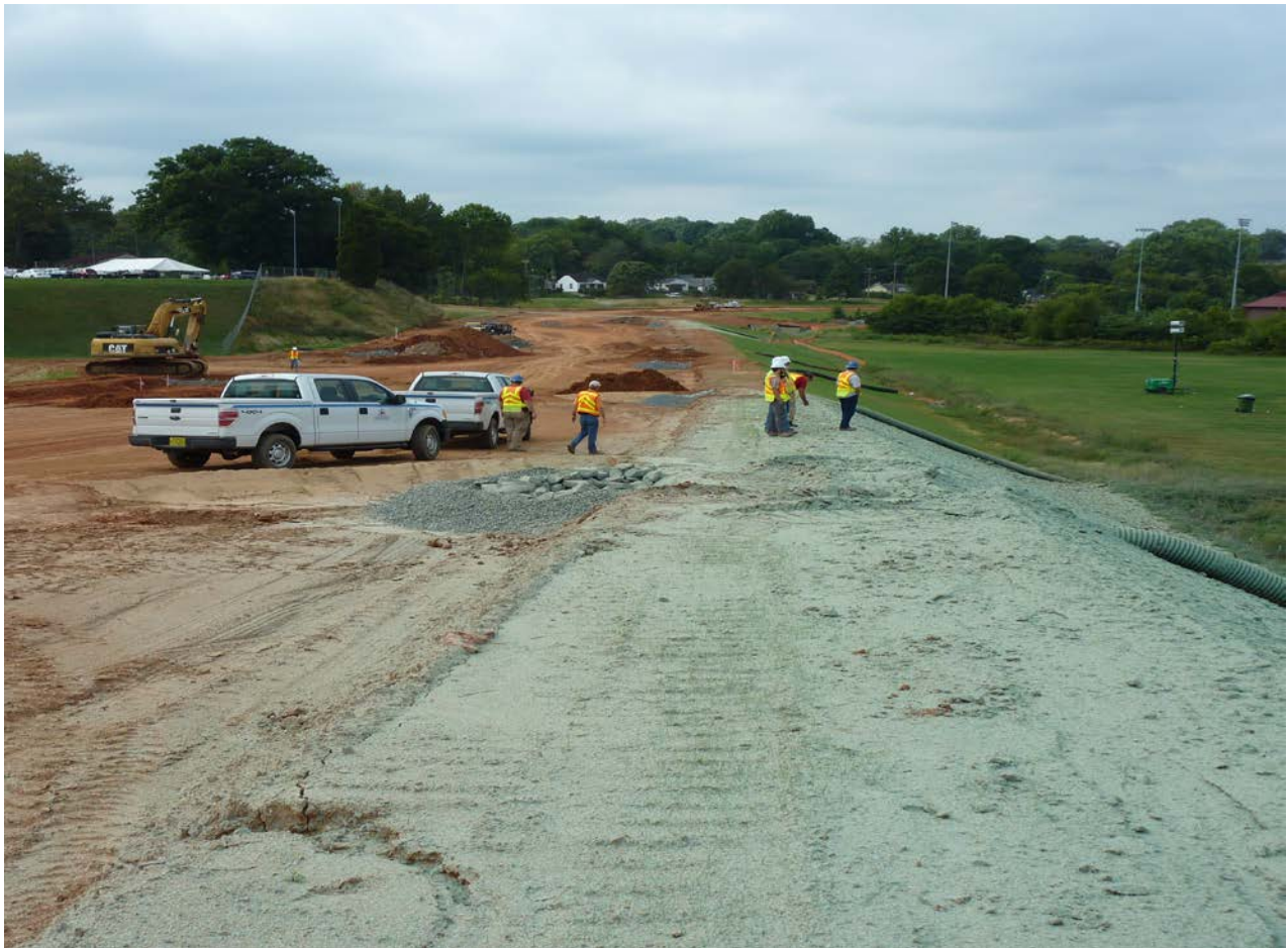
Flexterra used on slope, Salem Creek Connector, Forsyth County
