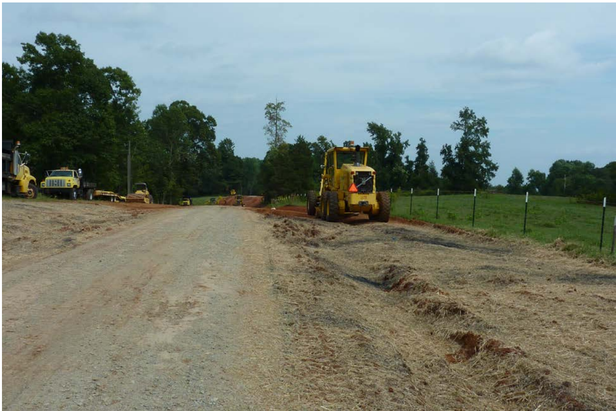
Phased Construction on Road Maintenance Project, Chatham County
