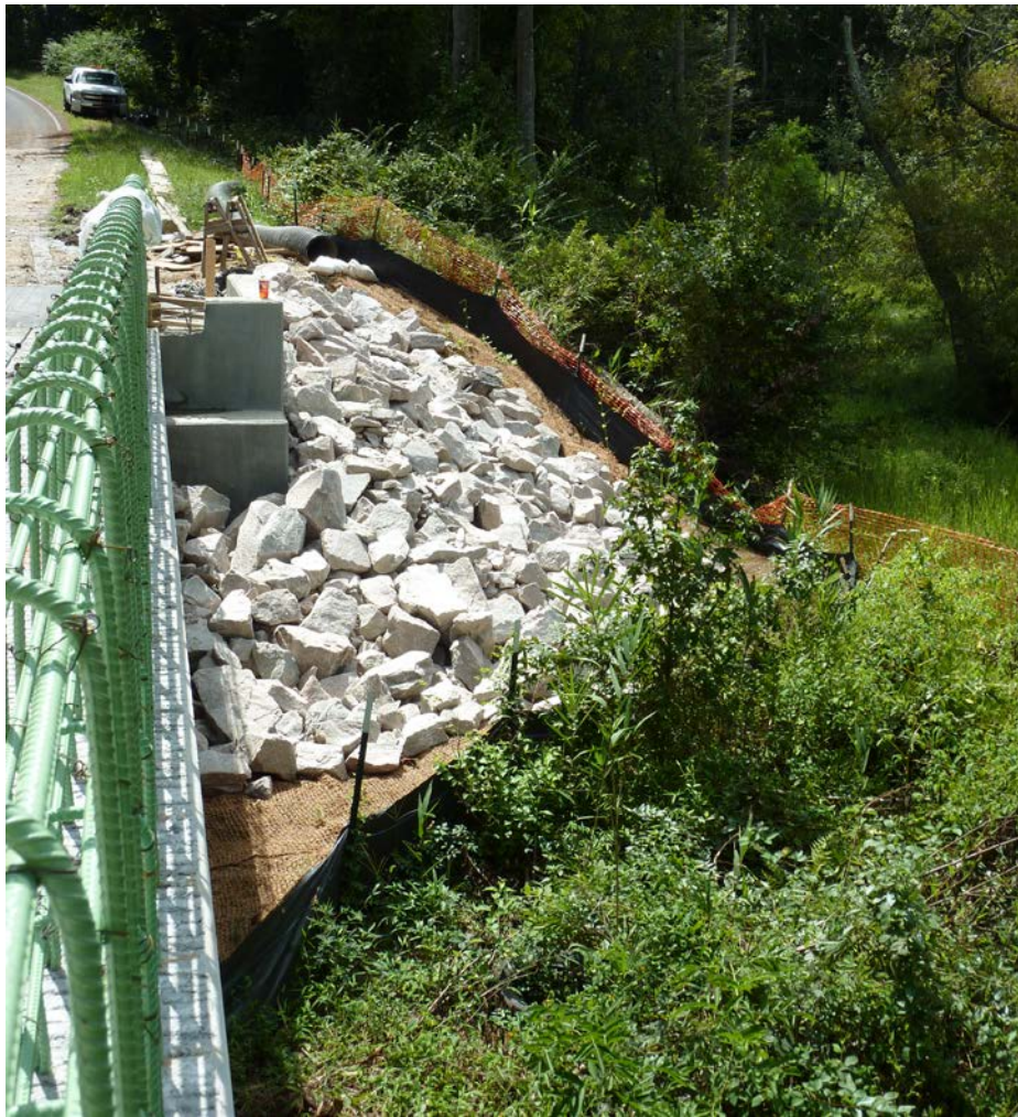
Well protected area along wingwall, Wake County
