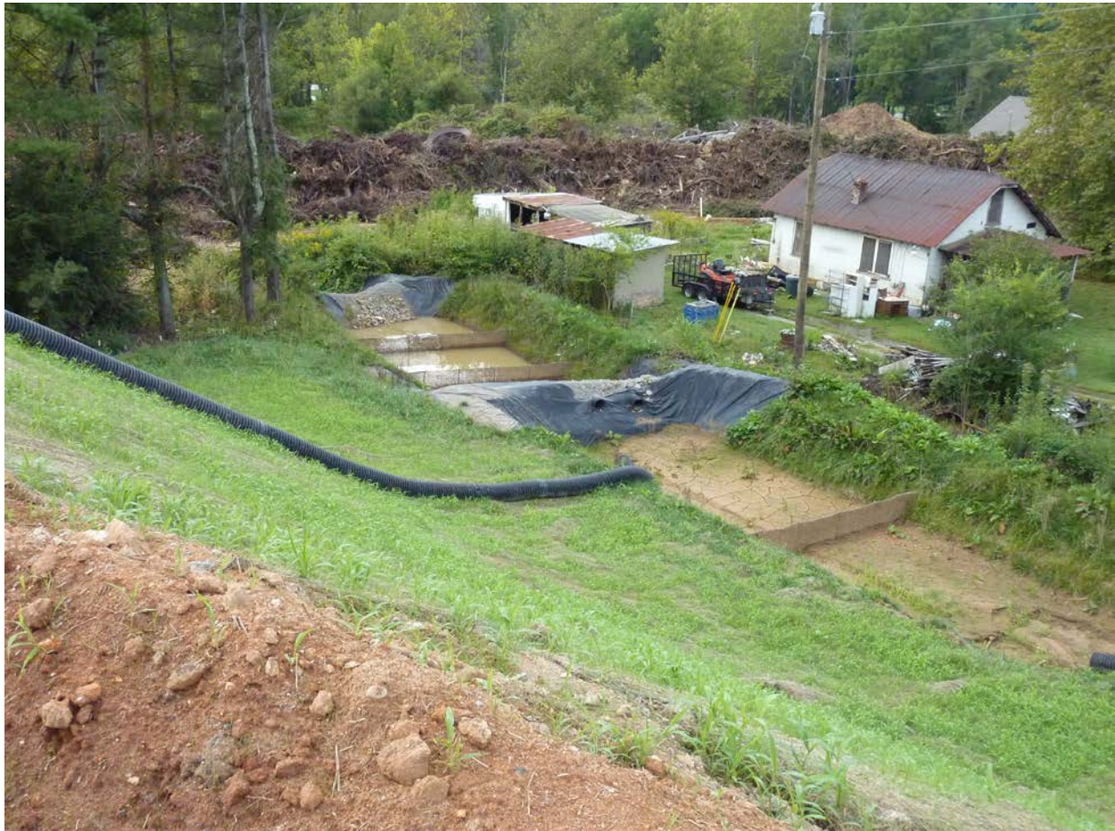
Tiered Basin at Howell Mill Road Widening Project, Haywood County
