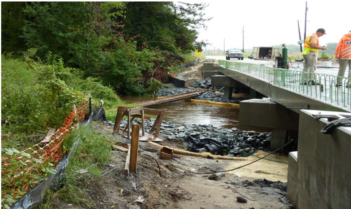
Bridge Replacement Work, Pitt County
