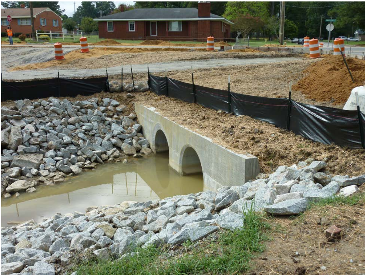
Culvert and Stream Protection, Kingston Ave Widening
