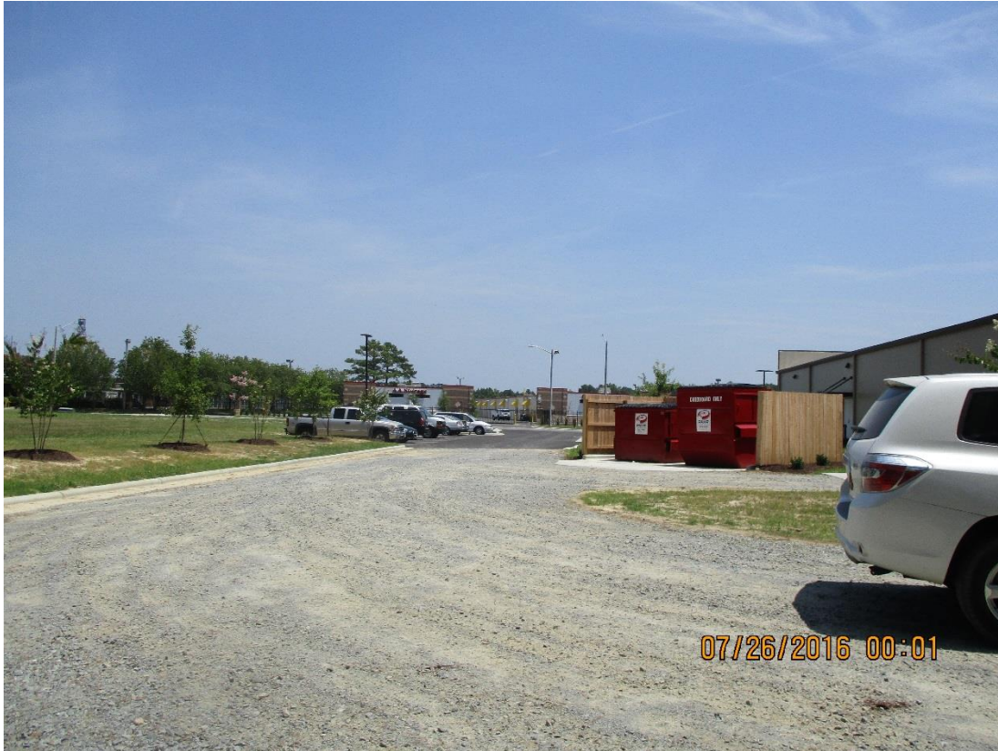
Site 3 – Groundcover establishment underway on completed site.
