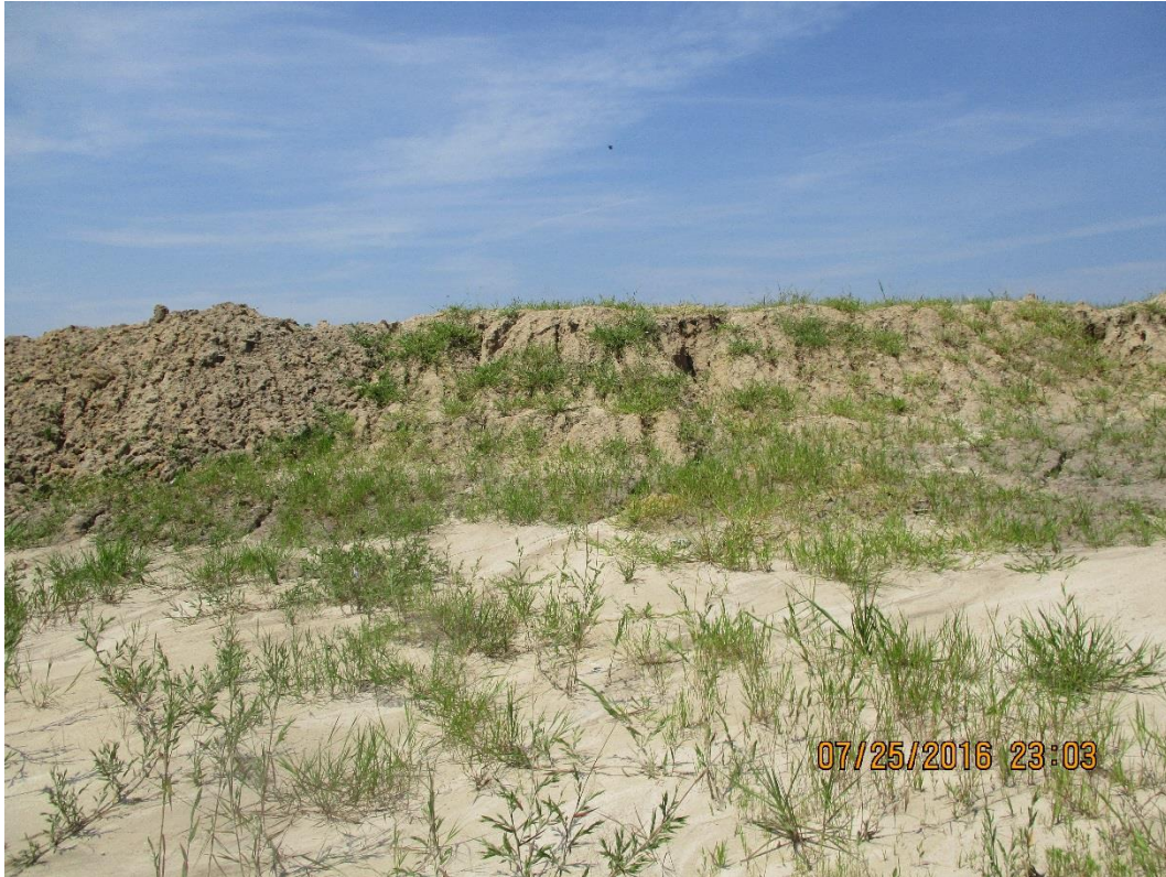
Site 1 – Poor groundcover observed on eroding stockpile areas.
