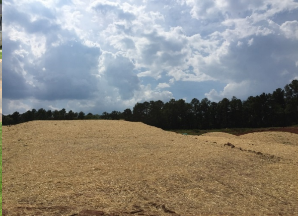
Figure 4 - Example of Good Application of Ground Cover
