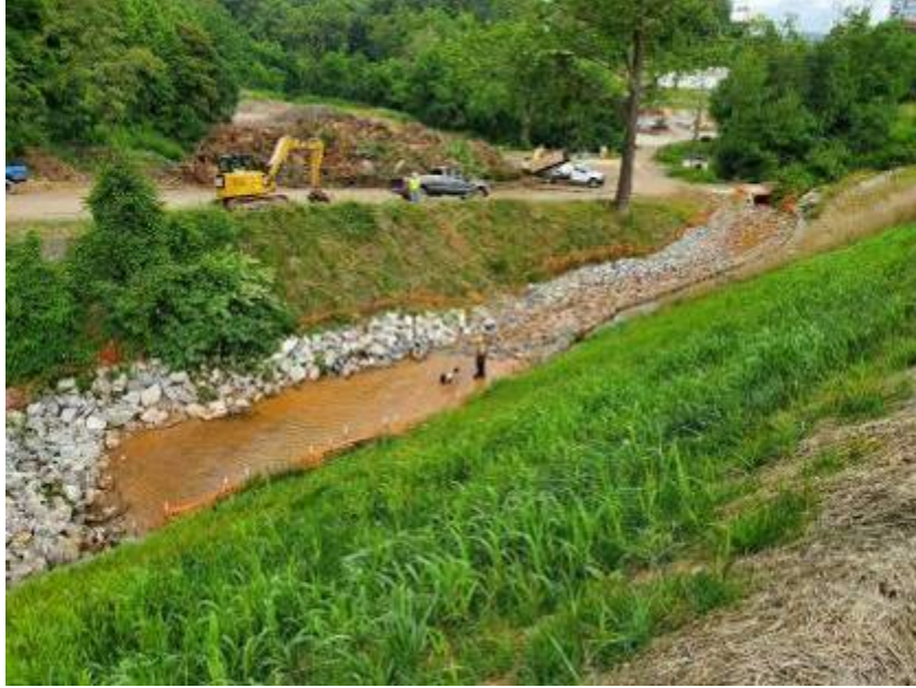
Photo - Pumping offsite sedimentation out of creek. (6/25/2019)
