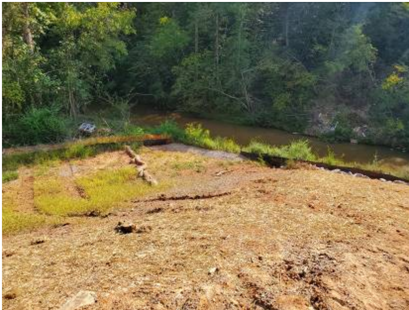
Photo - Slope above outlet in need for more straw and seeding. (9/12/19)
