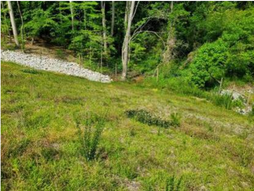
Photo - Riprap Diversion Ditch (5/16/2019)
