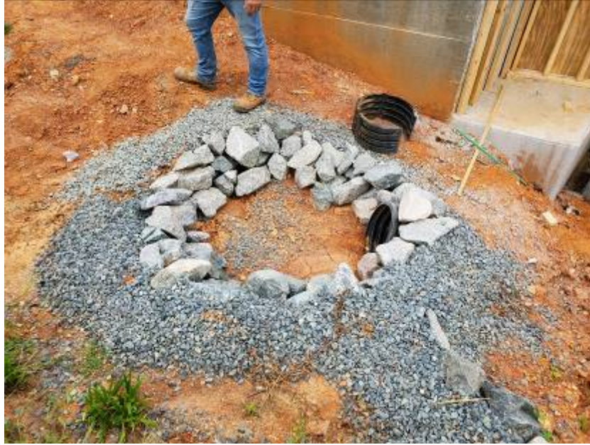
Photo - Slope drain protection. (9/5/2019)
