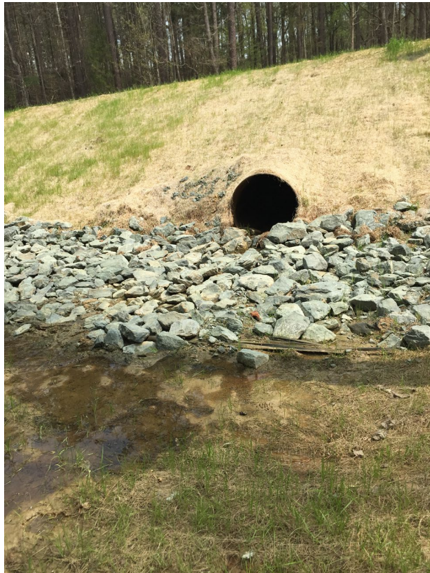
Photo - Culvert outlet. (4/5/2019)
