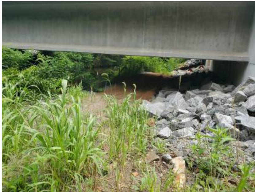
Photo - Well maintained measures underneath new bridge. (6/25/2019)
