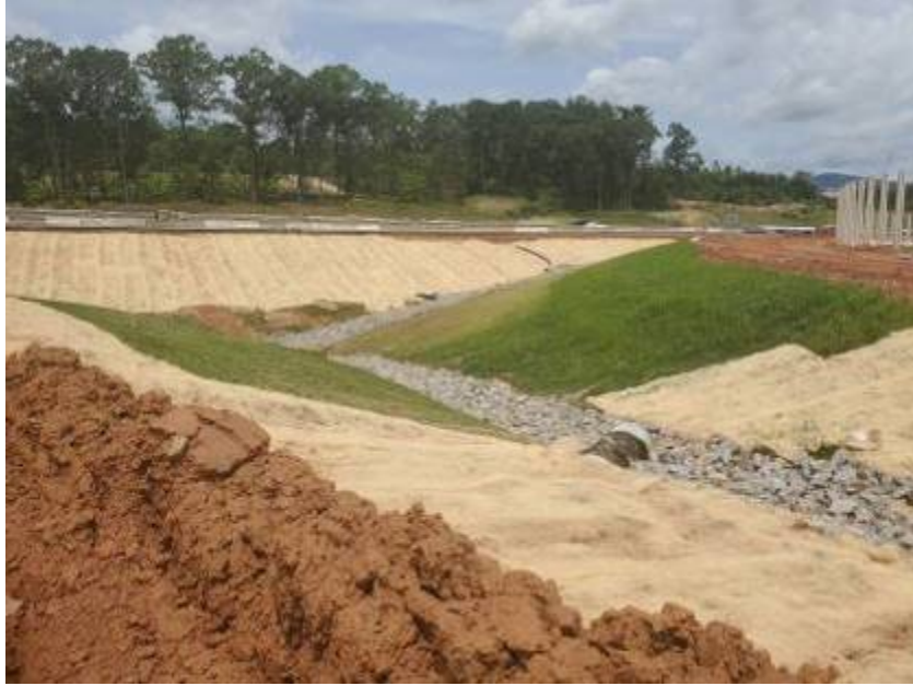
Photo - Good stabilization on slopes and well-maintained channel. (6/25/2019)
