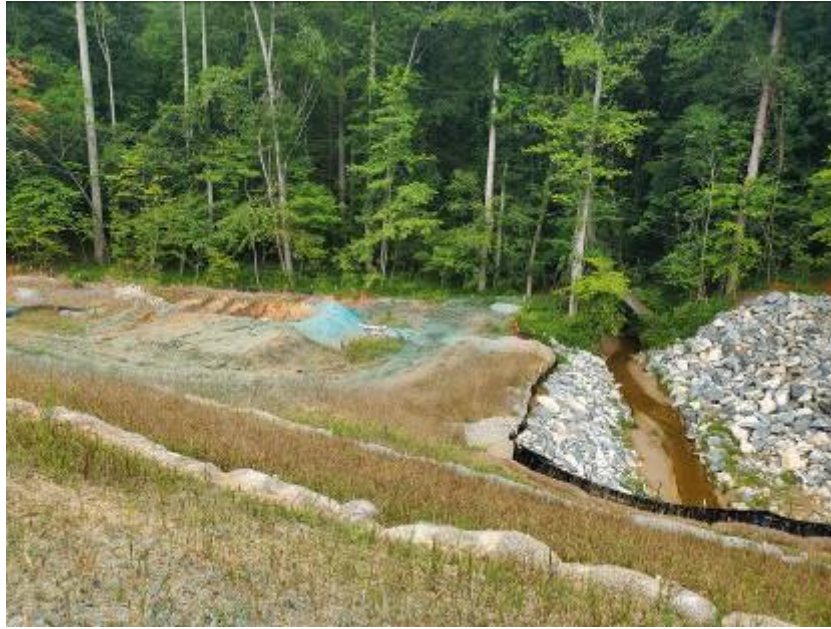
Photo - Skimmer basin outlet to well protected creek. (8/7/2019)
