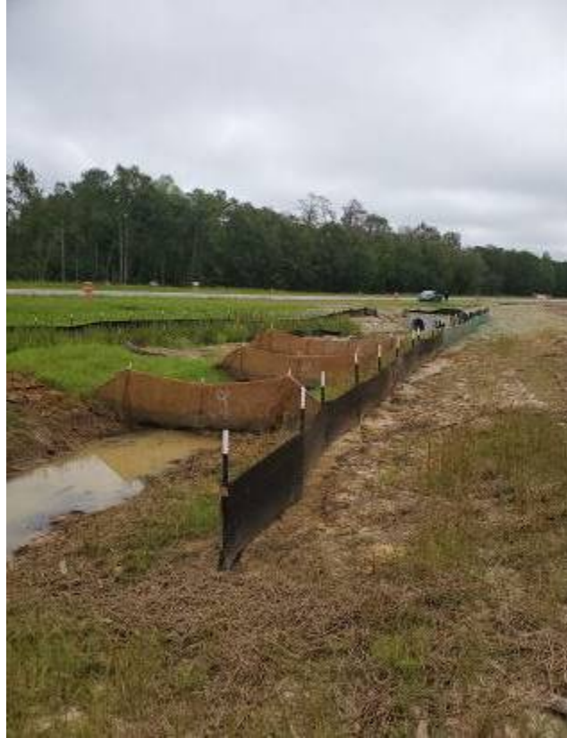
Photo -Well maintained skimmer diversion ditch. (8/27/2019)
