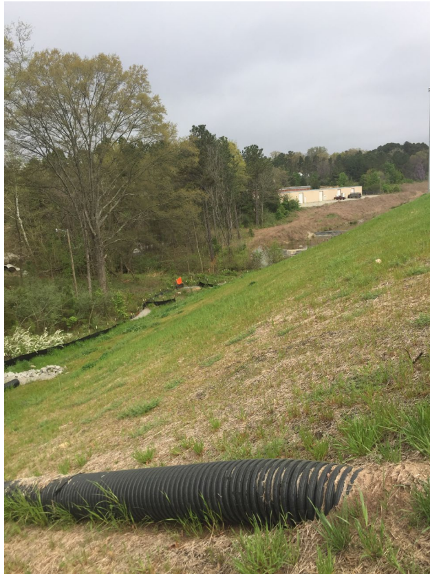
Photo - Good vegetation on slope and diversion ditch w/ check dams. (4/5/2019)
