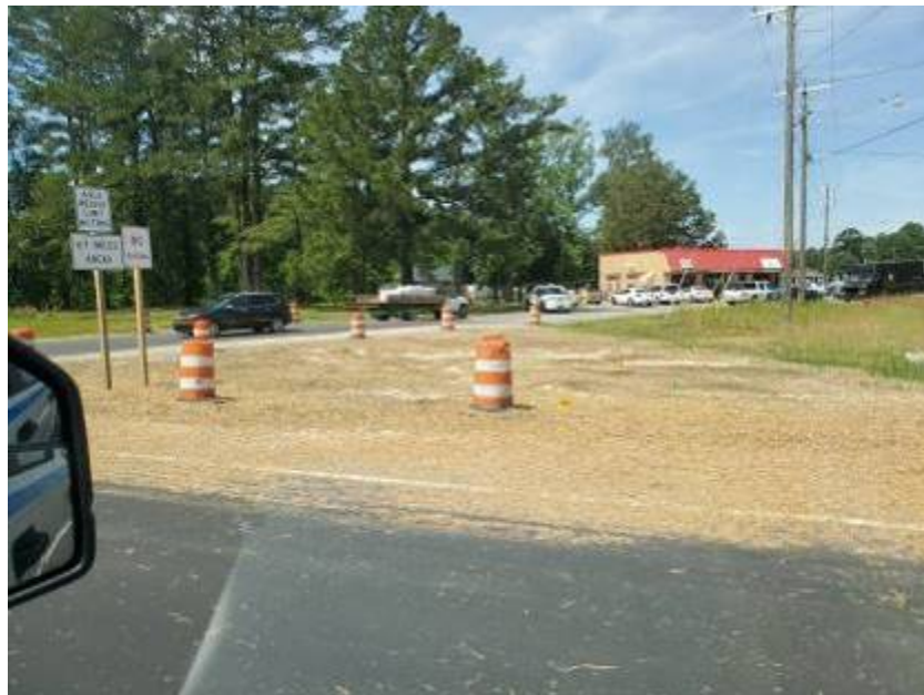
Photo - Straw and Tack with Bare Patches. (5/16/2019)
