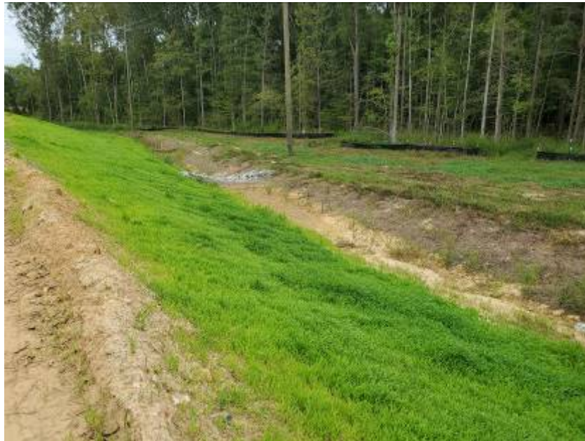
Photo - Well maintained diversion ditch and good slope stabilization. (9/5/2019)
