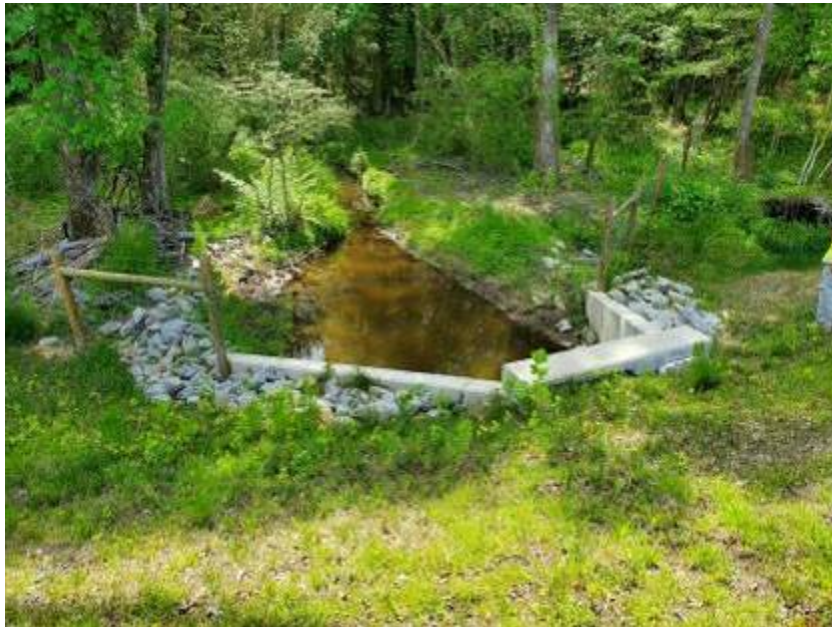
Photo - Culvert with Good Vegetation and Maintained Stone. (5/16/2019)
