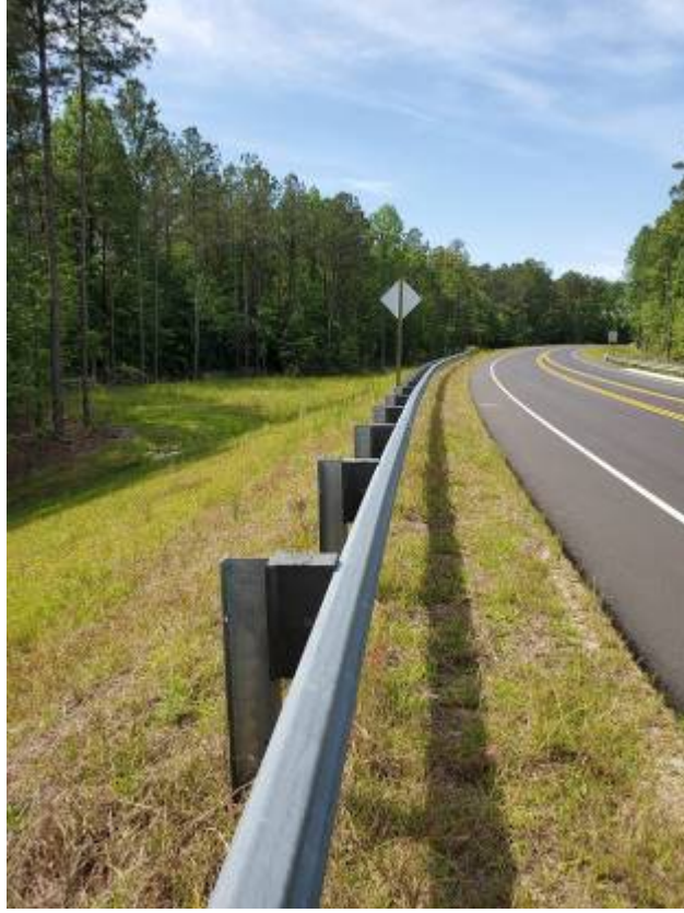
Photo - Roadside Slope with Good Vegetation. (5/16/2019)
