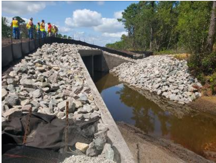
Photo - Stream box culvert. (8/27/2019)
