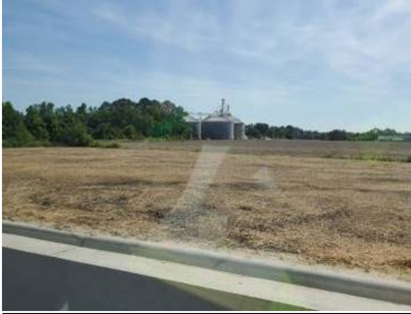
Photo - Straw and Tack Coverage. (5/16/2019)
