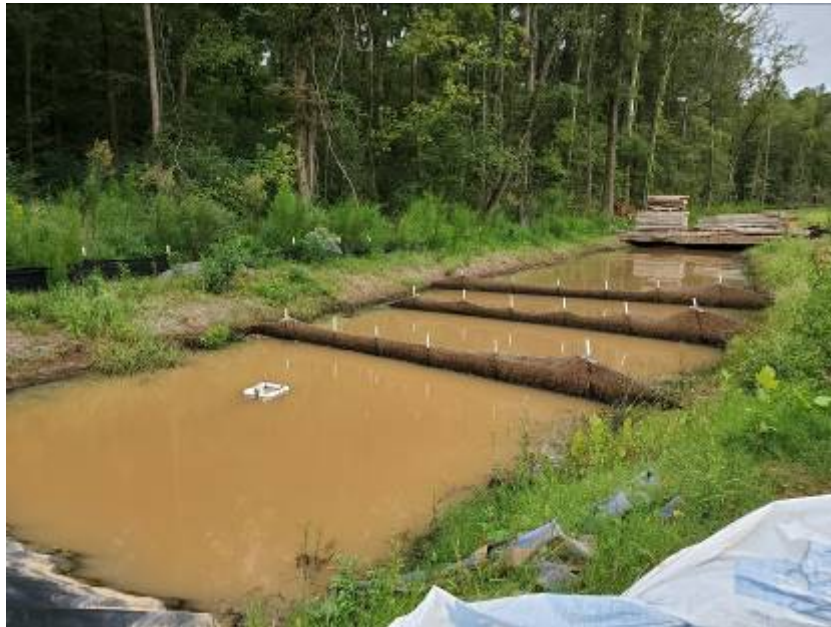
Photo - Well maintained skimmer basin. (9/5/2019)
