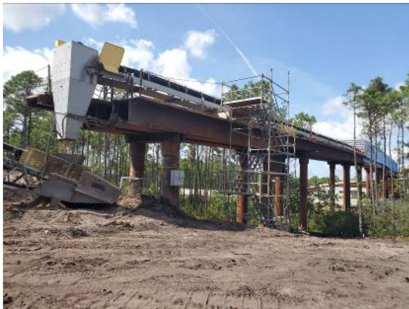
Photo - Conveyor bring soil from borrow pit to site. (8/27/2019)
