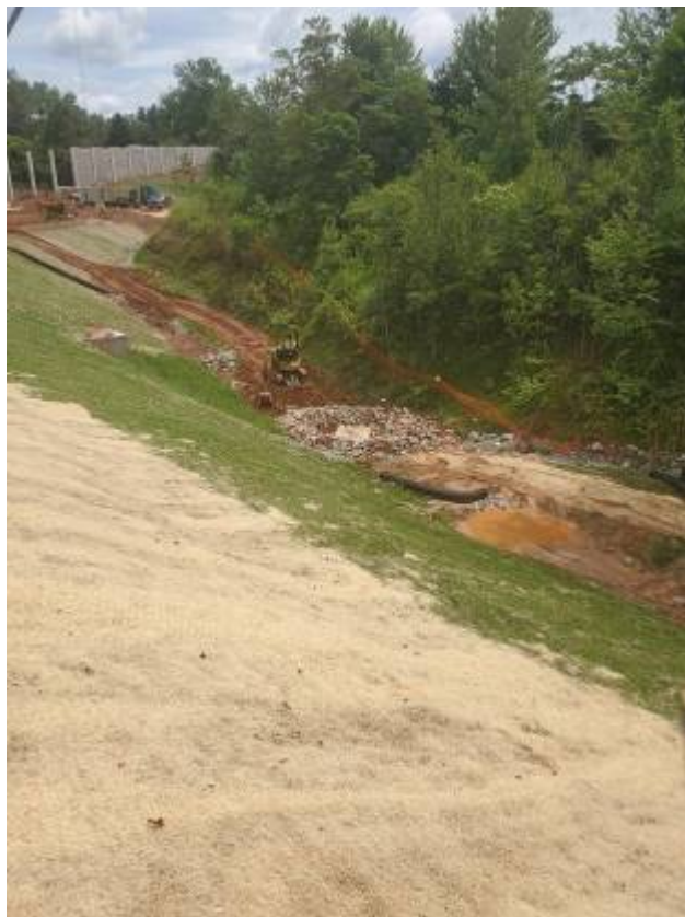
Photo - Increasing control measures. (6/25/2019)
