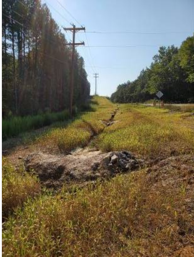
Photo - Well maintain diversion ditch with check dams (9/12/19)
