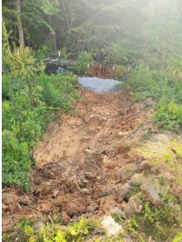
Photo - Unprotected soil between skimmer basin outlet and silt fence outlet. (8/7/2019)
