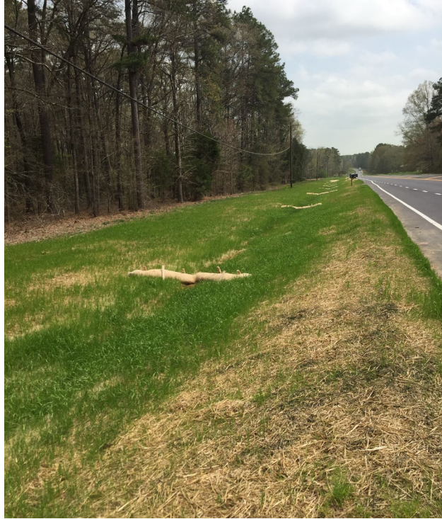
Photo - Good ground cover in permanent diversion ditch. (4/5/2019)
