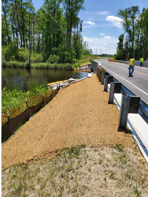
Photo - Good temporary ground cover on the slope. (5/16/19)
