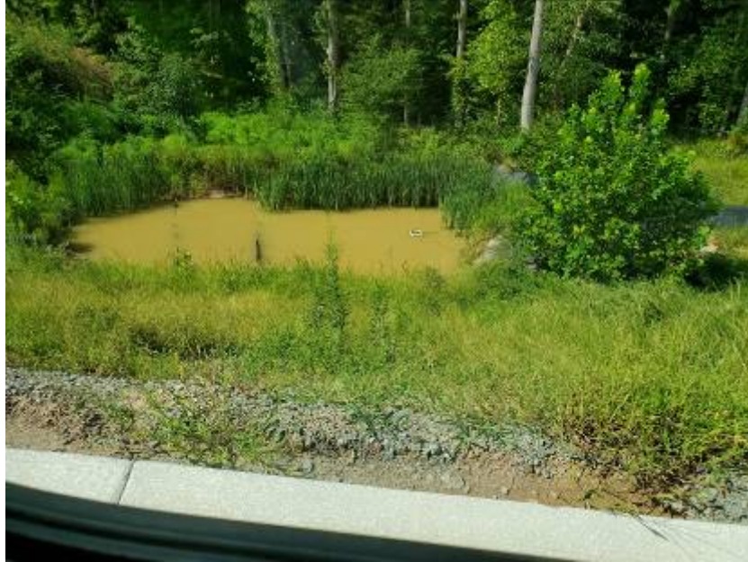
Photo - Skimmer basin with well-established groundcover on embankments. (8/28/2019)
