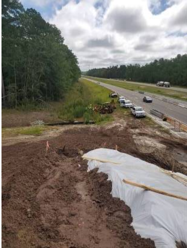
Photo - Bucket crew cleaning up slight offsite sediment. (8/27/2019)
