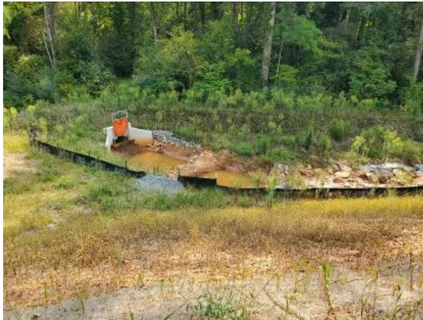
Photo - Well maintained diversion channel and forebay. (9/18/19)
