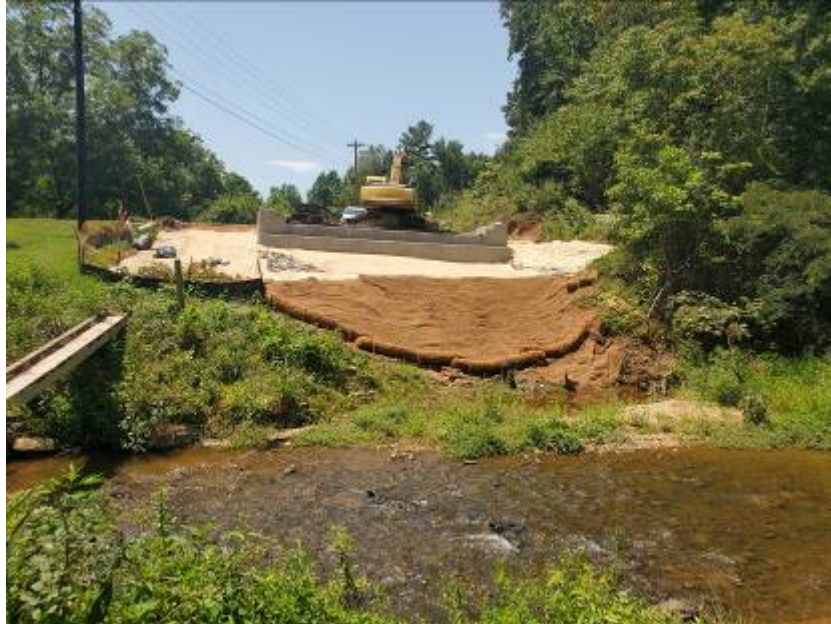
Photo - Slope protected with matting. (8/7/2019)
