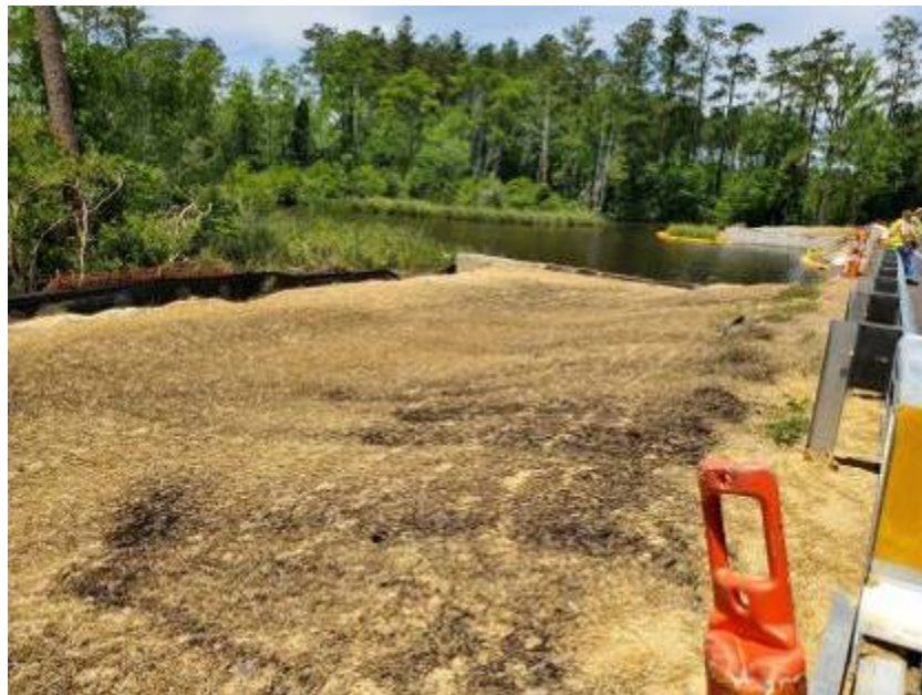
Photo - straw and tack on fill slope. (5/16/19)
