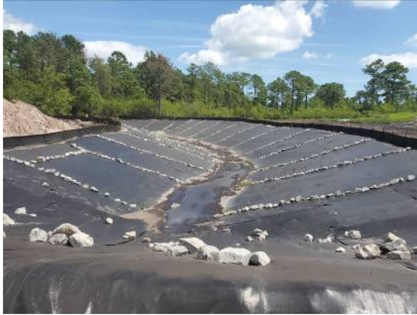
Photo - Stream diversion channel. (8/27/2019)
