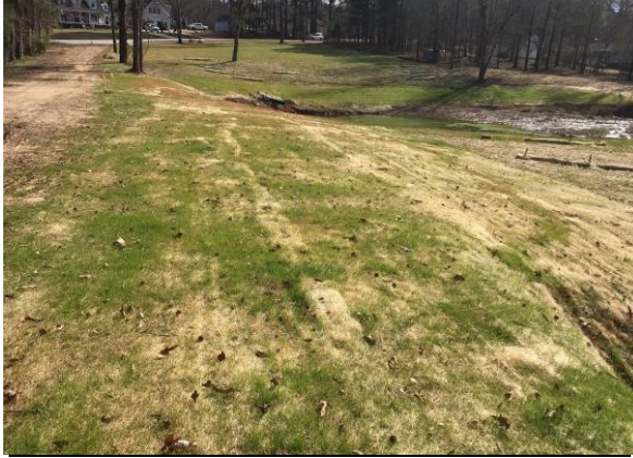
1. Most of disturbed areas stabilized.
