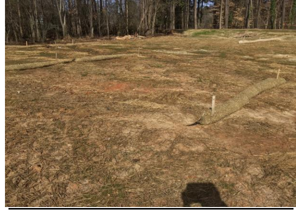
2. Area where matting may need to be installed to establish ground cover.
