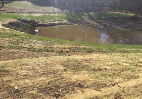
1. Most of disturbed areas stabilized.
