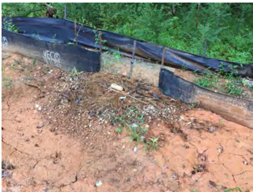
Comment: refresh stone at silt fence outlet left of lot 90
