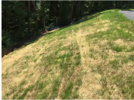
Comment: Slope stabilized
