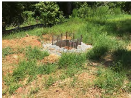
Comment: inlet protection installed
