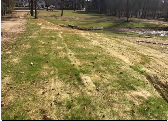
1. Most of disturbed areas stabilized.
