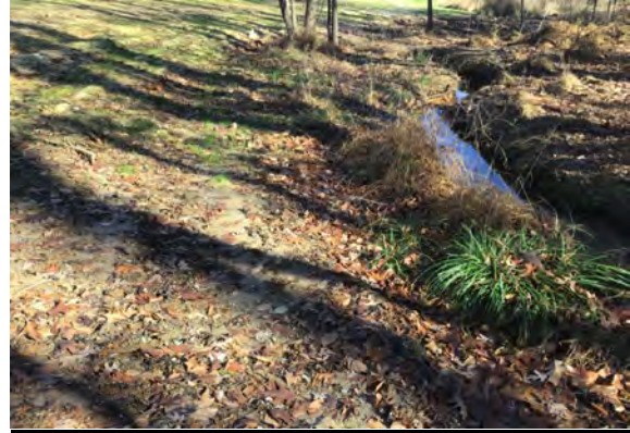
2. Small area near stream needs better ground cover.
