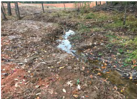
5. Damage to unclassified stream on site.
