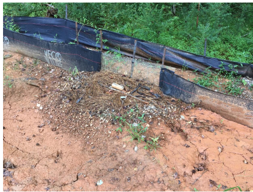
Comment: refresh stone at silt fence outlet left of lot 90
