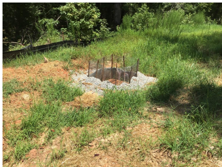
Comment: inlet protection installed
