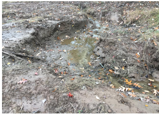
6. Damage to unclassified stream on site.
