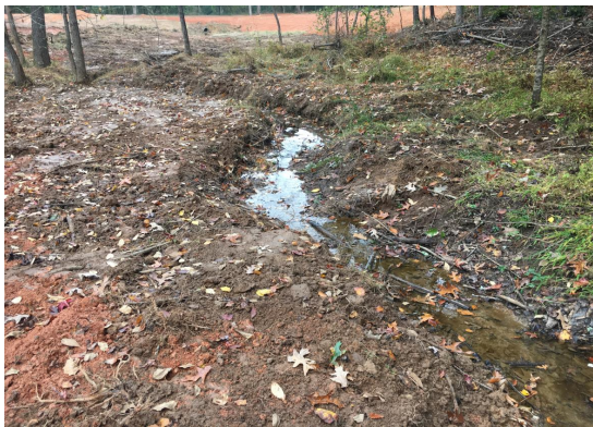
5. Damage to unclassified stream on site.
