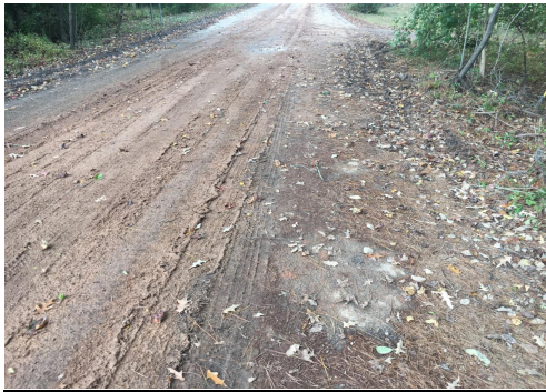
7. Mud tracked onto road
