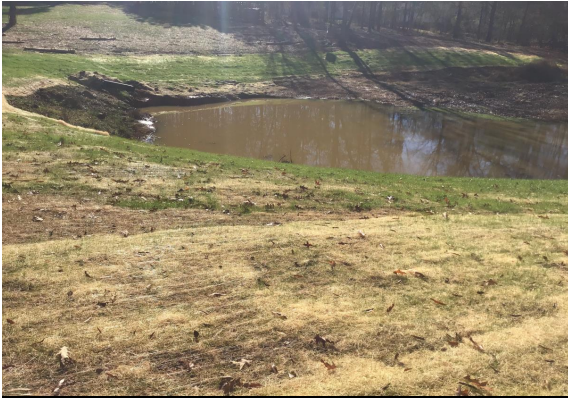
1. Most of disturbed areas stabilized.
