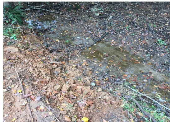
4. Damage to unclassified stream on site.
