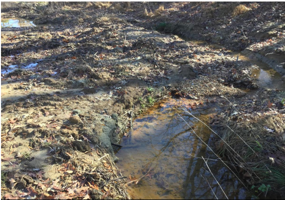
3. Small area near stream needs better ground cover.
