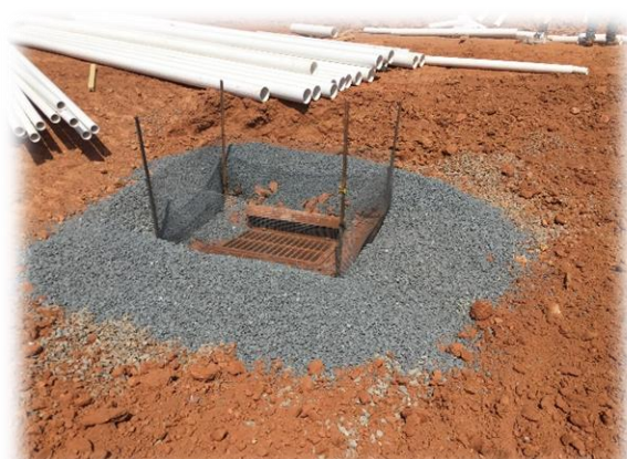
Figure 13 - Good Inlet Protection
