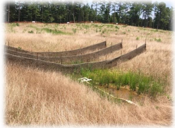
Figure 12 - Good Vegetative Stabilization
