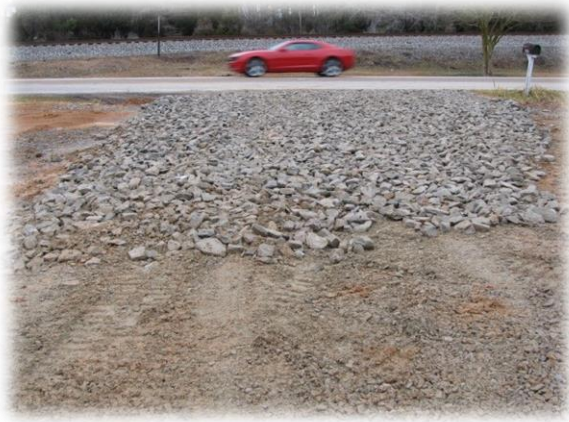
Figure 7 - Good Construction Entrance
