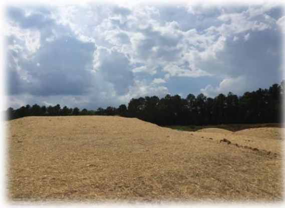
Figure 9 - Good Application of Ground Cover
