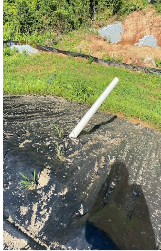
Skimmer basin and outlet pipe
