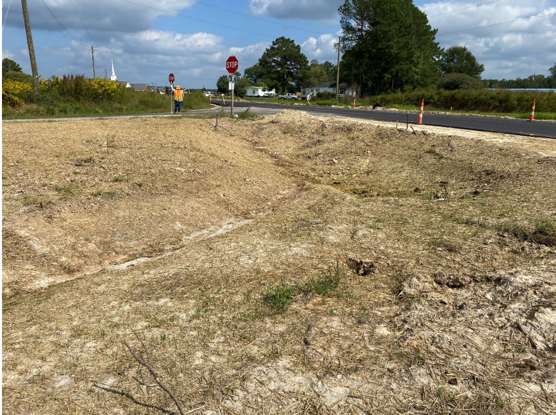
Recently graded area with straw mulch
