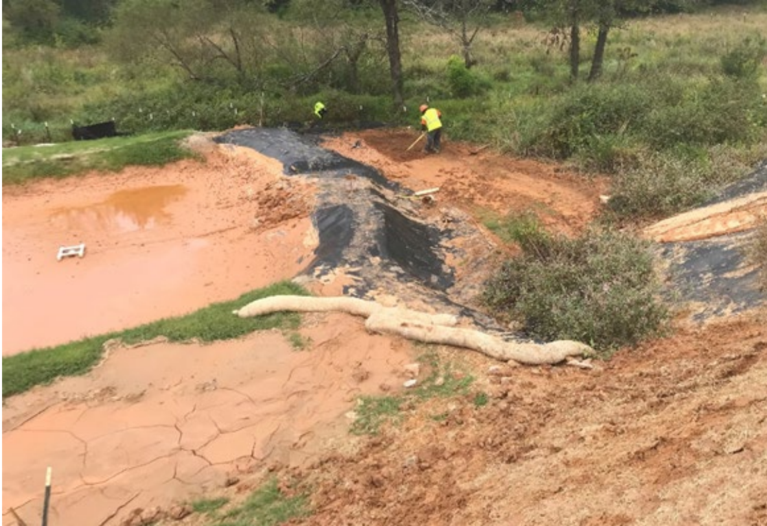
Basin west of Swift Creek repairs underway (9/29/23 follow up)
