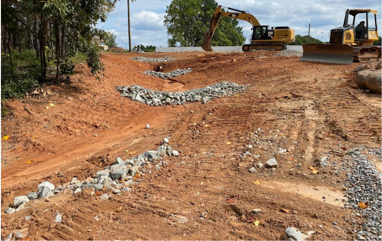
Check dams installed
