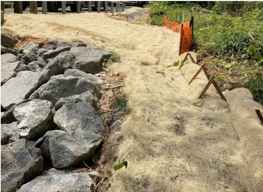
Recently completed areas being stabilized
