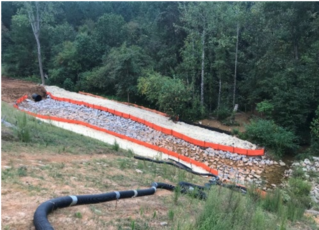
Channel repaired and stabilized (9/29/23 follow up)
