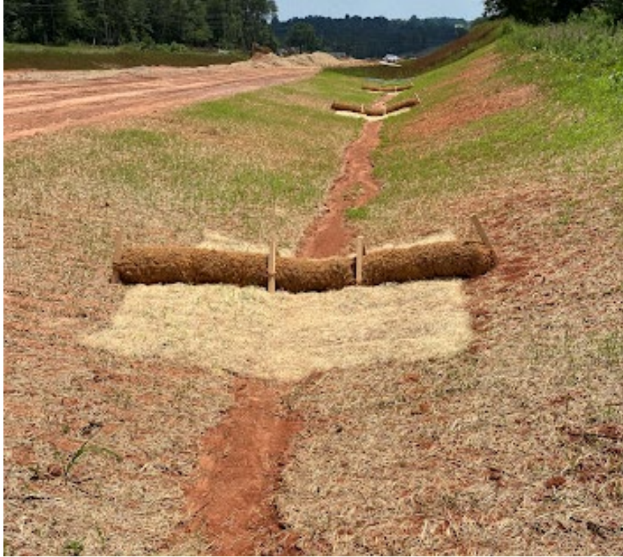
Wattles with PAM installed
