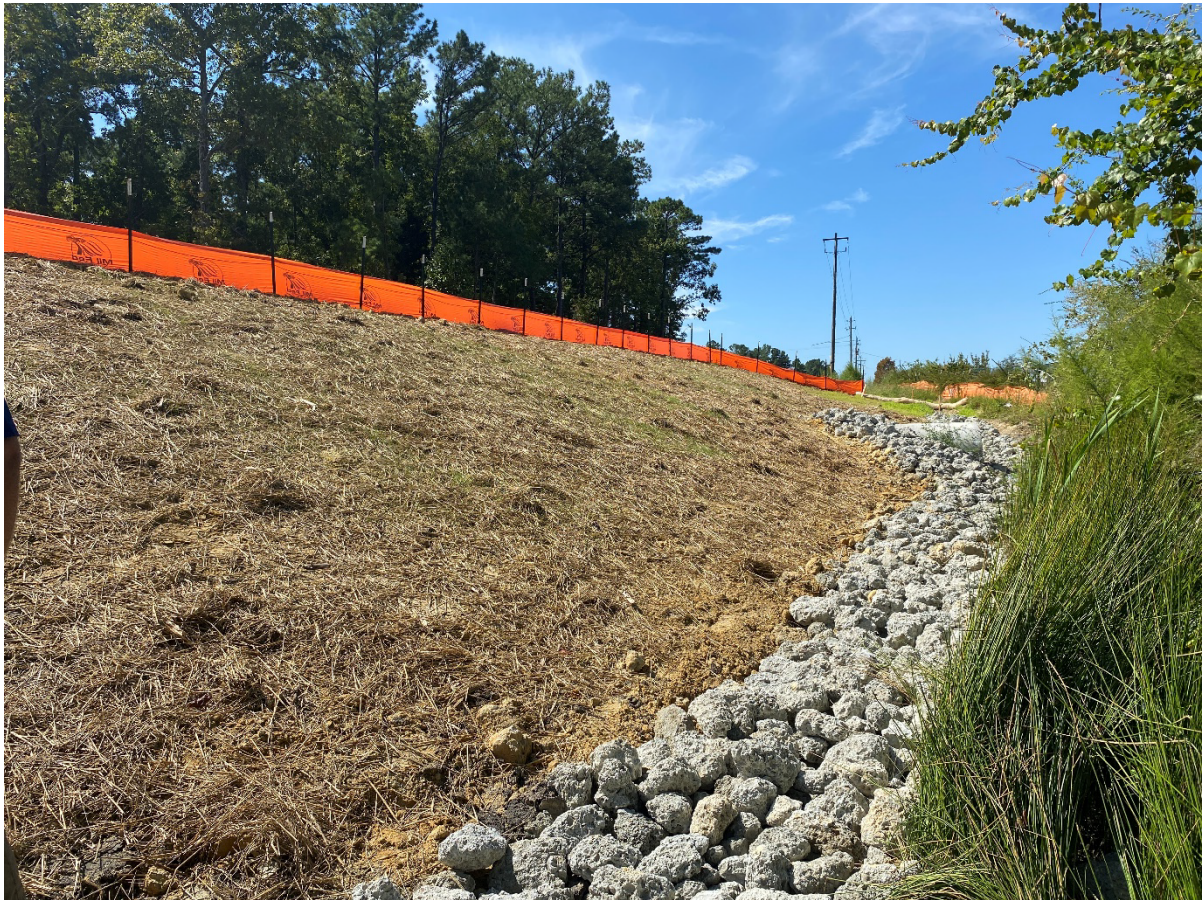
Completed permanent ditch and slope being stabilized
