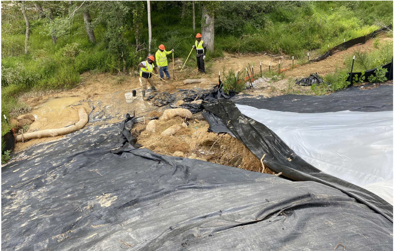
Basin berm east of Swift Creek
