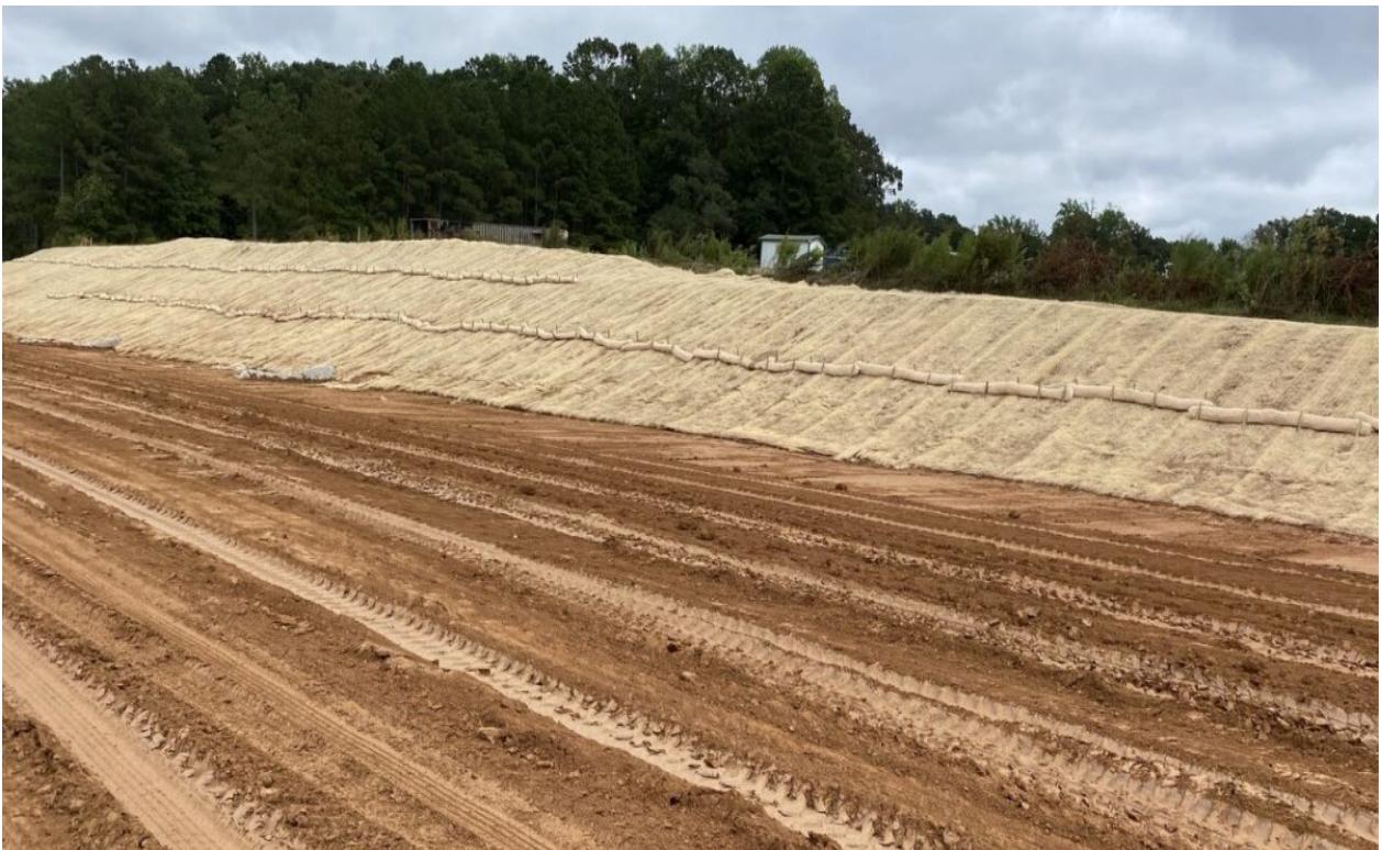
Slopes matted and wattle breaks installed
