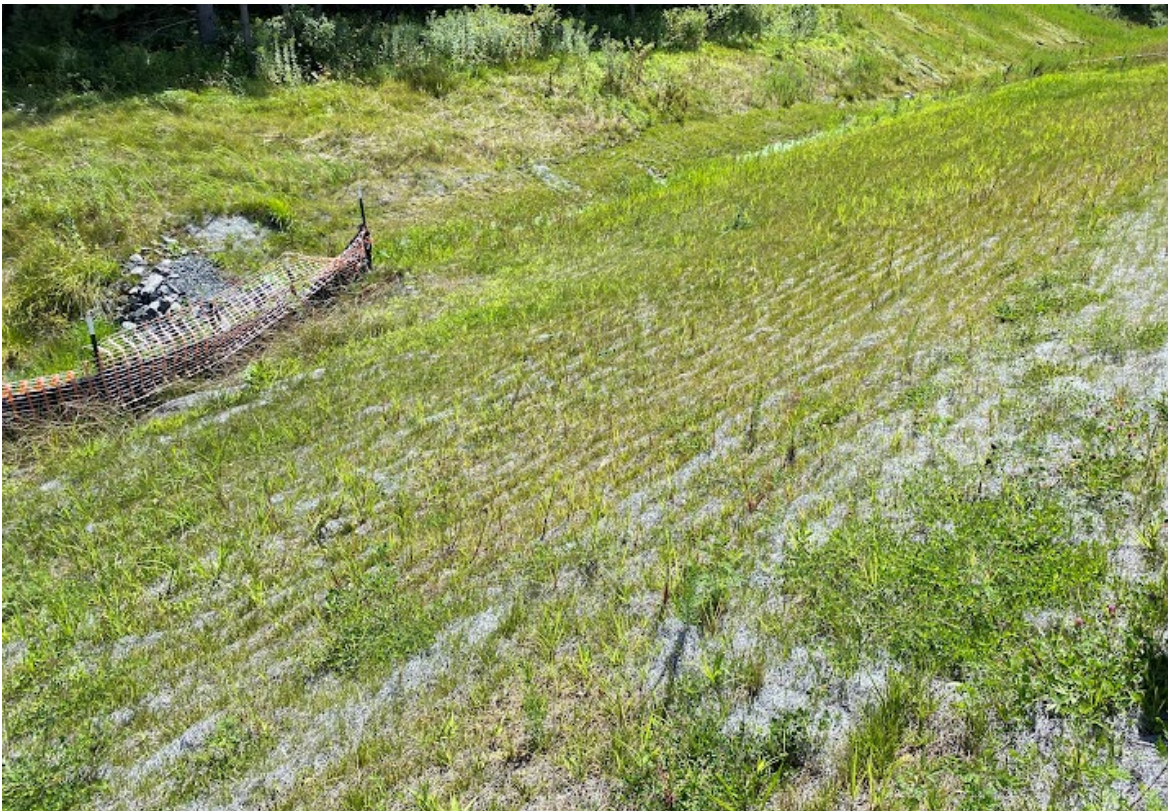
Vegetation establishing on slope
