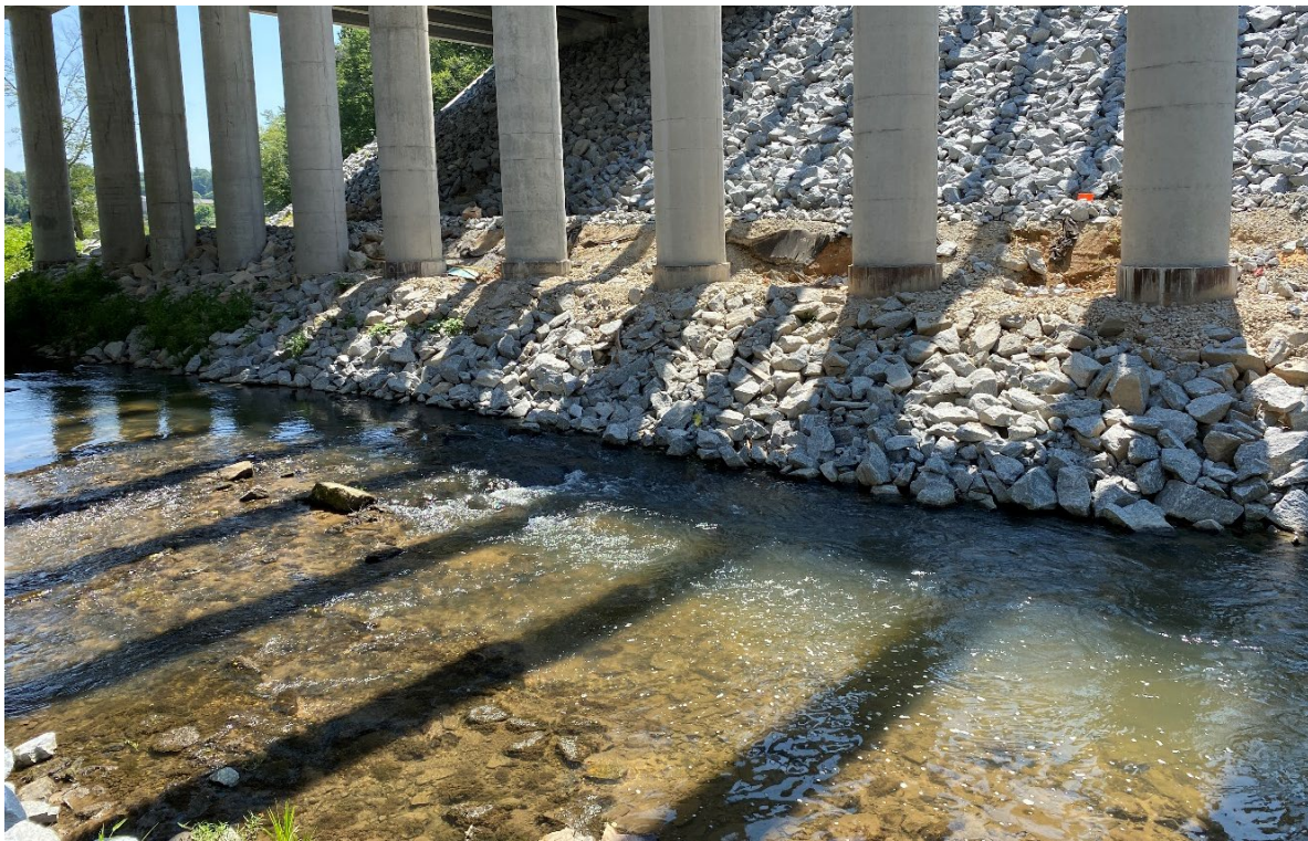
Stream bank stabilization under new bridge
