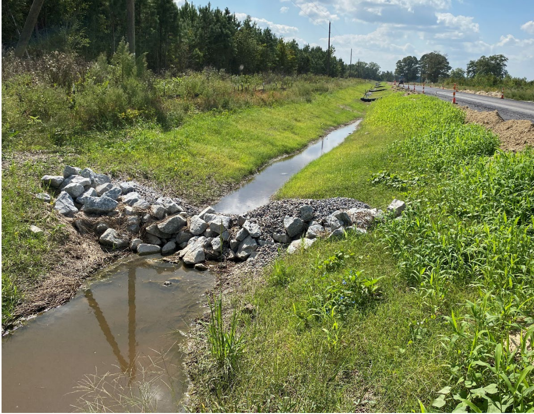
Roadside ditch with vegetation establishing
