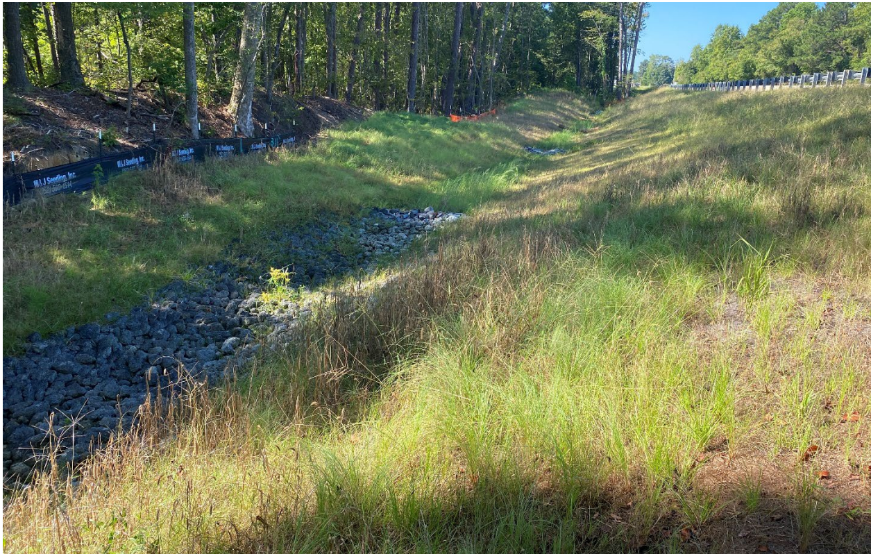
Stabilized ditch adjacent to detour bridge
