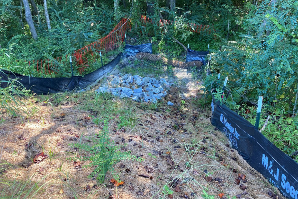
Maintained and stabilized outlet
