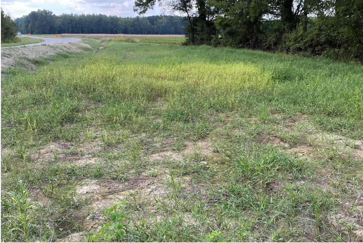
Roadway realignment complete and area stabilized
