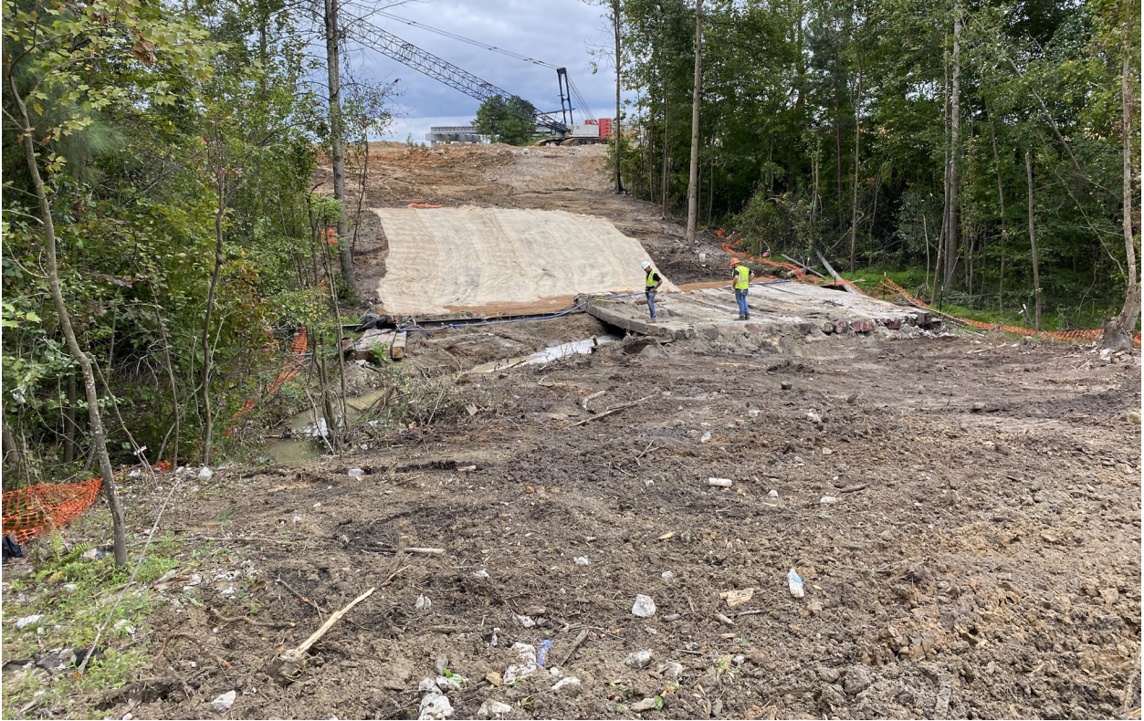
Stream where bridge demolition had occurred
