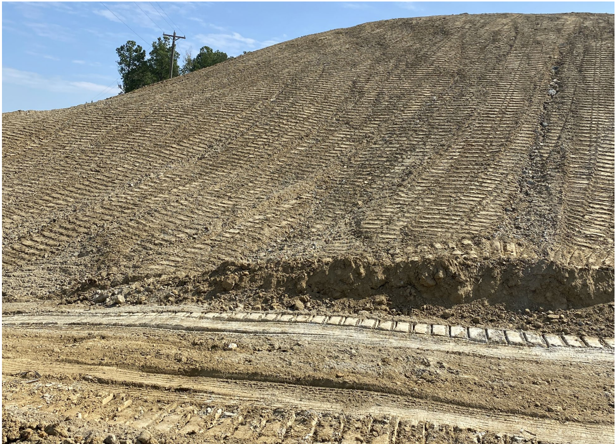
Stockpile on waste site awaiting stabilization
