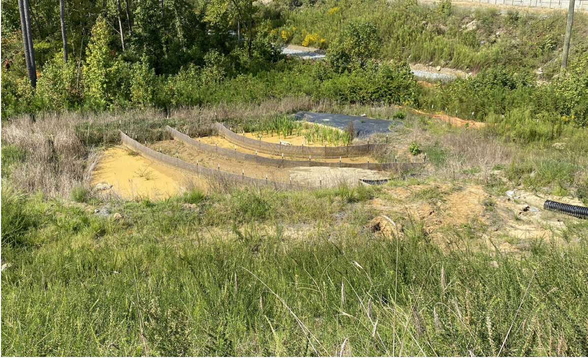
Slope drain in second bay of waste site basin
