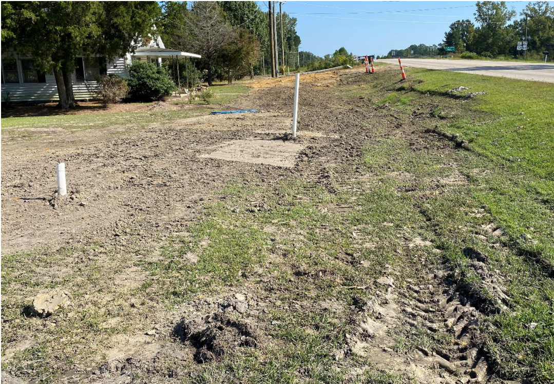
Utilities by Others being installed
