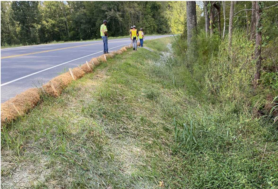
Wattles that were added in preparation for rain event as slope was being stabilized
