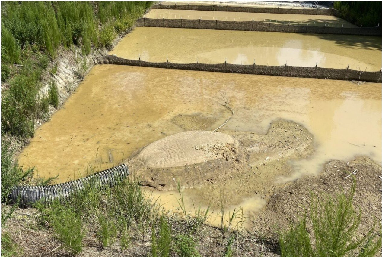
Skimmer basin on waste site
