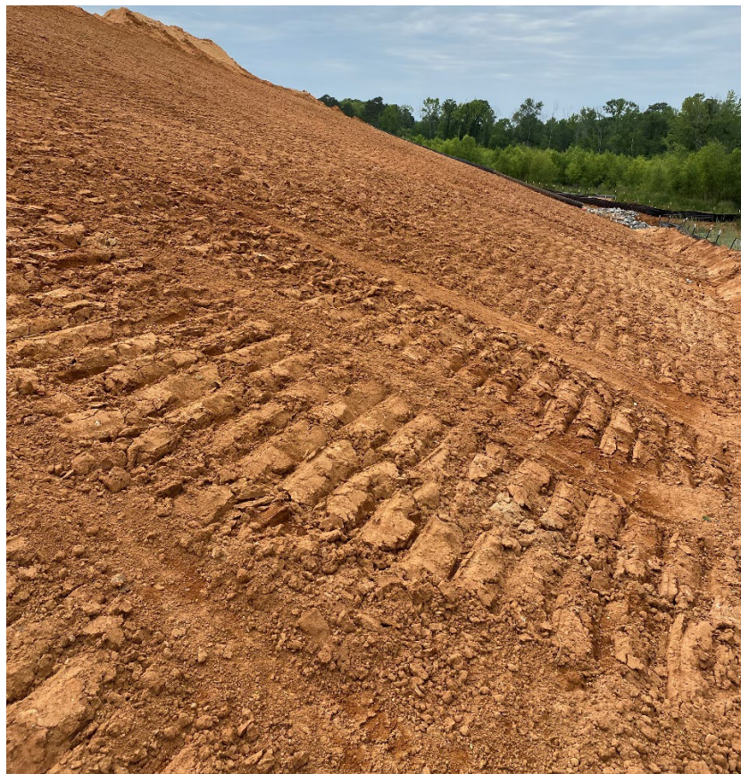
Recently graded slopes tracked properly
