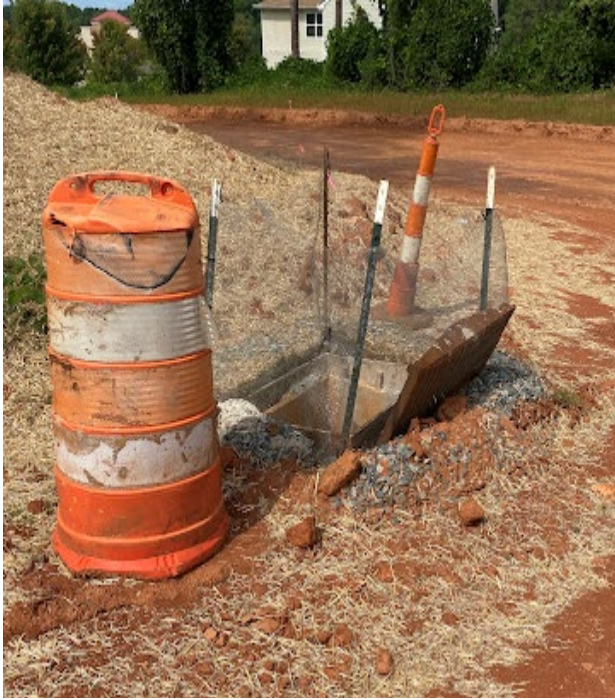
Inlet protection measures
