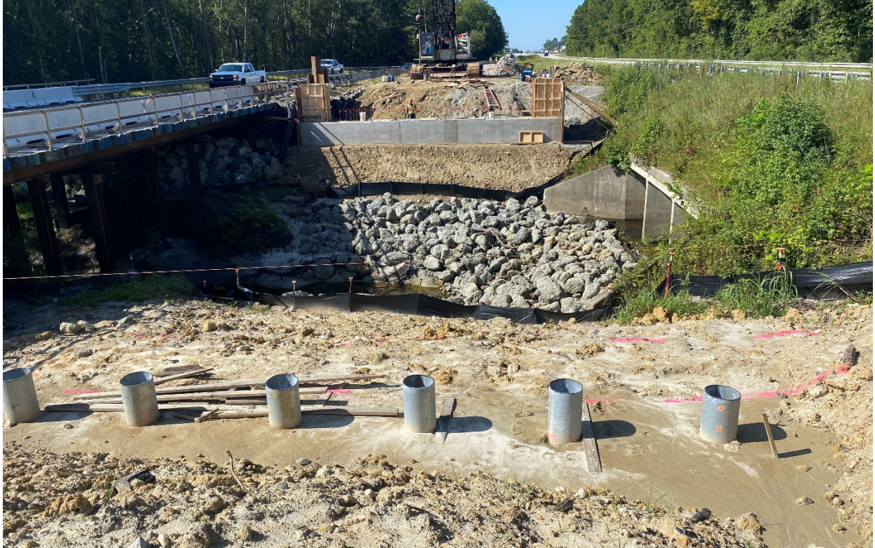
Stream banks lined with riprap and new bridge foundations being installed
