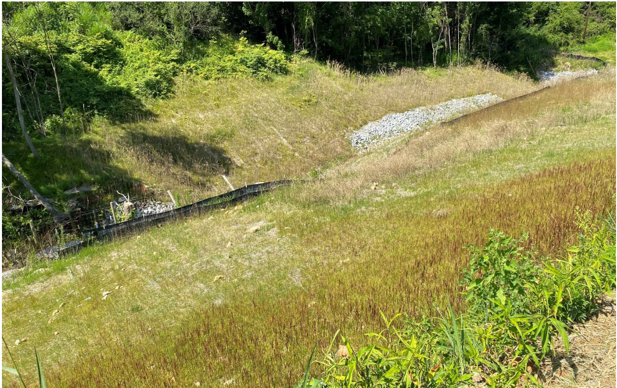
Channel change completed and area stabilized
