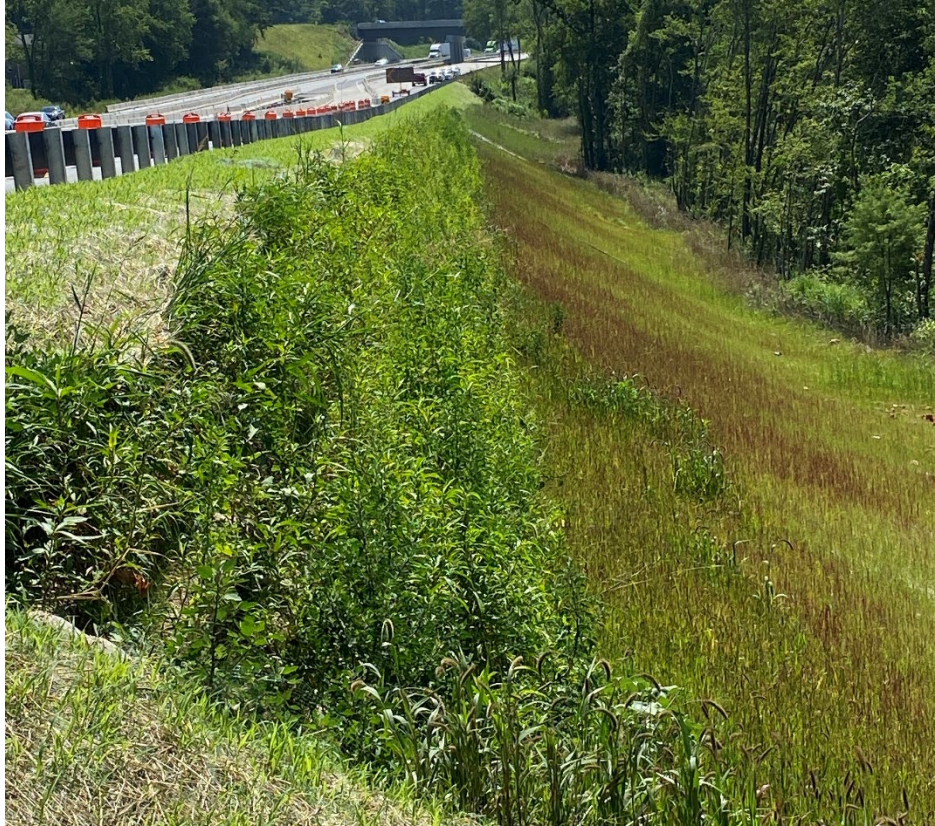
Living retaining wall installed and slopes stabilized
