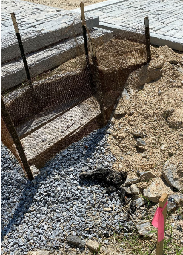
Drop inlet protection measure needing maintenance
