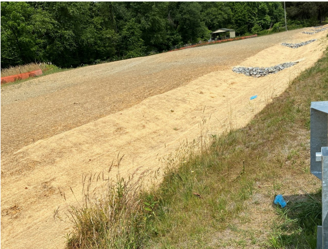
Staging Area seeded and mulched with straw
