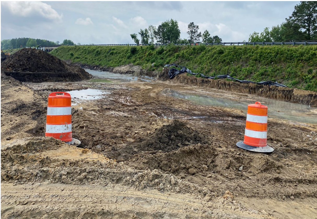
Area being dewatered and pumped into basin
