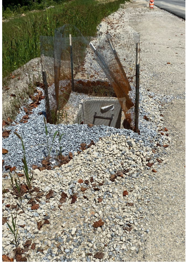
Drop inlet protection measure needing maintenance
