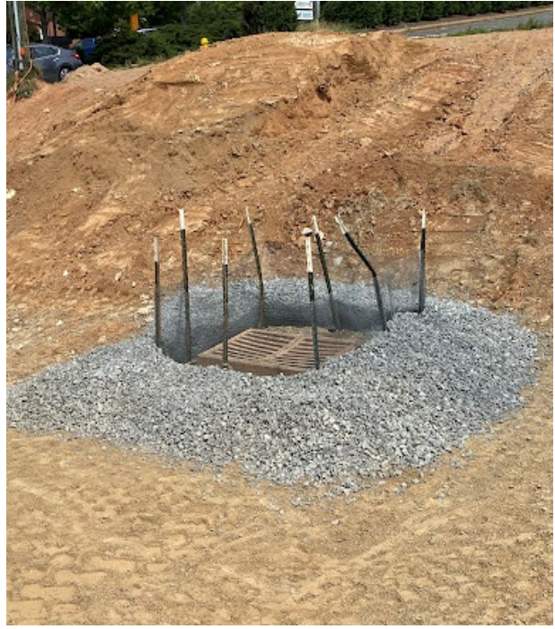
Inlet protection measures
