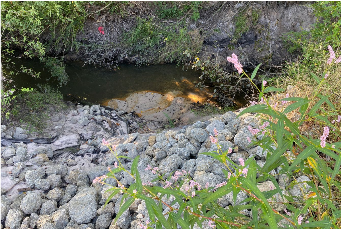
Sediment loss into stream
