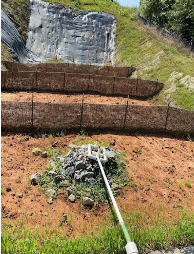
Skimmer basin and outlet pipe
