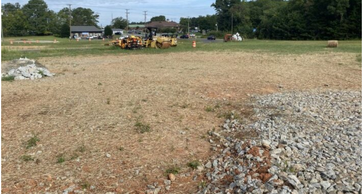
Laydown yard area being stabilized
