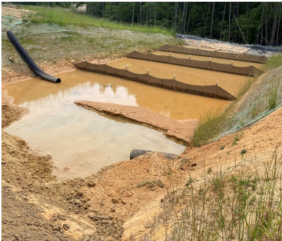
Skimmer basin at Borrow Pit
