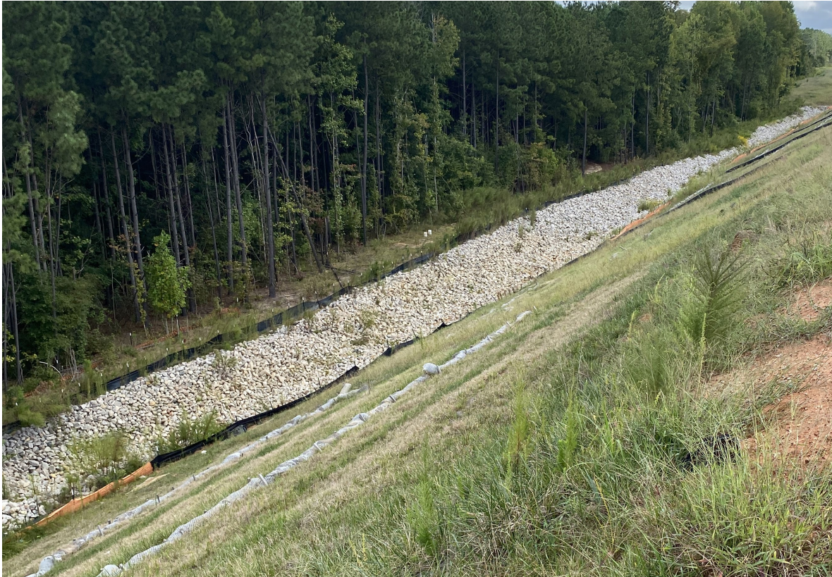
Completed slope and channel change
