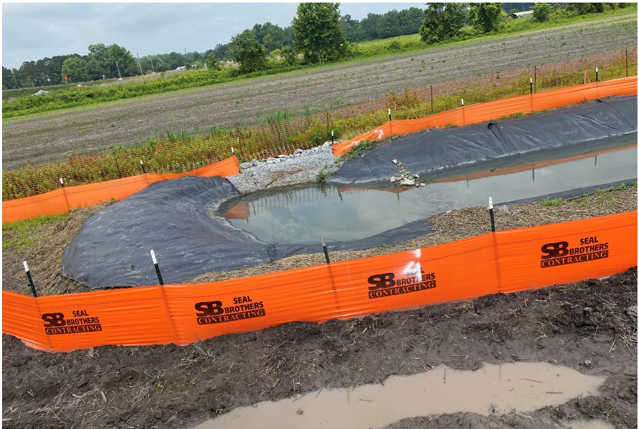
Basin and stabilized outlet on Borrow site
