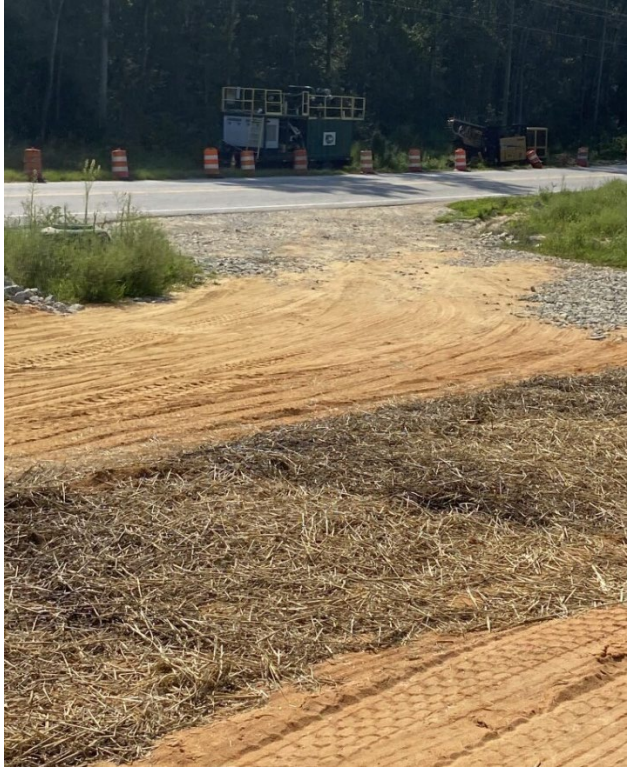
Construction entrances needing maintenance
