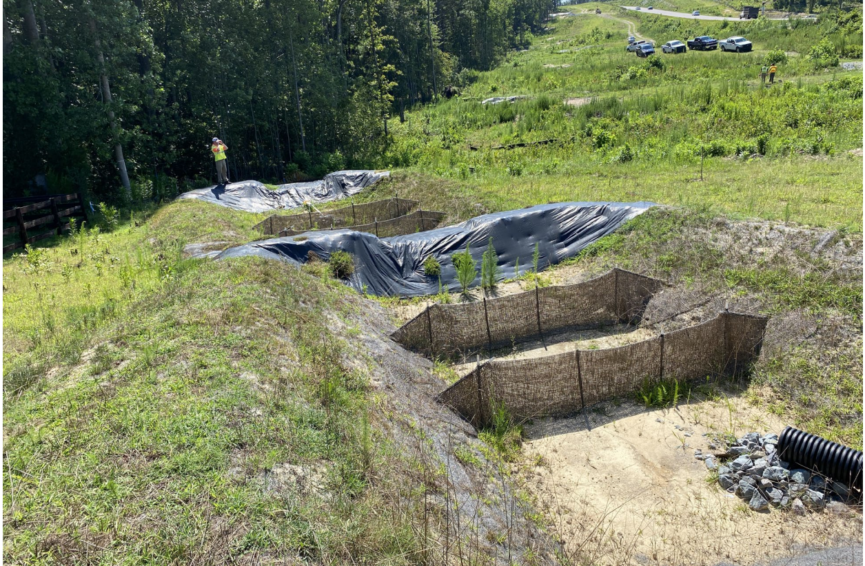
Tiered basin installed and cleared area stabilized
