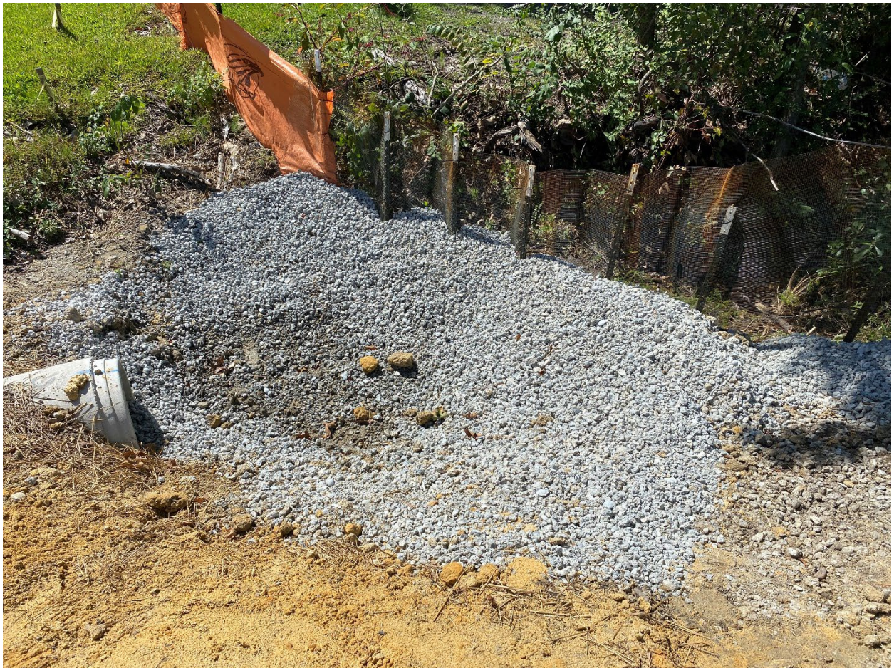
Silt fence outlets maintained
