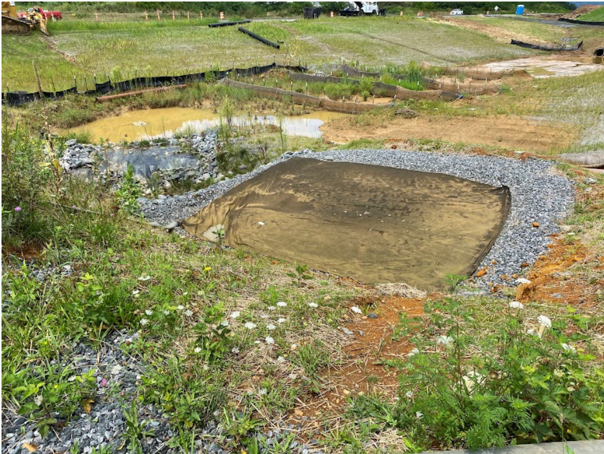
Special stilling basin (silt bag) for dewatering basin being converted
