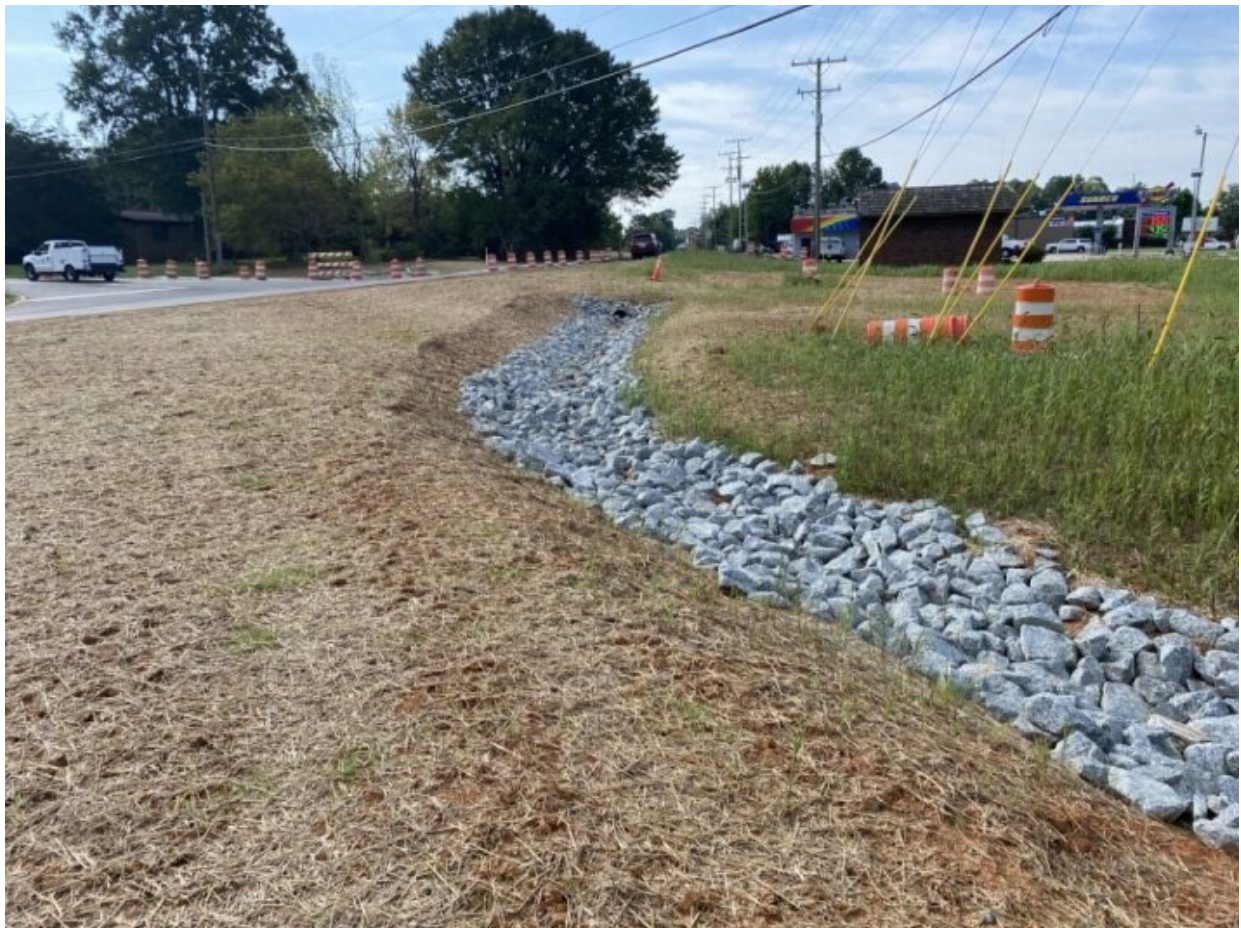
Permanent ditch completed and area being stabilized
