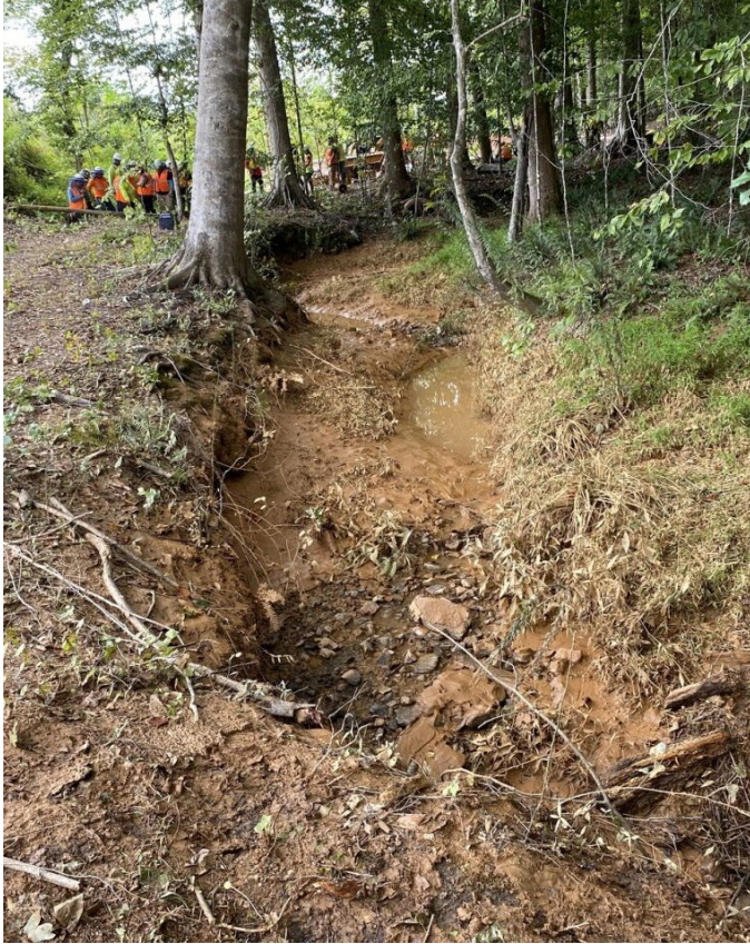
Sediment loss into stream adjacent to channel change
