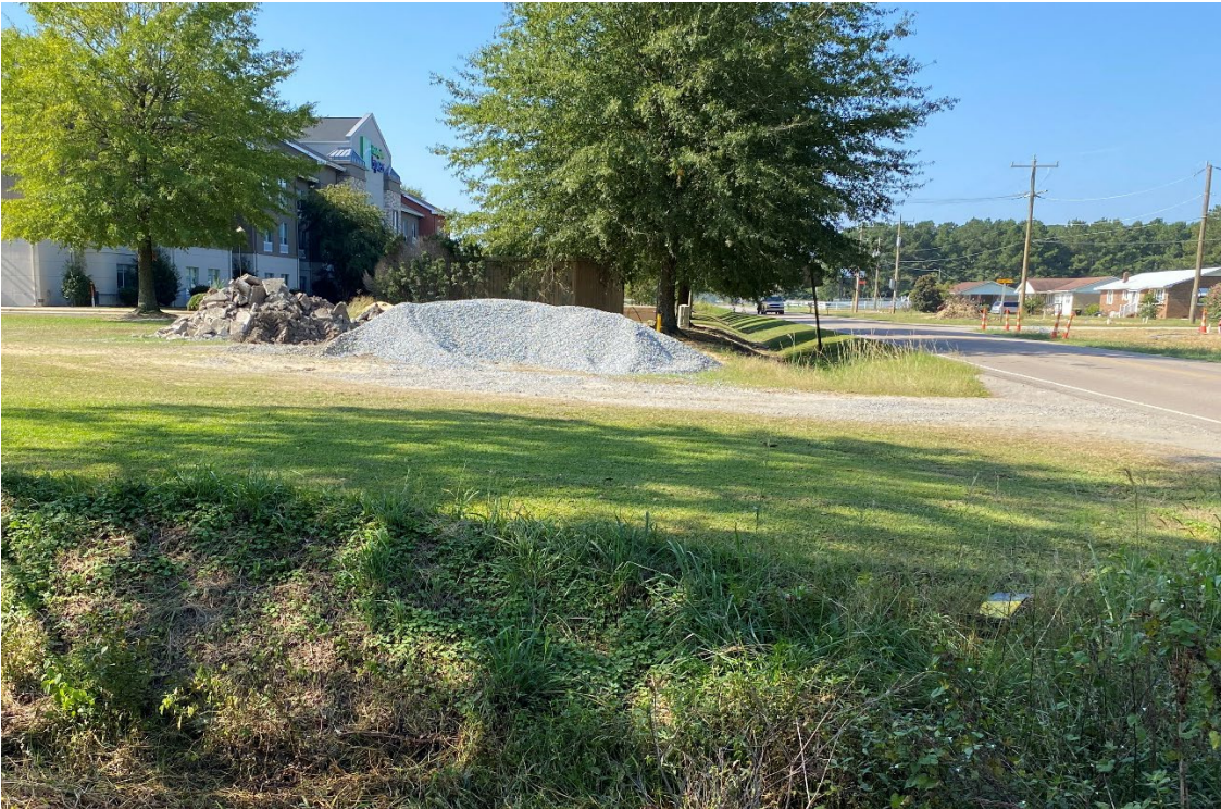
Stone and debris stockpiled outside of ROW and Easements
