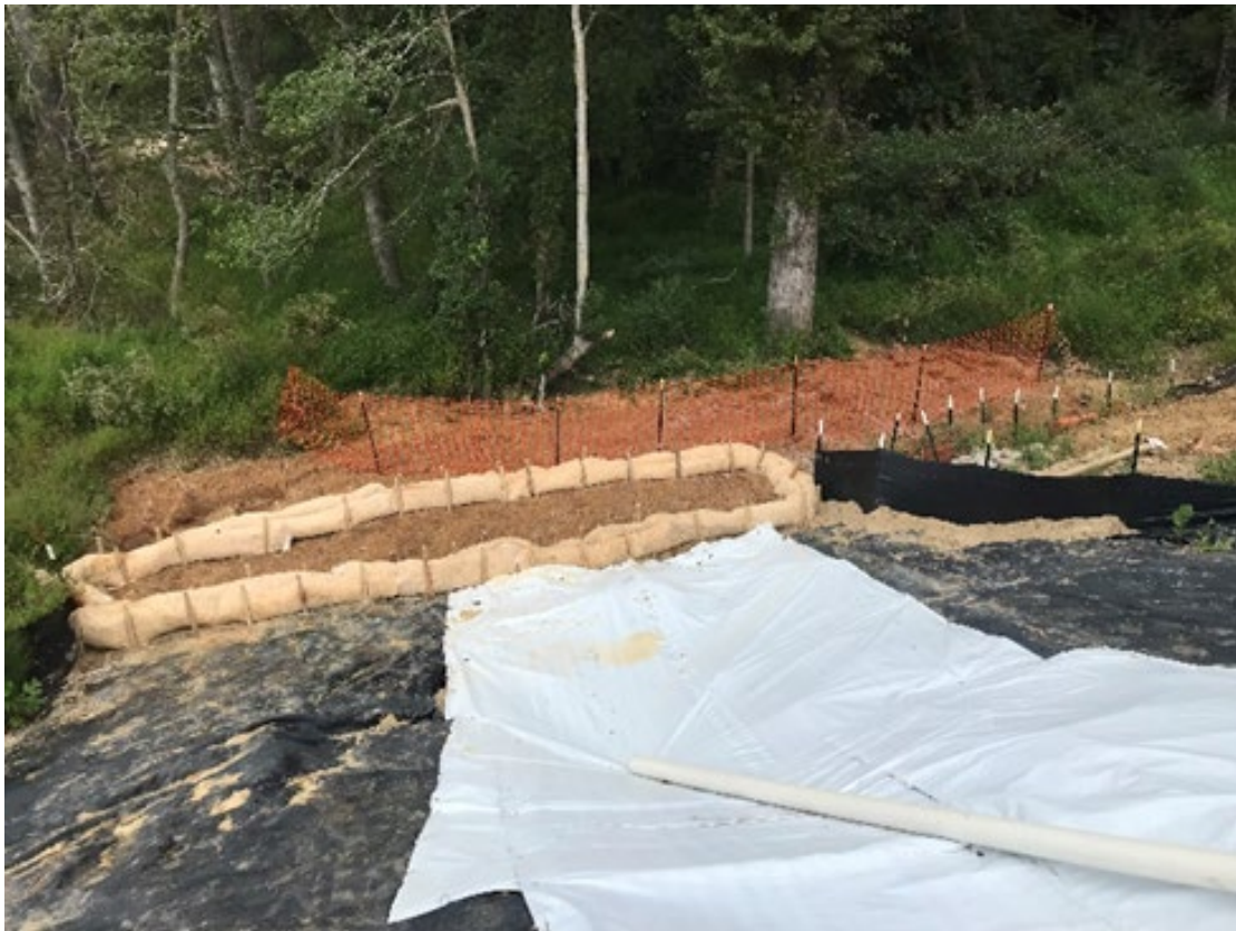
Basin berm east of Swift Creek repaired (9/29/23 follow up)
