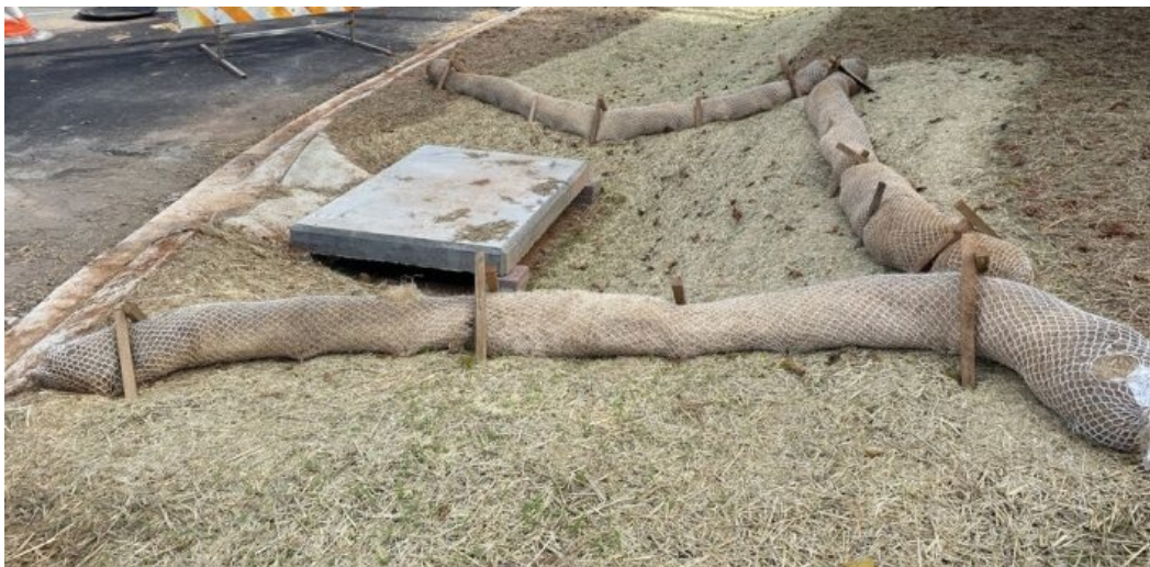
Recently matted area and wattles installed
