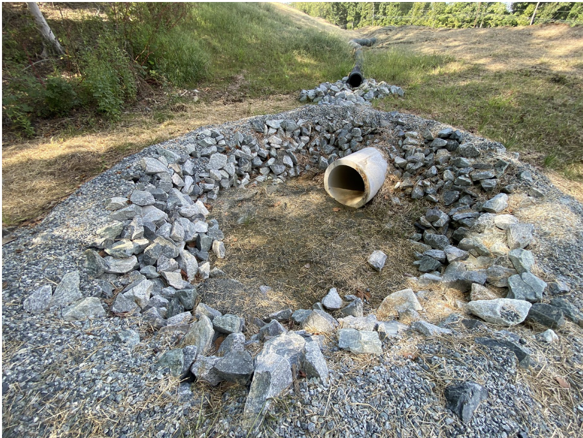
Rock doughnut inlet protection
