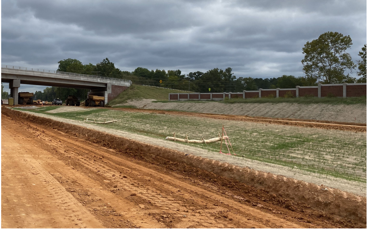
Stabilization of median and slope, with wattle checks installed
