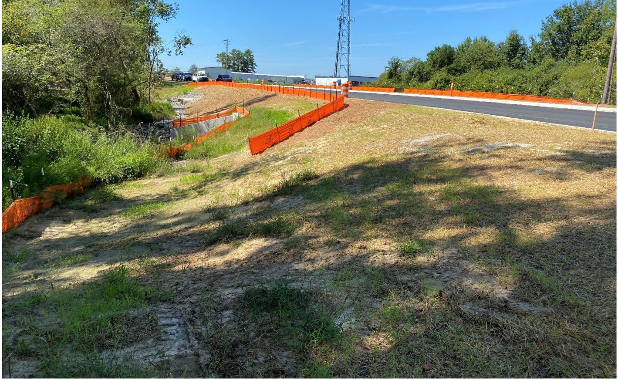
Culvert installed and areas being stabilized
