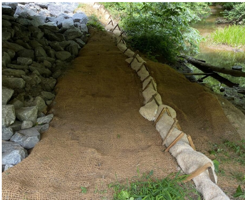
Perimeter wattles installed along stream bank
