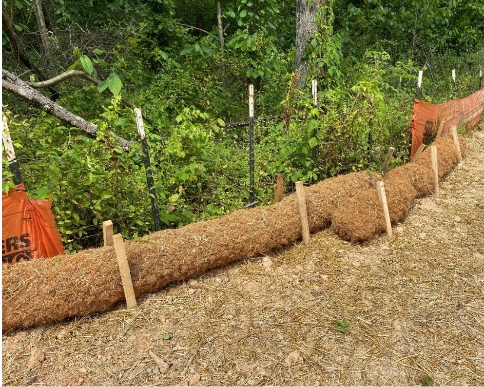
Silt fence wattle break
