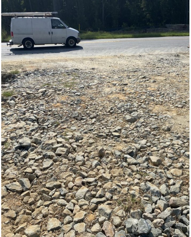
Construction entrances needing maintenance
