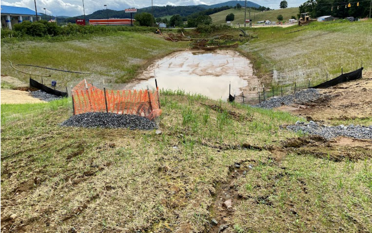
Basin being converted to permanent stormwater measure
