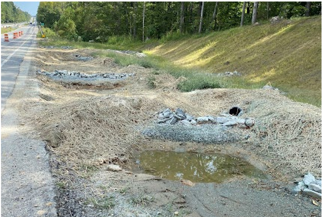
Slope drains and inlet protection measures
