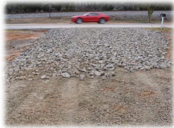
Figure 7 - Good Construction Entrance
