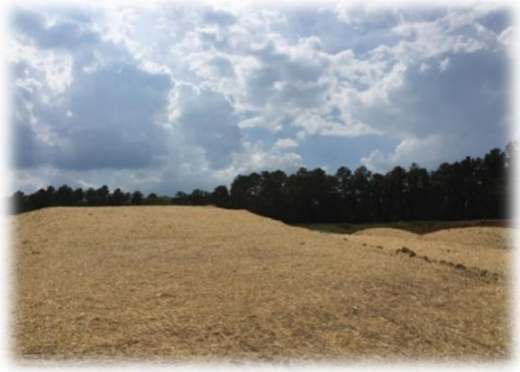
Figure 9 - Good Application of Ground Cover
