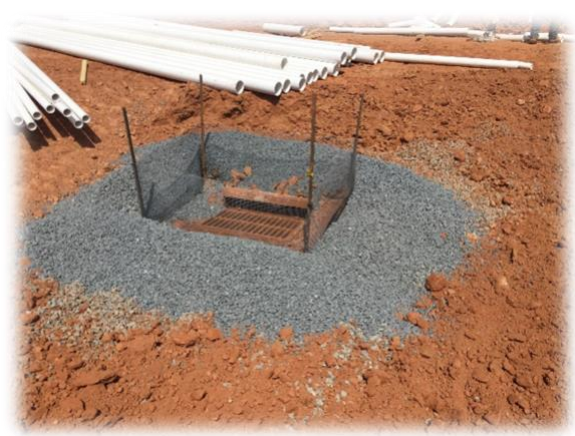
Figure 13 - Good Inlet Protection
