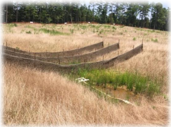
Figure 12 - Good Vegetative Stabilization
