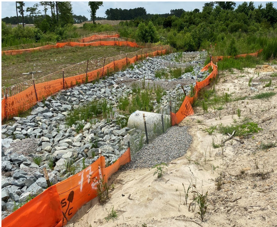
Permanent ditches completed along new ramp grade.
