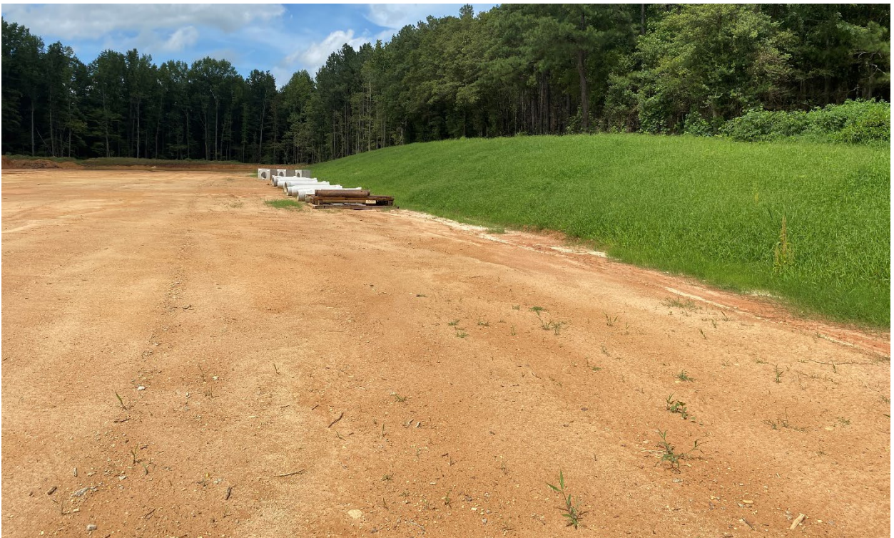
Waste site berm vegetated.
