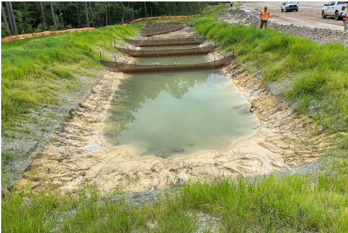
Revised skimmer basin installed to provide additional storage.
