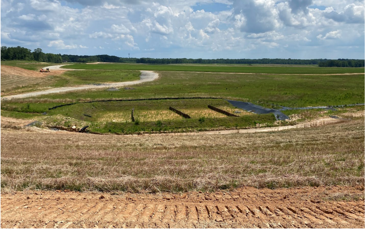
Skimmer basin and diversion ditch.
