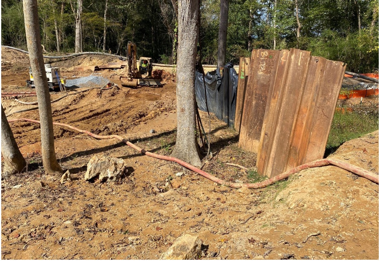
Pump around operation being installed for culvert installation.
