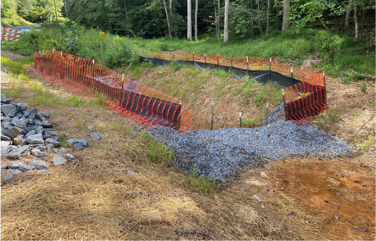
Permanent ditch completed and perimeter measures installed.
