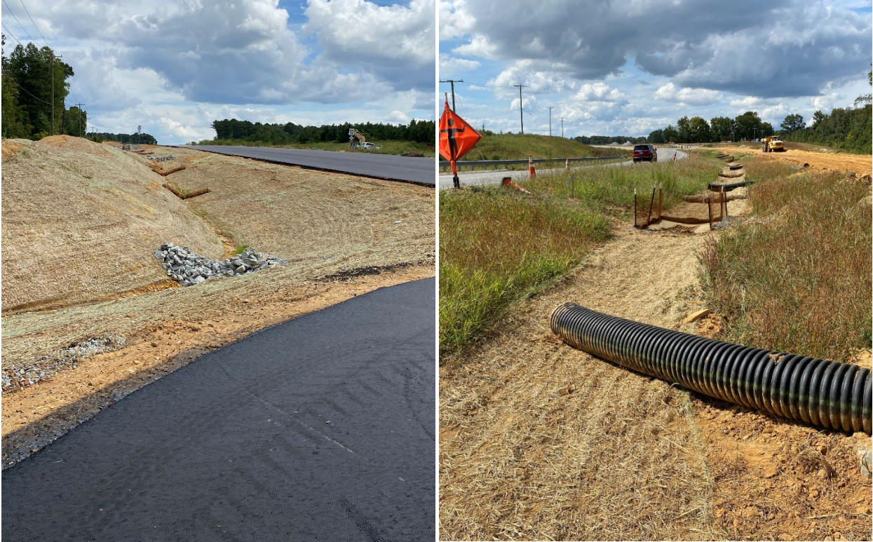
Ditches matted and check dams and wattles installed.
