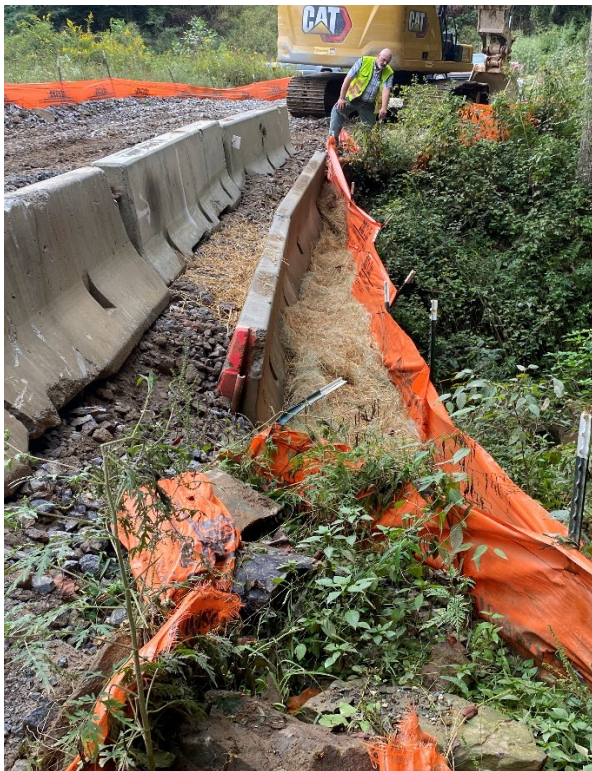
Repairs to existing measures and additional measures installed along the waste site access road.
