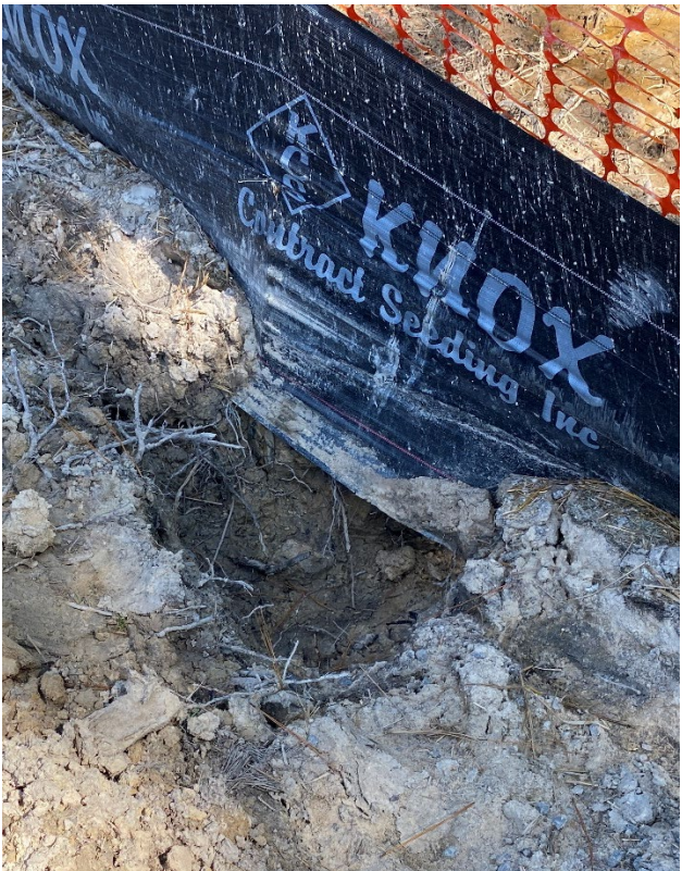
Silt fence needing repair and sediment loss beyond wattle break clean up needed.
