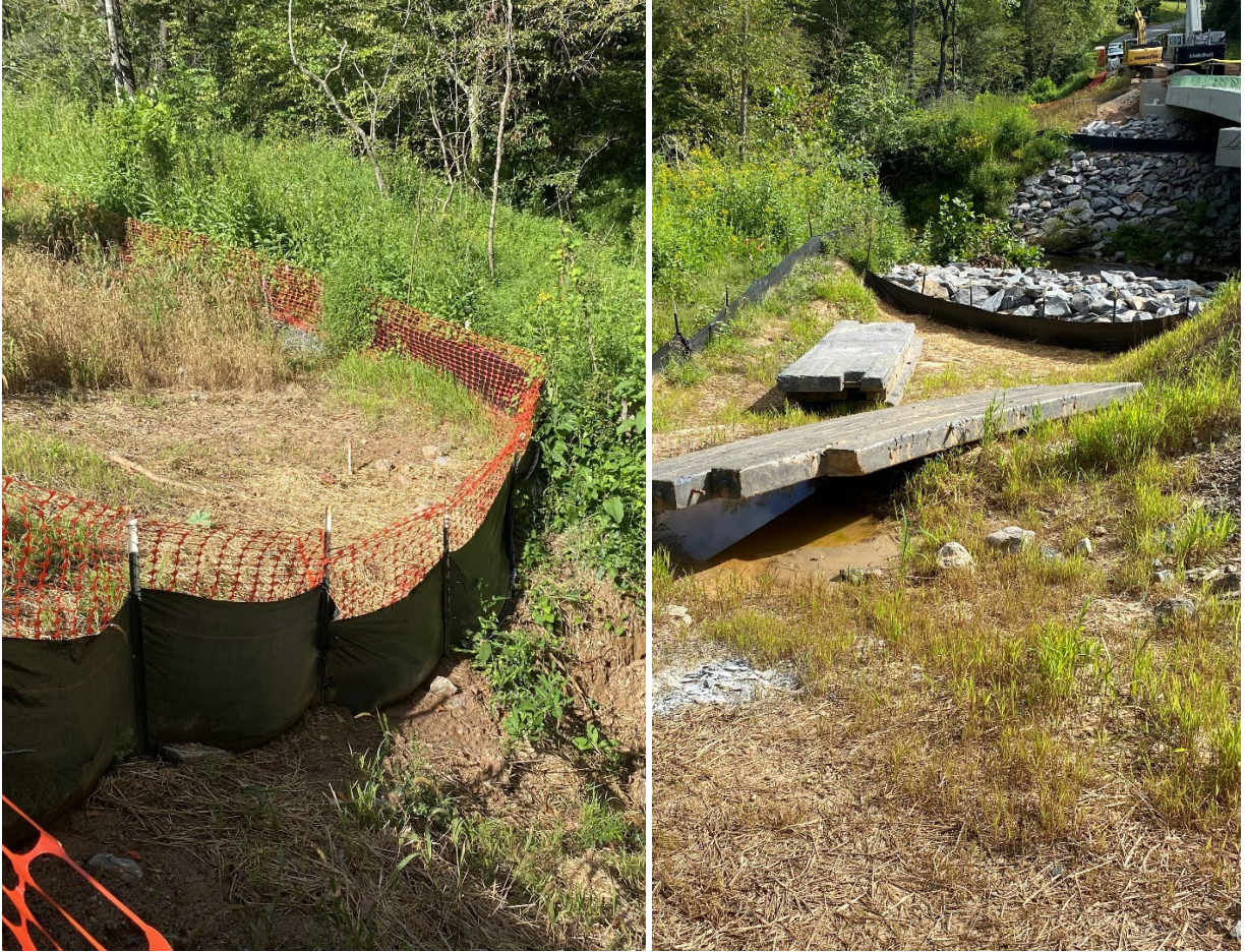
Perimeter silt fence appeared to be maintained.
