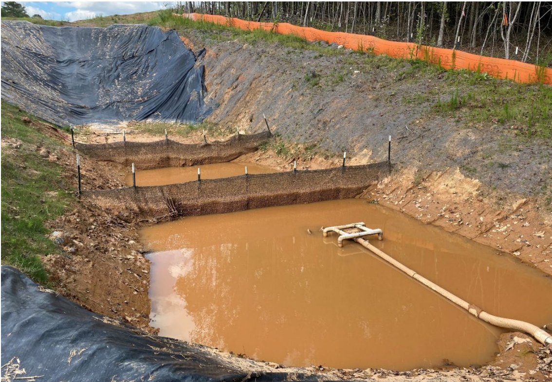
Tiered skimmer basin appears to be maintained.
