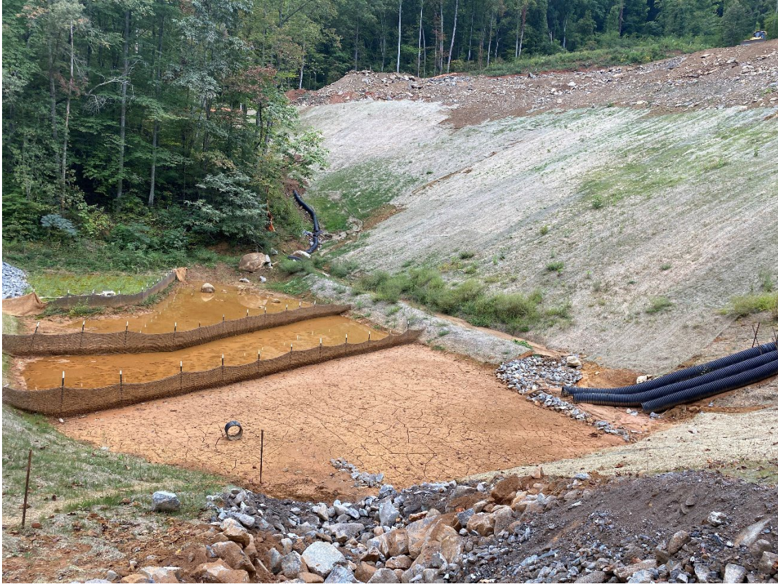
Skimmer basin and slope of waste site.
