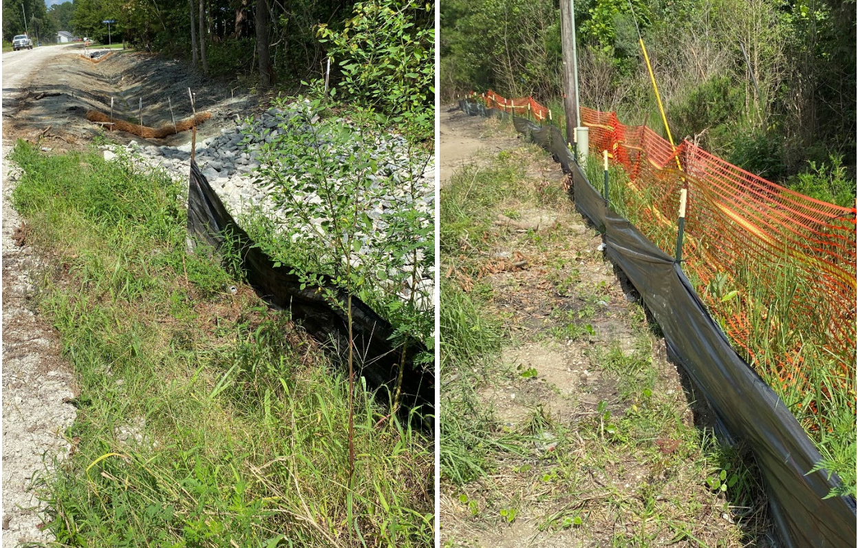
Perimeter silt fence maintained.
