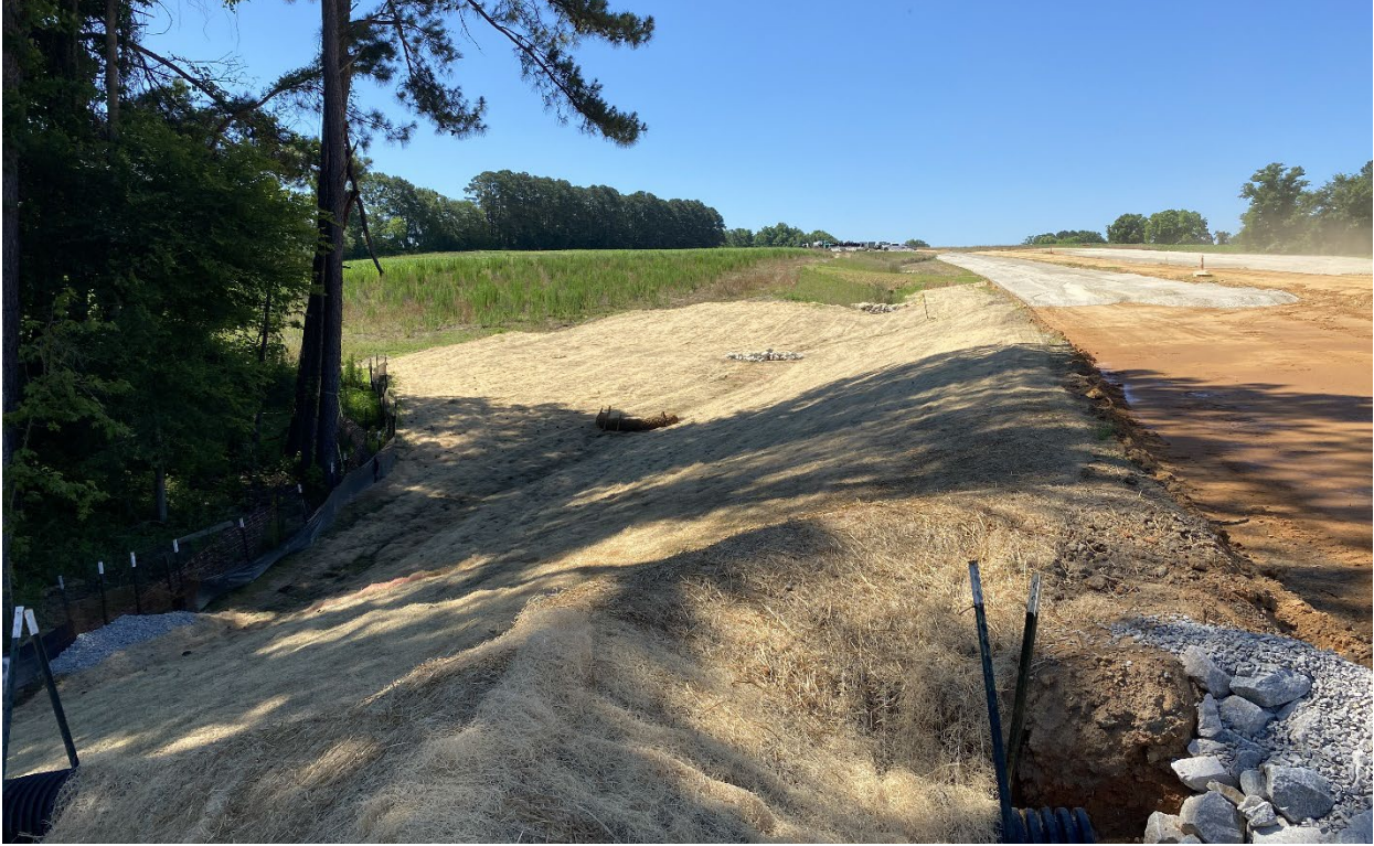
Basin removed and disturbed areas being stabilized.
