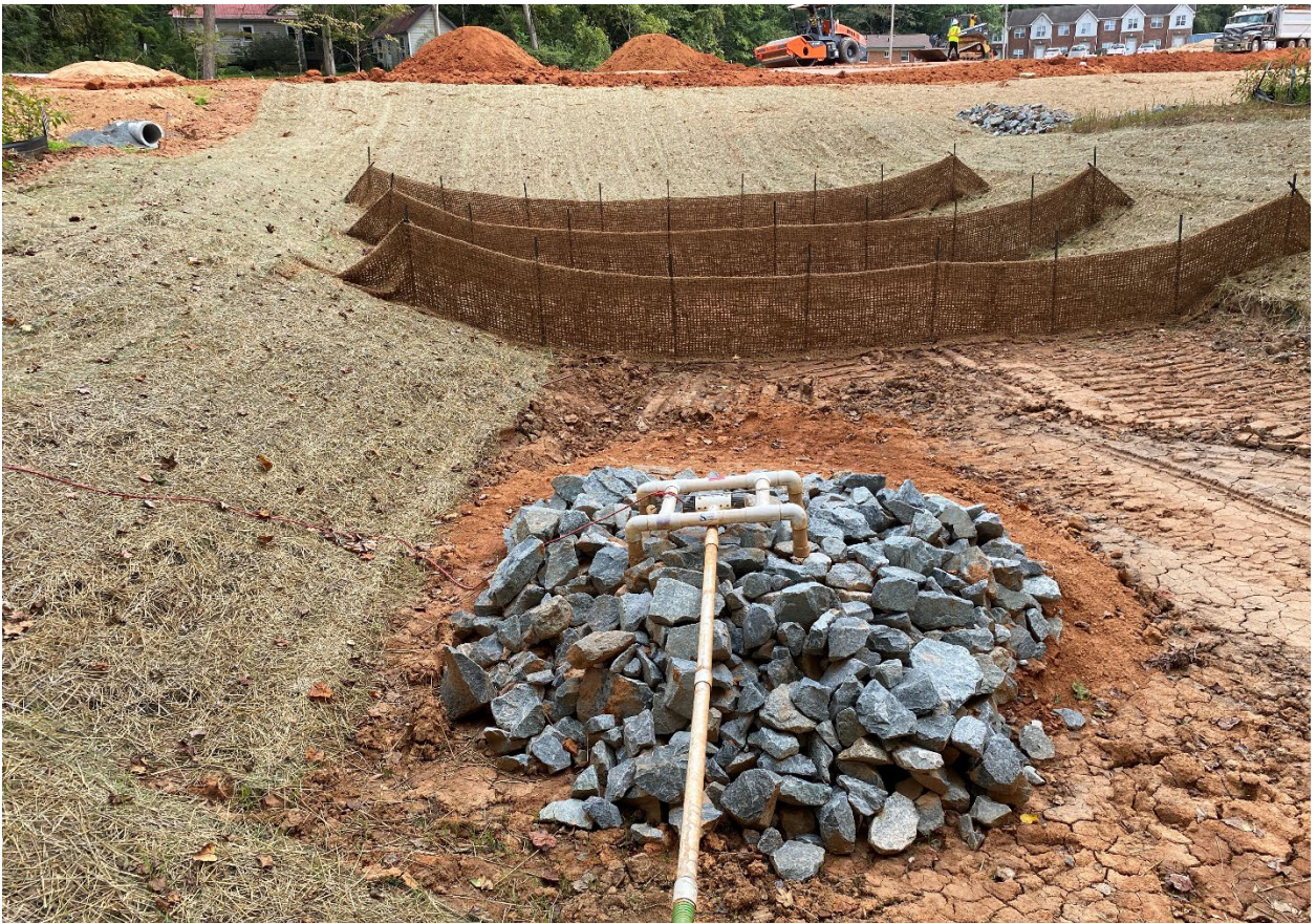
Skimmer basin recently installed.
