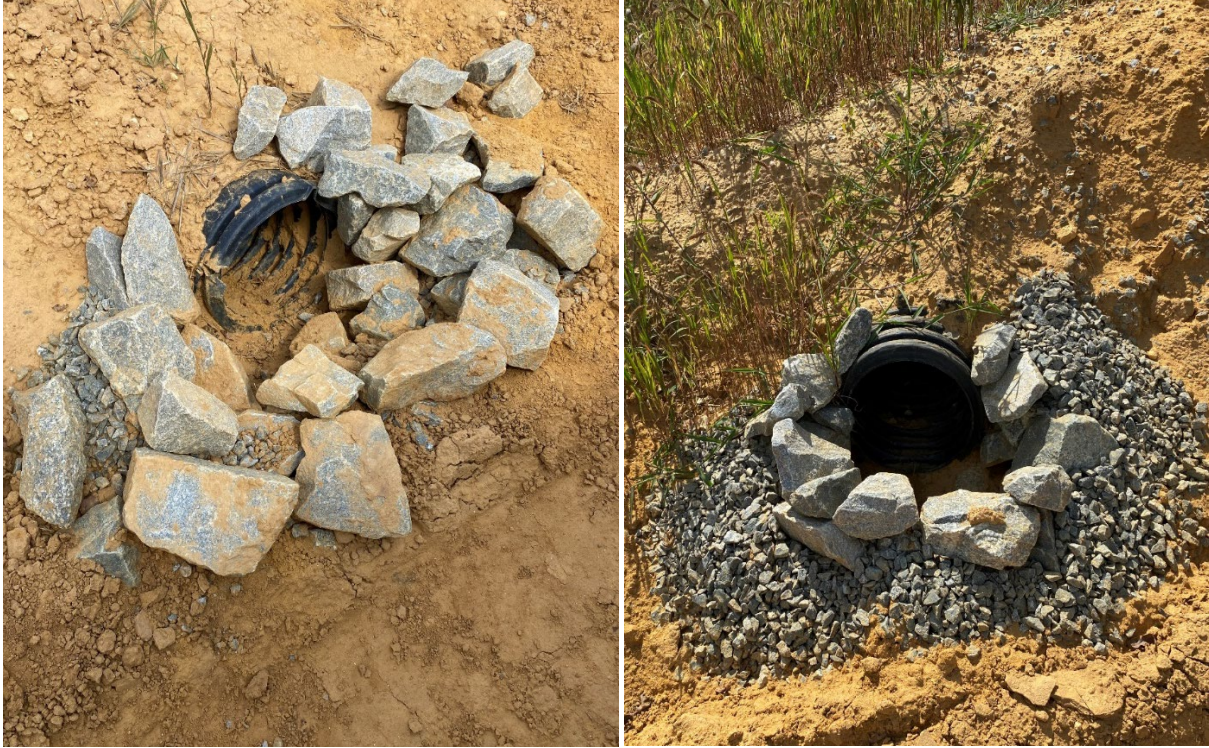
Slope drain inlet protection measures.
