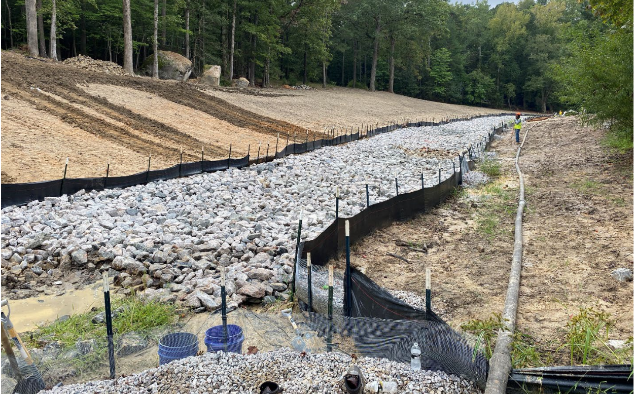
Stream relocation area repairs and sediment loss cleanup
