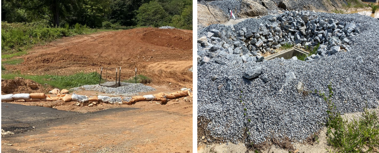
Inlet protection measures.
