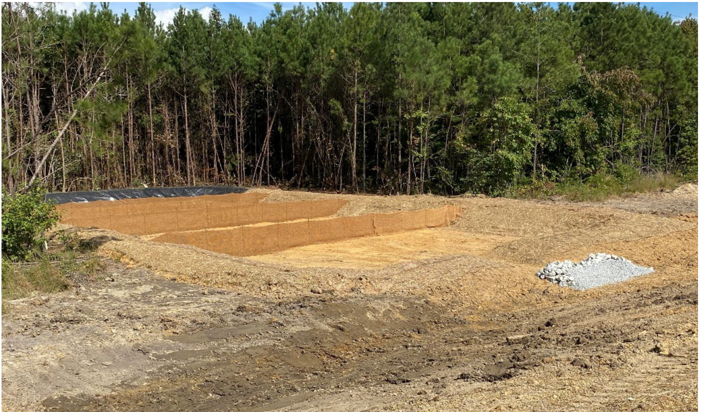
Recently maintained skimmer basin
