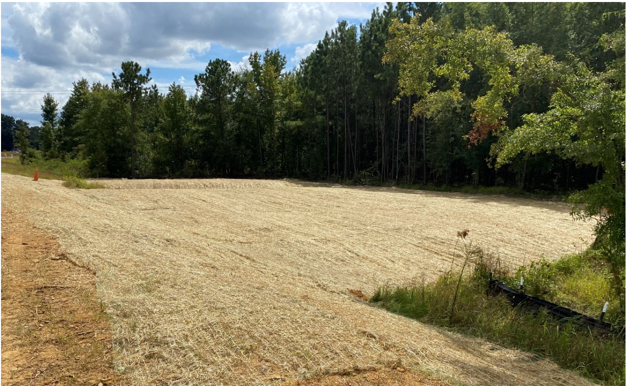
Area matted where skimmer basin was recently removed.
