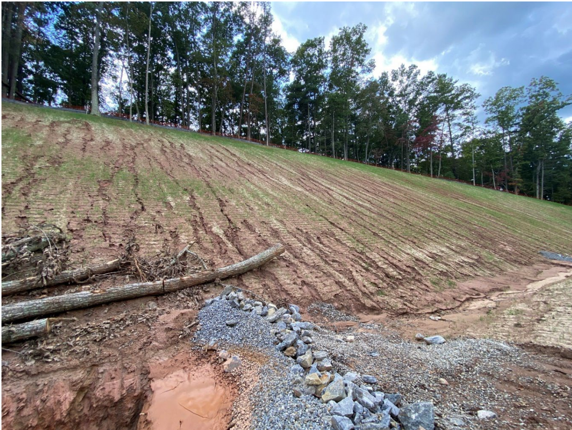
Slopes adjacent to the new Blue Ridge Parkway Bridge.
