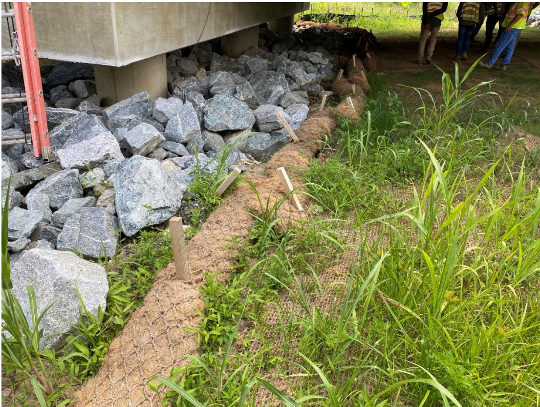
Wattles installed along top of riprap bank stabilization below new bridge.
