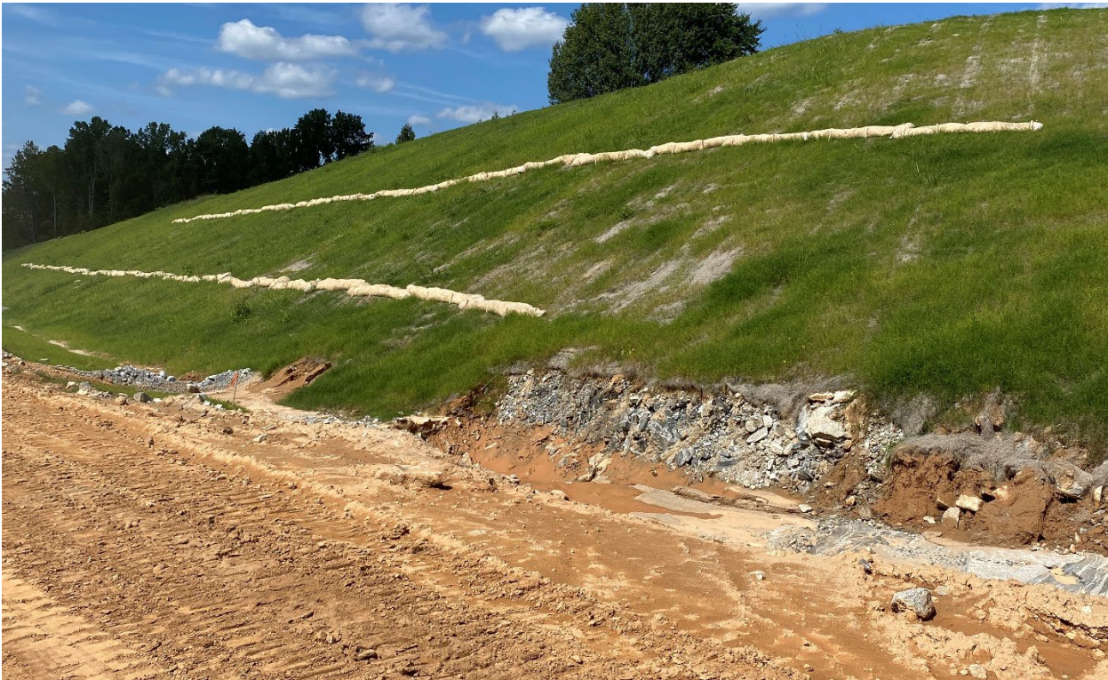
Completed slopes being stabilized.
