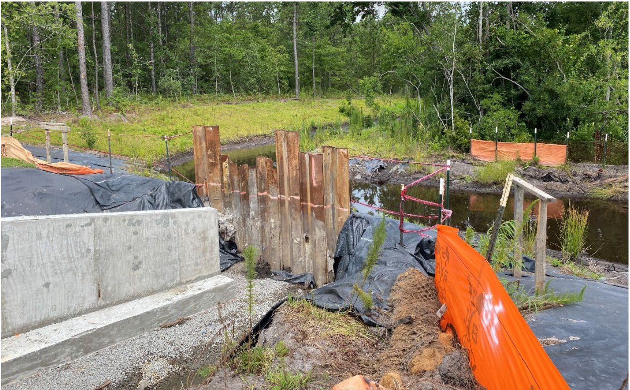
Impervious dike and stream diversion for culvert installation.
