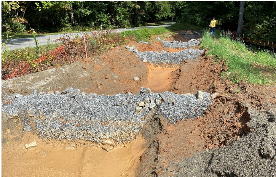
Additional check dams installed in diversion ditches.
