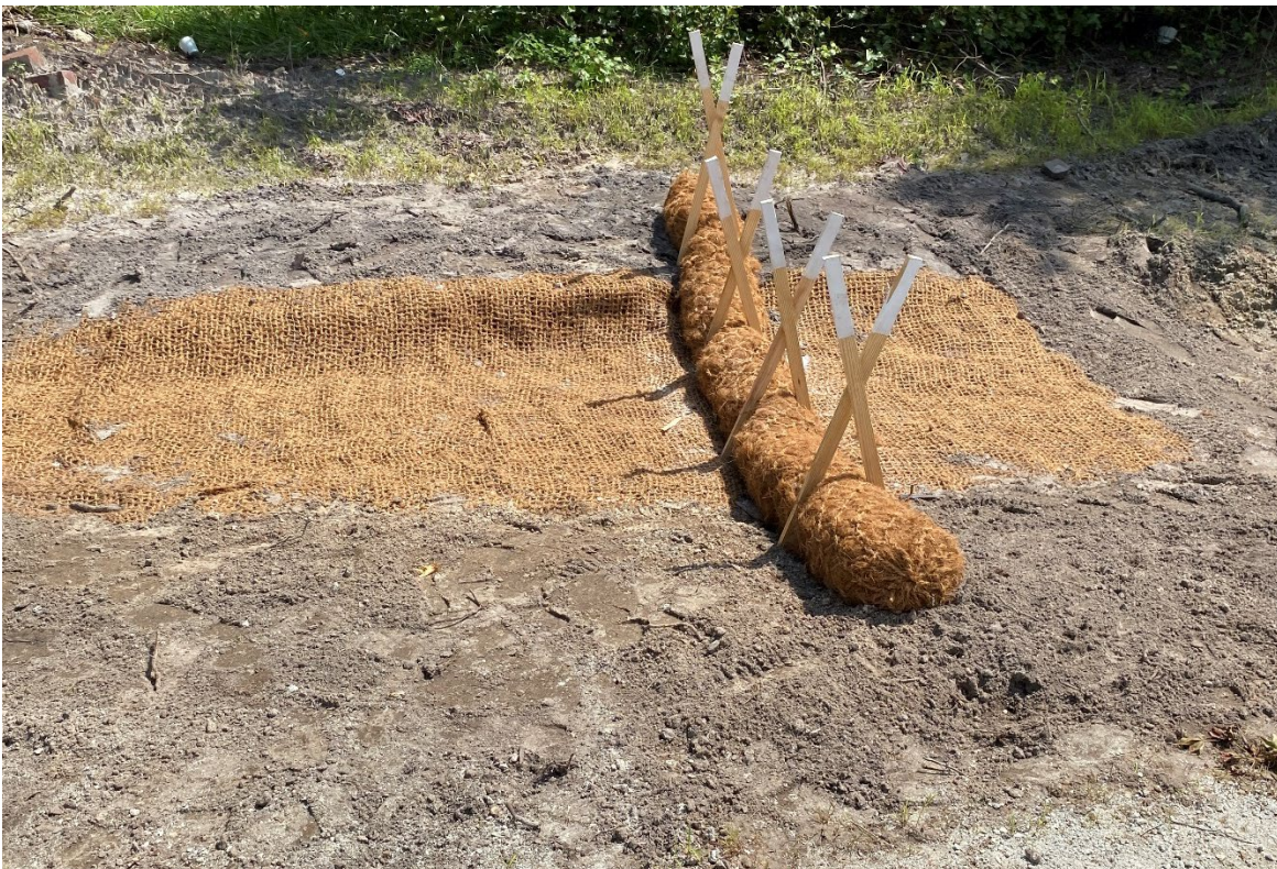
Wattle recently installed or replaced.
