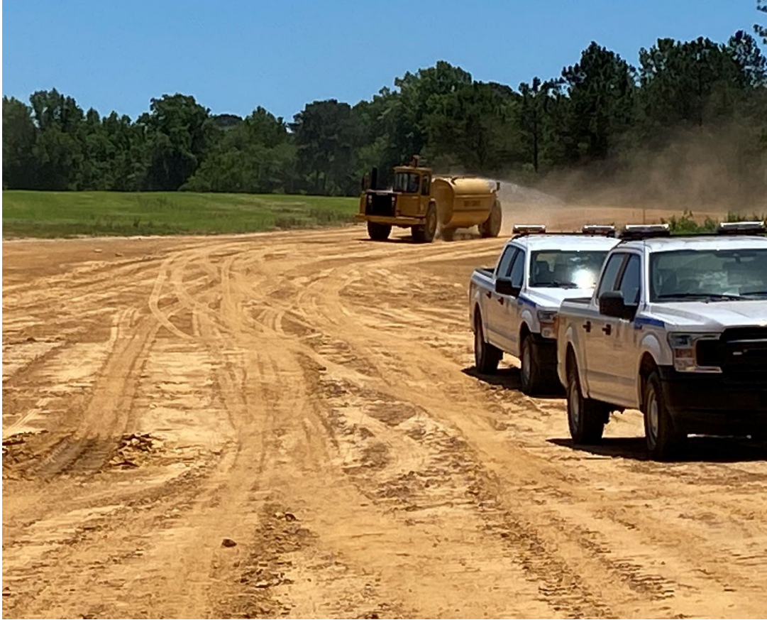
Water truck running to provide dust control.
