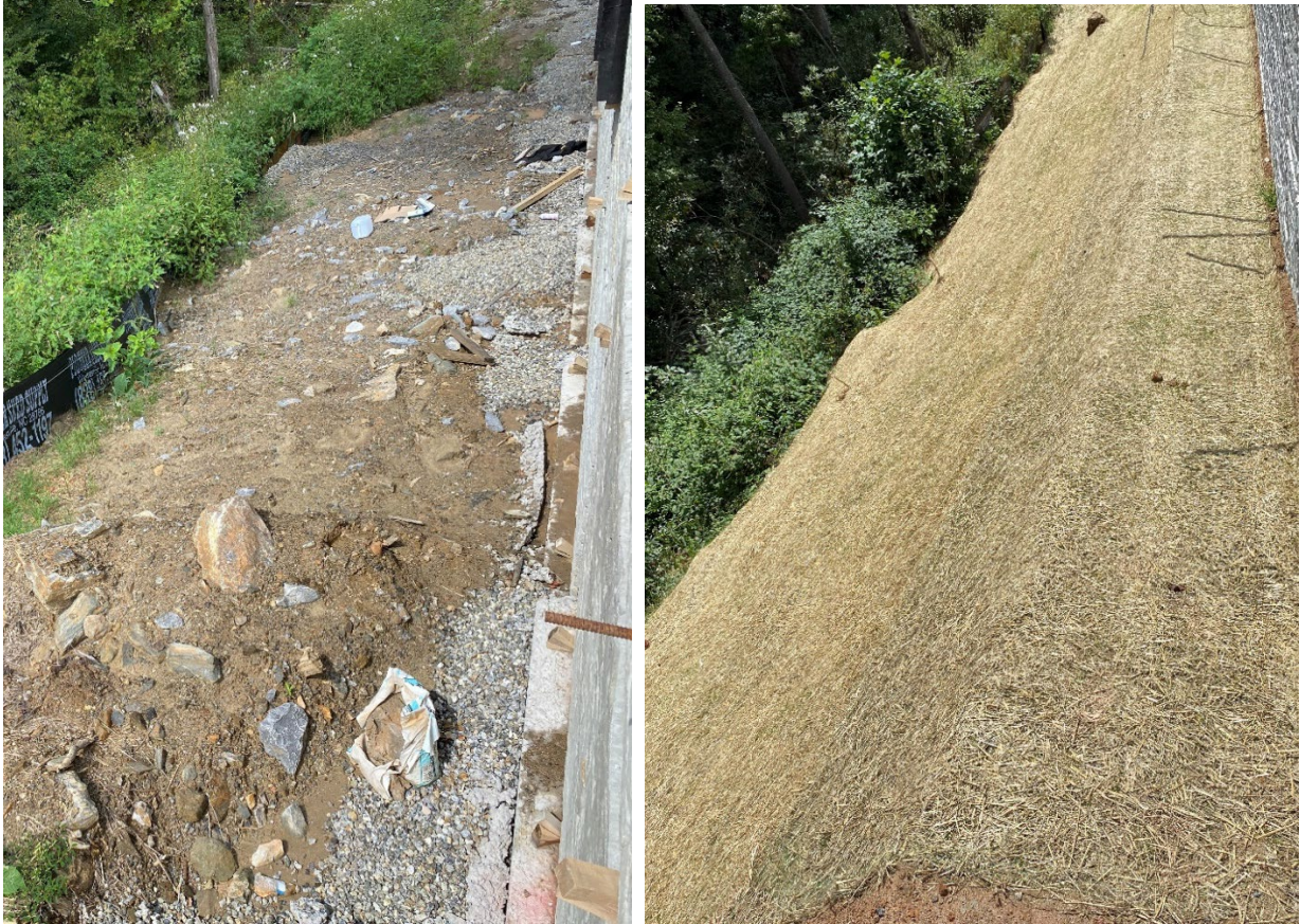
Areas below the retaining wall.
