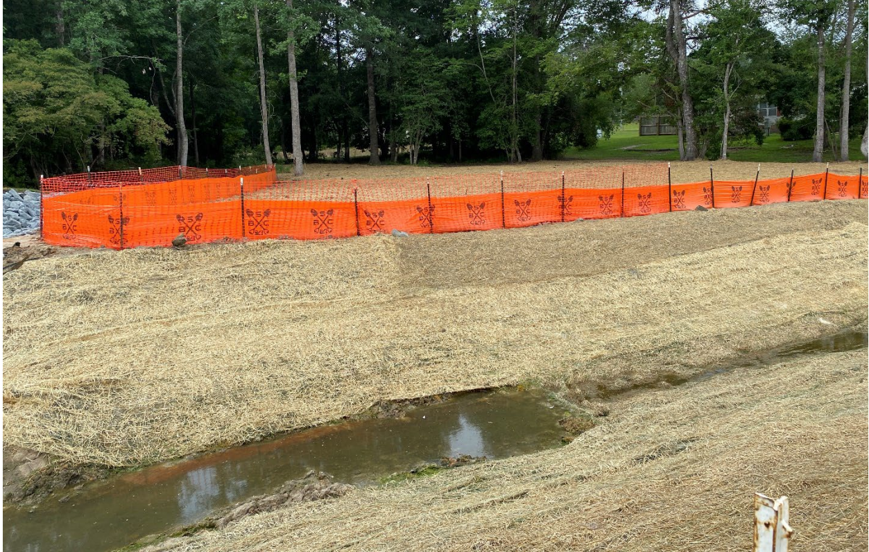
Recently completed ditch and adjacent areas stabilized
