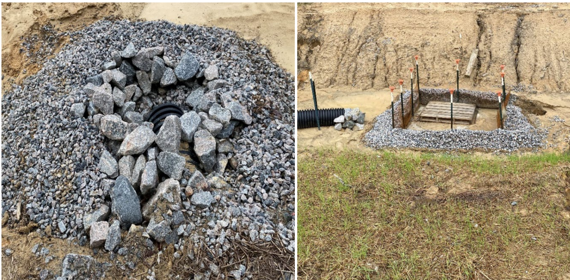
Inlet protection measures.
