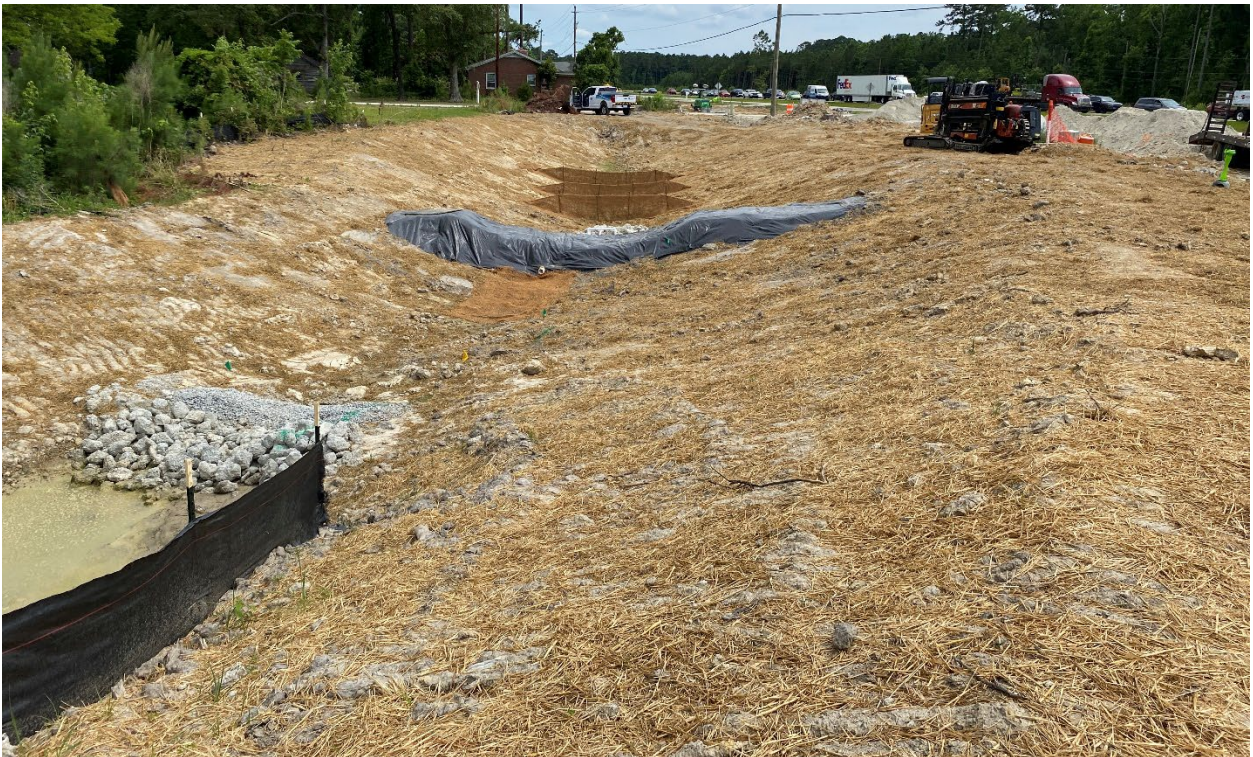
Skimmer basin recently installed, and ditch seeded and mulched with straw.
