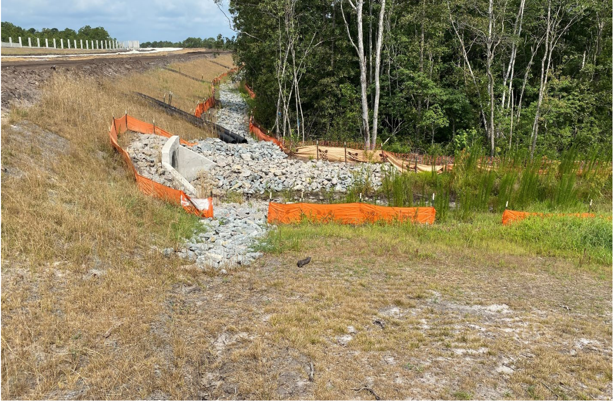
Completed slopes, permanent ditch and culvert.
