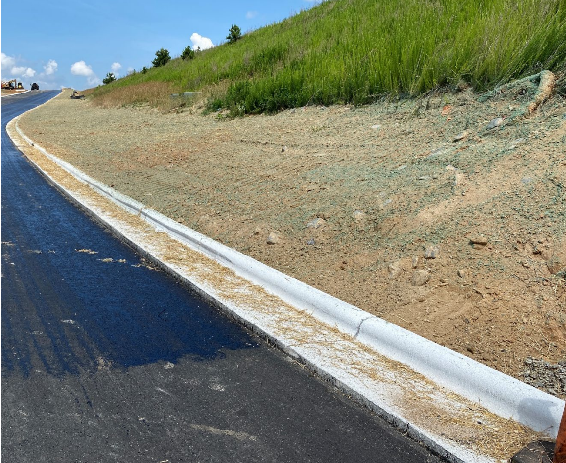
Slope completed and being stabilized.
