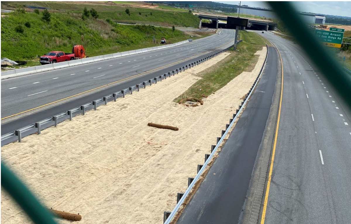
Disturbed areas in the media matted and wattles installed.
