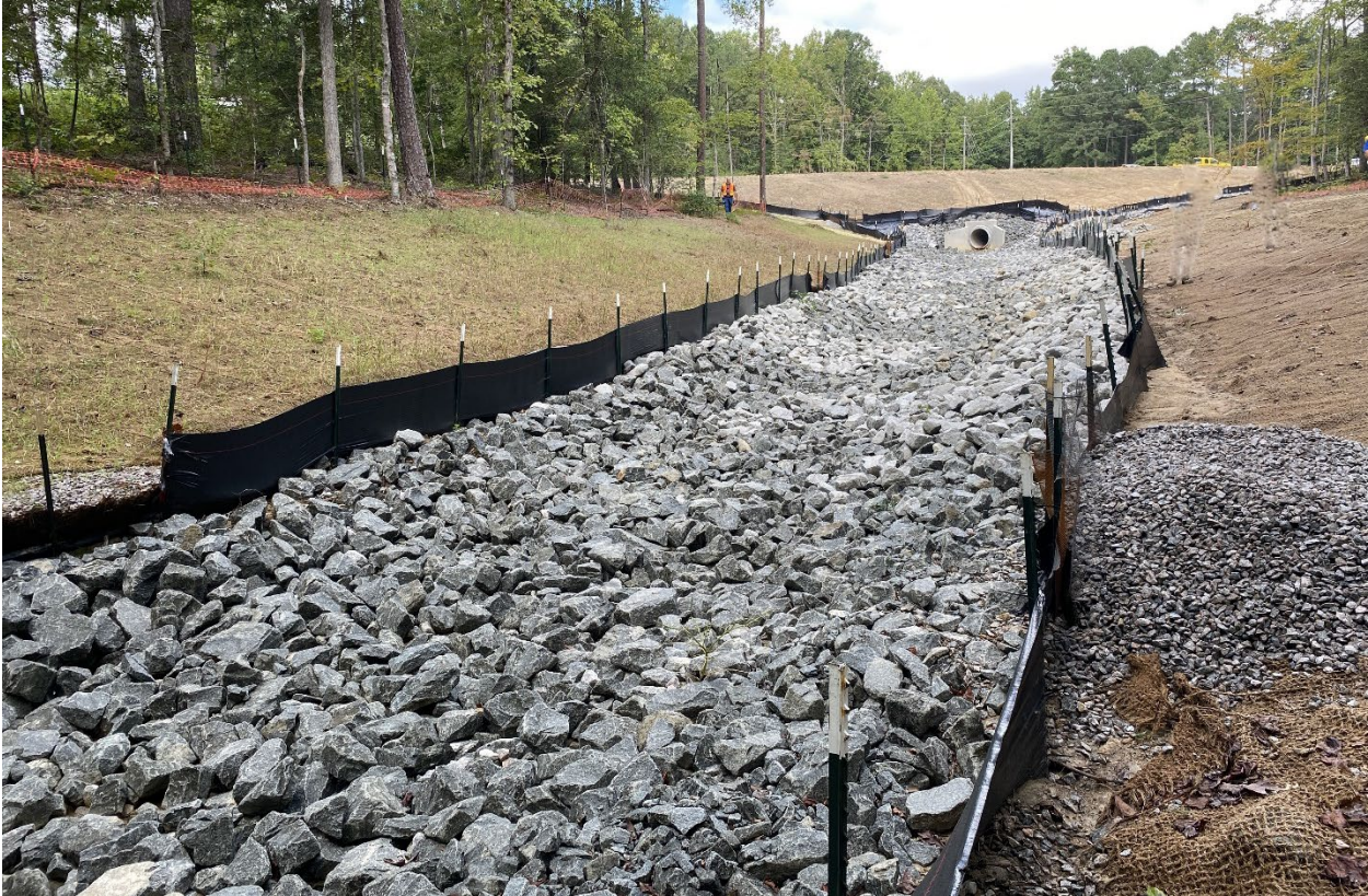
Repairs made and sediment loss retrieved at channel stabilization area.
