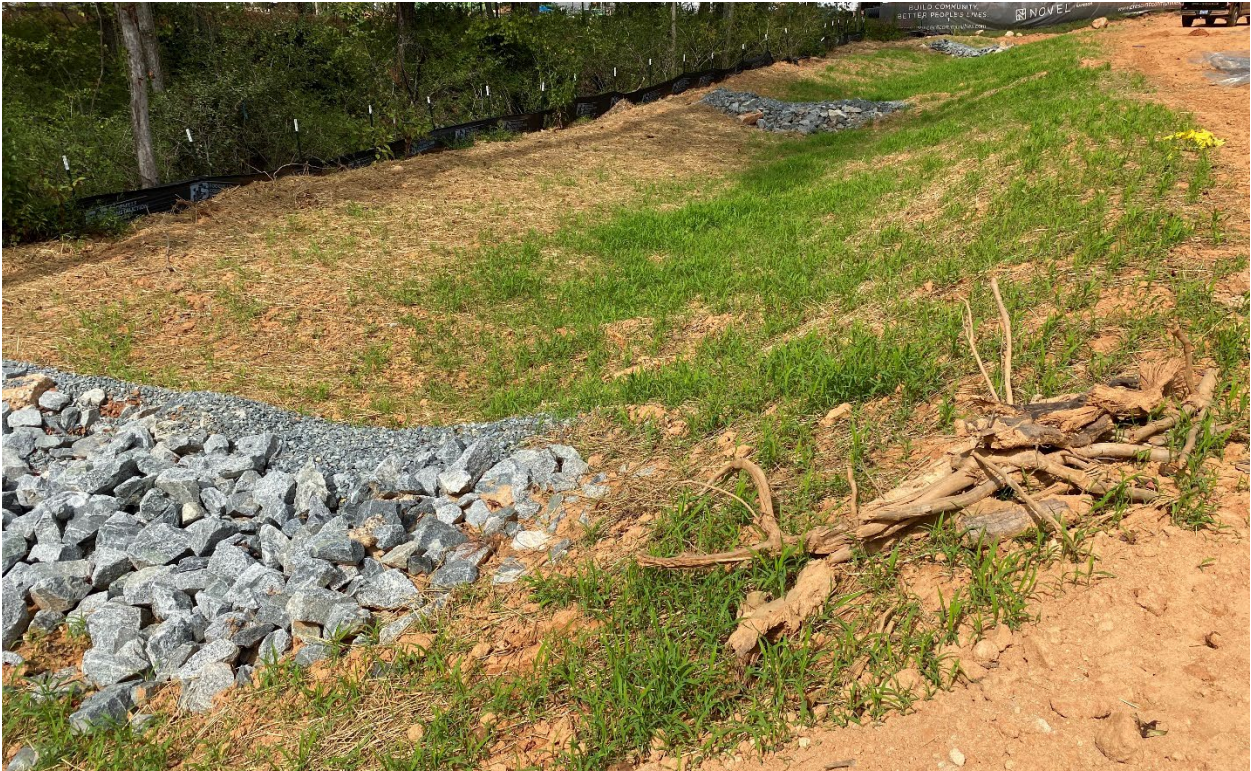
Ditch being vegetated and check dams installed.
