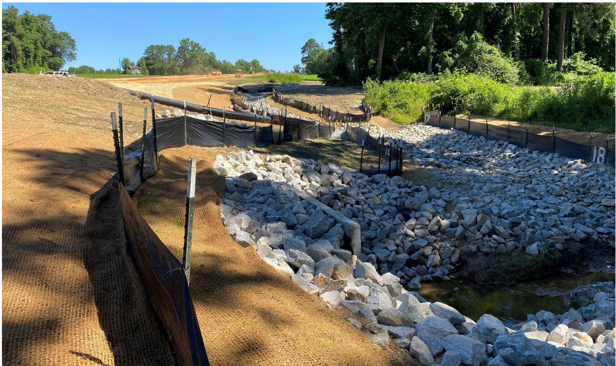
Culvert installed and area being stabilized.
