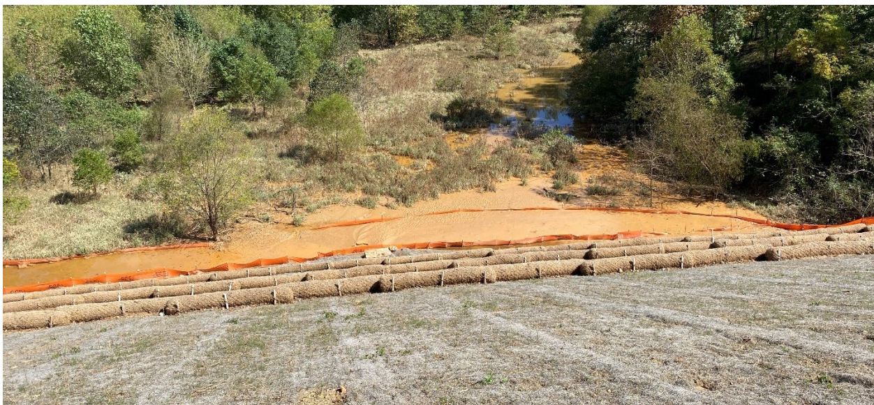
Site where sediment loss has occurred into wetland area.
