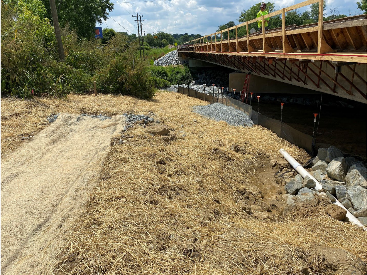
Eastbound ditch matted and areas seeded and mulched with straw.
