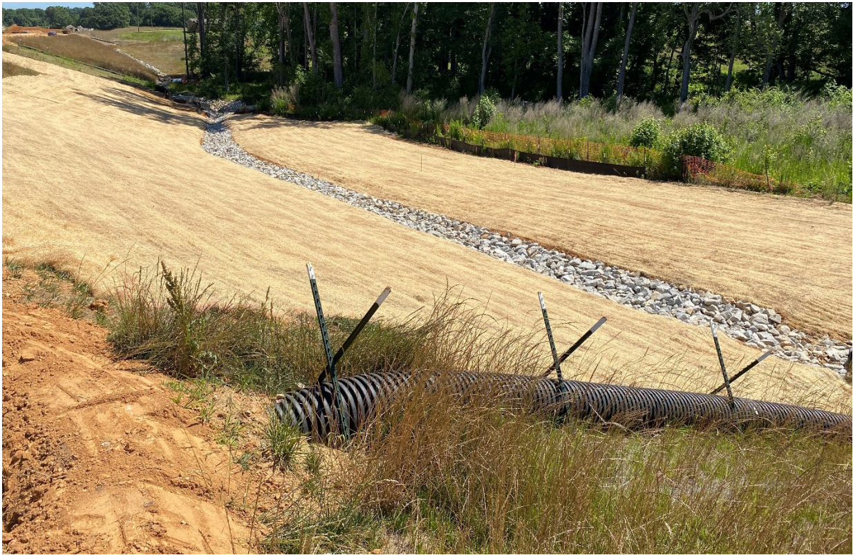
Slope recently graded and matted.
