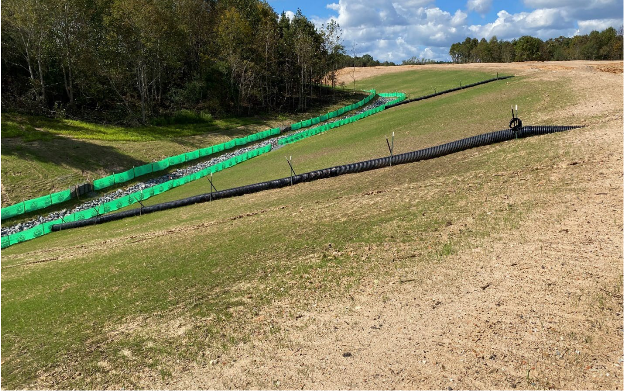
Completed slopes and permanent ditch.
