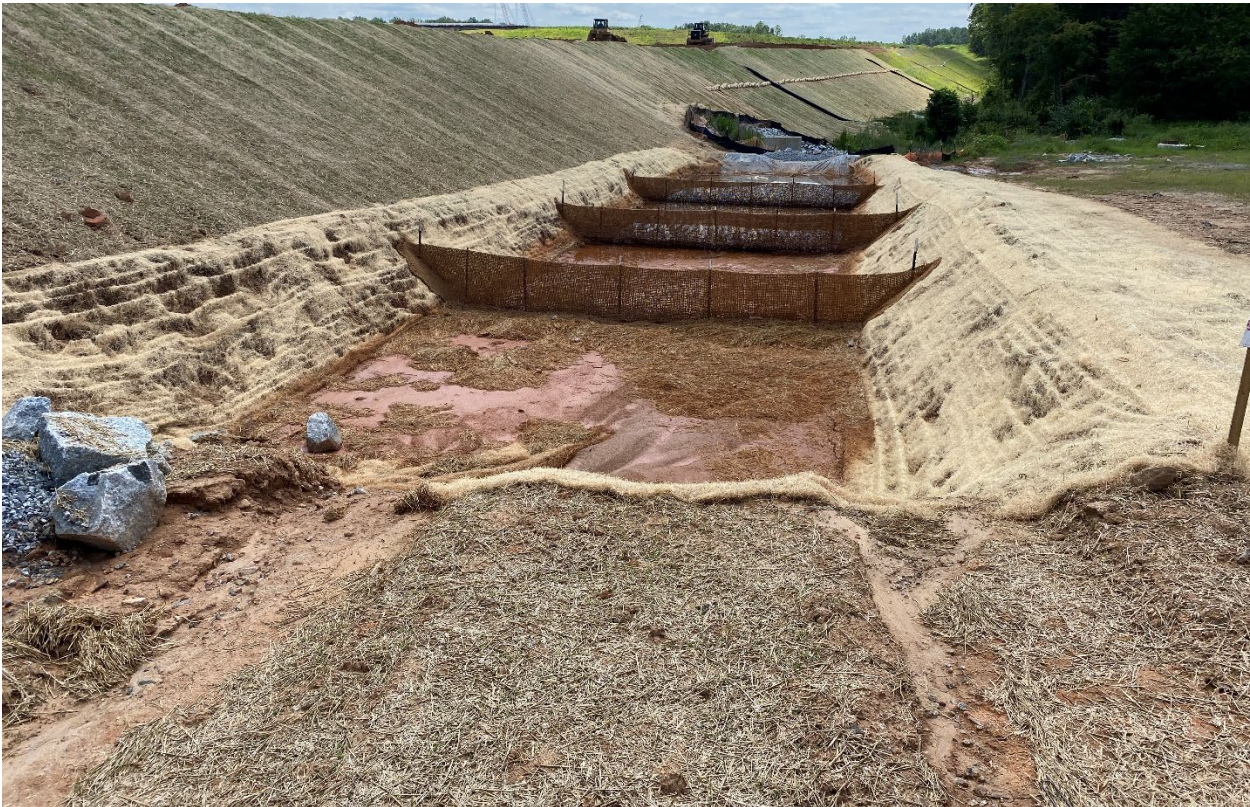
Skimmer basin and adjacent slopes matted.
