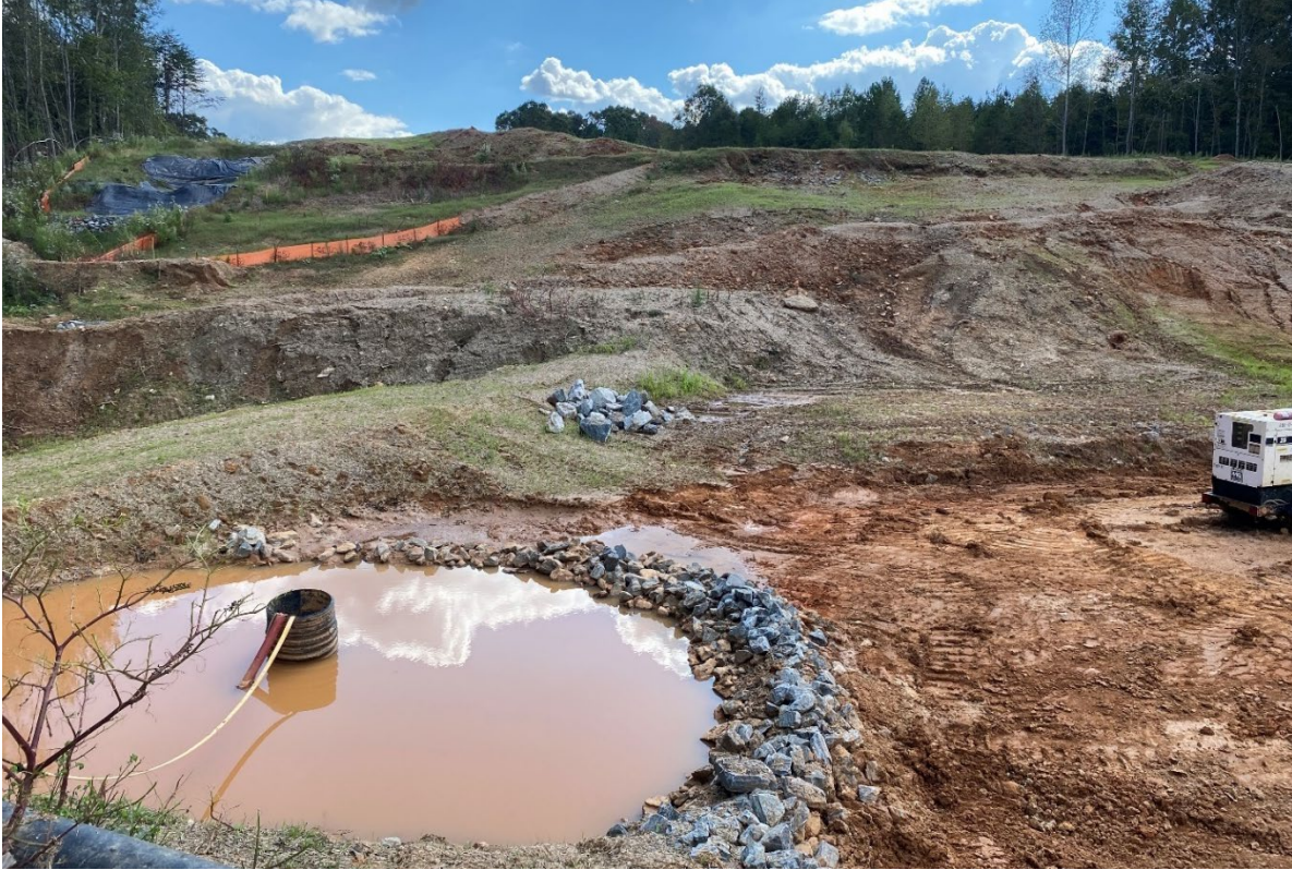
Idle areas being stabilized, and perimeter measures maintained.
