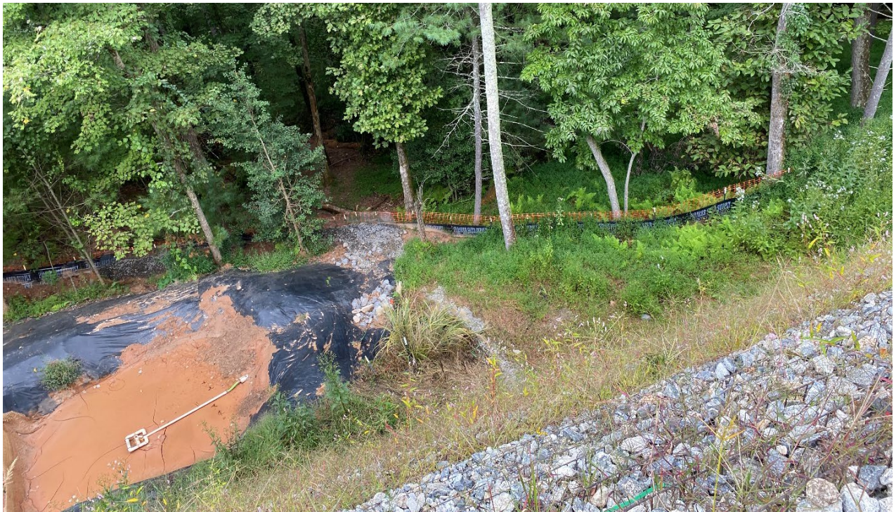
Areas of previous sediment loss, measures repaired, and sediment retrieval completed.
