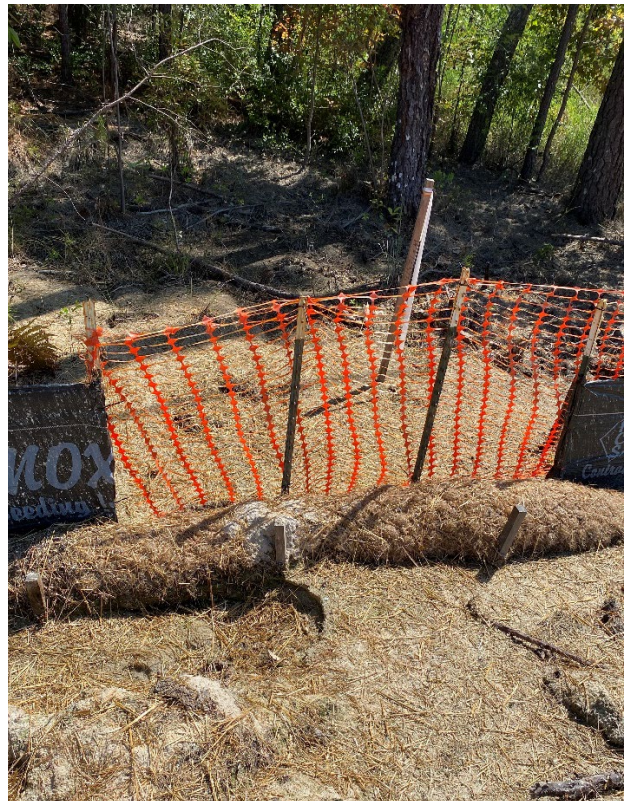
Silt fence needing repair and sediment loss beyond wattle break clean up needed.
