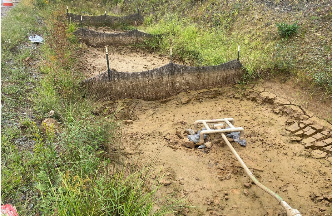
Recently maintained Skimmer basin.
