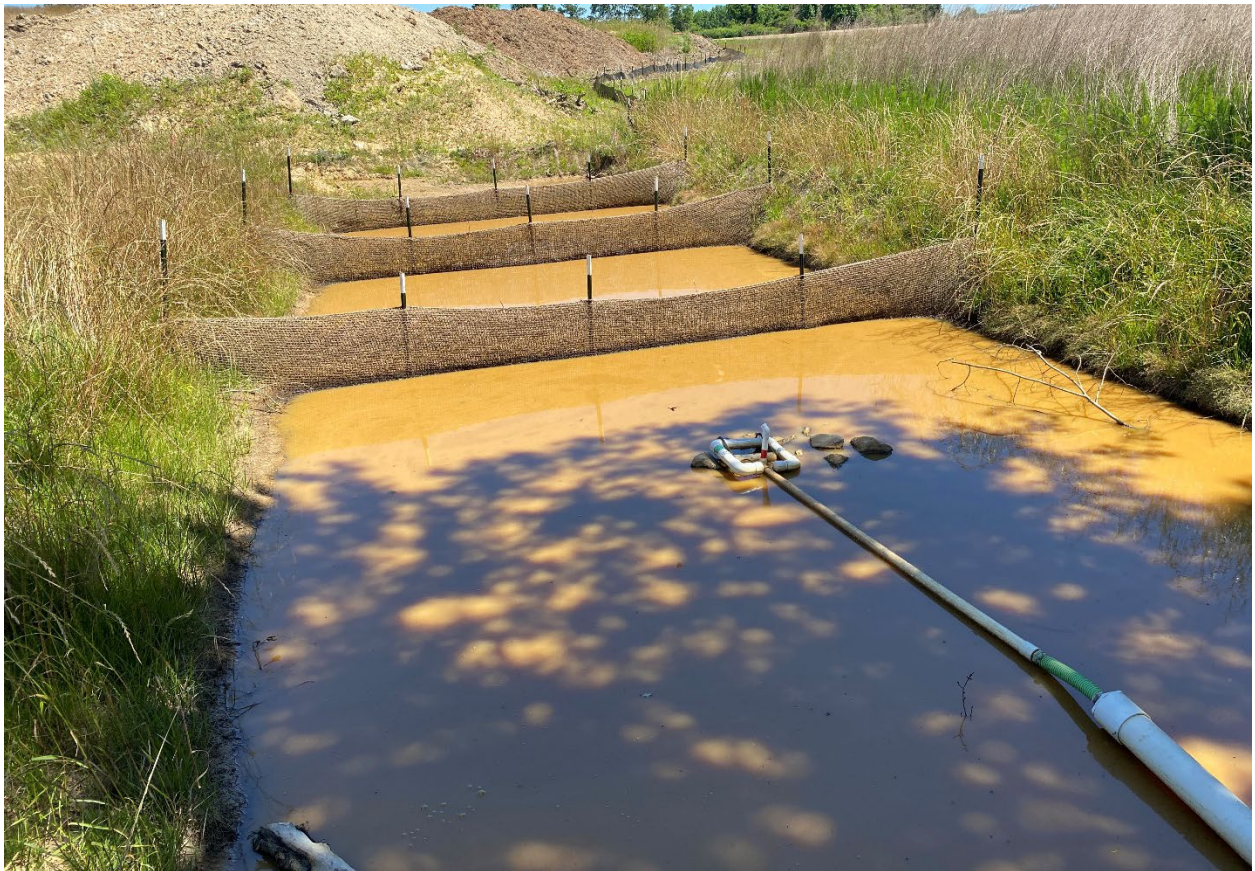
Skimmer basins maintained.
