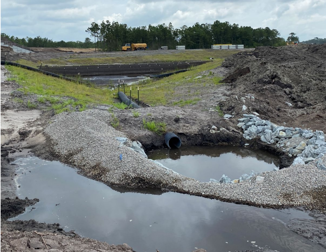
Skimmer basin and slope drains maintained.
