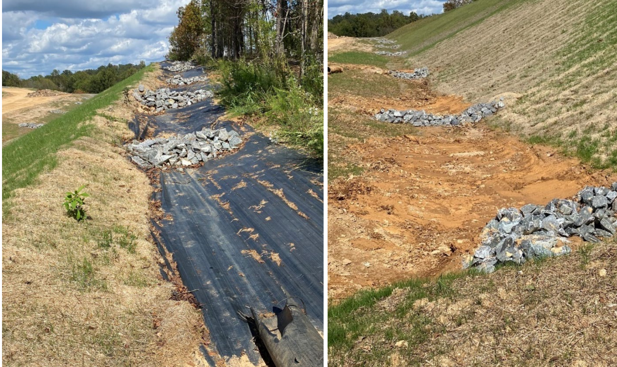
Clean water diversion and diversion ditch installed and being maintained.
