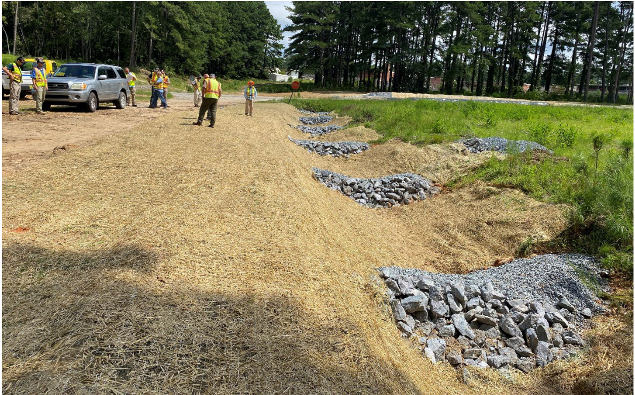
Repaired ditch where previous sediment loss occurred.
