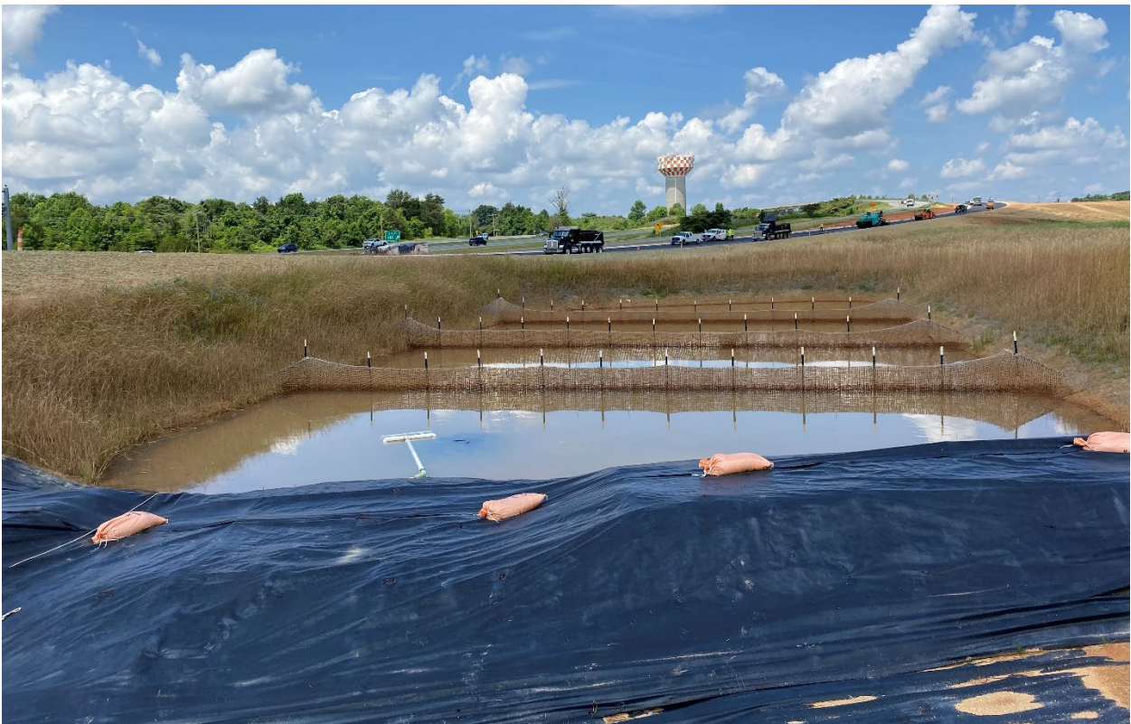
Skimmer basin appeared to be maintained.
