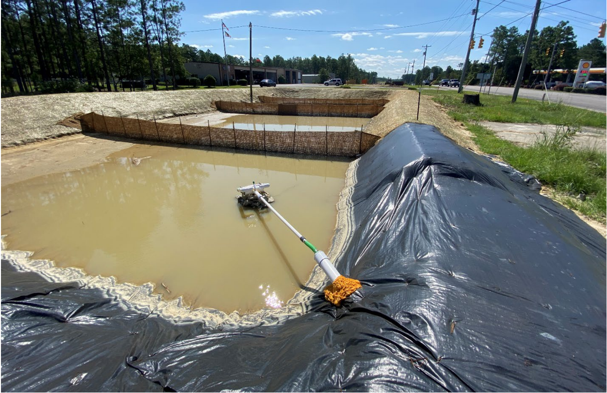
Recently installed skimmer basin
