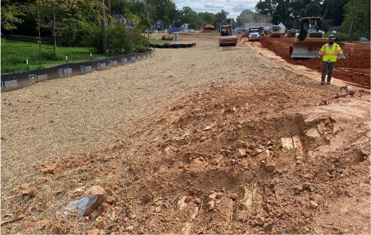
Areas seeded and mulched with straw
