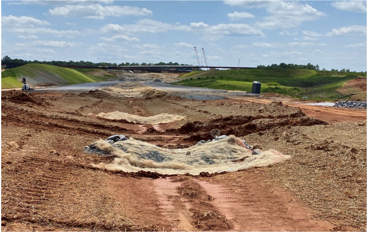
Check dams repaired in median ditch.
