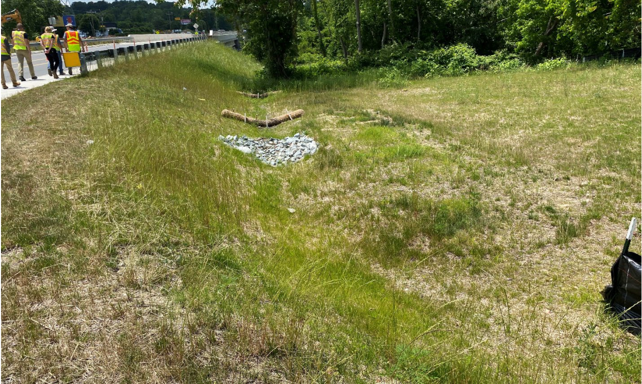
Wattles and check dams maintained in ditches and completed areas stabilized.
