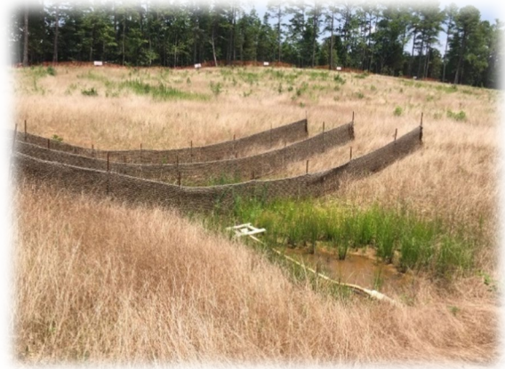
Figure 12 - Good Vegetative Stabilization
