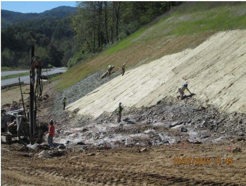
Slope Stabilization Efforts Underway
