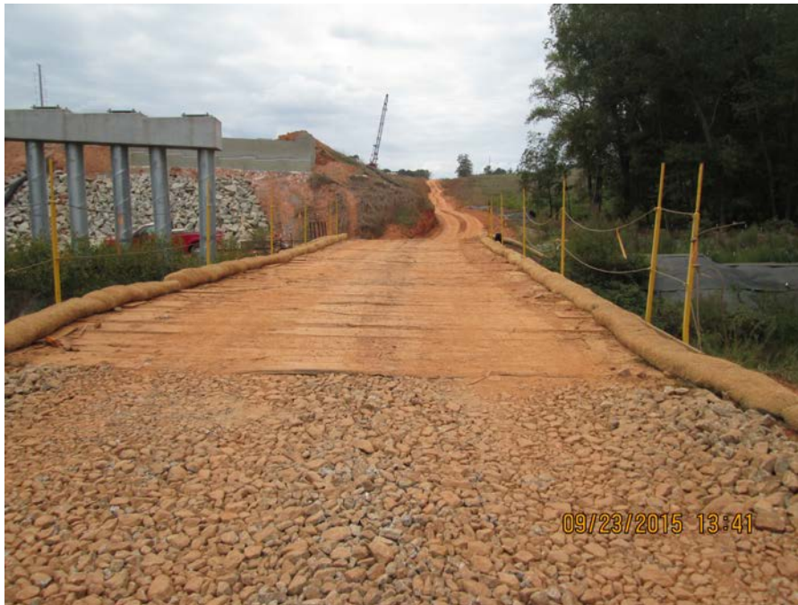
Innovative stream crossing with riprap approaches, geotextile underlayment, and wattles to minimize deposition from the sides.
