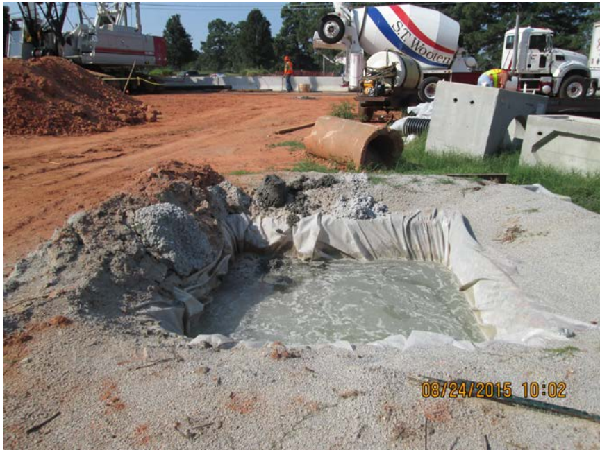
Designated concrete washout area near bridge where contractor is actively working.
