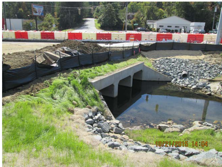
Culvert work at Reynolda Road/Winona Street project, Forsyth County
