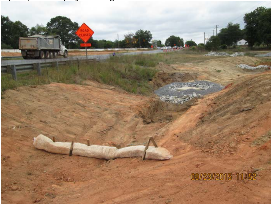
Installation of inline sediment and erosion control measures under way.
