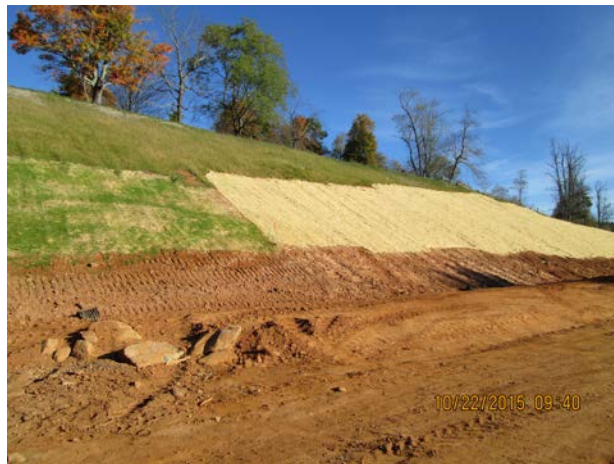
Stabilization of slopes, below
