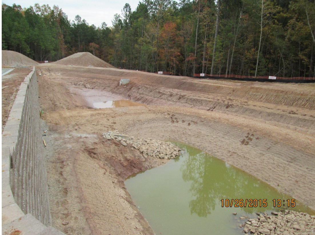
Site 2 – Bare slopes of sediment basin being converted to Stormwater pond.
