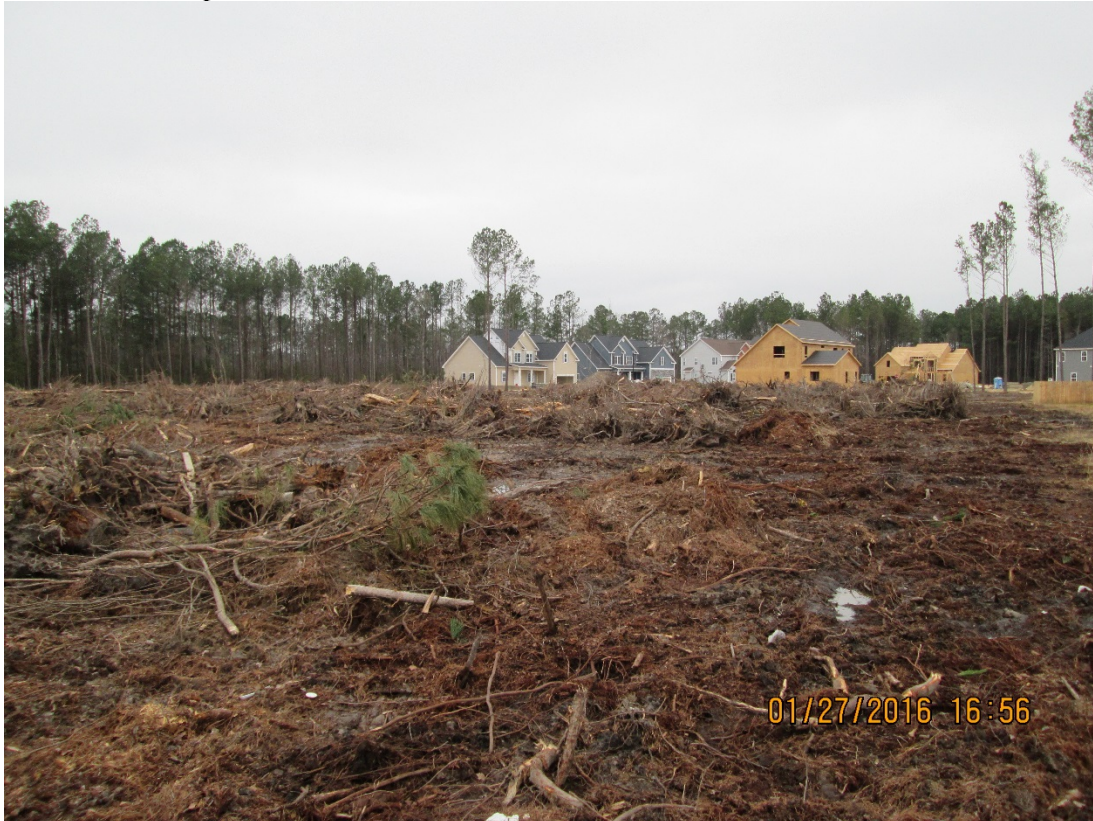
Site 4 – Sediment and erosion control installation underway.
