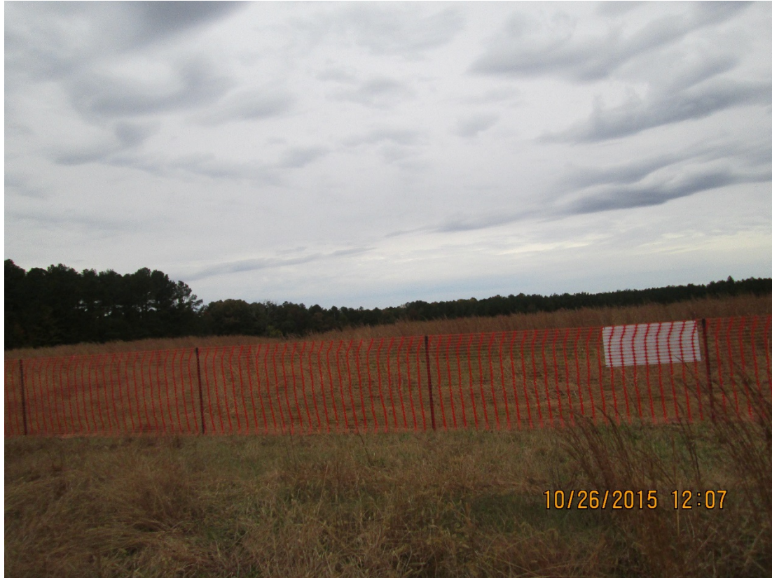
Site 1 – Installation of measures just beginning, site still vegetated.
