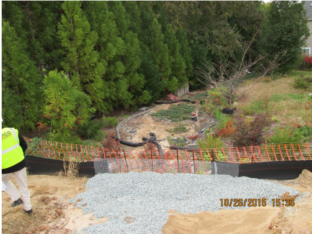
Site 3 – Offsite sediment downstream of sediment basin and skimmer outlet.
