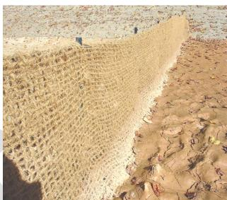
Figure 6.65d Close-up of a porous baffle.
