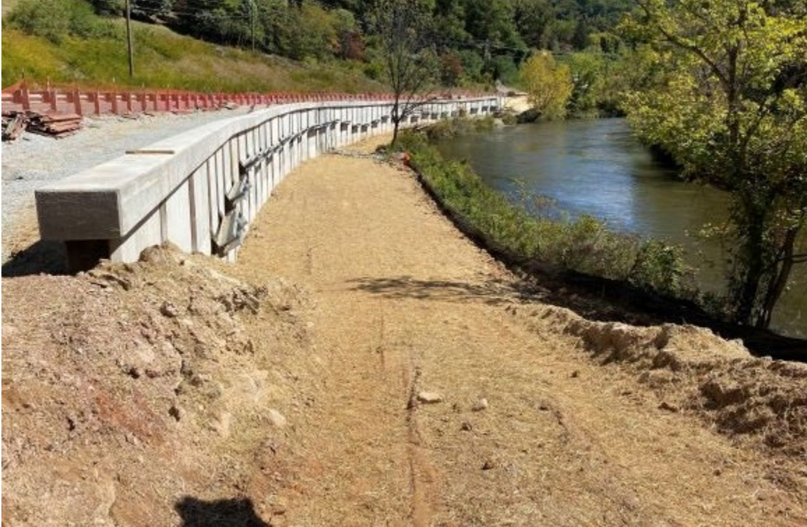
Photo- Completed areas seeded and mulched with straw or matting
