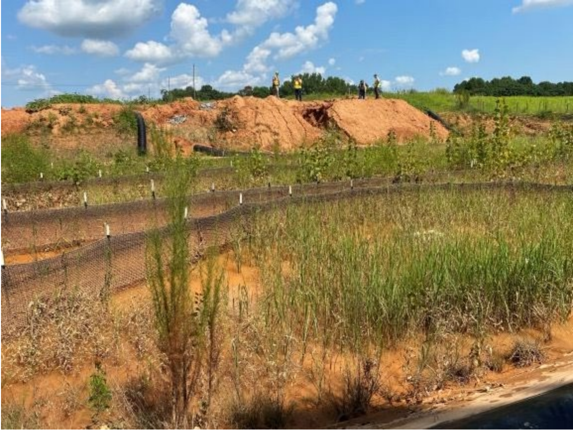
Photo- Skimmer basin above sediment loss needing maintenance
