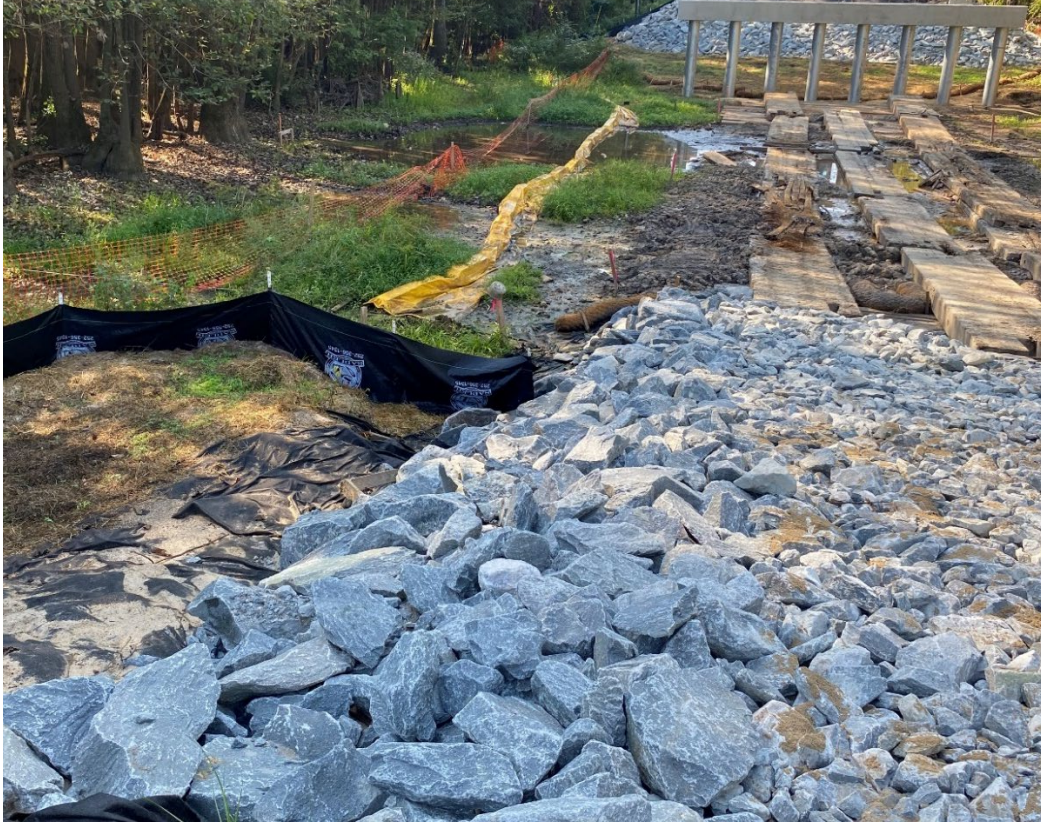
Photo- Active bridge construction and turbidity curtain installed
