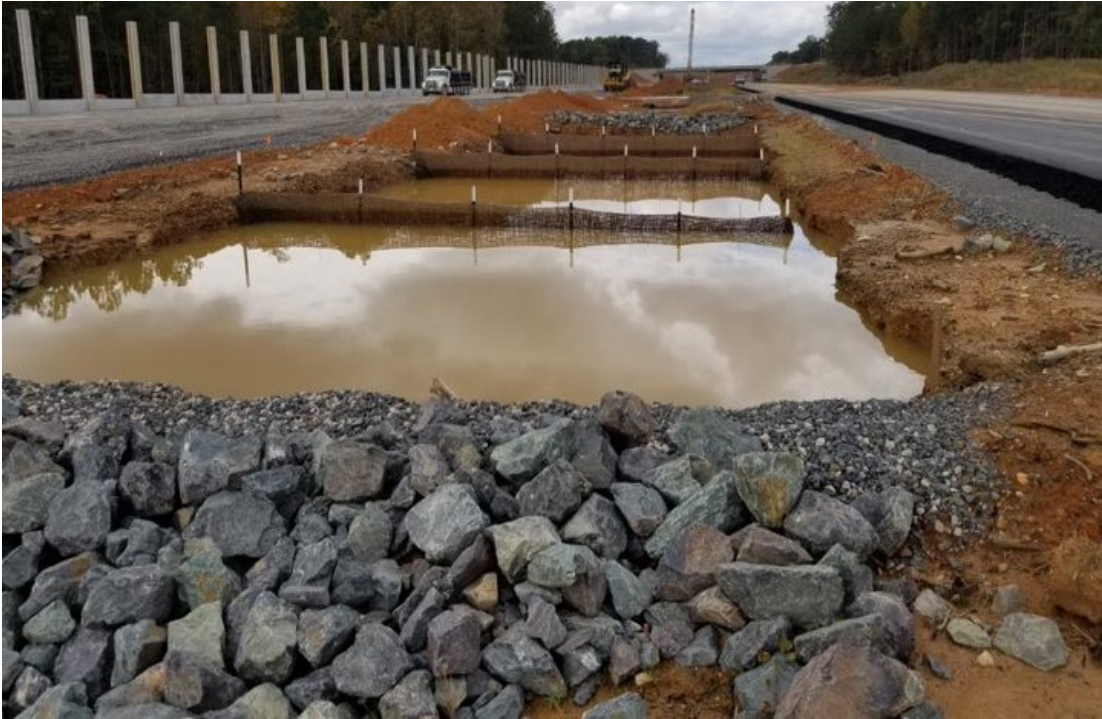
Photo- Silt Basin Type-B
