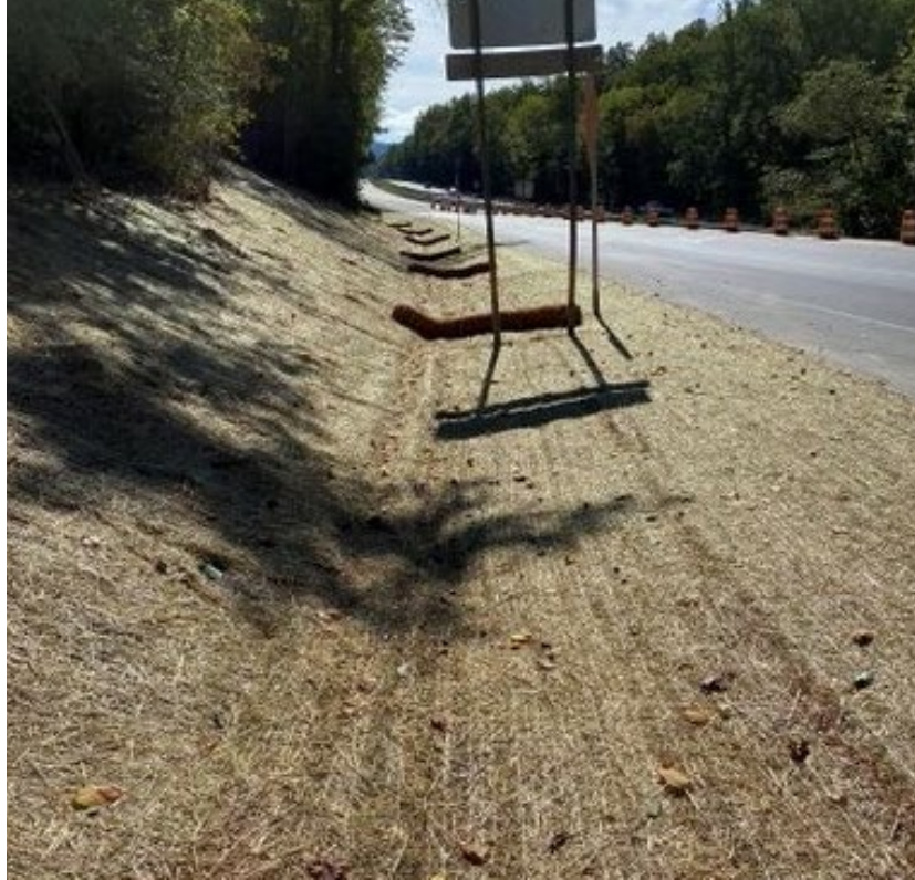
Photo- Recently completed ditch matted
