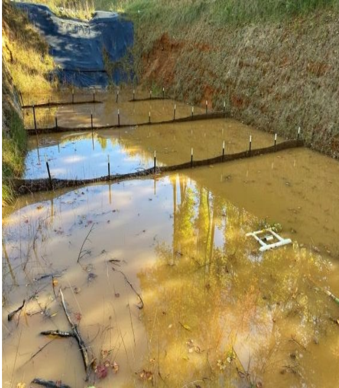
Photo- Tiered Skimmer Basin, skimmer not installed at proper elevation
