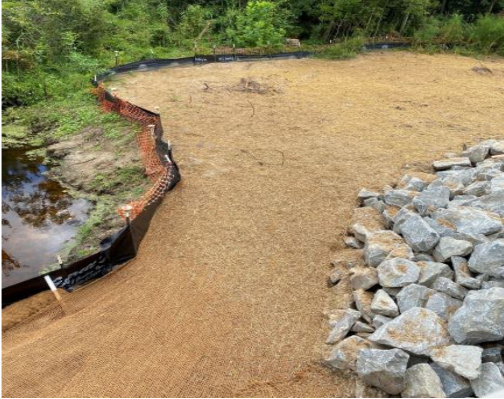
Photo- Completed areas stabilized with matting and straw
