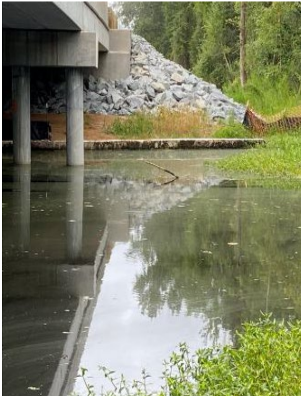
Photo-Section of silt fence missing along stream bank
