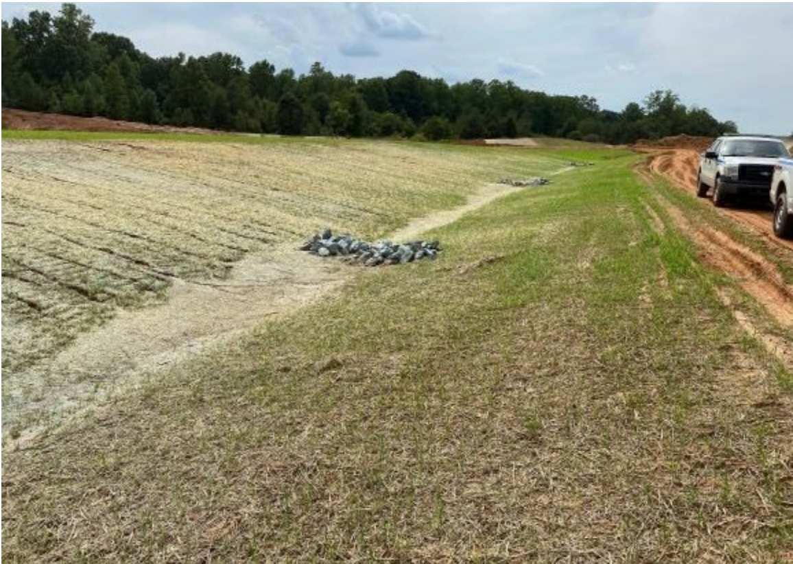
Photo- Completed areas being stabilized
