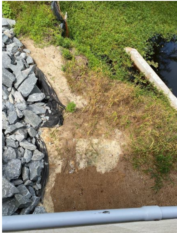
Photo-Section of silt fence missing along stream bank
