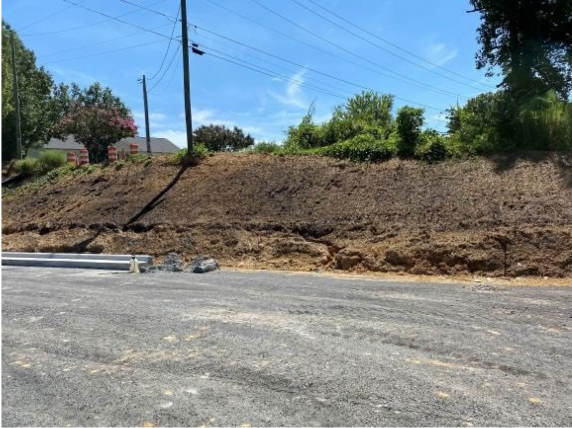
Photo- Slope mulched with straw and tackifier
