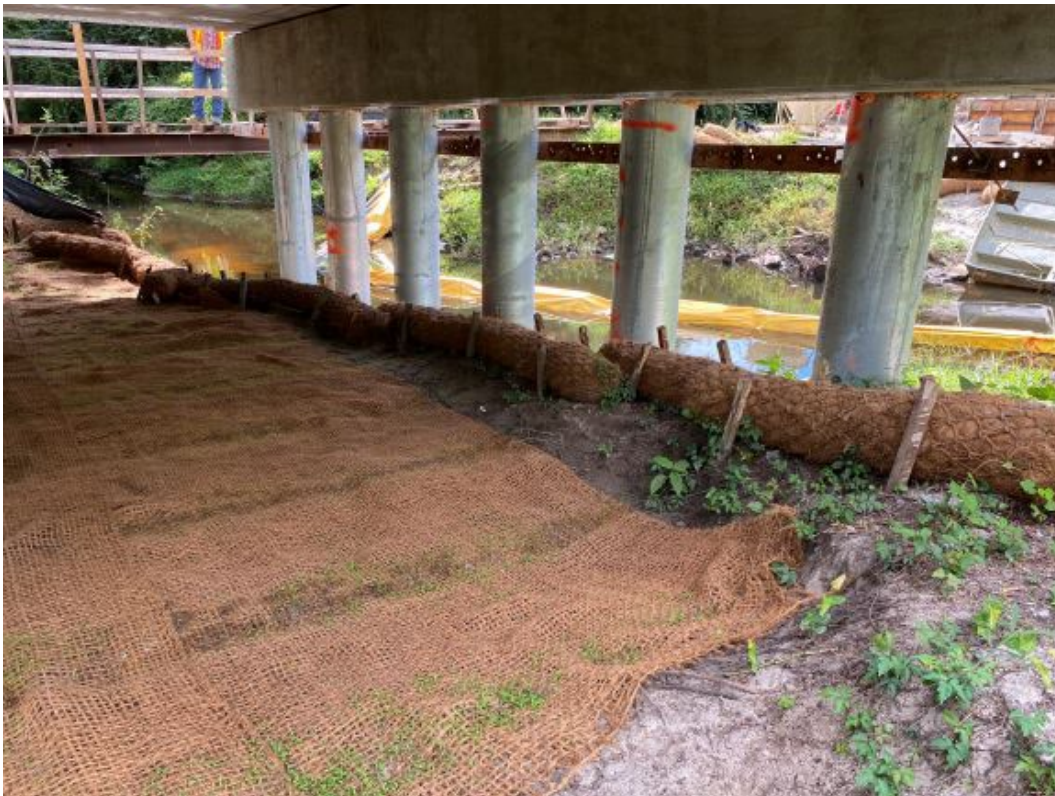
Photo-Wattles and coir fiber matting installed above stream bank
