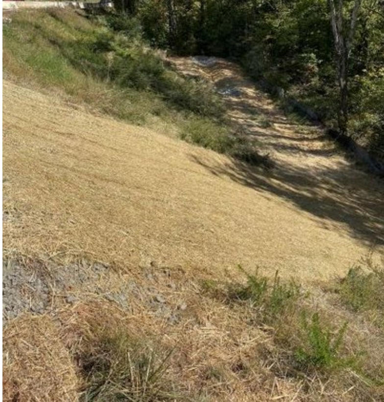
Photo- Skimmer Basin removed and area stabilized
