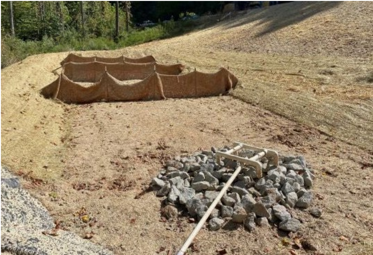
Photo- Recently installed Skimmer Basin
