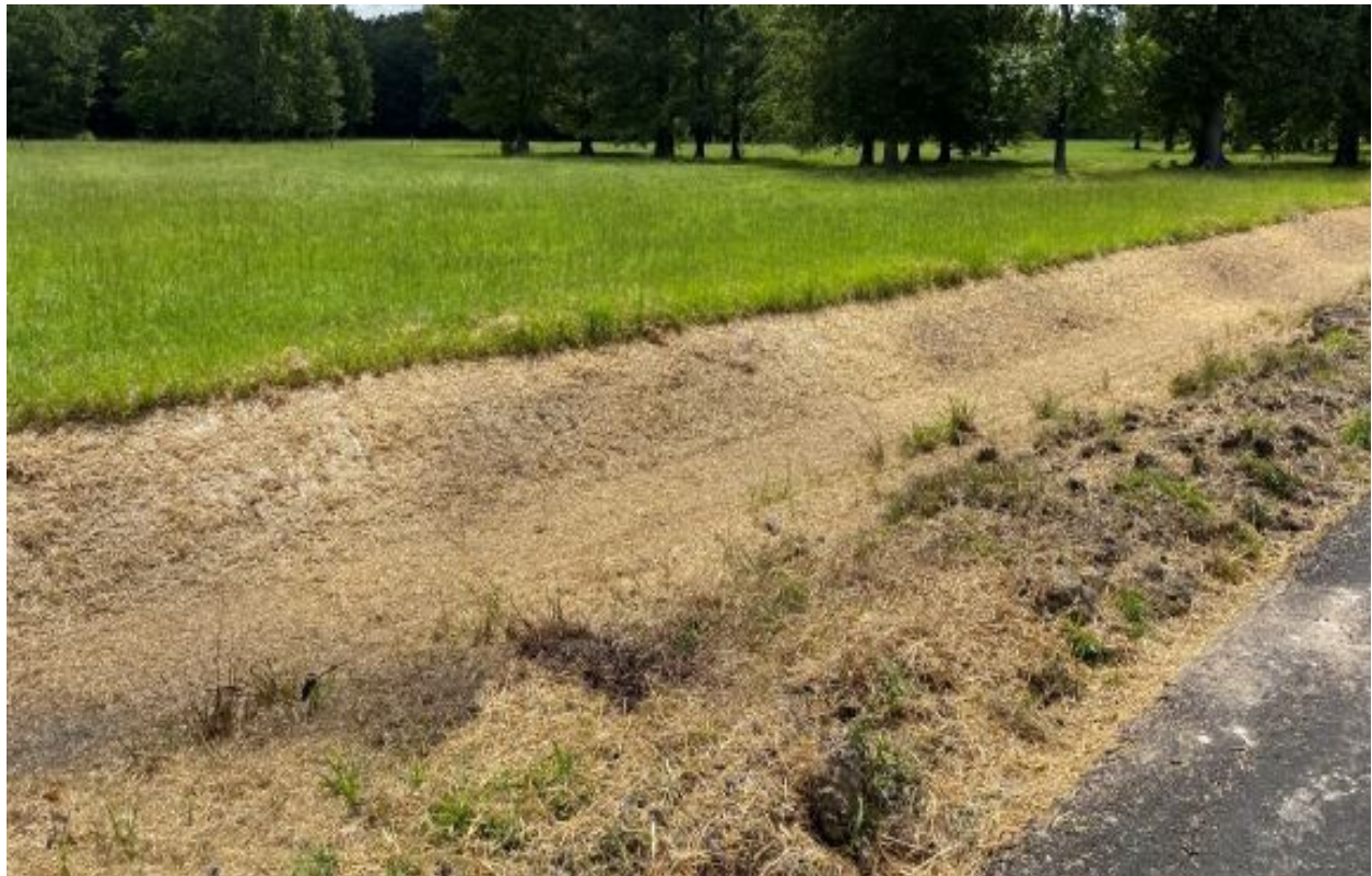
Photo- Ditch mulched with straw and sparse tackifier
