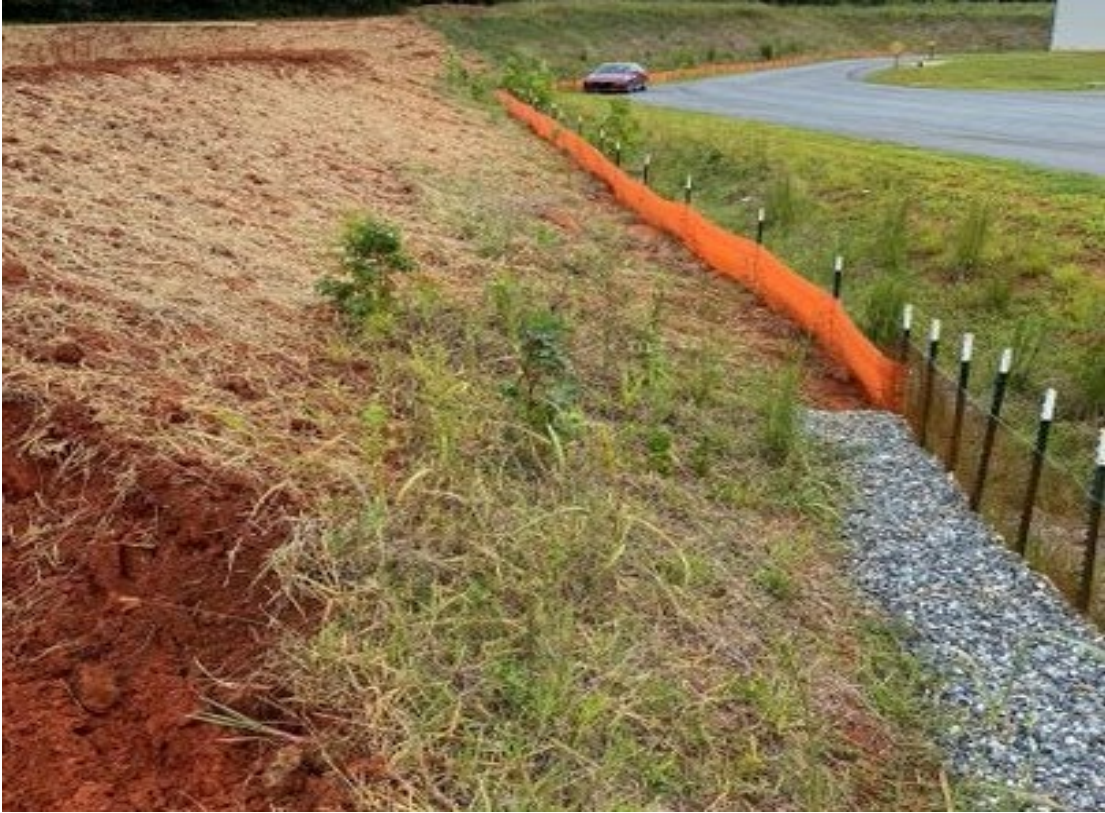
Photo- Borrow Site perimeter measures
