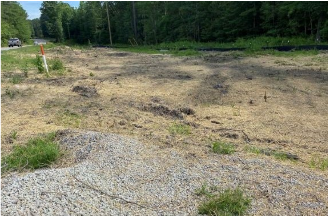
Photo- Clearing complete, areas mulched with straw
