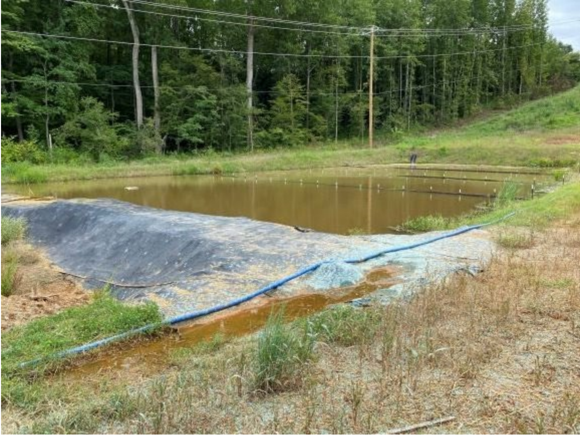
Photo- Skimmer Basin receiving water from culvert work area being dewatered
