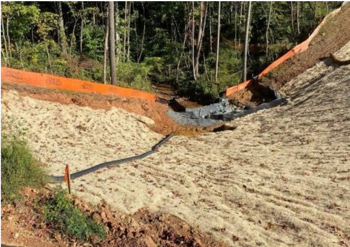
Photo- Slope repaired and matted
