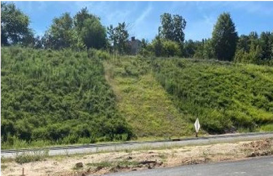
Photo- Previous slope failure repaired and stabilized
