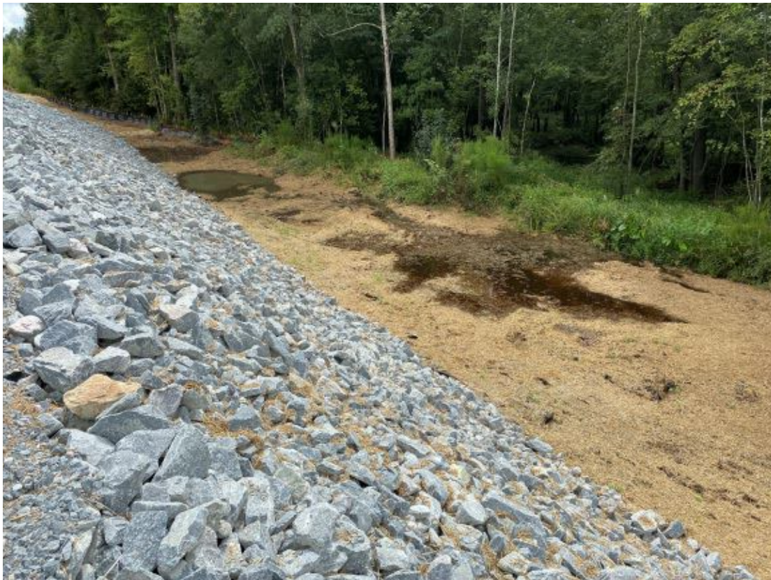
Photo- slopes complete and areas mulched with straw
