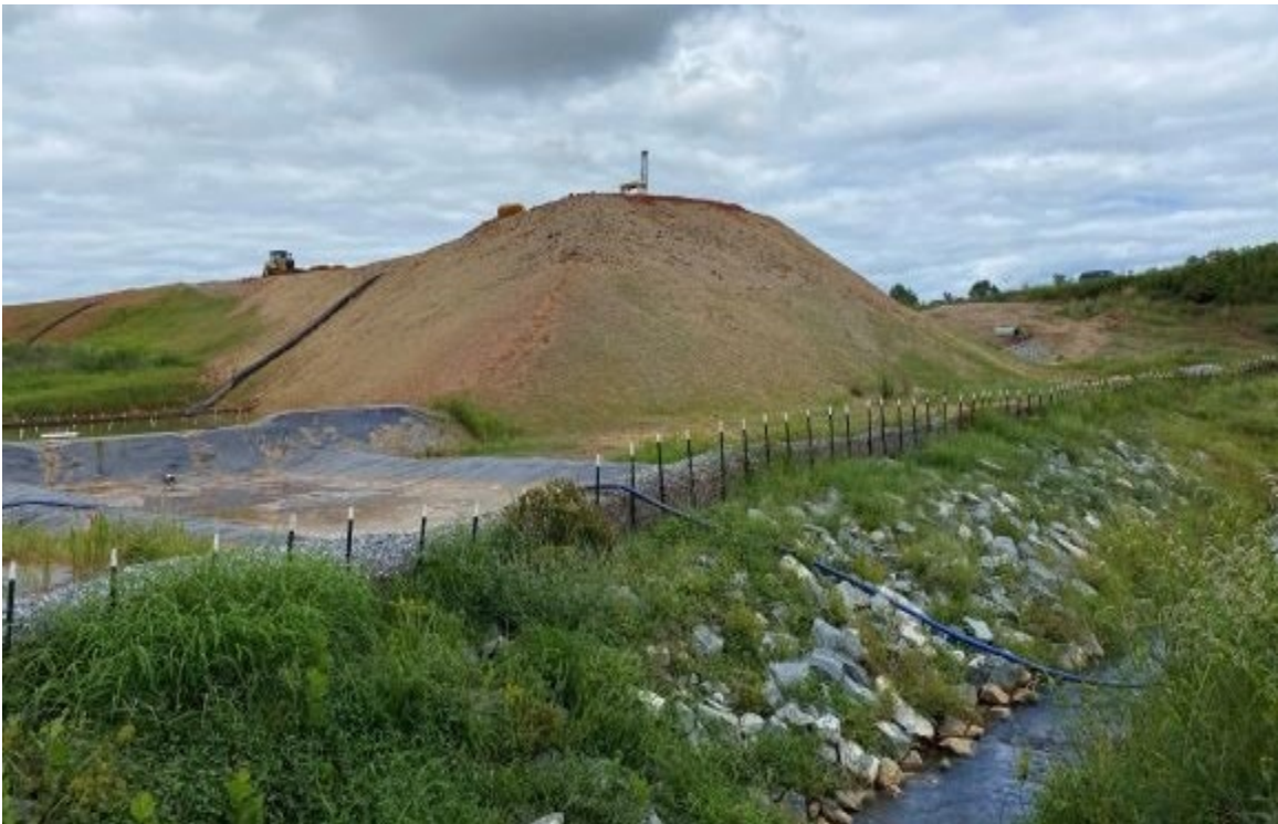
Photo- Slope being stabilized
