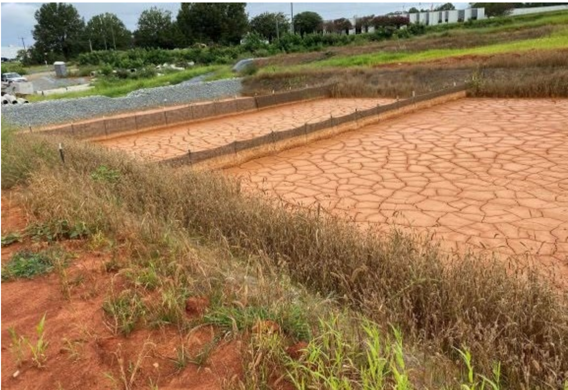
Photo- Temporary Rock Sediment Dam, Type B with trap area
