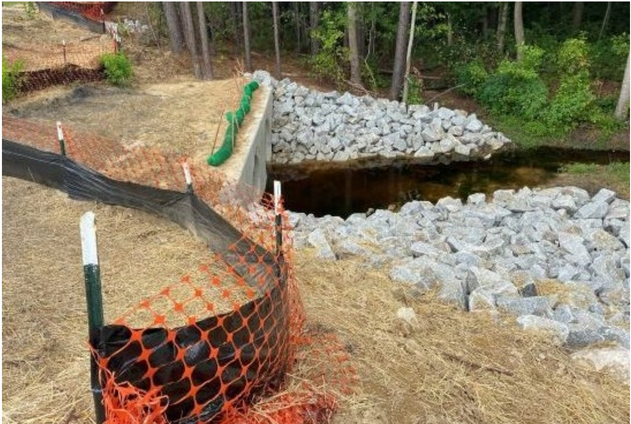
Photo- Culvert construction complete
