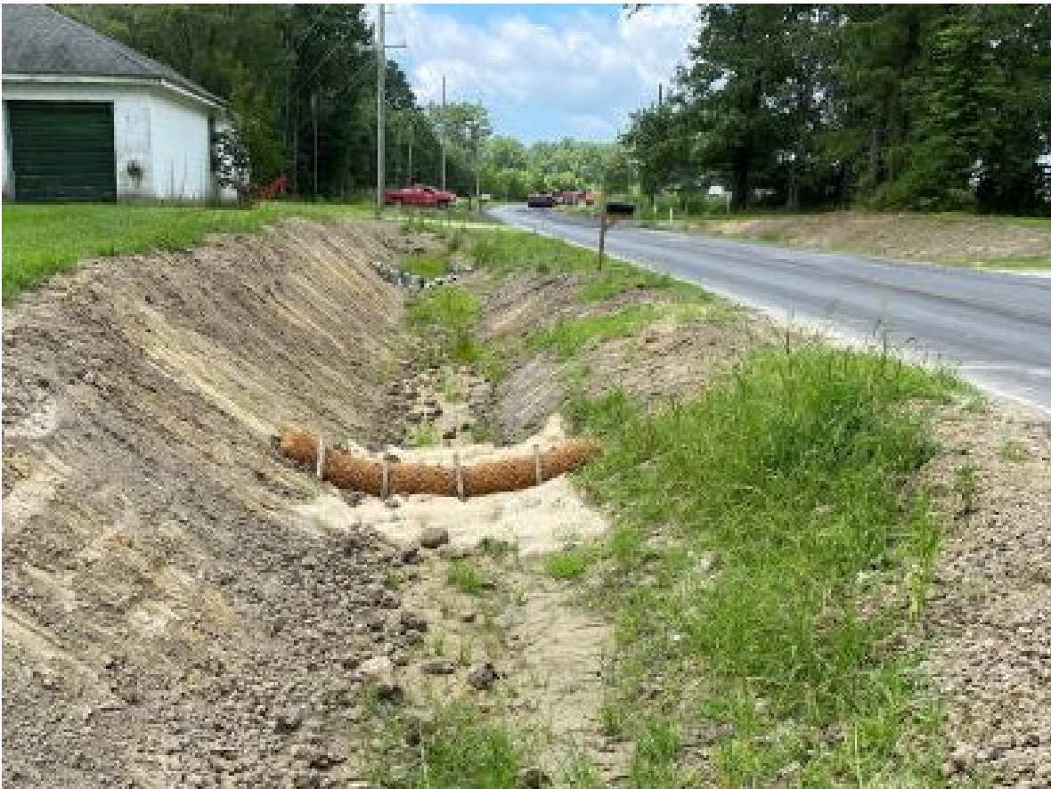
Photo- Wattle and check dam recently replaced
