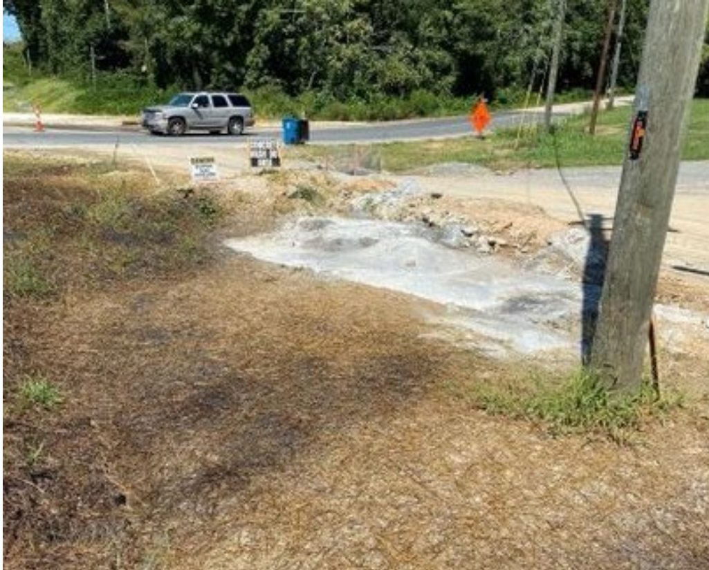
Photo- Concrete washout pit
