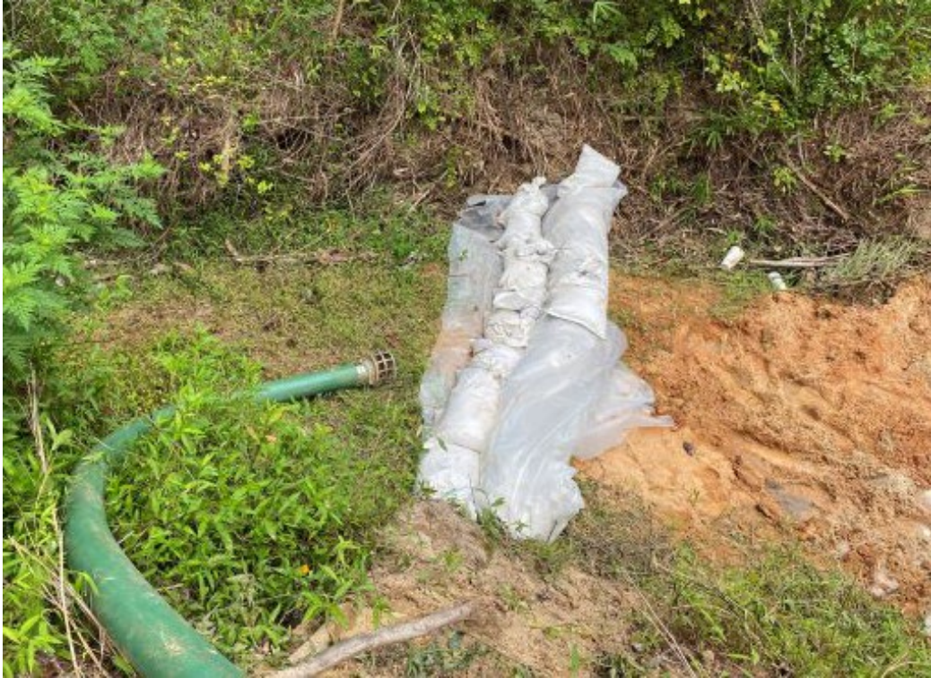
Photo- Downstream impervious dike
