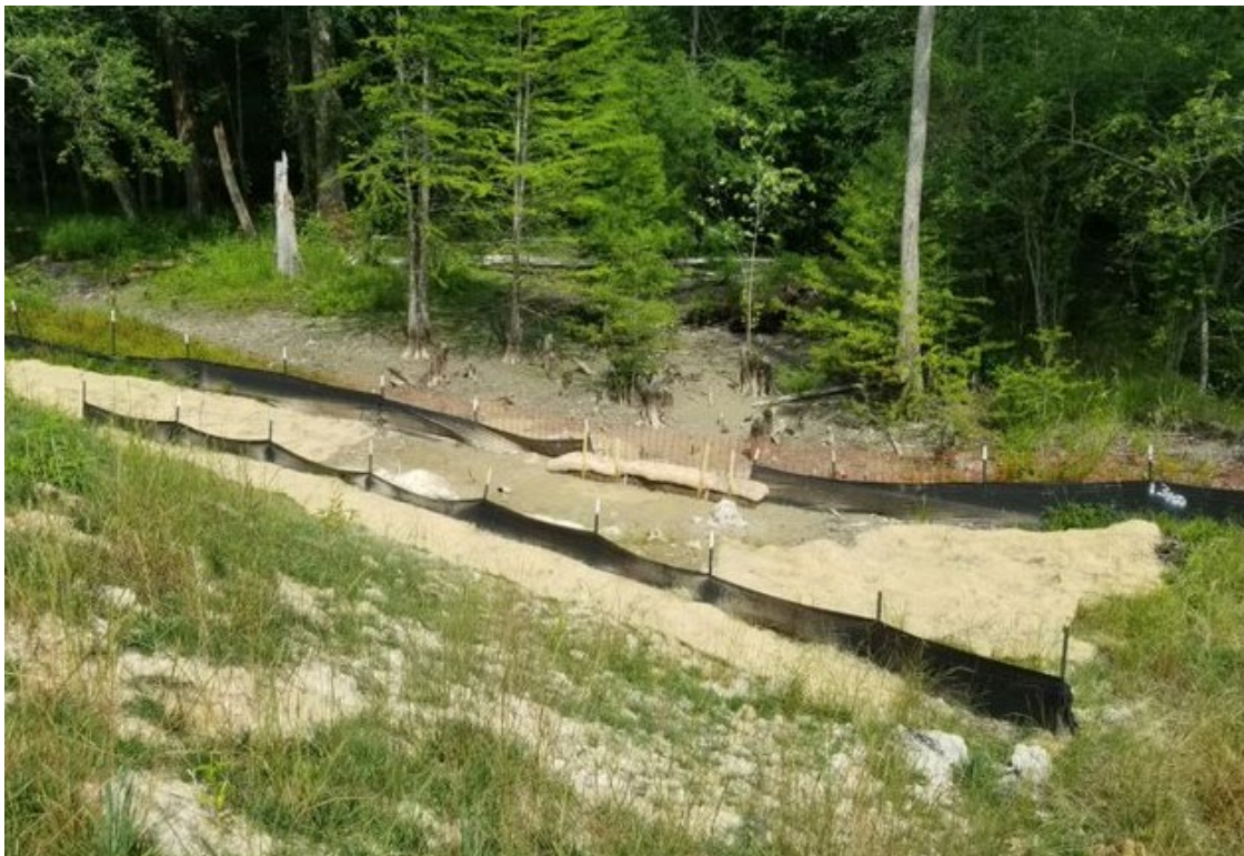
Photo- Additional silt fence row and wattle break repaired
