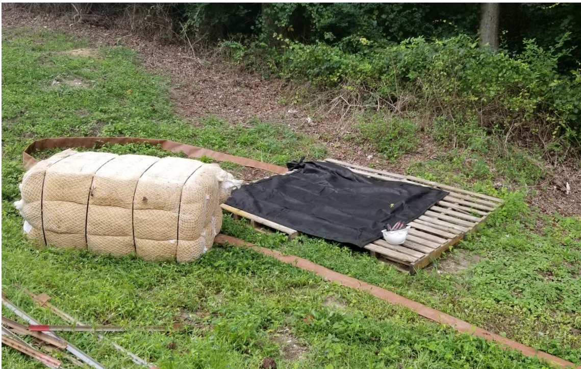
Photo- Silt Bag for work area dewatering
