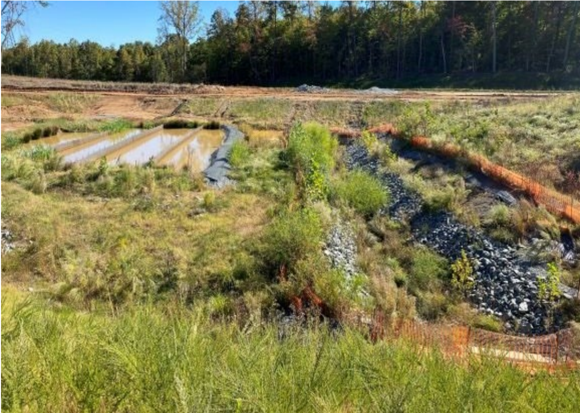
Photo- Skimmer basin and channel stabilization
