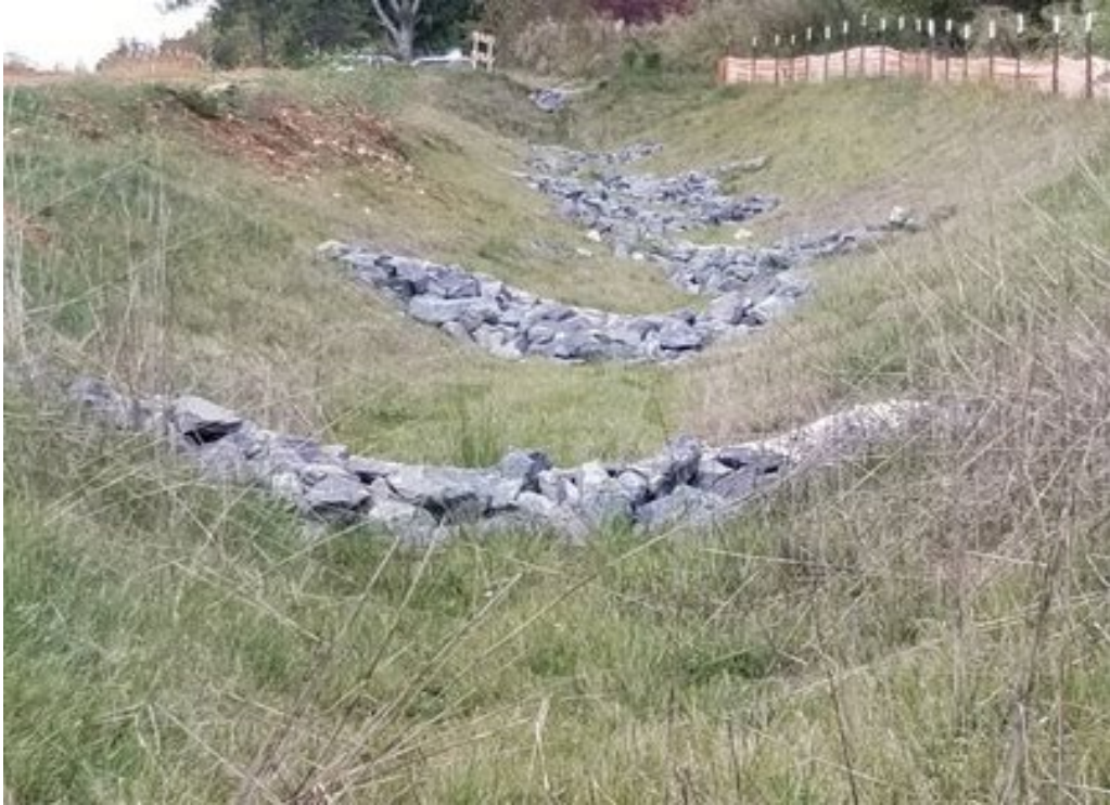
Photo- Stabilized ditch with rock check dams
