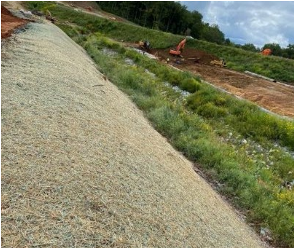
Photo- Completed slopes and channel stabilization
