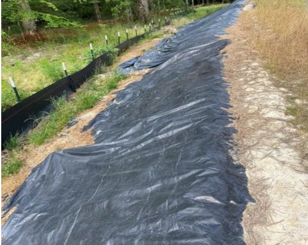
Photo- Geotextile liner on slope
