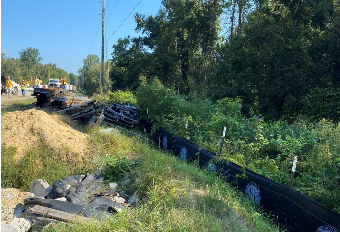
Photo- Materials lying on top of silt fence
