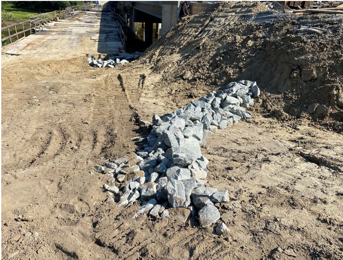
Photo- Rock checks added to control runoff
