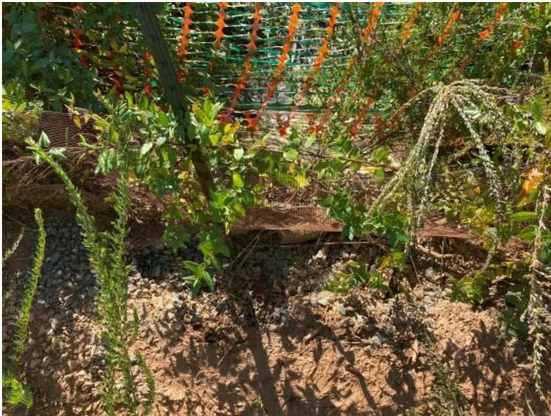
Photo- Silt fence outlet at basin outlet undermining
