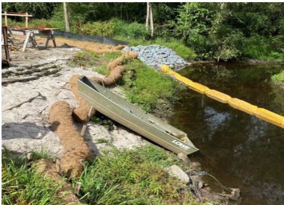
Photo- Wattles and turbidity curtain installed
