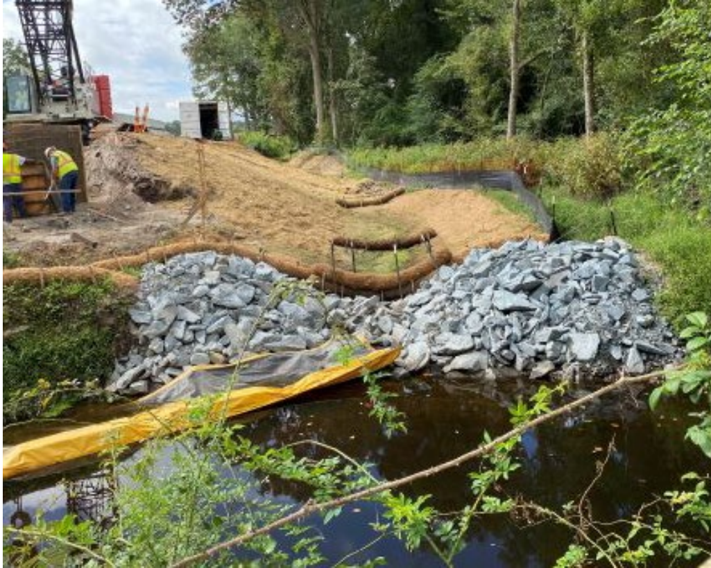
Photo- Completed ditch and slope mulched with straw
