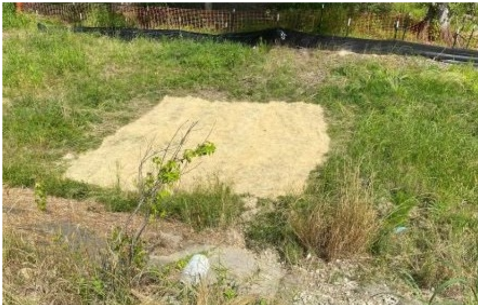
Photo- Slope repaired and matted
