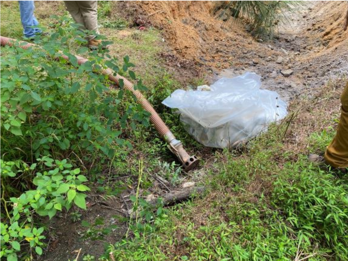
Photo- Upstream impervious dike
