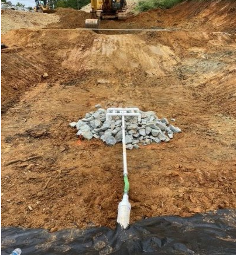
Photo- Tiered Skimmer Basin construction
