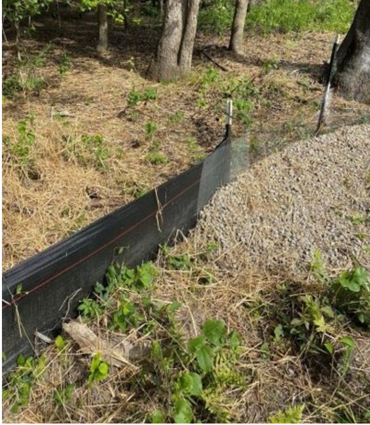
Photo- Previous minor losses cleaned up and area mulched with straw
