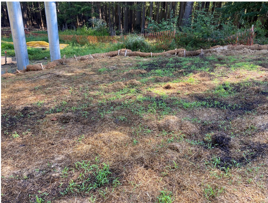
Photo- Completed areas being stabilized
