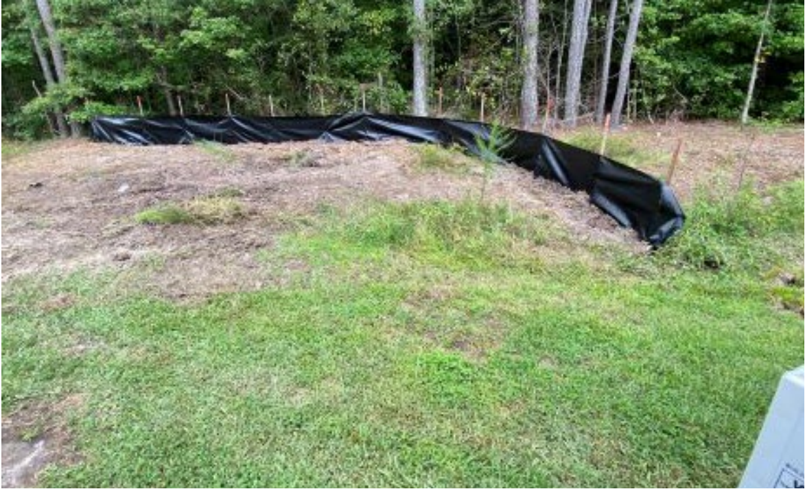
Photo- Area disturbed for pipe storage
