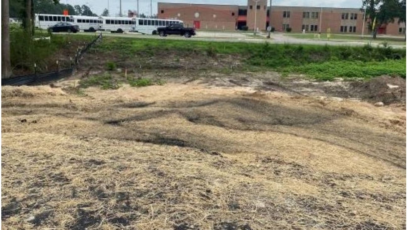
Photo- Completed Areas mulched with straw
