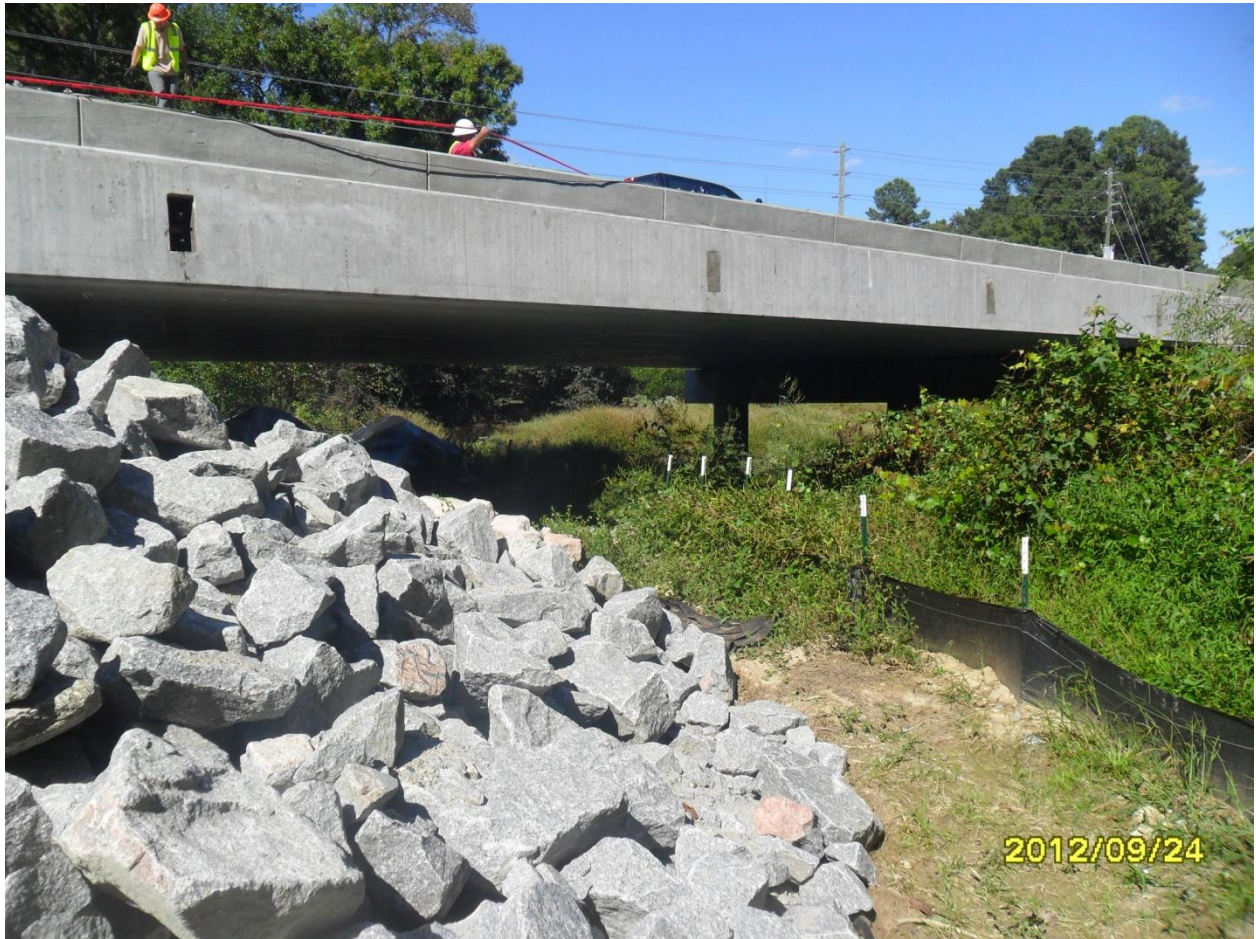
Bridge over Stoney Creek, SR 1670
