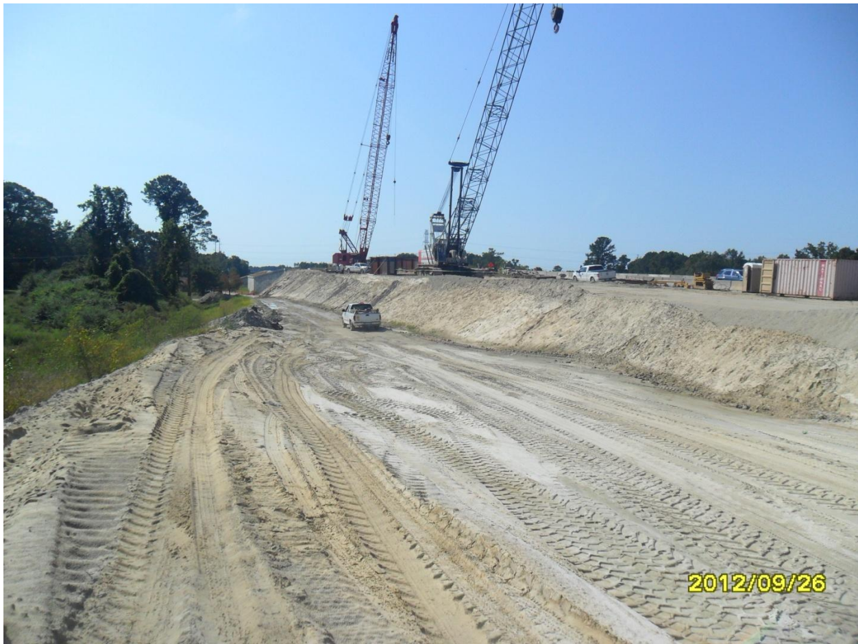
Bridge construction on Western Parkway
