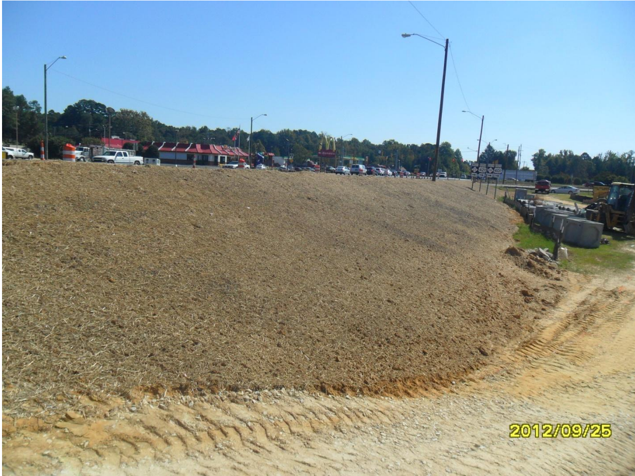
Fill slope on US 401, Lillington
