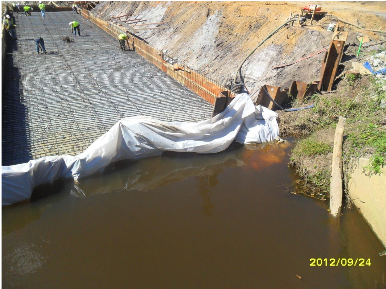
Box culvert being formed on US 158, Murfreesboro Bypass
