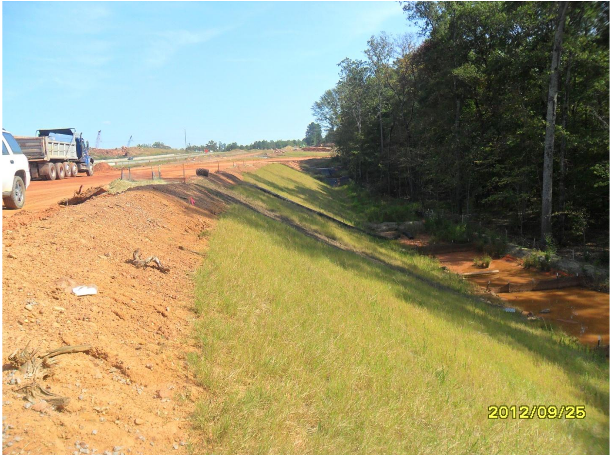
US 421, Sanford Bypass
