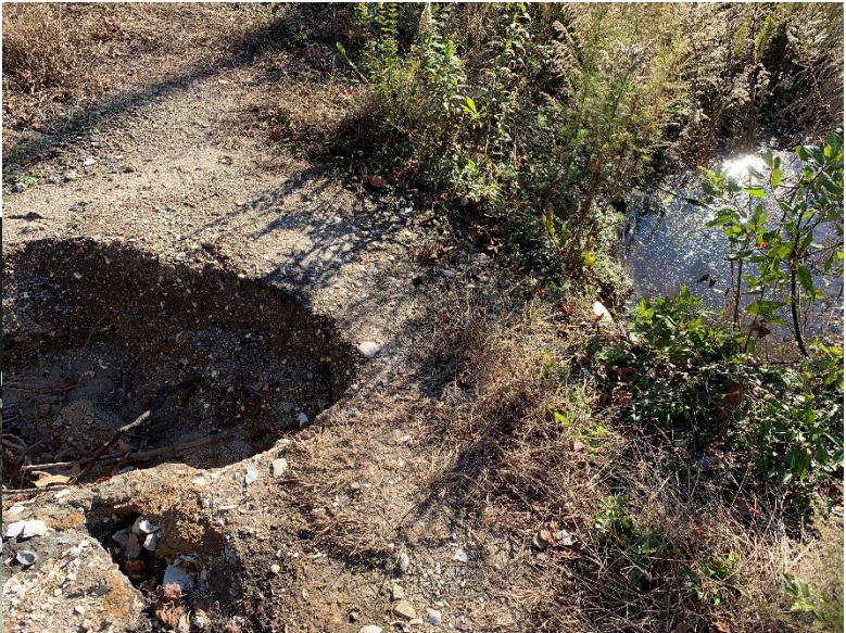
Looking to the west. December 8, 2020. Erosional gully along the waterway.
