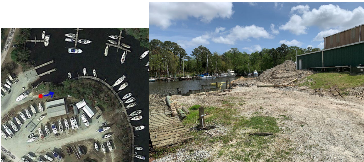
Looking to the east. April 14, 2022. Unpermitted work.
