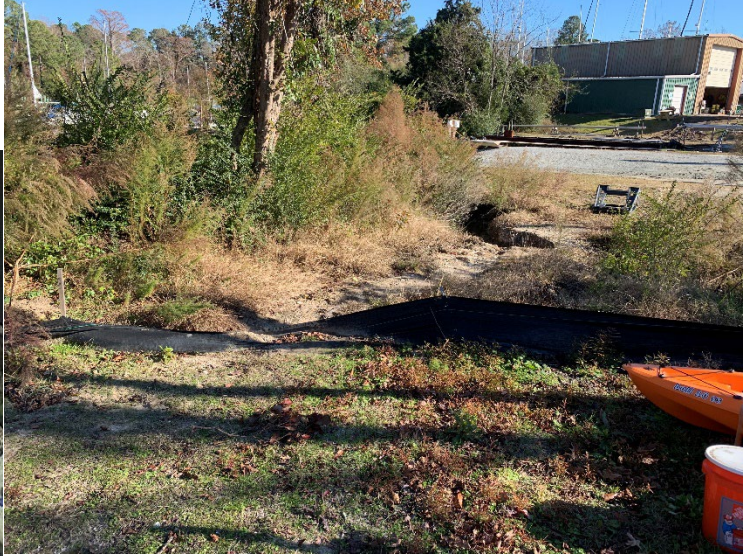
Looking to the east. December 8, 2020. Erosional gully forming behind overwashed silt fence.
