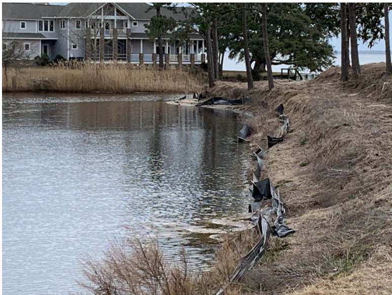
Looking to the east. February 10, 2021. Unpermitted work and off-site sediment washed into the waterway.
