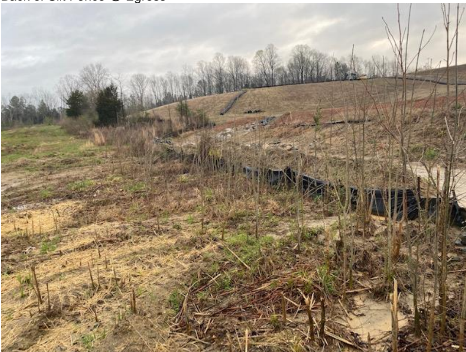
Back of Silt Fence @ Egress
