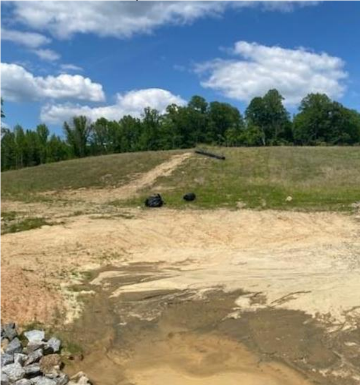
Drain Work/Scour Repair
