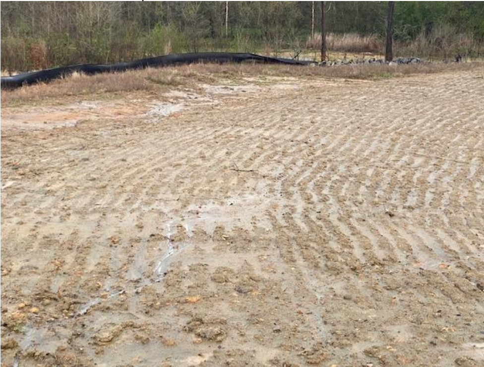
Re-Grade Bottom of Slope
