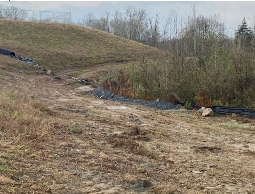
Repaired Stone Outfall
