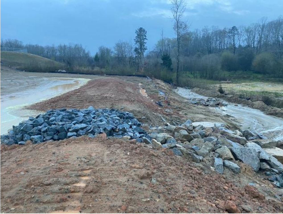
Repaired Stone Outfall
