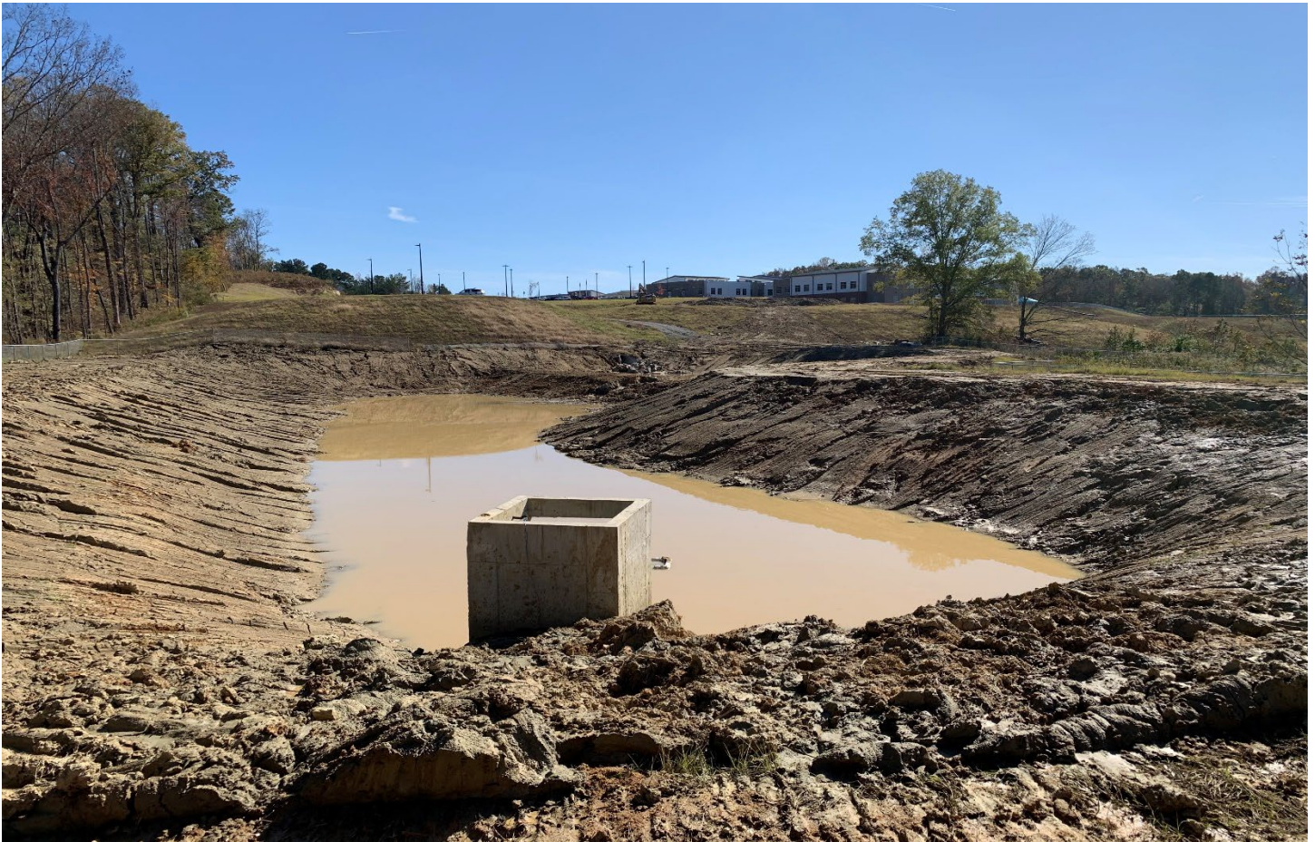
Picture #1: 11/05/2020 Sediment Basin
