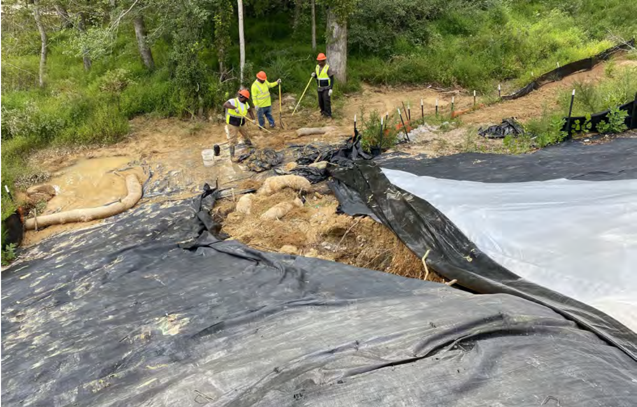
Basin berm east of Swift Creek
