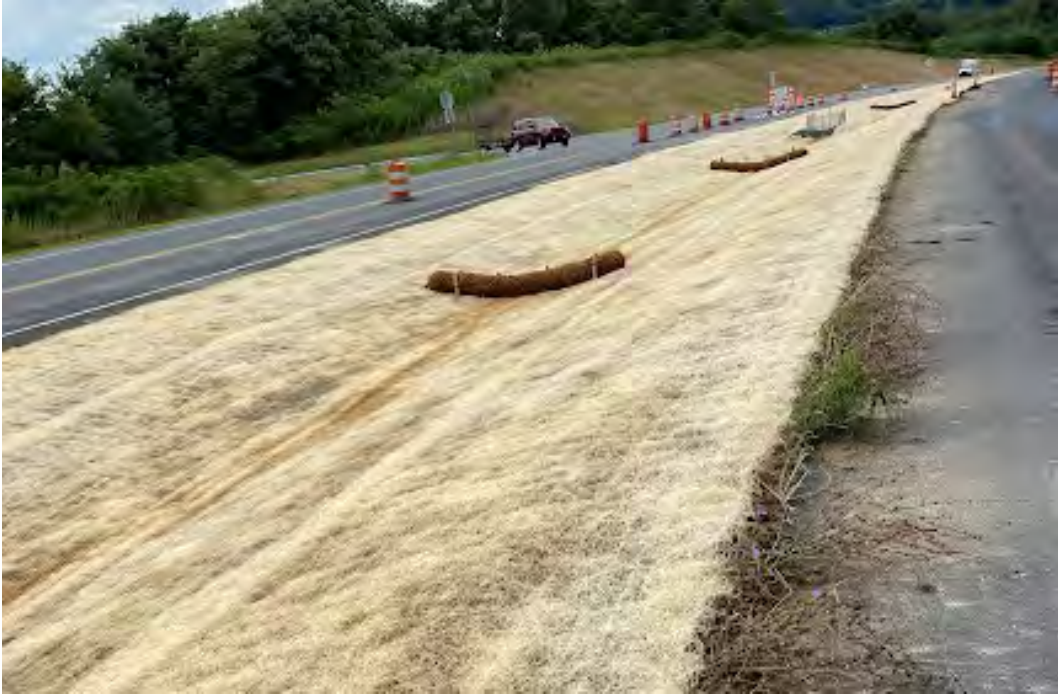
Median matted with wattles and drop inlet protection measures installed
