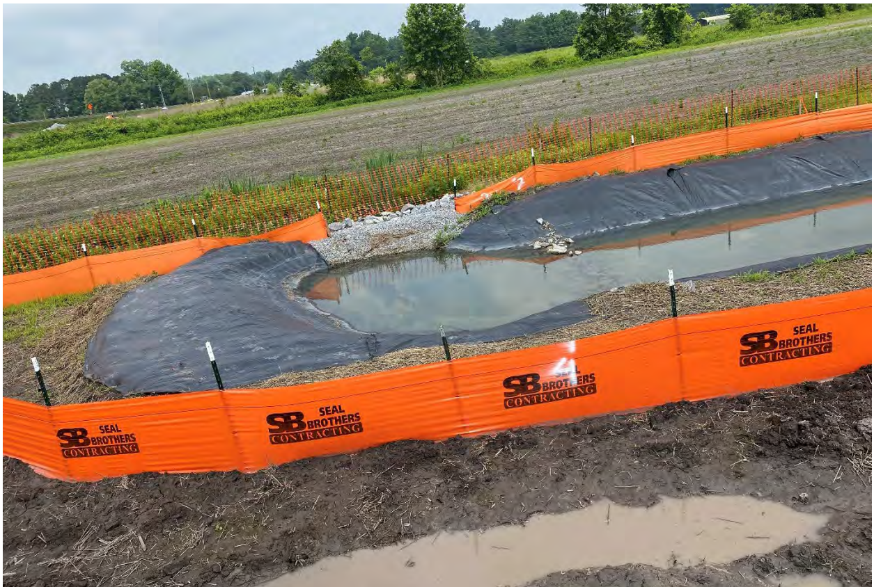
Basin and stabilized outlet on Borrow site
