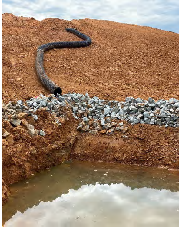
Slope drains needing to be staked down (both) and an outlet protection measure needed (left)
