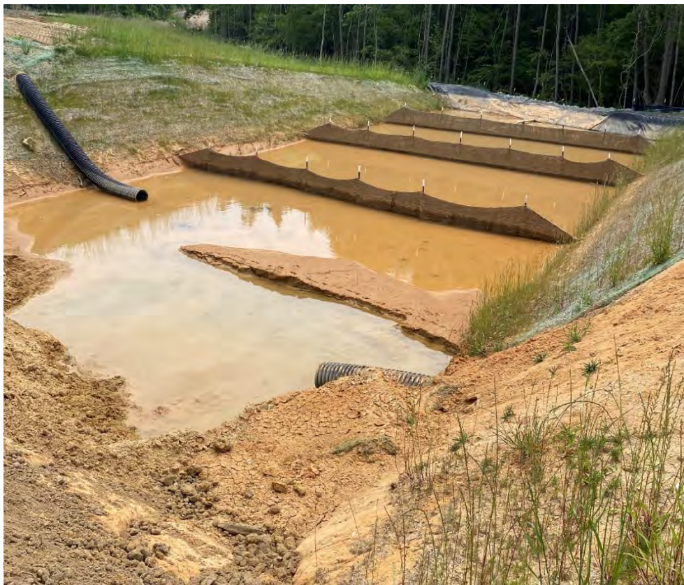
Skimmer basin at Borrow Pit
