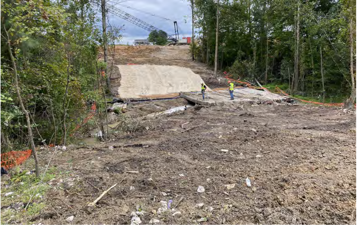
Stream where bridge demolition had occurred
