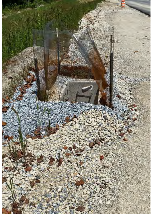
Drop inlet protection measure needing maintenance
