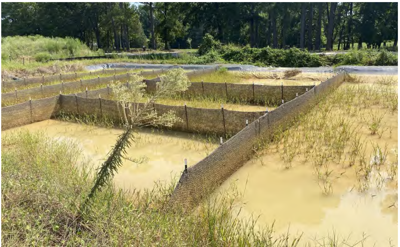
Skimmer Basin appeared to be functioning and maintained
