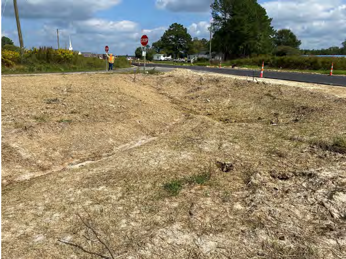
Recently graded area with straw mulch
