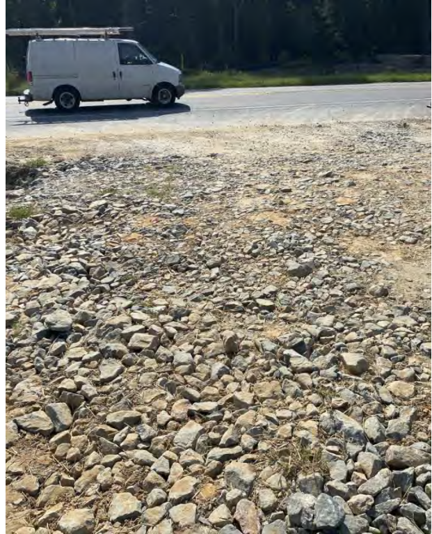
Construction entrances needing maintenance
