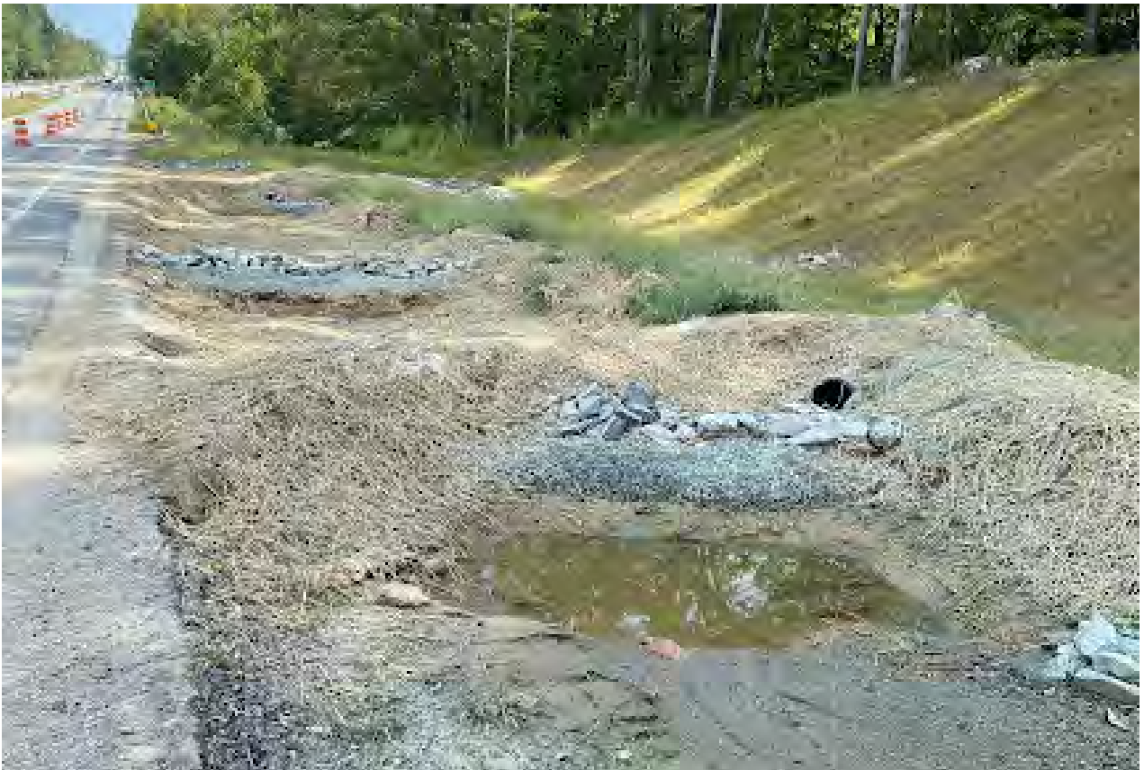
Slope drains and inlet protection measures
