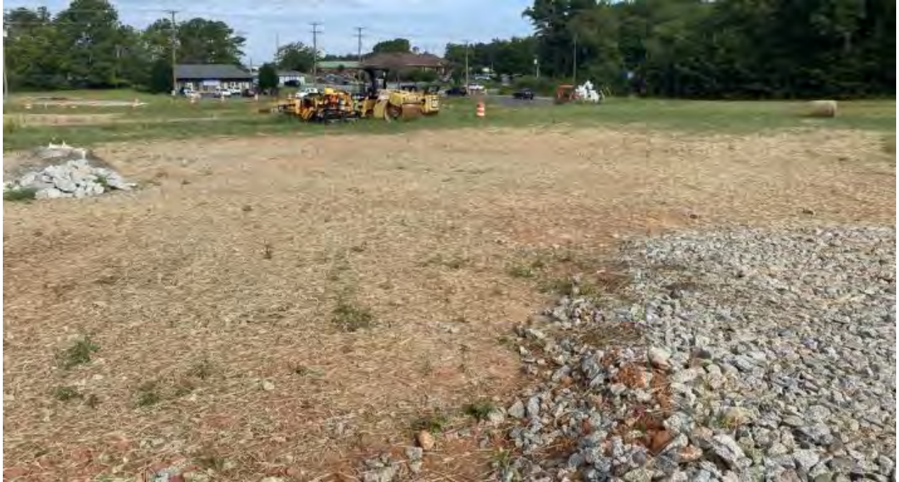
Laydown yard area being stabilized
