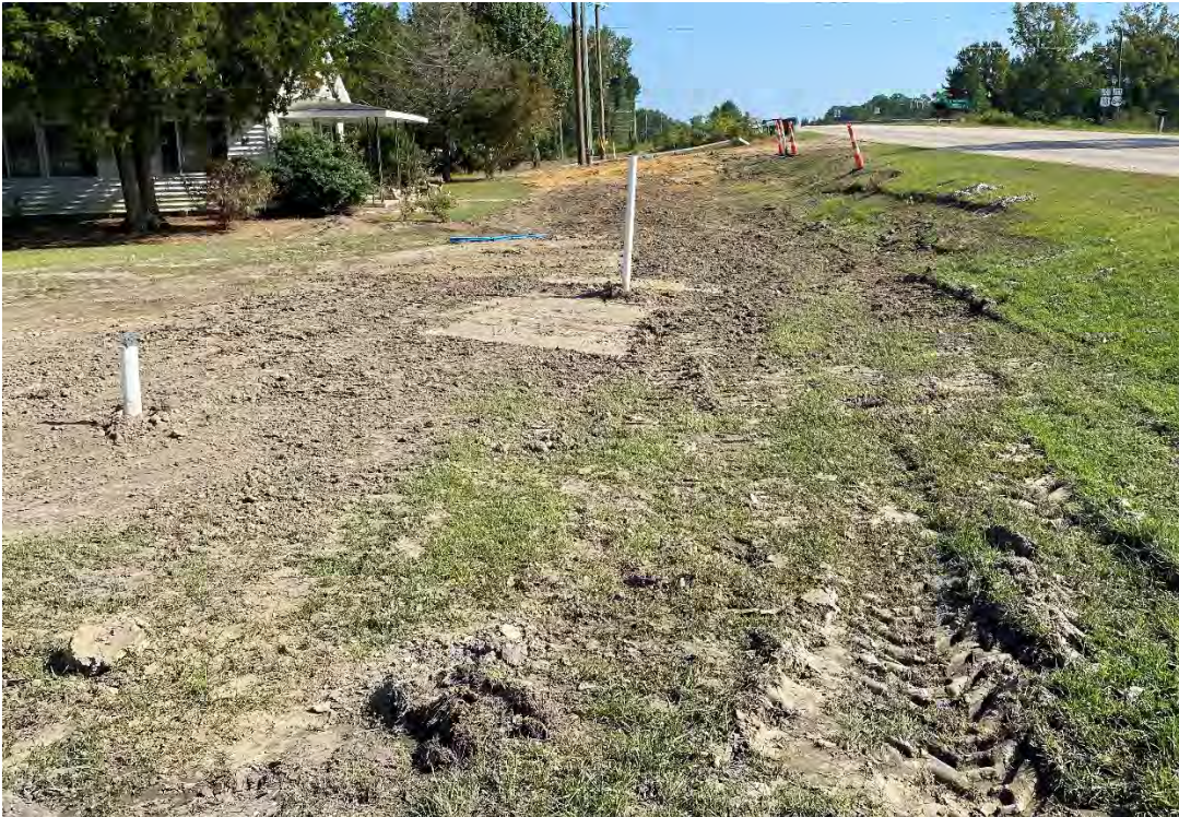
Utilities by Others being installed
