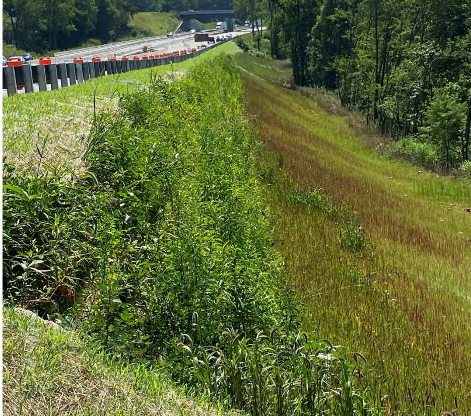
Living retaining wall installed and slopes stabilized
