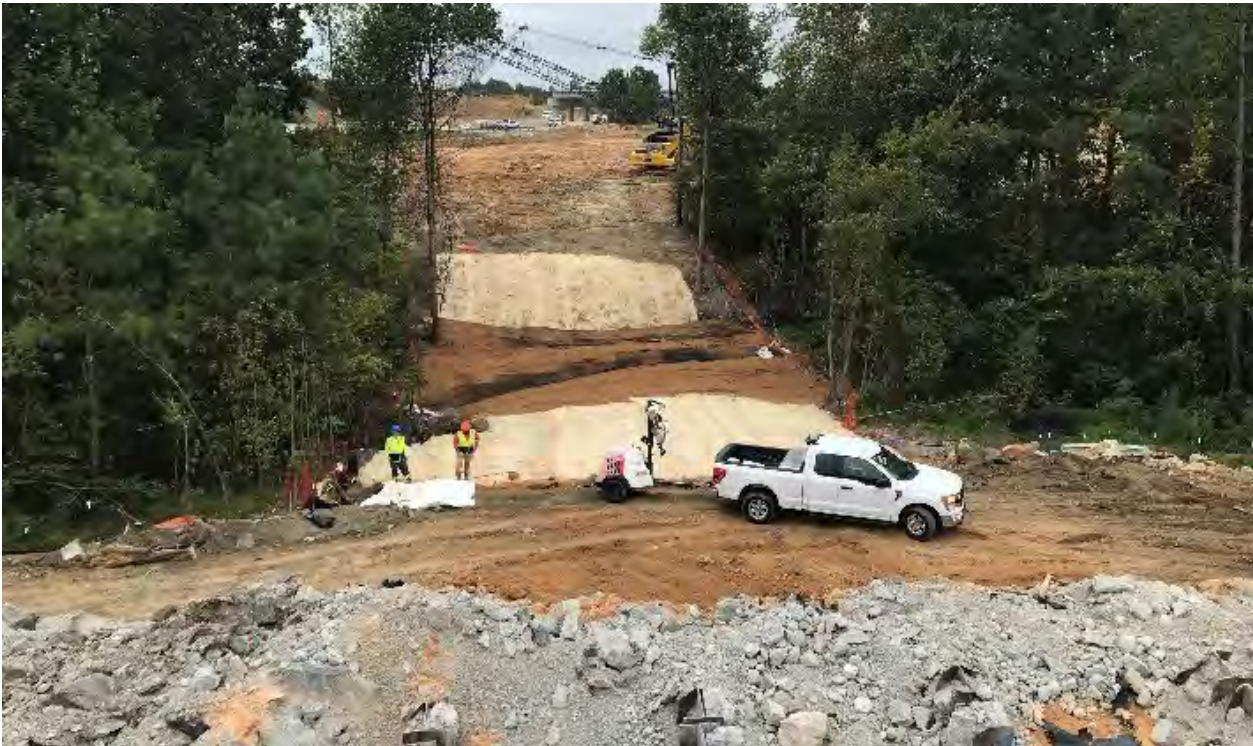
Stabilization around stream where bridge demolition had occurred
