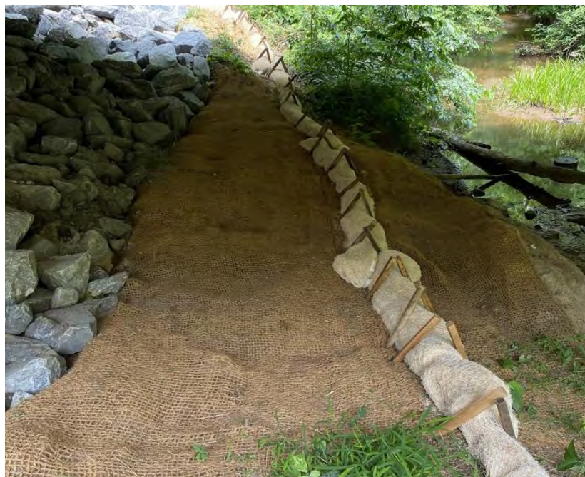
Perimeter wattles installed along stream bank
