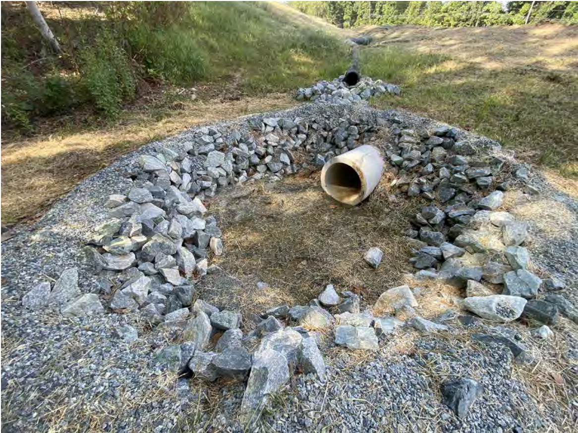
Rock doughnut inlet protection
