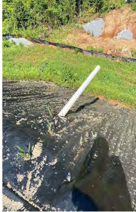
Skimmer basin and outlet pipe
