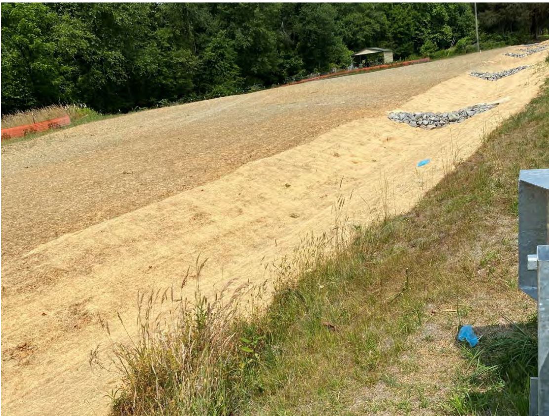
Staging Area seeded and mulched with straw
