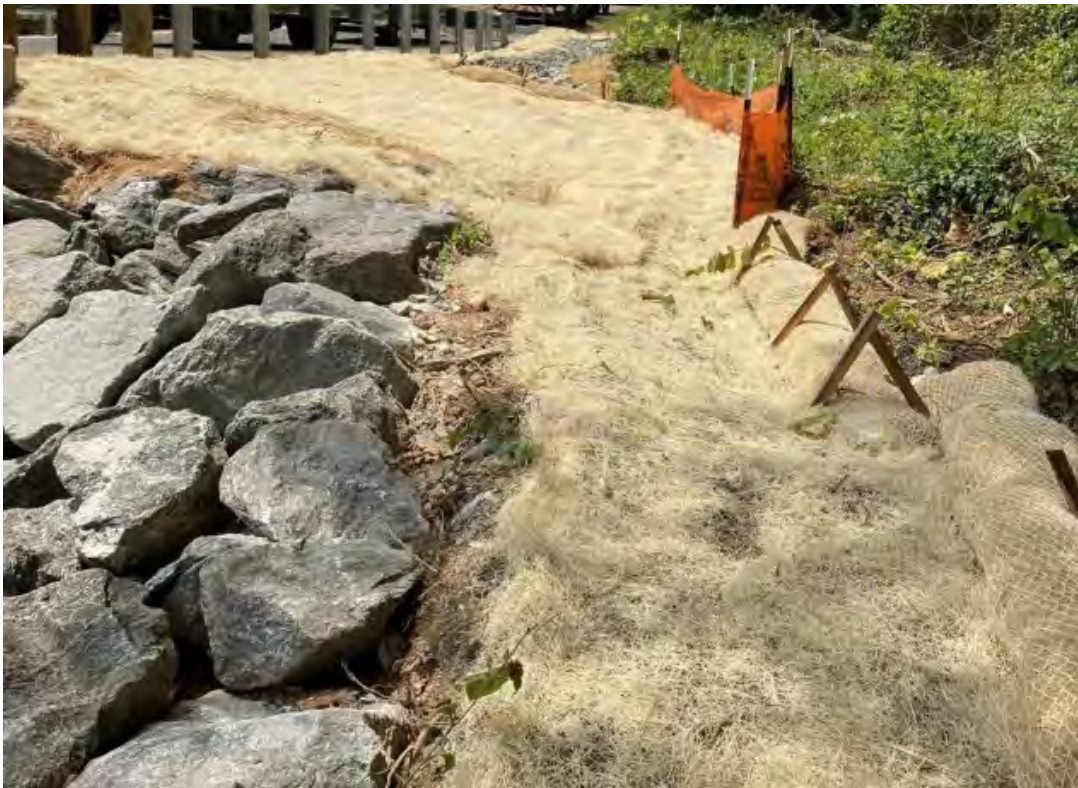
Recently completed areas being stabilized
