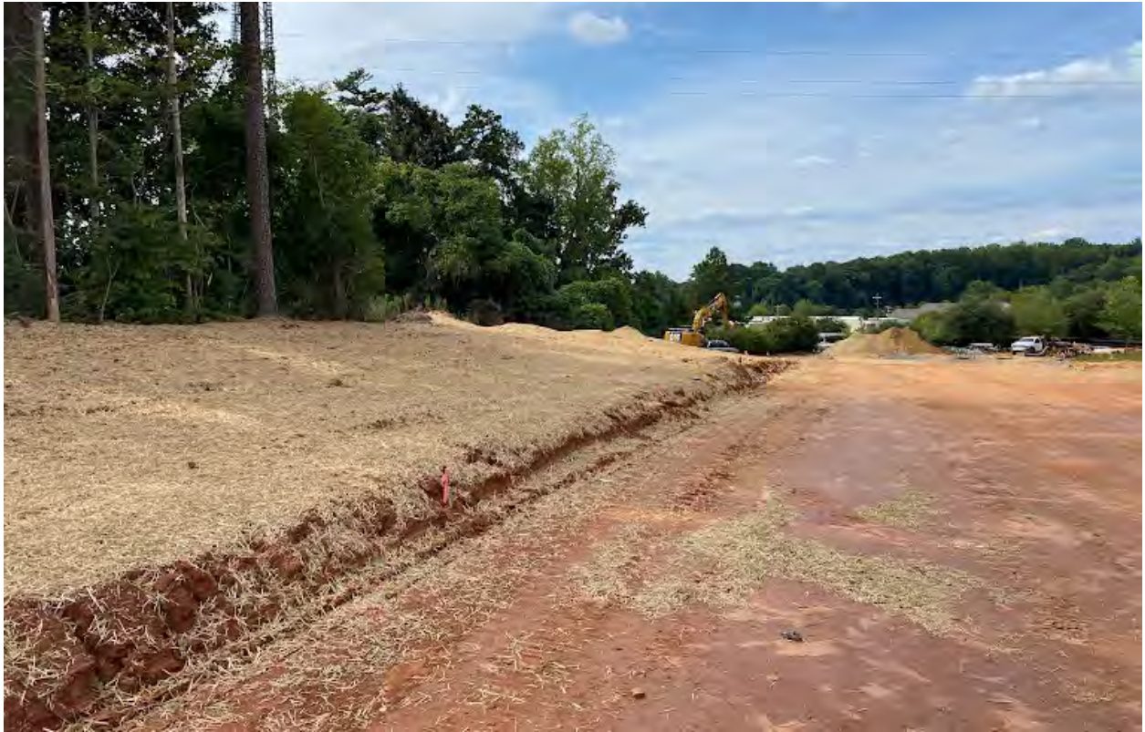
Areas recently seeded and mulched with straw
