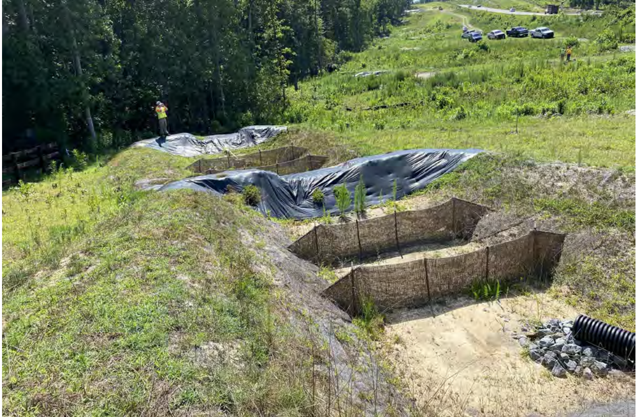
Tiered basin installed and cleared area stabilized
