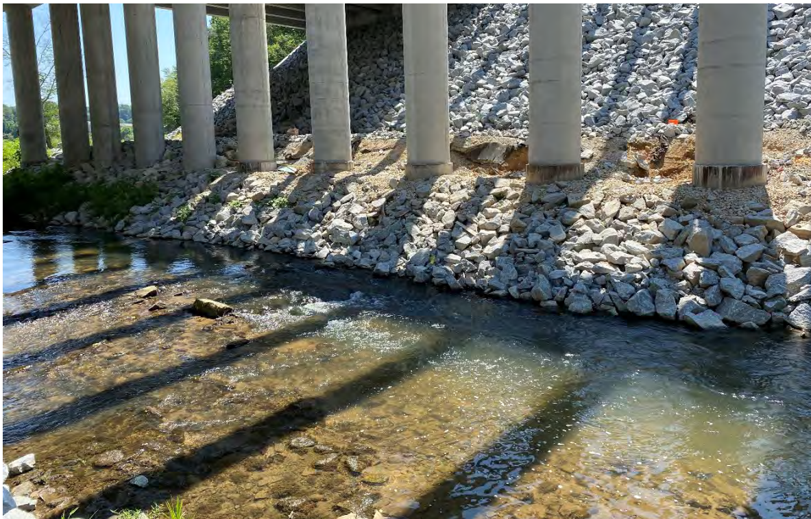
Stream bank stabilization under new bridge
