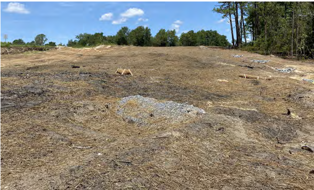
Area seeded and mulched with straw
