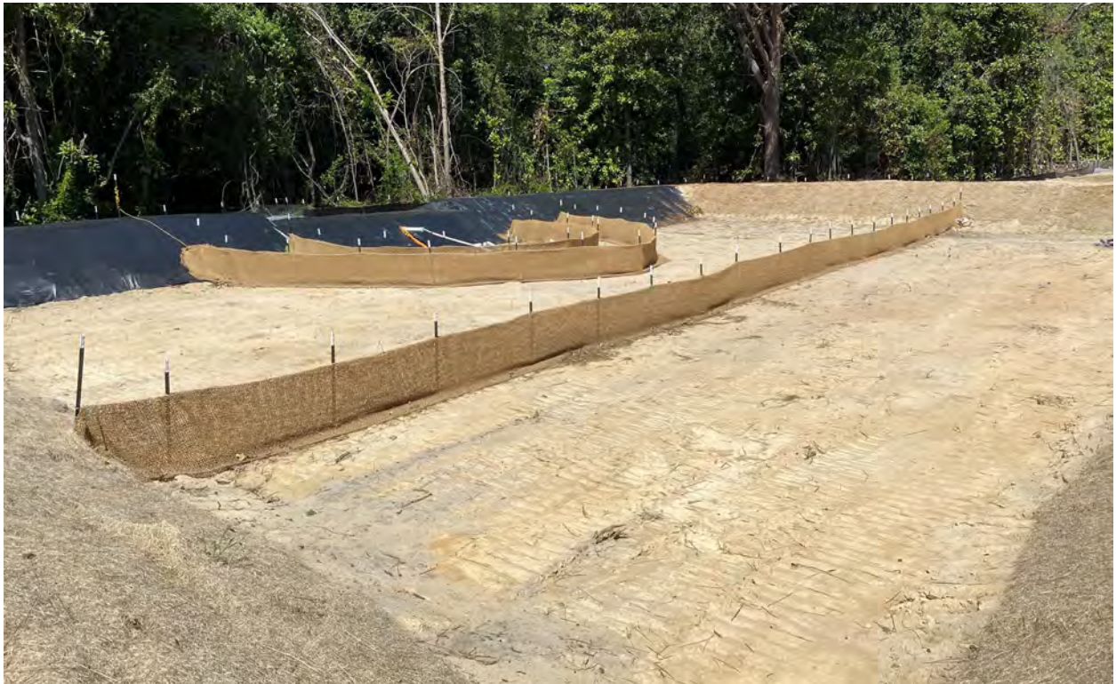
Recently installed basin
