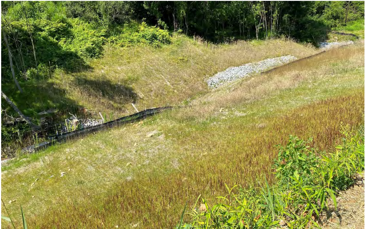
Channel change completed and area stabilized
