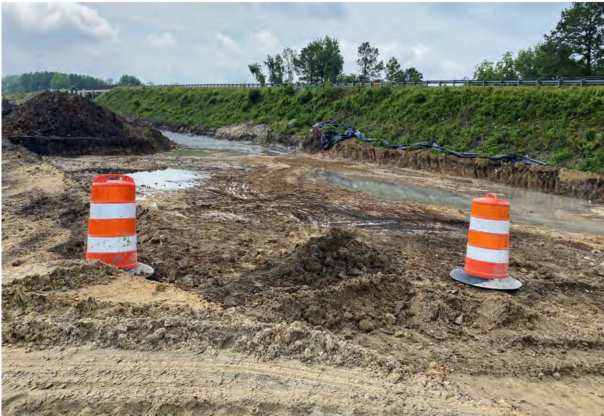
Area being dewatered and pumped into basin
