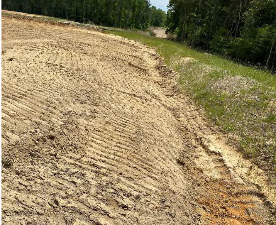
Diversion Ditch at Borrow Pit
