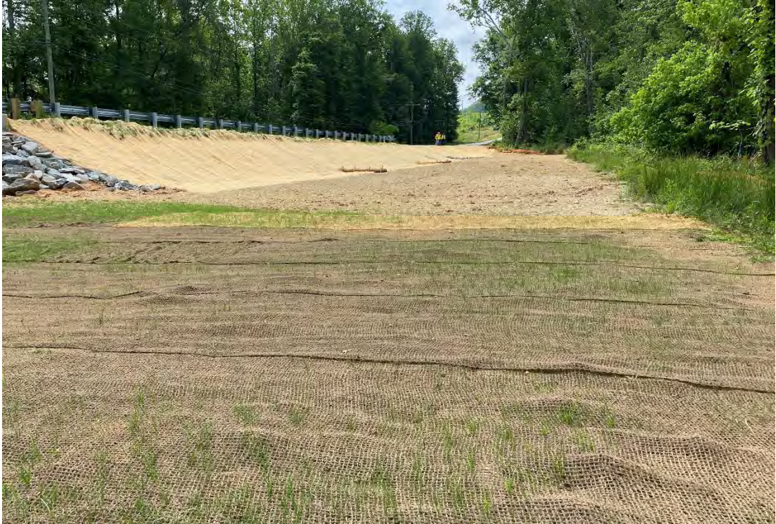
Areas being stabilized
