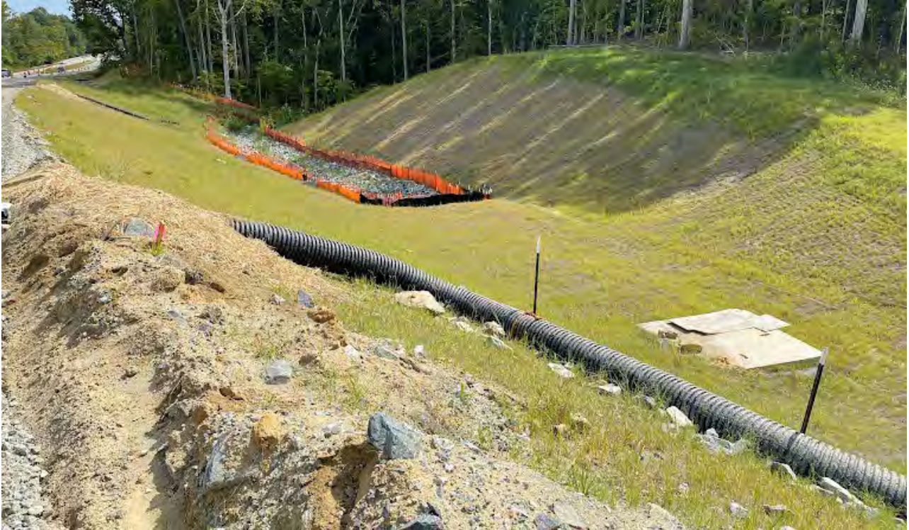
Completed channel change
