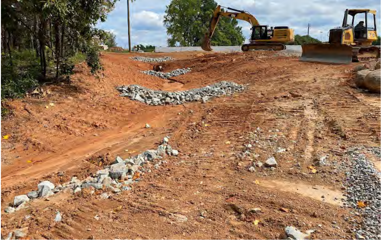
Check dams installed
