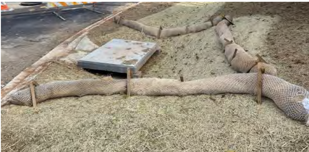
Recently matted area and wattles installed
