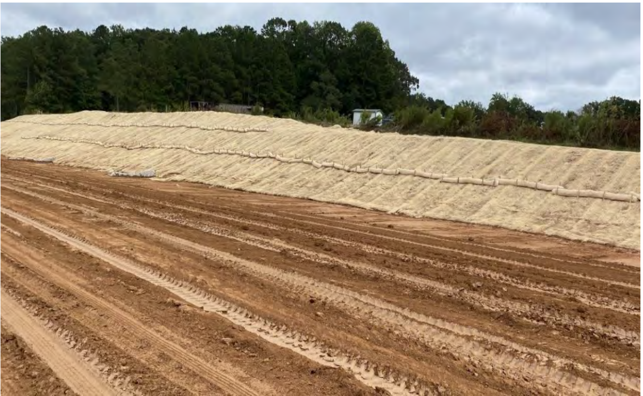
Slopes matted and wattle breaks installed
