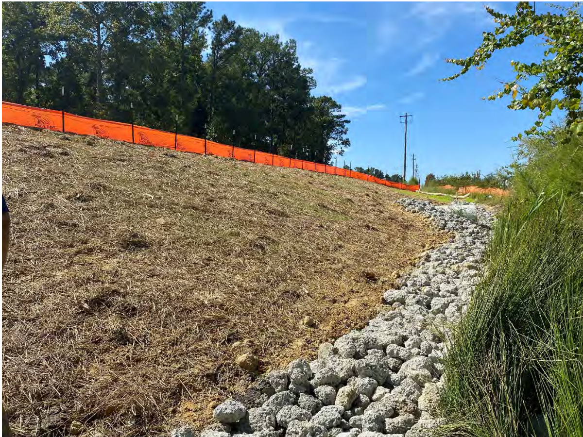
Completed permanent ditch and slope being stabilized
