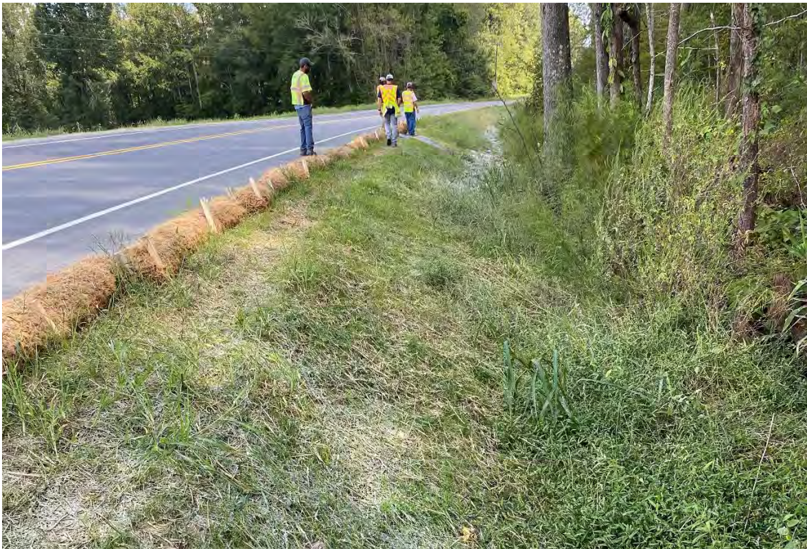
Wattles that were added in preparation for rain event as slope was being stabilized
