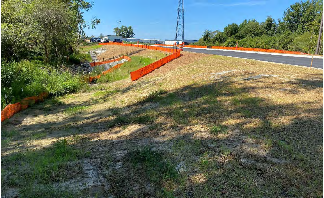
Culvert installed and areas being stabilized
