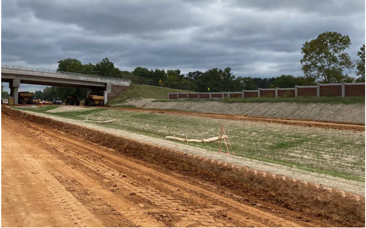
Stabilization of median and slope, with wattle checks installed
