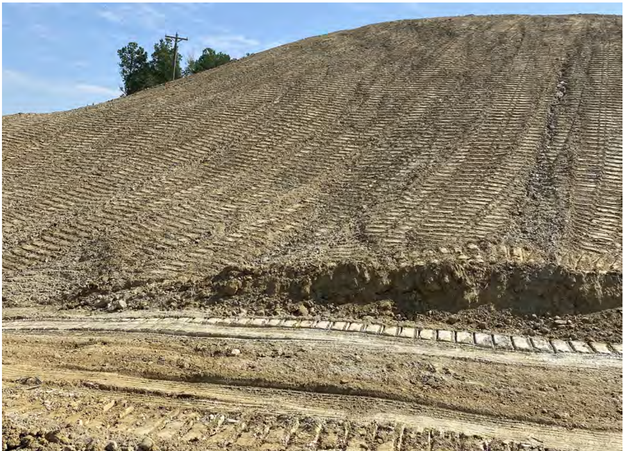
Stockpile on waste site awaiting stabilization
