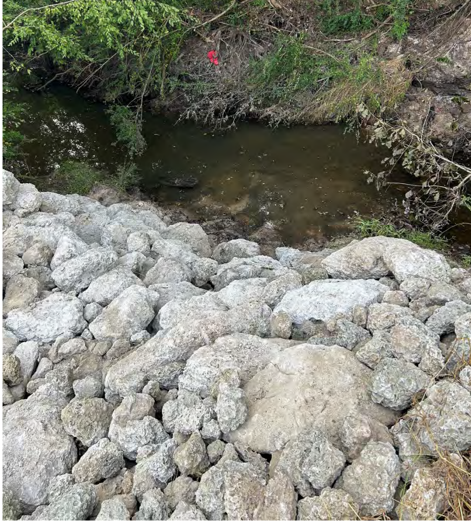
Sediment loss retrieved and ditch with check dam repaired (9/25/2023)
