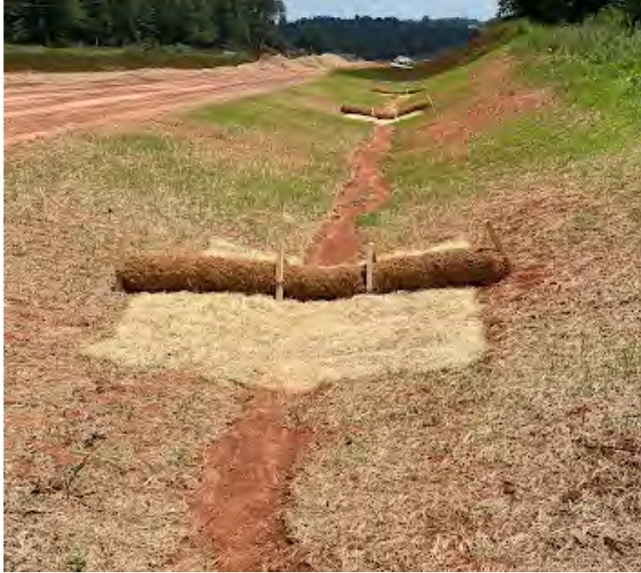
Wattles with PAM installed
