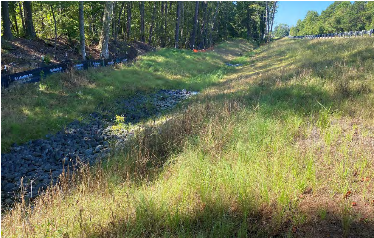
Stabilized ditch adjacent to detour bridge
