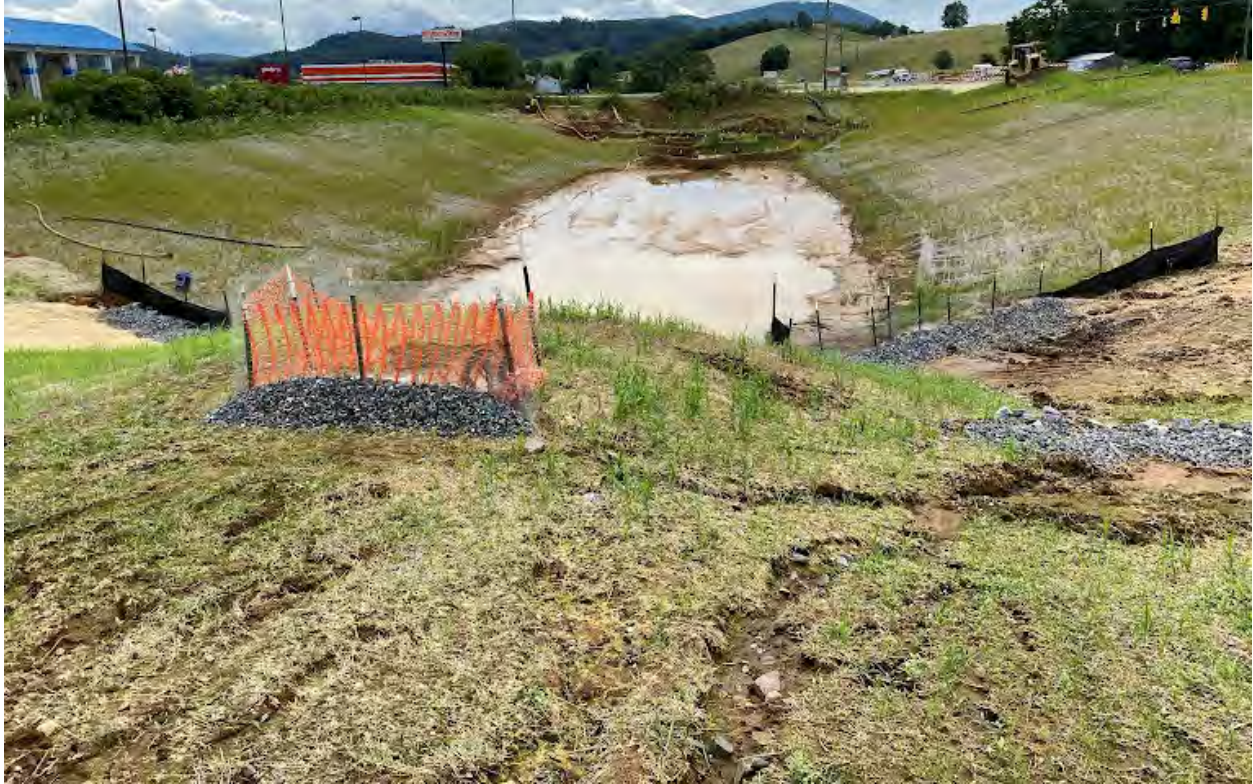
Basin being converted to permanent stormwater measure
