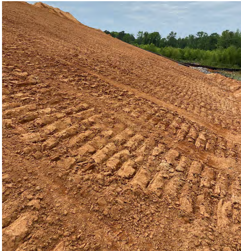
Recently graded slopes tracked properly
