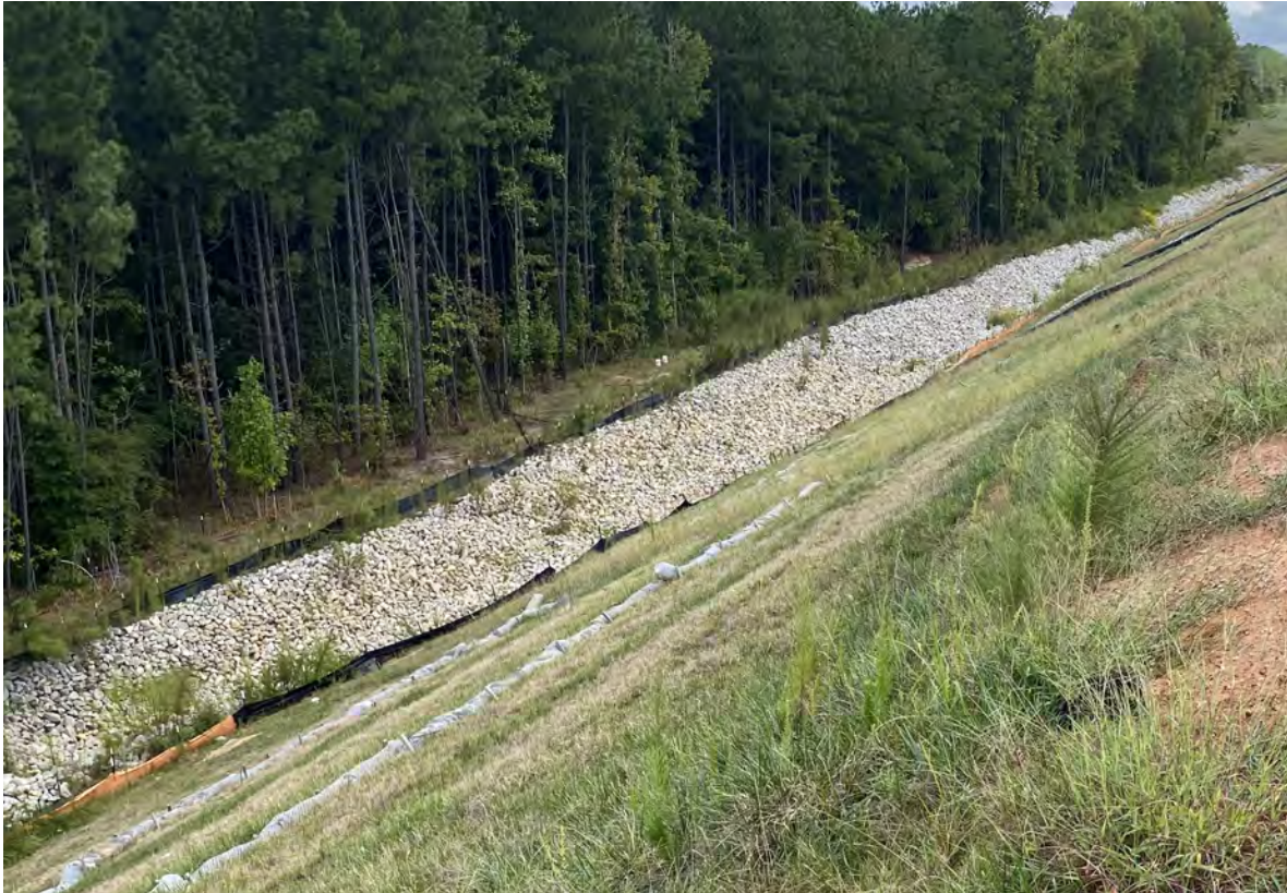
Completed slope and channel change
