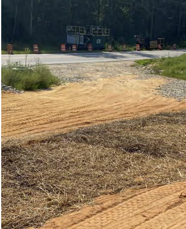
Construction entrances needing maintenance
