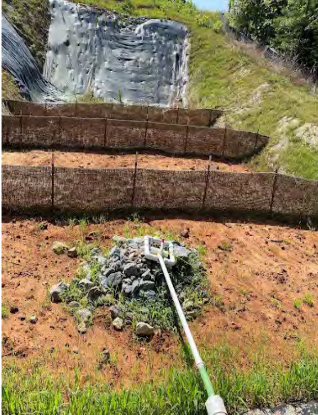
Skimmer basin and outlet pipe
