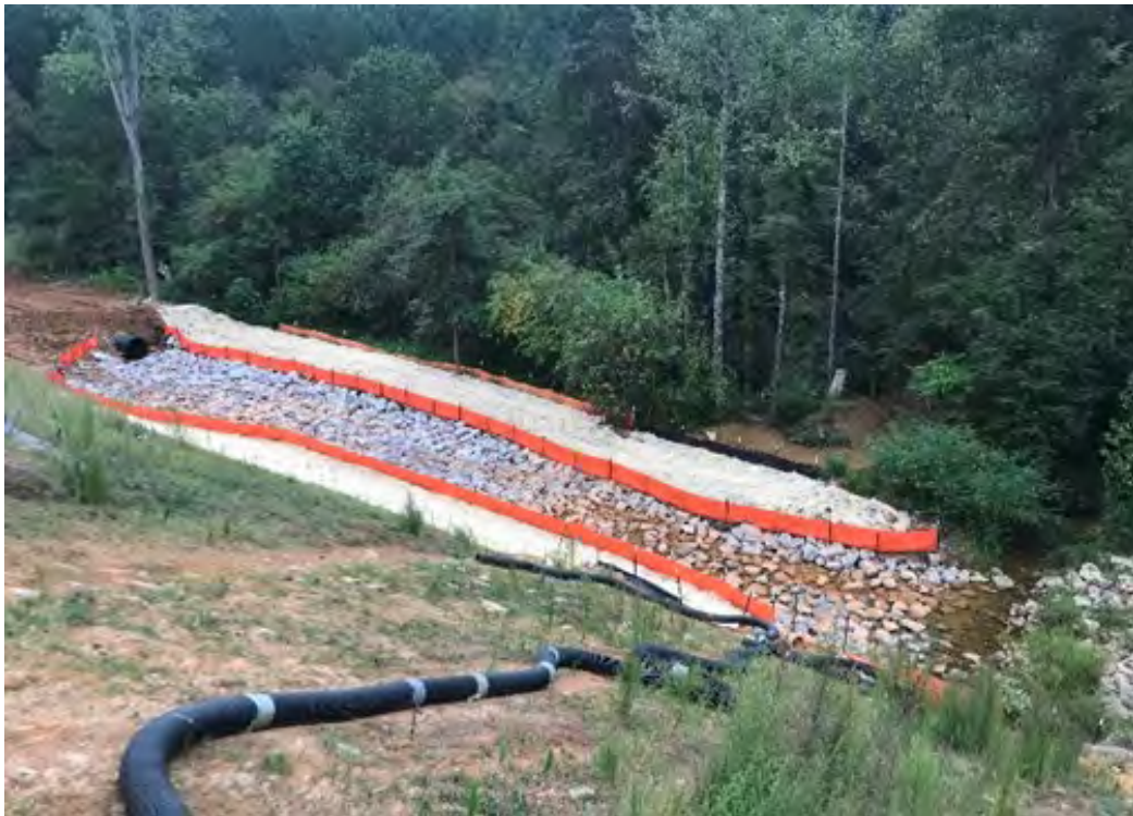
Channel repaired and stabilized (9/29/23 follow up)
