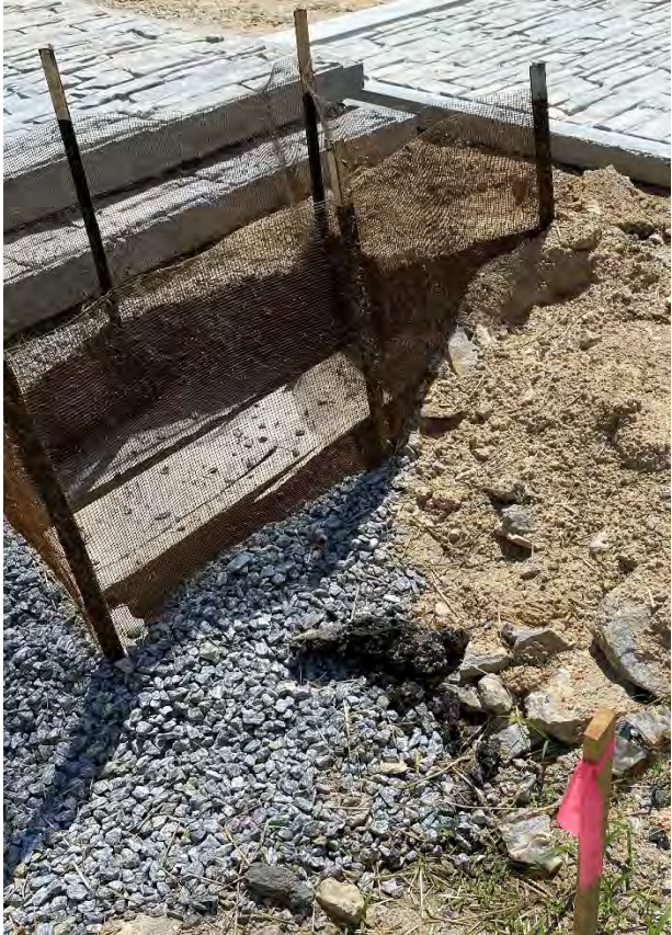
Drop inlet protection measure needing maintenance
