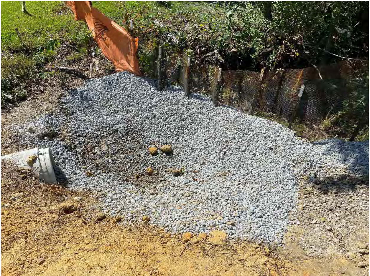
Silt fence outlets maintained
