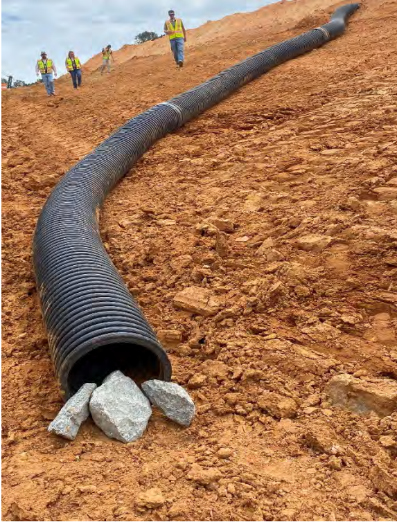
Slope drains needing to be staked down (both) and an outlet protection measure needed (left)
