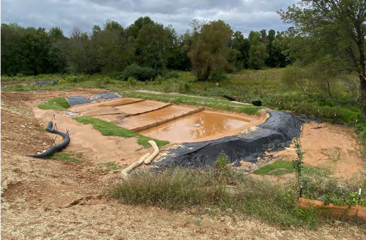
Basin west of Swift Creek
