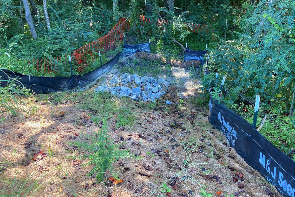
Maintained and stabilized outlet
