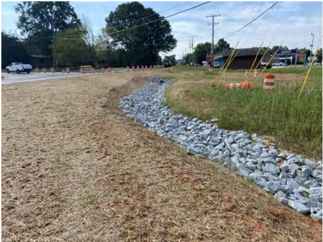
Permanent ditch completed and area being stabilized
