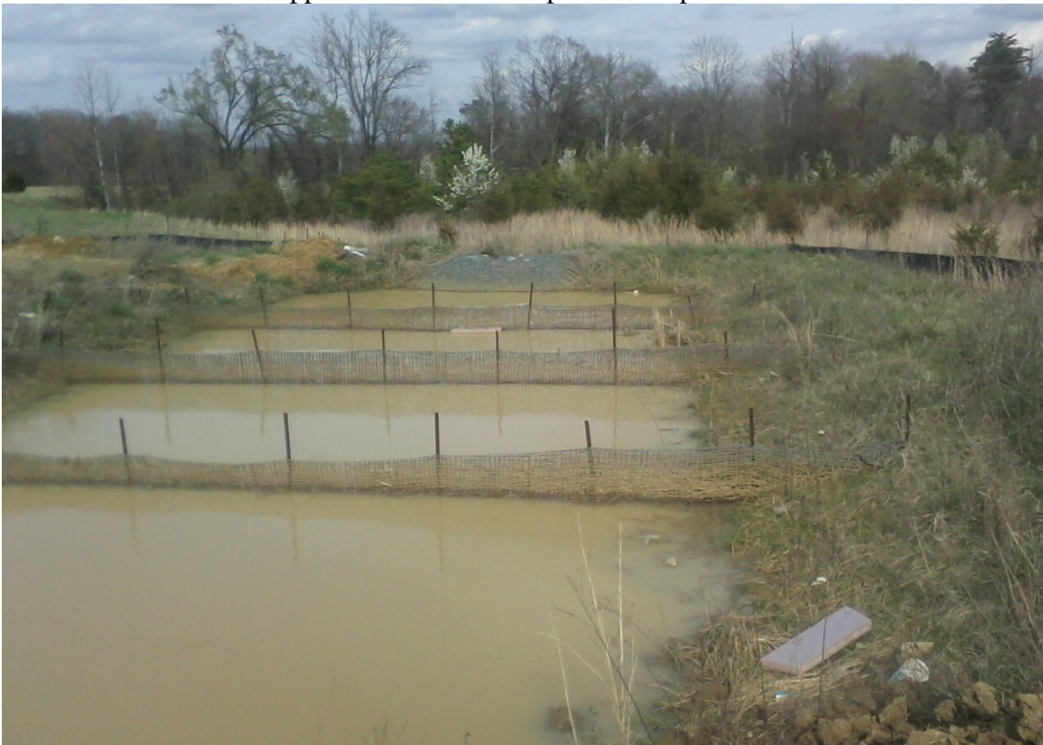
Site 4 – Temporary Sediment Trap sized for 3.3 acres.
