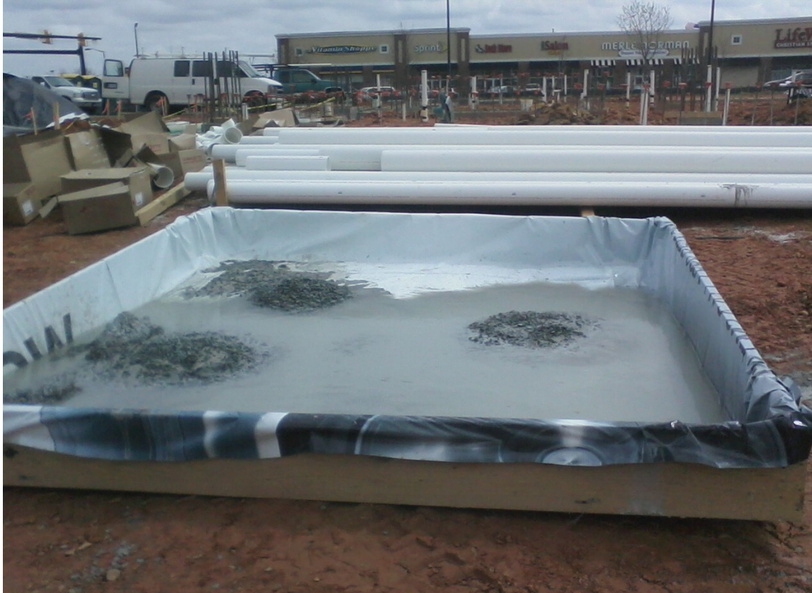
Site 1 – Innovative concrete washout area – 2x10s, plywood, and billboard paneling.
