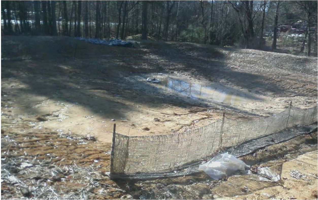
Site 1 – Sediment Basin
