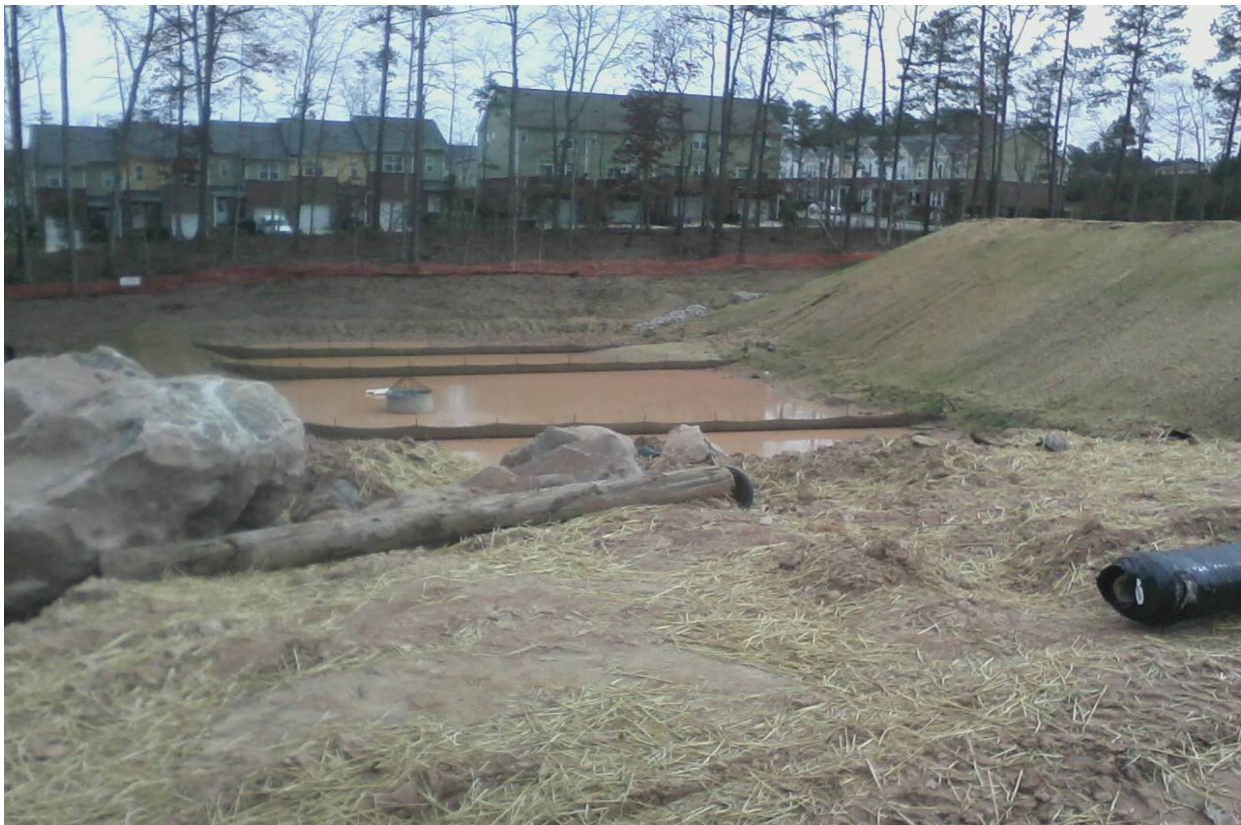
Site 2 – Temporary Skimmer Sediment Basin
