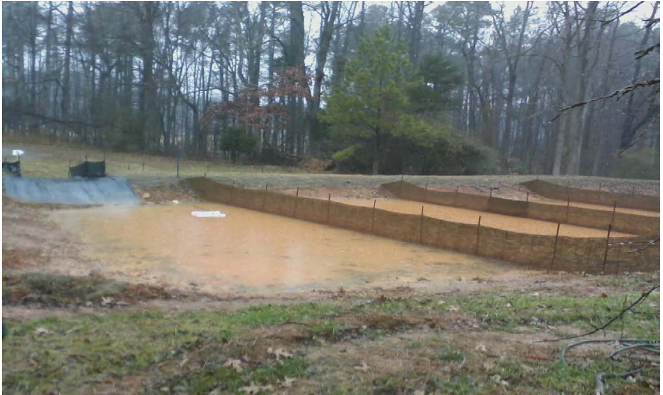
Site 1 – Sediment Basin
