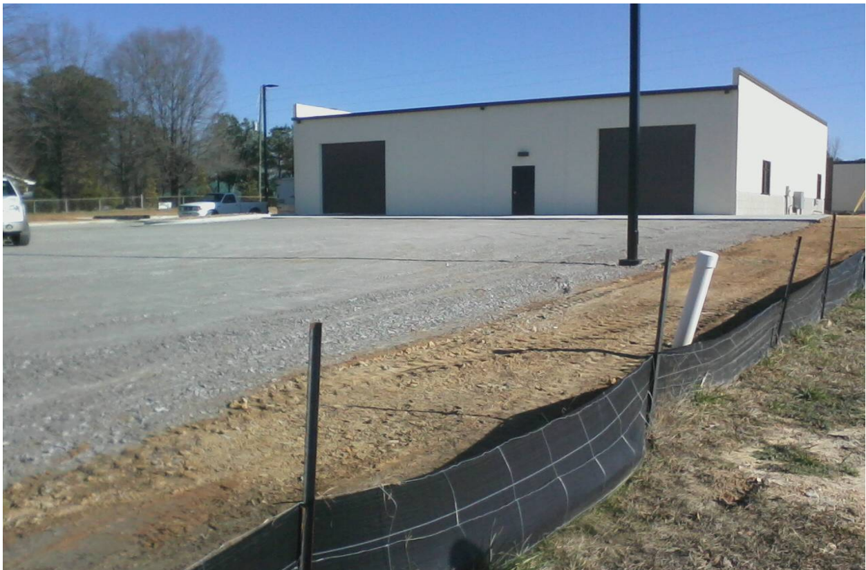
Site 2 – Final site preparation underway with ABC stone and seedbed preparation.
