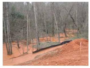
Fig. 3 Second place. Overload of sediment causes silt fence failure and fill in stream.
