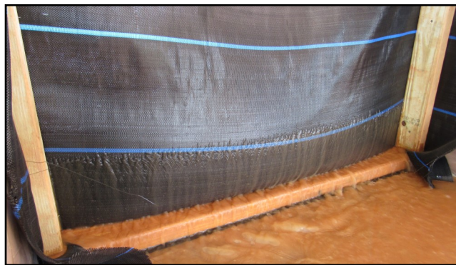
Example of flow through silt fence material in the test system devised by Whitman et al. Photo courtesy of Dr. Blake Whitman
