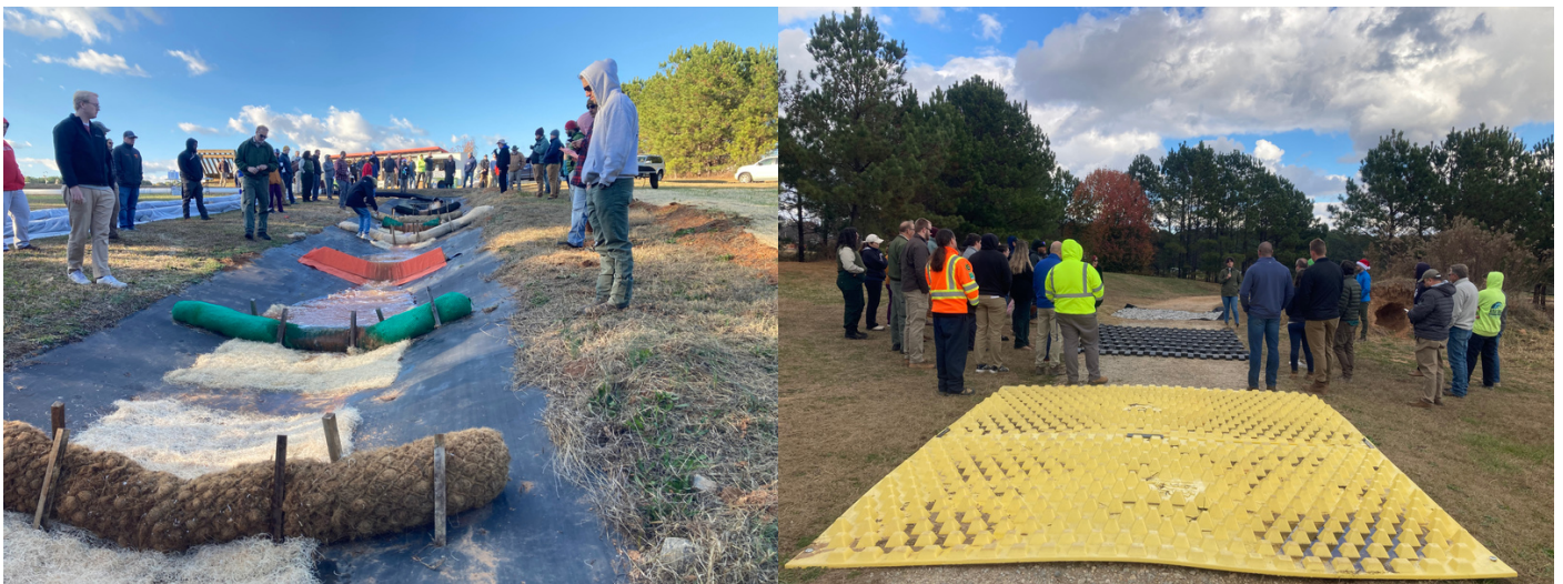
Pictured on the left is the wattle and check dam demonstration, and on the right are tree types of construction entrances: FODS trackout control mat, Rubberform trackout control mat, and gravel construction entrance. Photo Credit: Rebecca Coppa, NCDEQ
