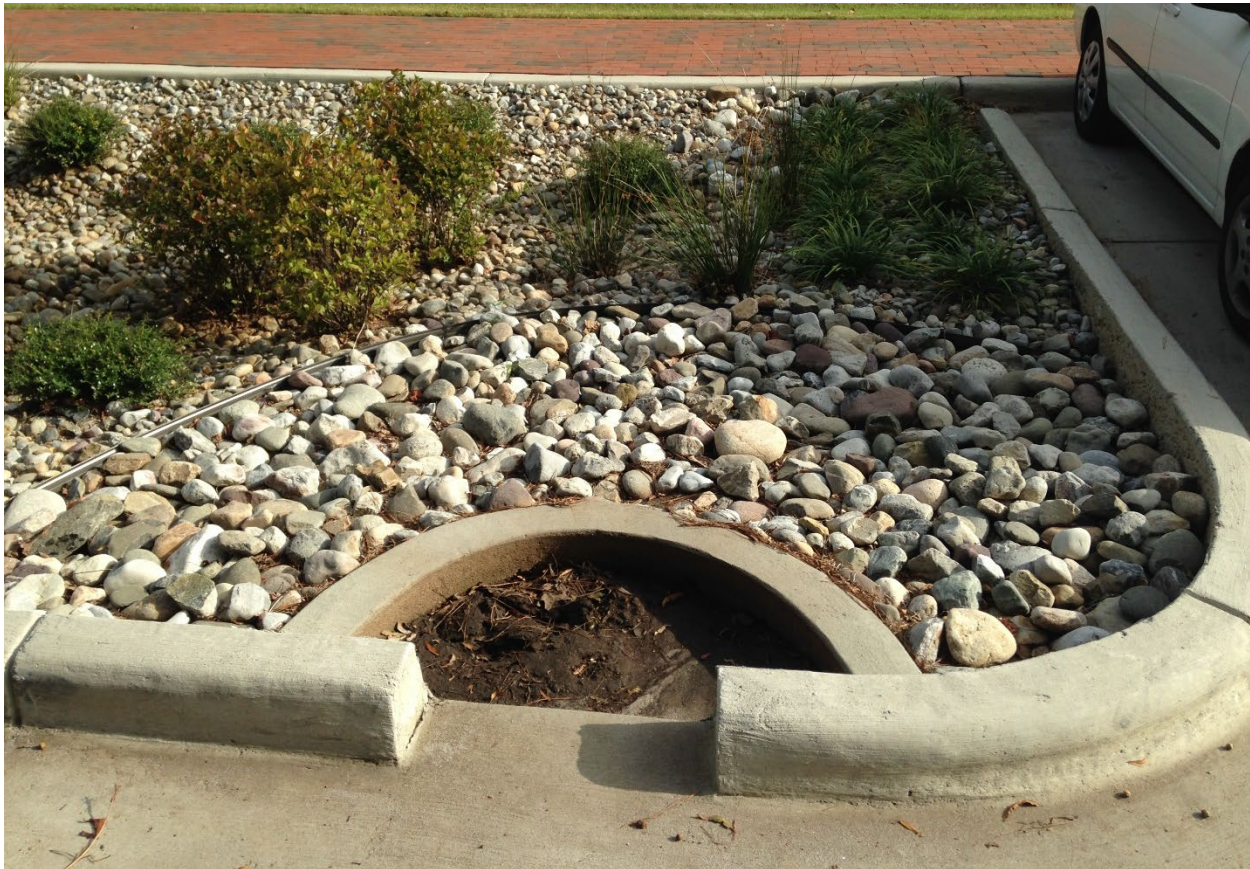
Figure 4: Example of Concrete-Lined Bioretention Forebay
