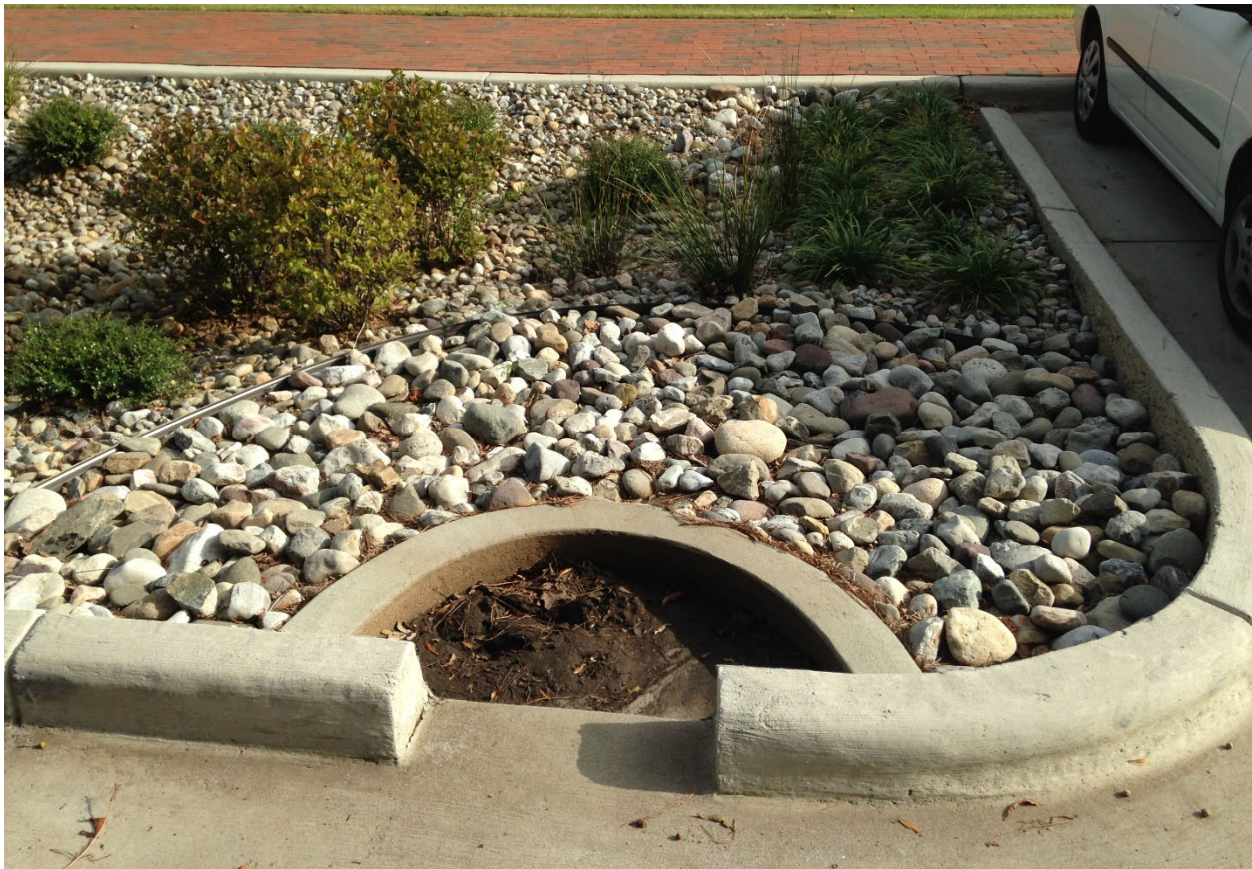
Figure 4: Example of Concrete-Lined Bioretention Forebay
