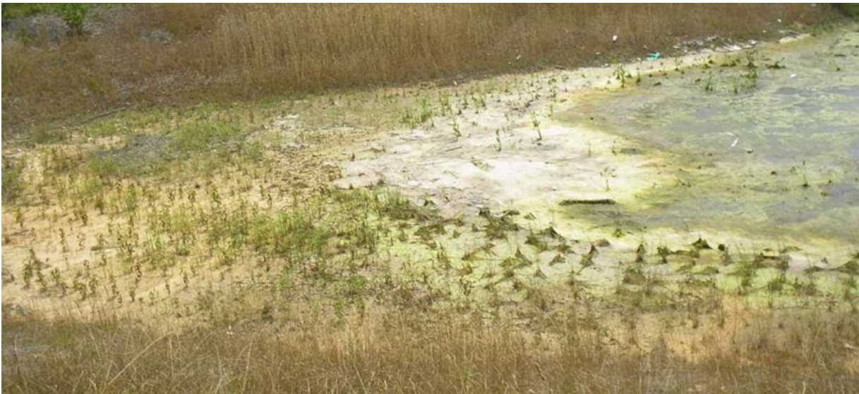
Figure 6: Stormwater Wetland Impacted by Infiltration
