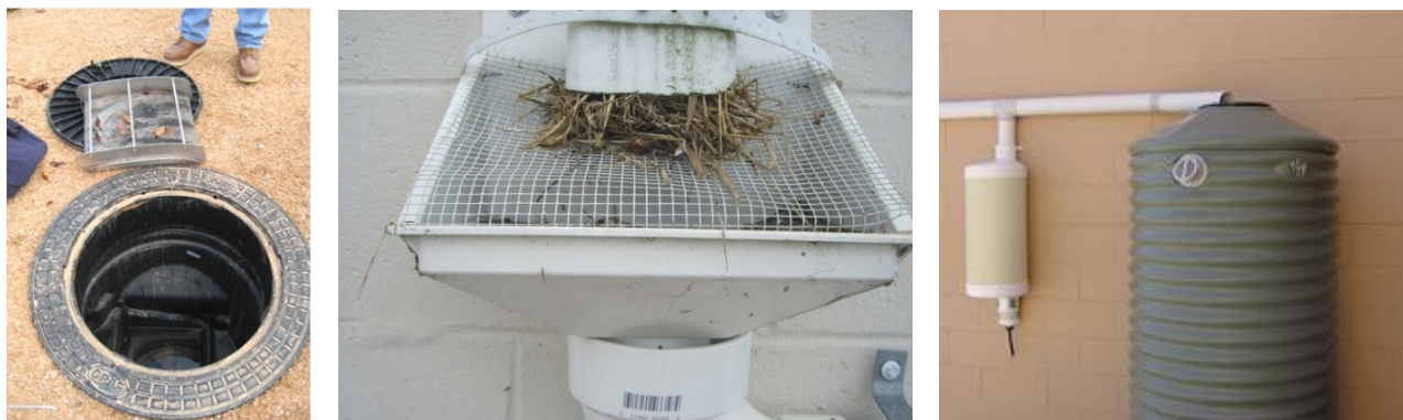
Figure 2. Fine filter used upstream of an underground cistern (left), gutter screen (center), downspout screen (right) (NCSU BAE left and center and UNC-CH right).
